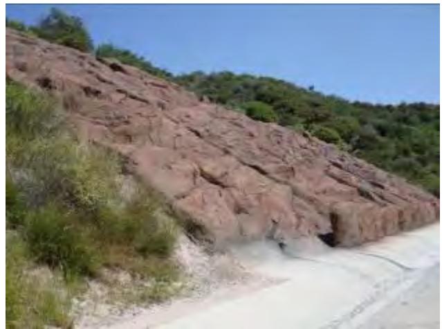
Figure 2 and 3: Naturalized concrete slope above the reservoir. Construction (left) and finished slope (right).
