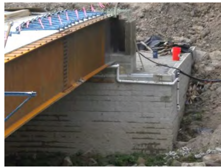
d) steel girders set on GRS abutment
