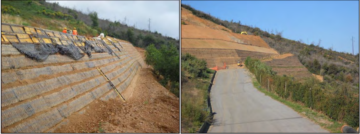
a) toe of the reinforced earth structures
