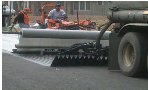
Fig. 3 Paving Mat Installation the fabric
