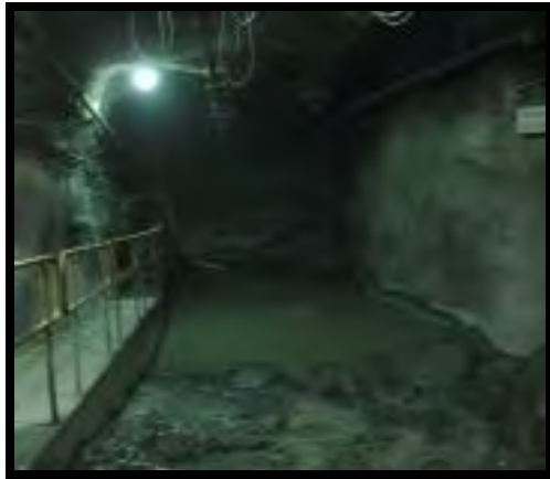
Picture 2 : Sump collecting Mine Water
