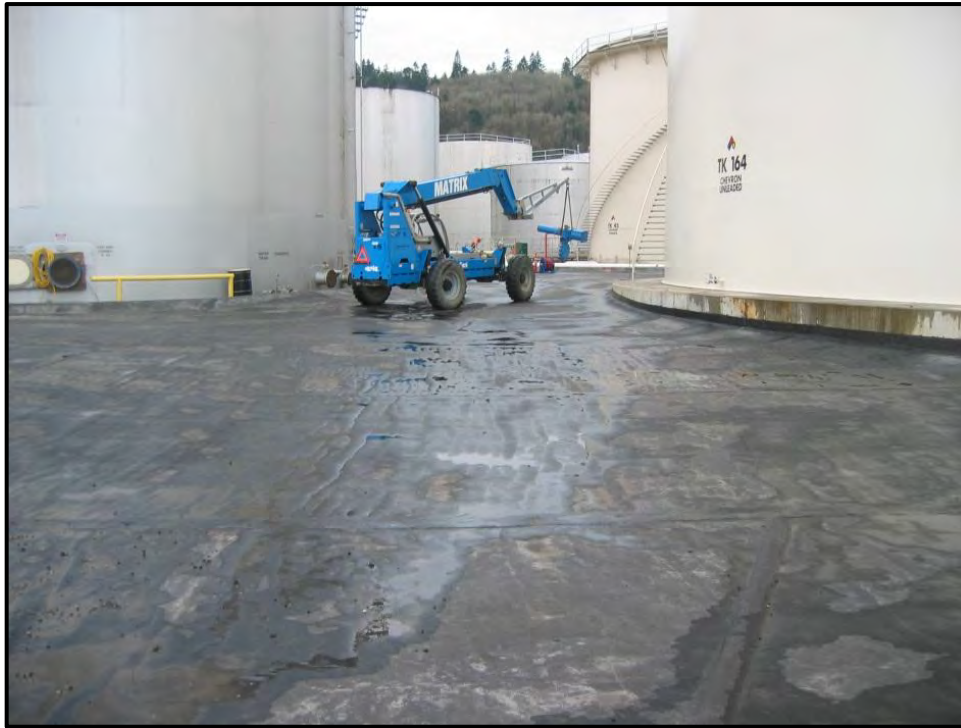
Figure 5: Vehicular Traffic on Top of Bituminous Geomembrane
