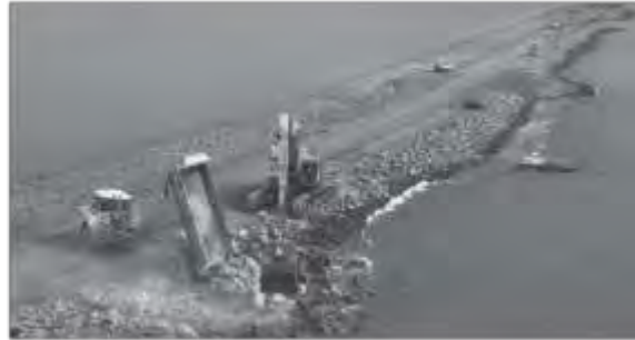
c) Placement of rock armour
