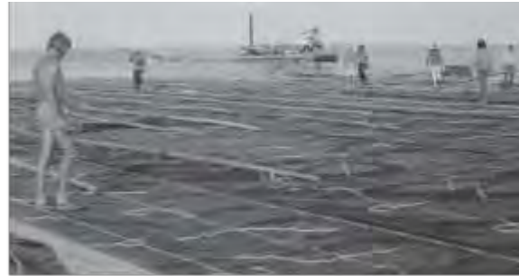
b) Fabrication of fascine mattress on land
