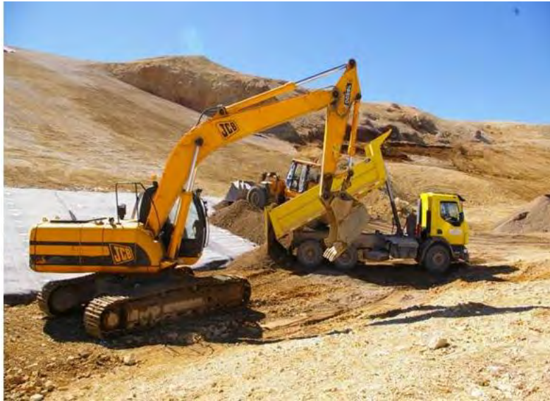
Figure 9: Placement of sand and gravel cover
