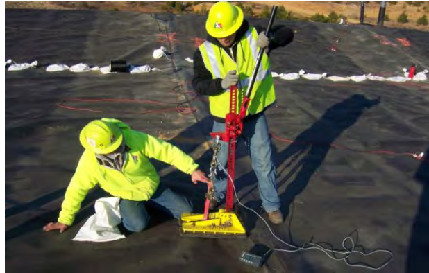
Figure 3. The anchor installation requires only a small penetration of the membrane. Lightweight, common equipment is used to drive the corrosion-resistant anchors.
