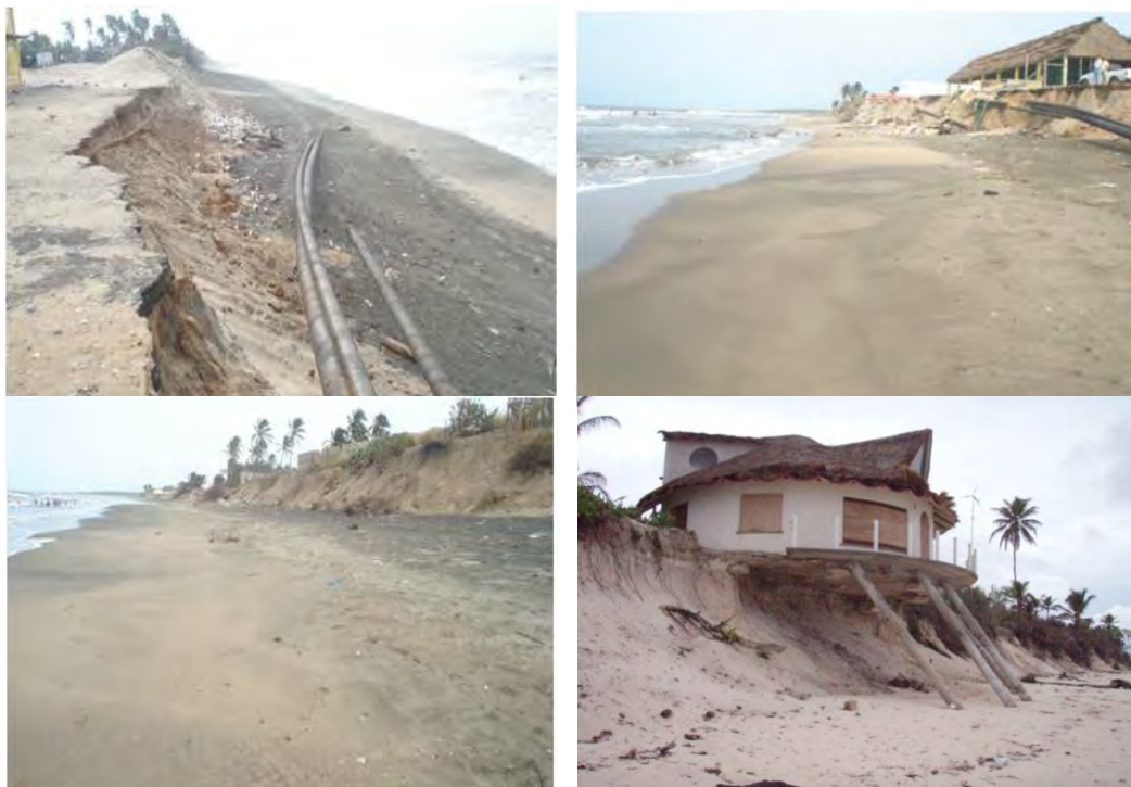
Figure 2. Heavy damage by erosion from the Cold Front #4 October 2007
