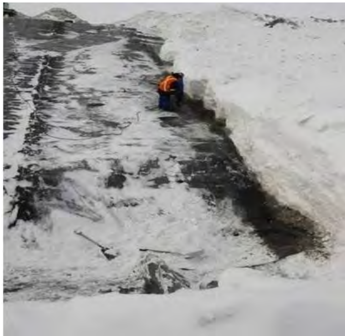
Figure 3: Snow clearing during bituminous geomembrane liner installation in Pond 2
