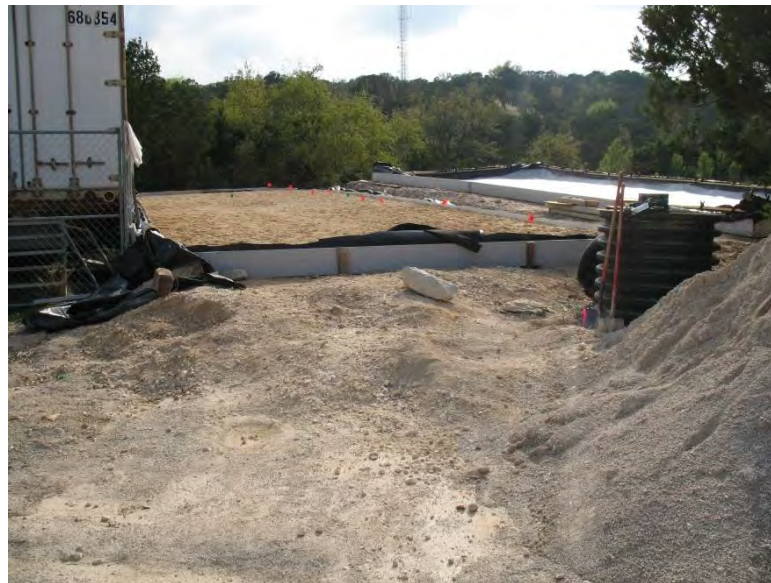
Figure 2. Soil-covered liner test cell with calibration/sensitivity test flags.
