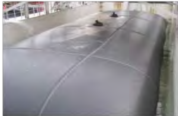
d) Filled geotextile container in installation barge
