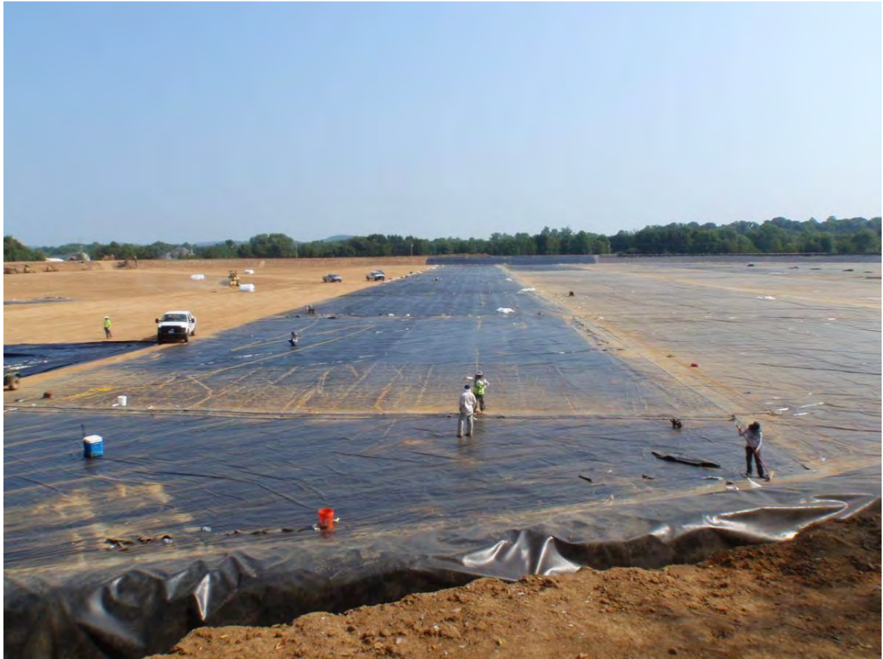
Figure 4: Geomembrane liner installation
