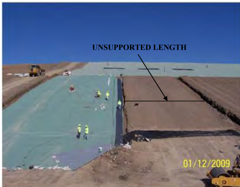
Figure 10. Example of exposed geomembrane anchorage (Courtesy of K. Perera, HDR)
