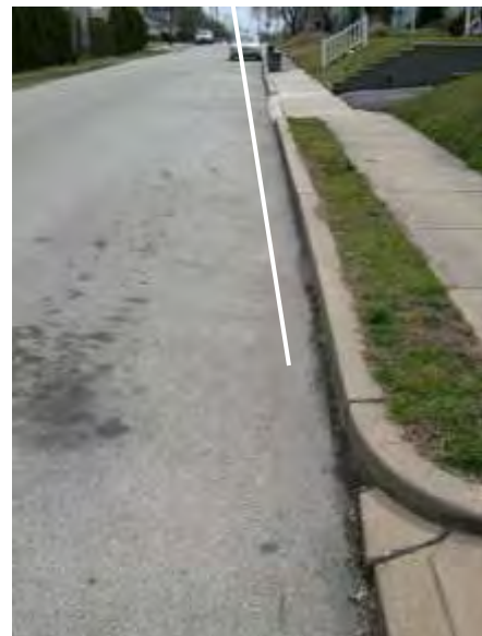
Figure 13. Longitudinal pavement cracking on unrestrained (left) pavement edge and none on curb retained (right) pavement edge.
