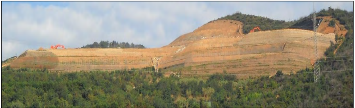
Figure 7. Front photography; slope at the end of construction
