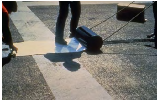
Fig. 5 Strip membrane over a joint before overlay
