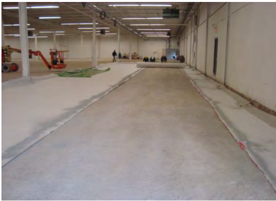
Figure 10. GCL being deployed inside a new production plant facility – lining underneath new machinery – Liquid Spills from equipment above (machine/equipment not shown).
