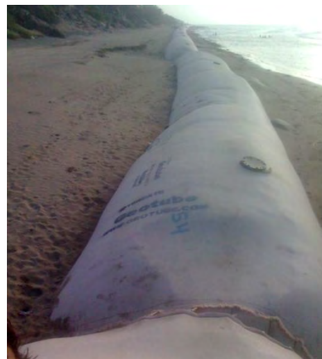
Fig. 11 Retention of sand behind the protection line with Geotube® Technology
