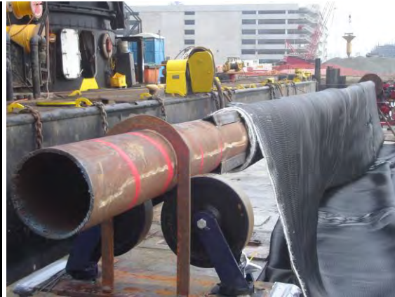
Figure 4. Roller on Barge with Panel.
