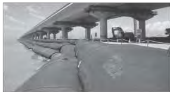
e) Construction of viaduct
