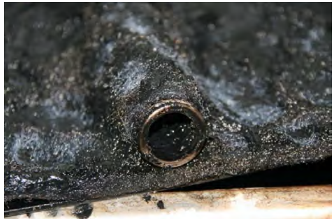
Figure 10. Side view of the geocomposite in cell 4 (type A).
