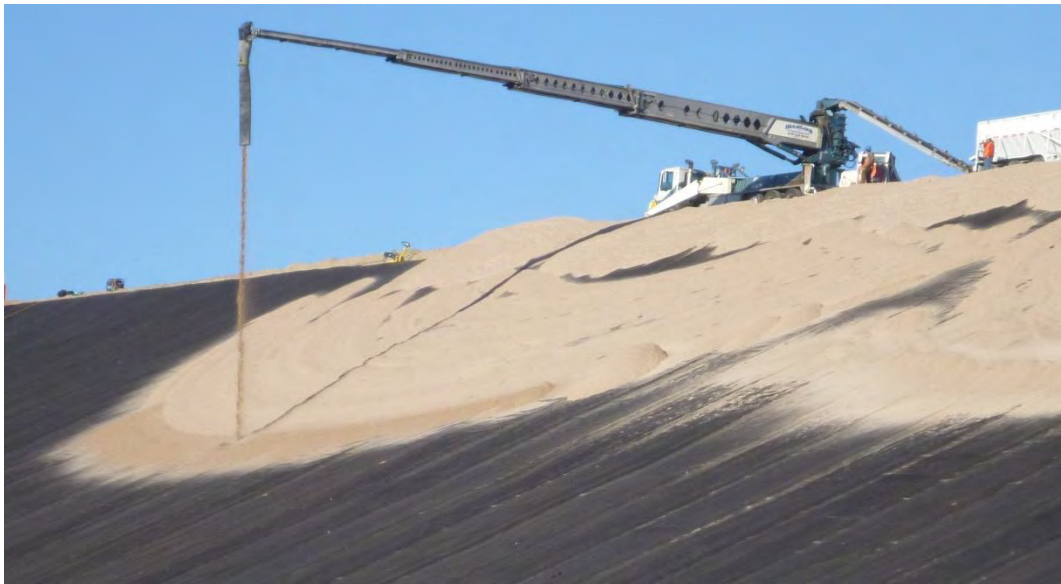
Figure 4. Telebelt spreading sand over the geonet. (Courtesy of Jack Gagliardi)
