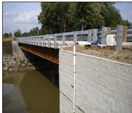
b) constructed bridge in Ohio
