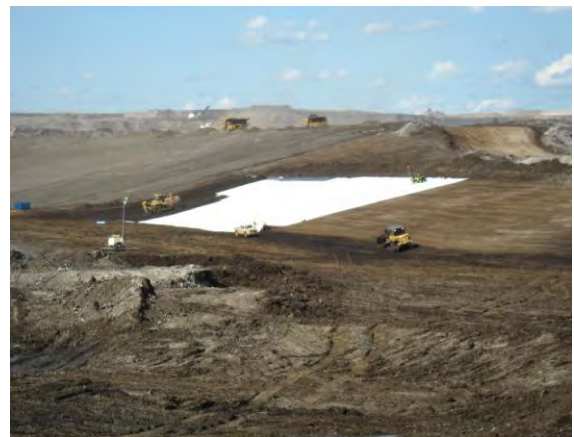
Figure 7. GCL being deployed in a dam lining application (Mining industry).
