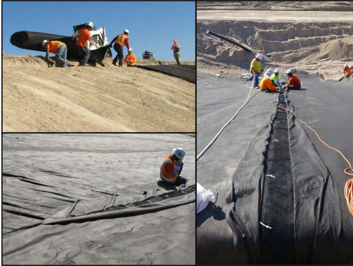
Figure 5. Shows sequencing of installation of geonet composite rolls.
