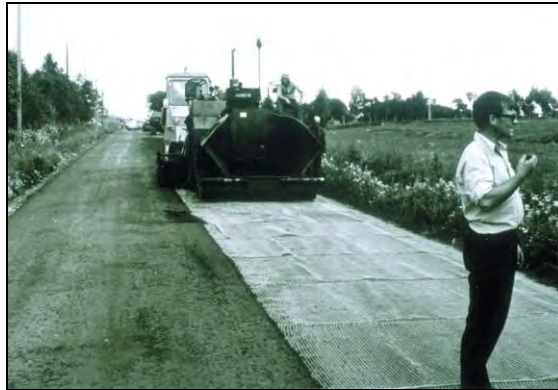
Figure 1. One of the first attempts to use a Geogrid in asphalt pavements at the early 1970s.
