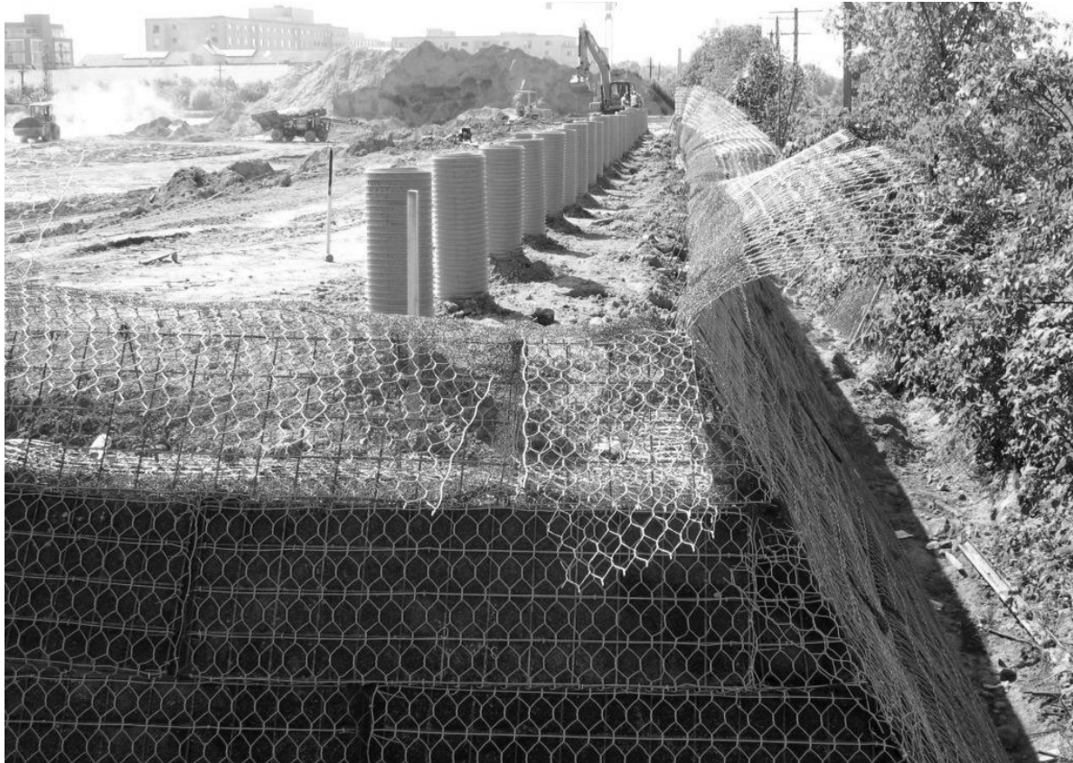
Figure 5. Circular forms for wooden fence
