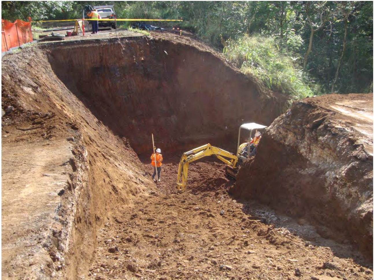
Photograph 2. Site 1 Excavation, Total Depth of 6.1 meters.
