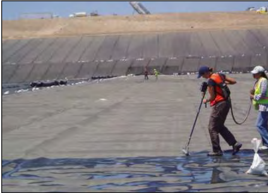
Figure 5: ASTM D7002 Leak Detection Testing
