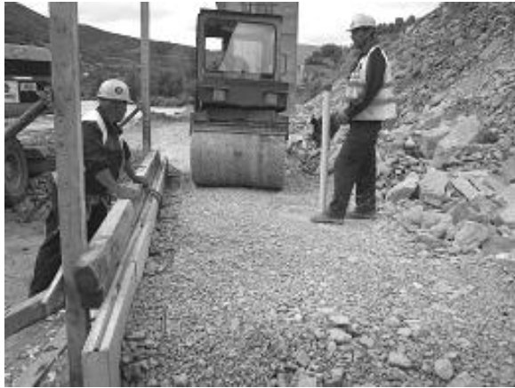
Figure 3. Compaction of backfill material
