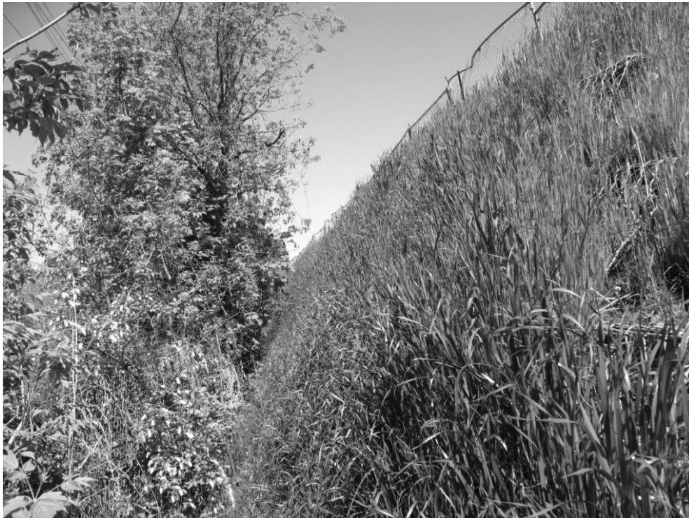
Figure 4. Reinforced slope after 6 months
