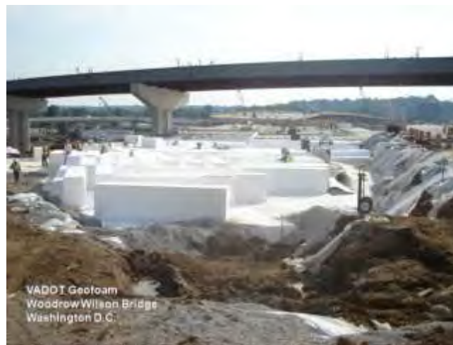
Figure 6 – Rt. #1 bridge approach in Washington, DC (Courtesy of InterGEO Services).
