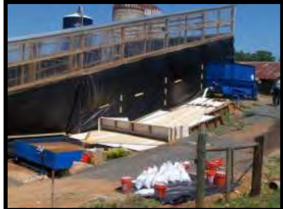
Figure 25 - ASTM D 7351 SRD Testing
