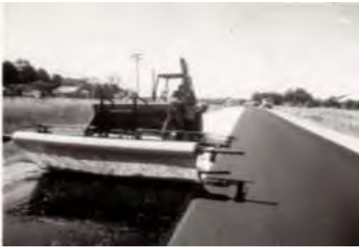
(c) Geotextile being placed by mechanical equipment
