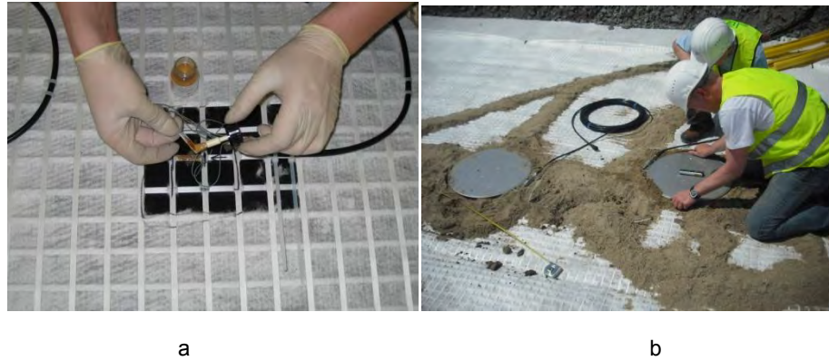
Figure 6 - Application of strain gauges (a) and pressure cells (b) on geocomposite
