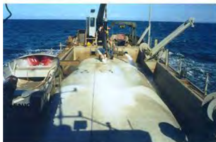
b) Geotextile containers for removal of harbor sediment (compl. TenCate)
