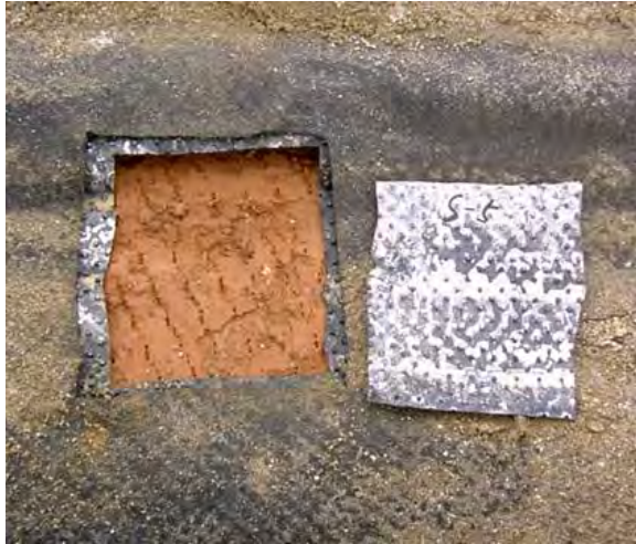
a Markings under Sample Taken at the Toe of the Slope
