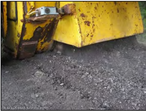
Figure 8. Milling the asphalt including the reinforcement
