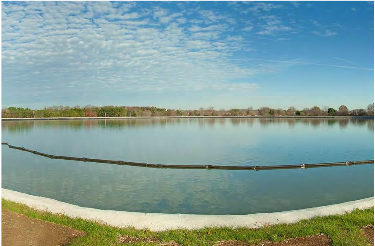
Figure 6: Completed reservoir rehabilitation shown now full of water
