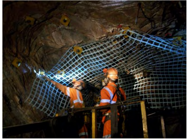
b) Manual installation.
