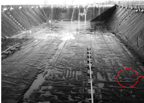
Photo 5. Position of test hole.
