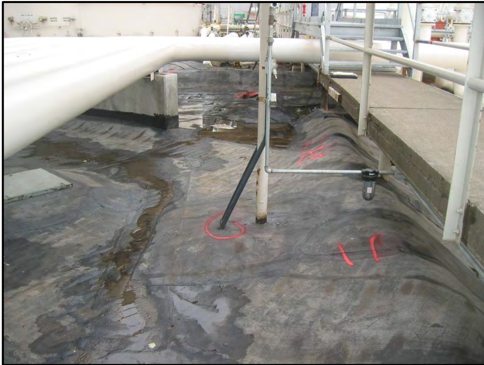
Figure 7: Geomembrane under pipes and around penetrations
