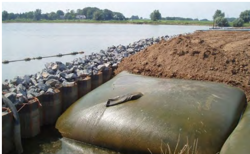
Figure 9. Backfilling over dewatered and stabilized geotextile tube.
