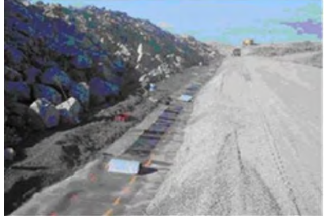
Figure 6: Flam Stick attached to HDPE
