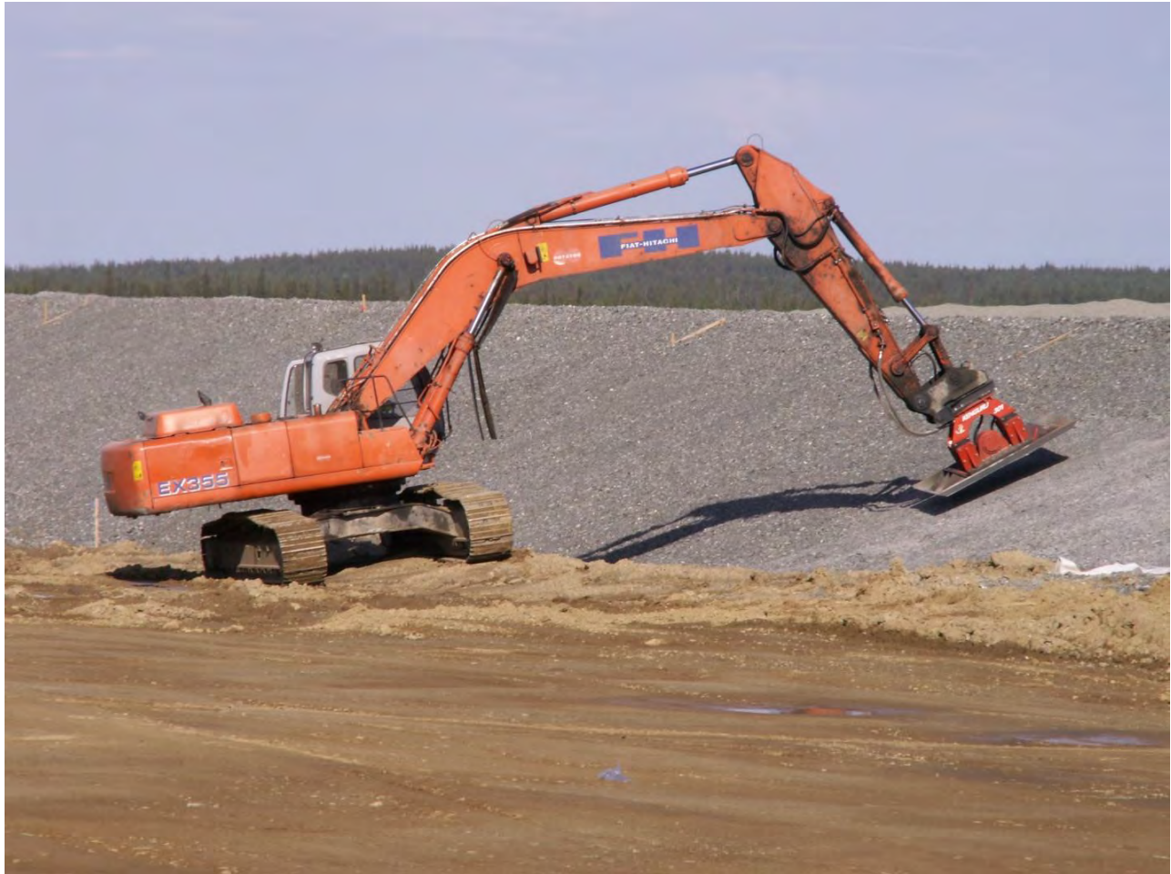
Figure 5: Compaction of side slopes
