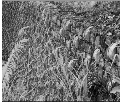
Figure 2. Reinforced Soil in Malaysia (1979).
