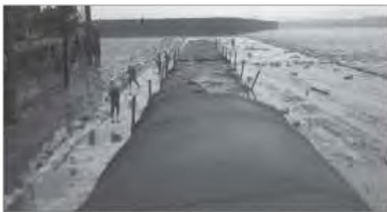
b) Installing initial geotextile tube
