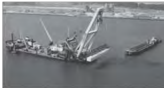
c) Installation of the prefabricated facing and reinforcement under water
