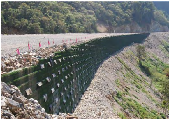
Completed permanent geosynthetic wrapped face MSERW.
