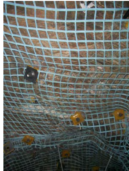
d) Geogrid installed and details of plates and its spacing.
