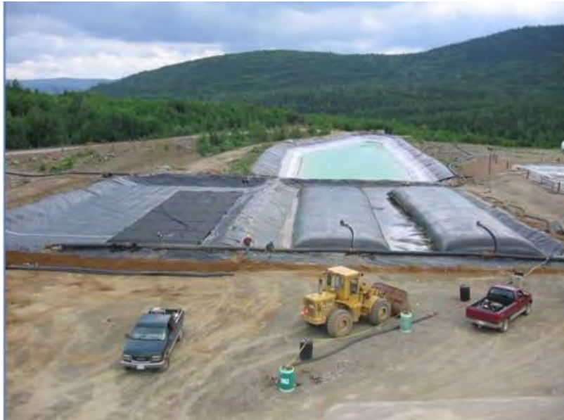
Figure 2. Geotextile containers inside dewatering cell
