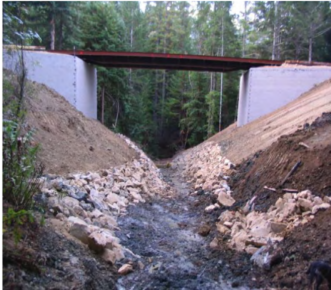
Figure 10. Completed railcar bridge.
