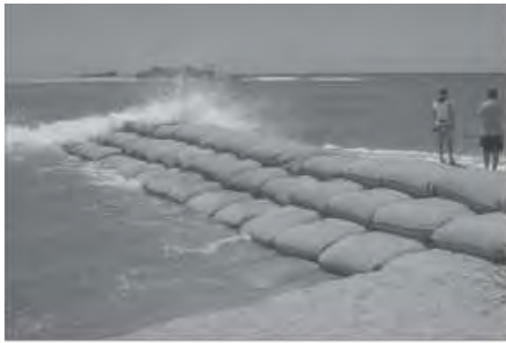
a) Geotextile bags
