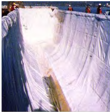
a) Large geotextile bags for coastal erosion control (compl. NAUE).
