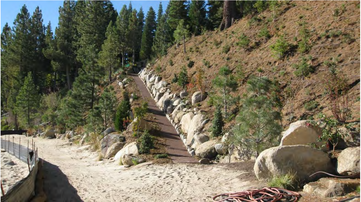
Figure 7 - Path surface and planting complete, irrigation is 80% complete.
