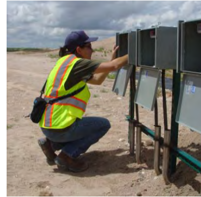
b) monitoring station at crest of slope
