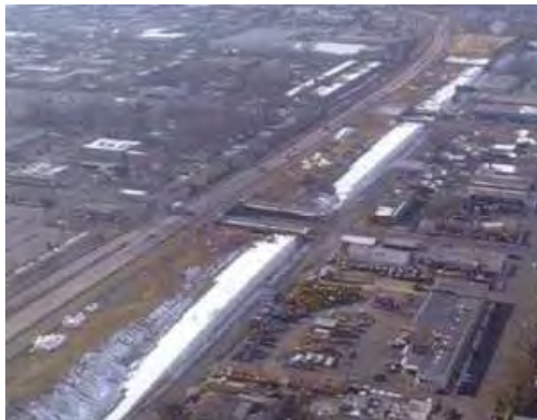
Figure 5 – I-15 lightweight fill project in Salt Lake City, Utah.
