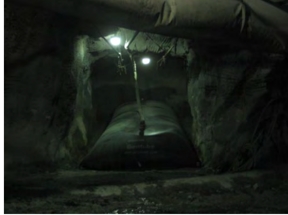
Picture 7: Geotextile tube in a gallery
