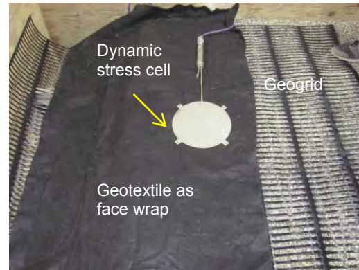
Figure 6. Dynamic soil stress cell and geosynthetics
