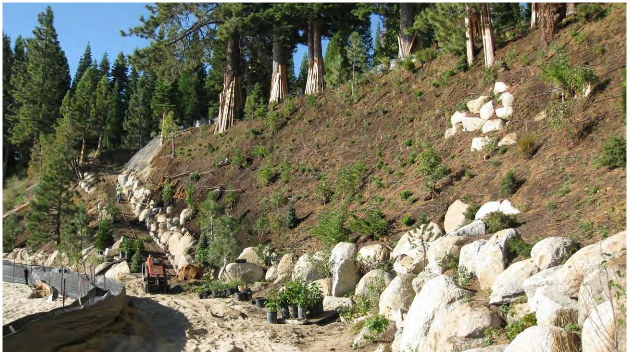
Figure 8 - Planting is 90% complete and path surface installation has started.
