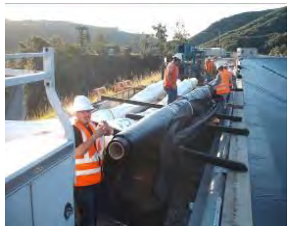
Figure 8: Installing a 35-ft-wide fabricated panel.
