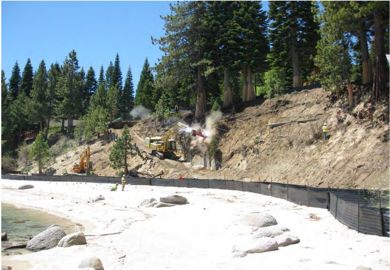
Figure 1 - Installation of Ballistic Soil Nails
