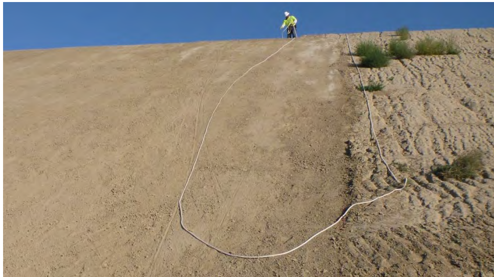
Figure 3. Approved and unapproved subgrade below geonet. (Courtesy of Jack Gagliardi)
