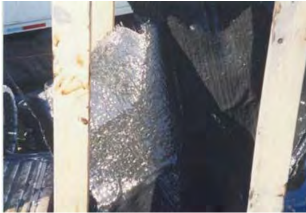
a) Filter cake buildup of sediment fines inside fabric bag enclosure
