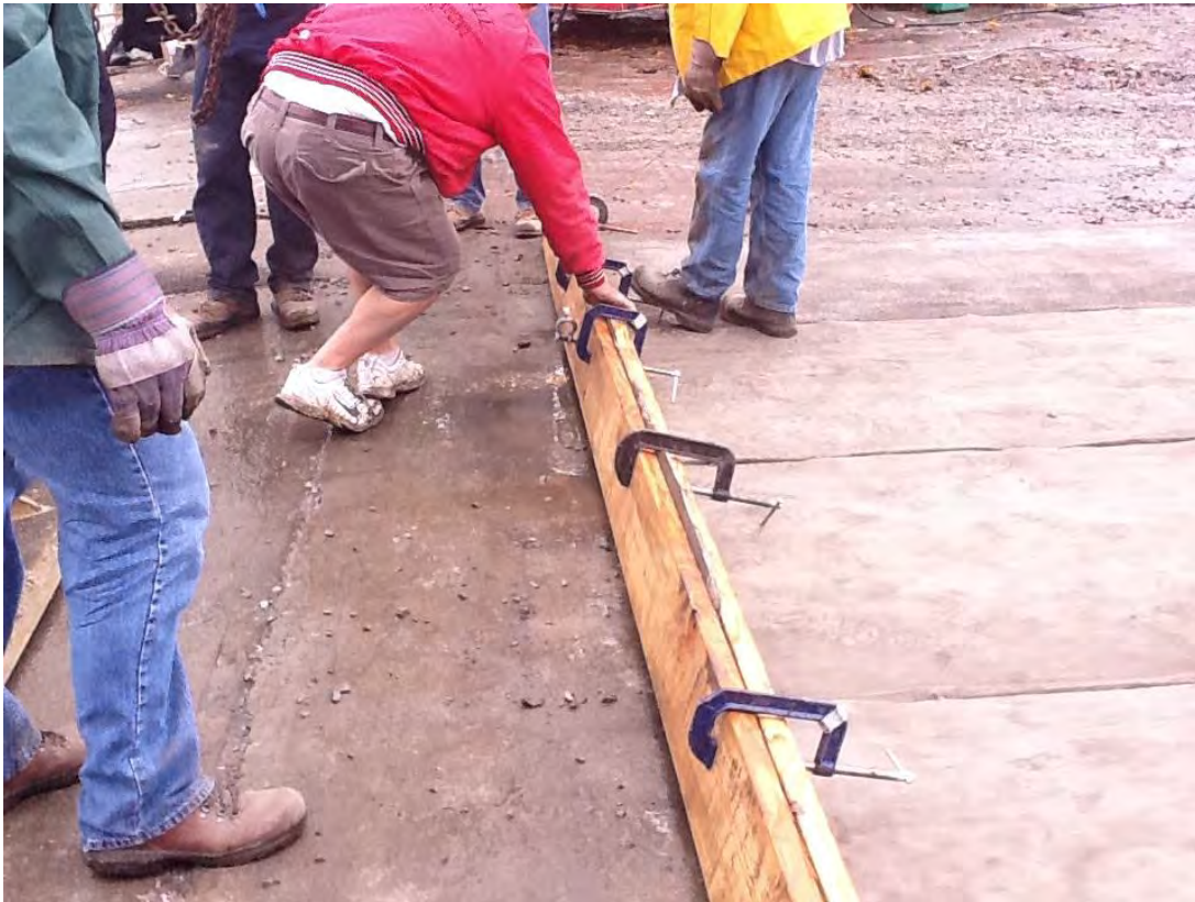
Figure 3 – Leading Edge Fabrication Concrete Cloth Composite
