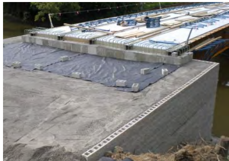
e) constructed GRS approach
