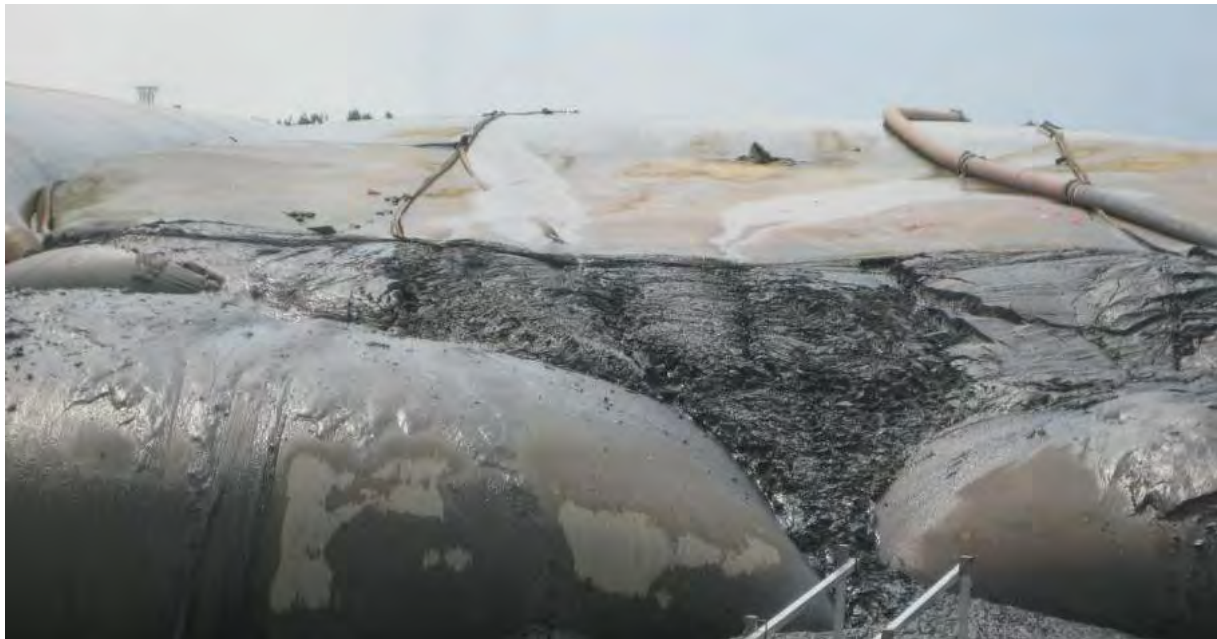
Figure 8. Example stacked tube configuration.
