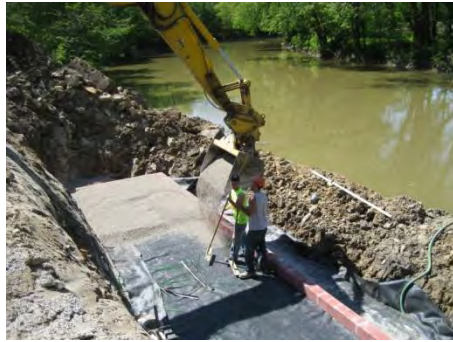
a) GRS abutment construction
