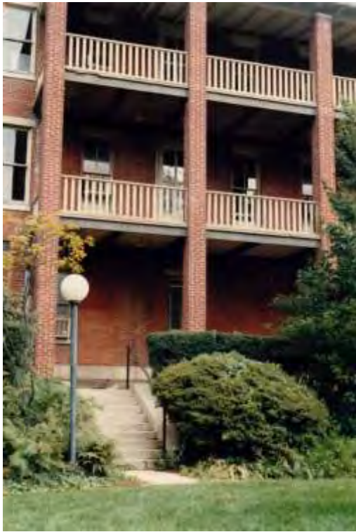
(a) Three floors plus a basement
