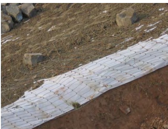
Protection work using Geotextiles and GI wires
