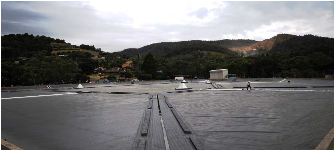
Figure 1: Wattle Park Potable Water Reservoir Floating Cover nearing installation completion stage
