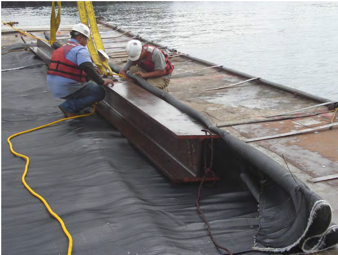
Figure 6. I-beam Attached to Cap Panel.
