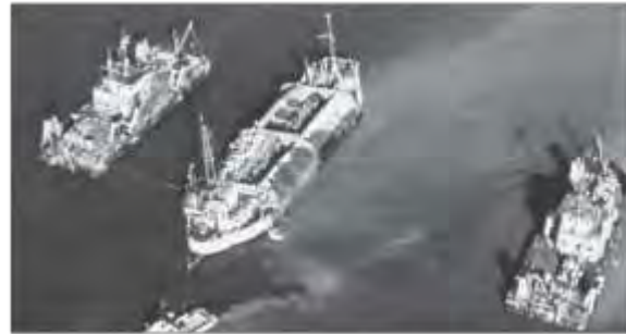
d) Sinking of fascine mattress on the seabed
