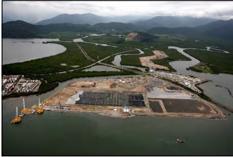
Figure 5 Drainage Layer and Overburden Placement March 2012
