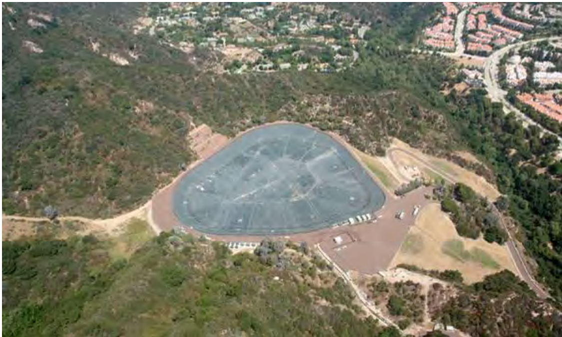
Figure 13: The completed project filled and in service. Note the road colors, rock texture above reservoir, plantings on the slopes below the reservoir, and the mottled color of the floating cover.
