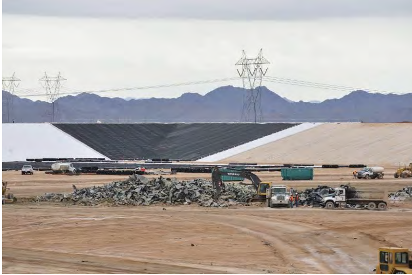
Figure 7. Removal of existing geomembrane material in Pond 2
