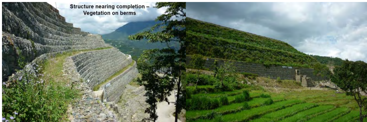
Figure 9. Two finished hybrid MSE structures at Sikkim airport project
