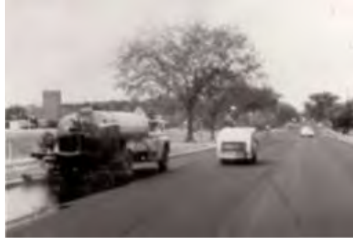
(b) Spraying asphalt-based sealant over existing pavement
