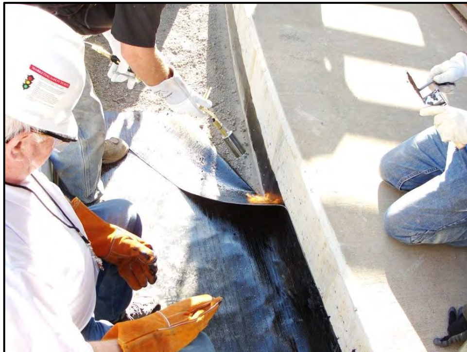
Figure 6: Connection to concrete ring foundation of tank
