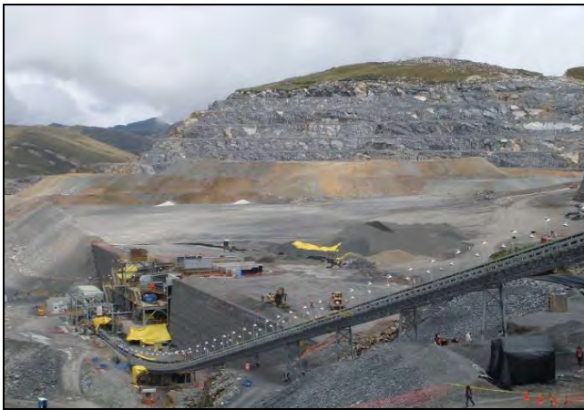
Figure 13. DTSW mesh/ Geosynthetic reinforcement System walls providing access to the primary crusher. Gold Fields ( h_{\max} = 16.50\text{m} - Peru).
