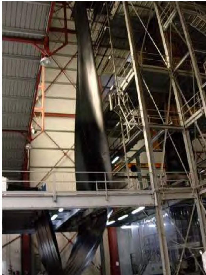
(c) Cylinder coming down from tower
