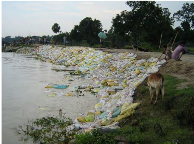
Slope Pitching by sand bags
