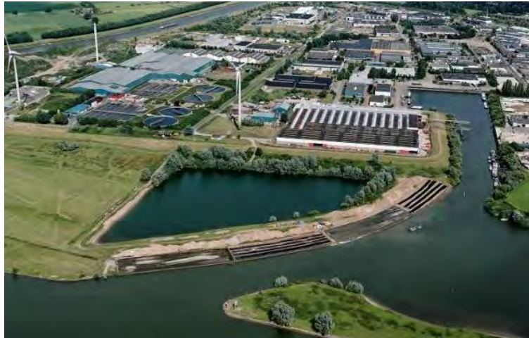
Figure 7. Aerial view of geotextile tube dewatering works along the riverbank.
