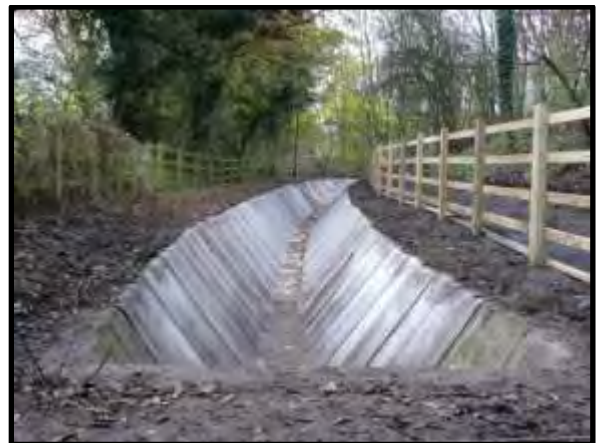
Figure 16 – 3D Cement/Fabric Composite
