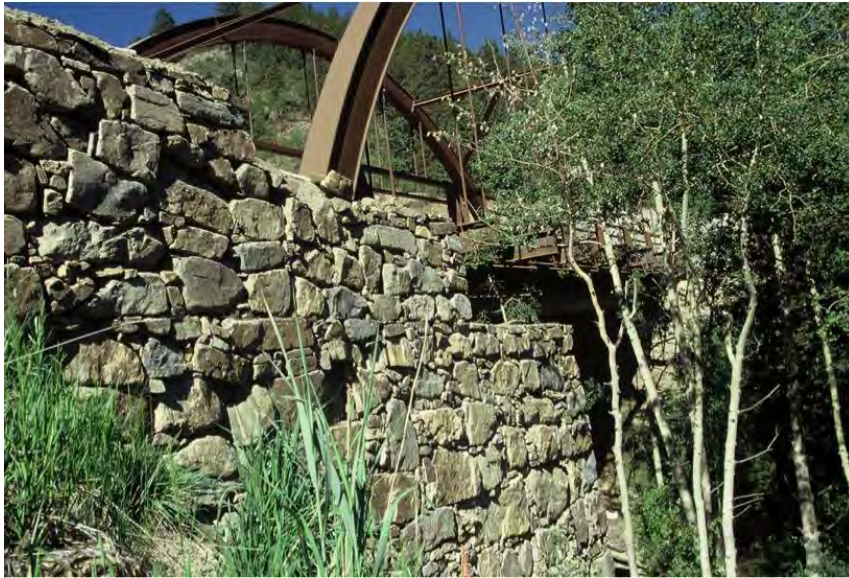
Figure 3. Black Hawk Bridge, with mortared native stone facing.
