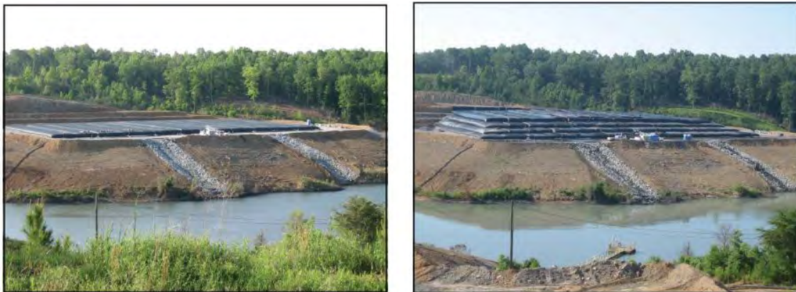
Figure 4. Dewatering cell and stacking progression.
