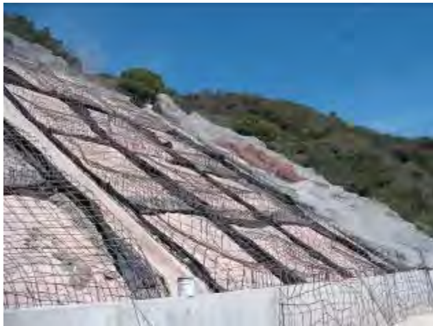
Figure 2 and 3: Naturalized concrete slope above the reservoir. Construction (left) and finished slope (right).
