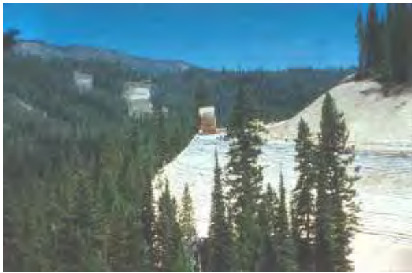
Figure 4. Salmon Lost Trail Pass instrumented reinforced soil slope on Hwy 93, designed by the Western Federal Lands Highway Division (FHWA) using decomposed granite soils.
