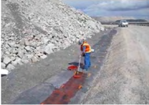
Figure 5: Primer being applied to HDPE
