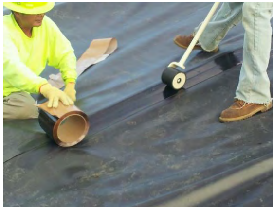
Figure 7. EPDM seaming procedure
