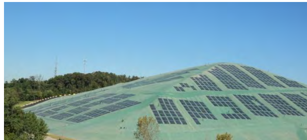
Figure 2. “Solar” exposed geomembrane cap on Hickory Ridge Landfill, Georgia.
