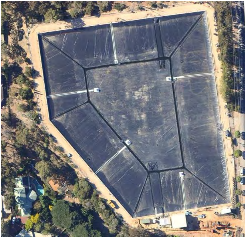
Figure 6: Aerial view of completed Wattle Park Floating Cover System
