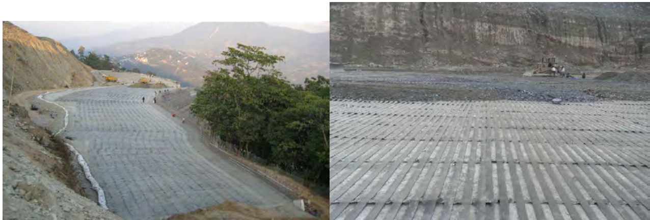
Figure 8. Geogrids installation at Sikkim airport project
