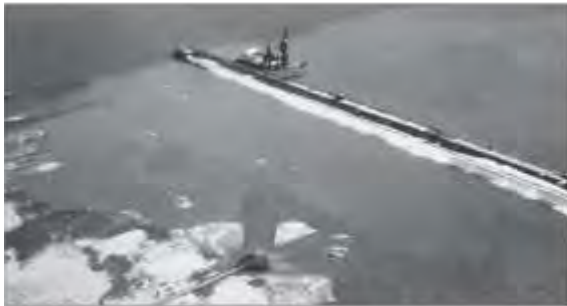
b) Placement of basal reinforcement and sand-fill
