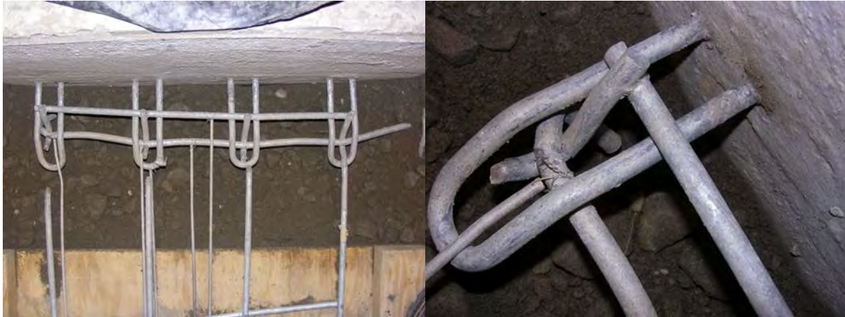
Figure 7. Photos of excavated Loop-Crimp connection after full-scale laboratory testing with confinement.
