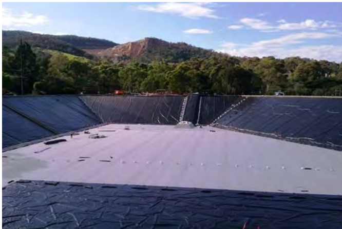
Figure 3: Geomembrane being installed over Geotextile
