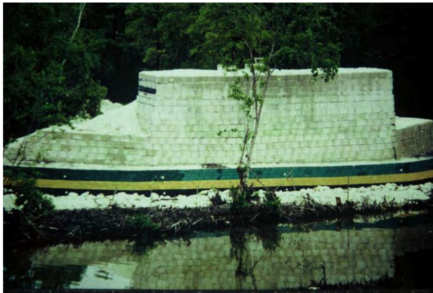
Figure 5. View of abutment after completion of surcharge loading.
