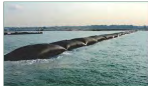
e) Geotextile tube crest of containment dyke
