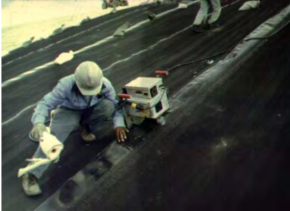
Figure 8. Example of Smart Welder.
