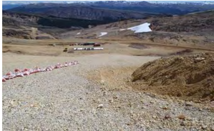
Figure 7 Support for the bituminous geomembrane (note particle size of the support)
