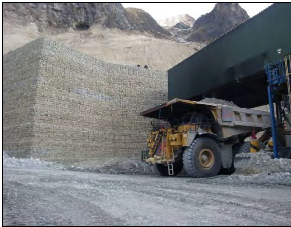
Figure 14. DTSW mesh/ Geosynthetic reinforcement System rockfall embankment for protecting the primary crusher and conveyor belts ( h_{\max} = 20.00\text{m} - Peru).
