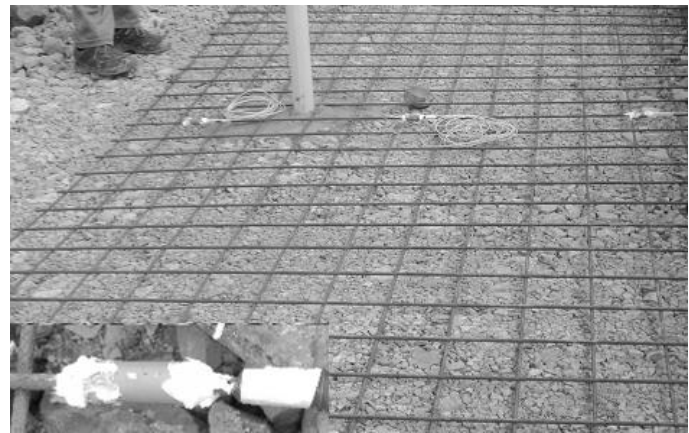
Figure 2. Q335 WWM with installed strain gauges, and strain gauge protection detail
