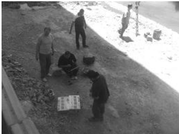
Figure 7. Geodetic survey of wall face
