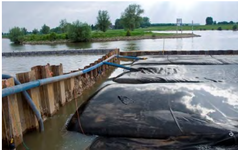
Figure 8. Filling of geotextile tube with dredged contaminated sediment.
