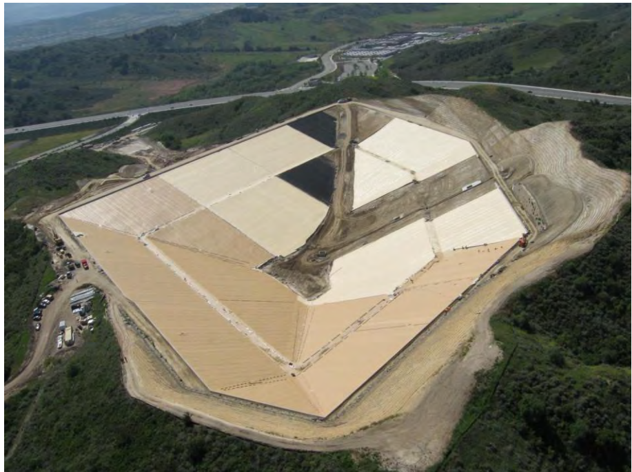
Figure 1: Aerial view of the Upper Chiquita Reservoir under construction.
