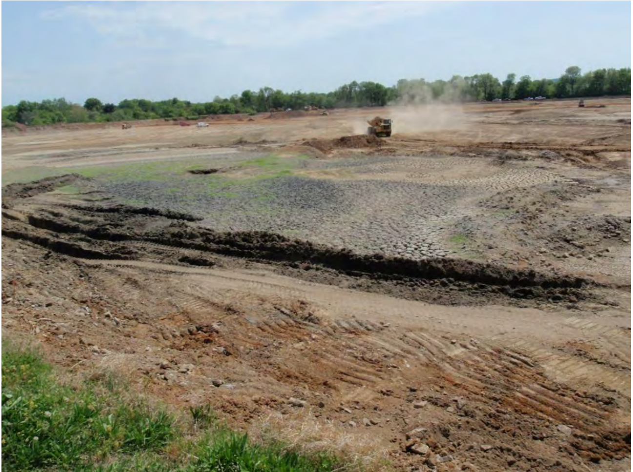
Figure 3: Disposal of filter backwash solids
