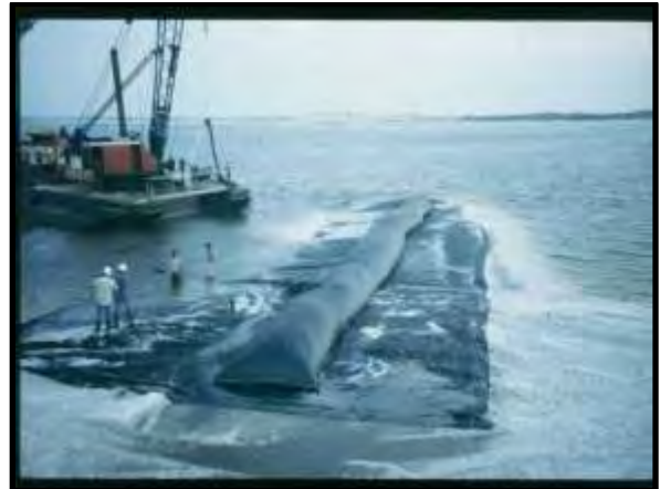
Figure 14 – Geotextile Tube / Groin
