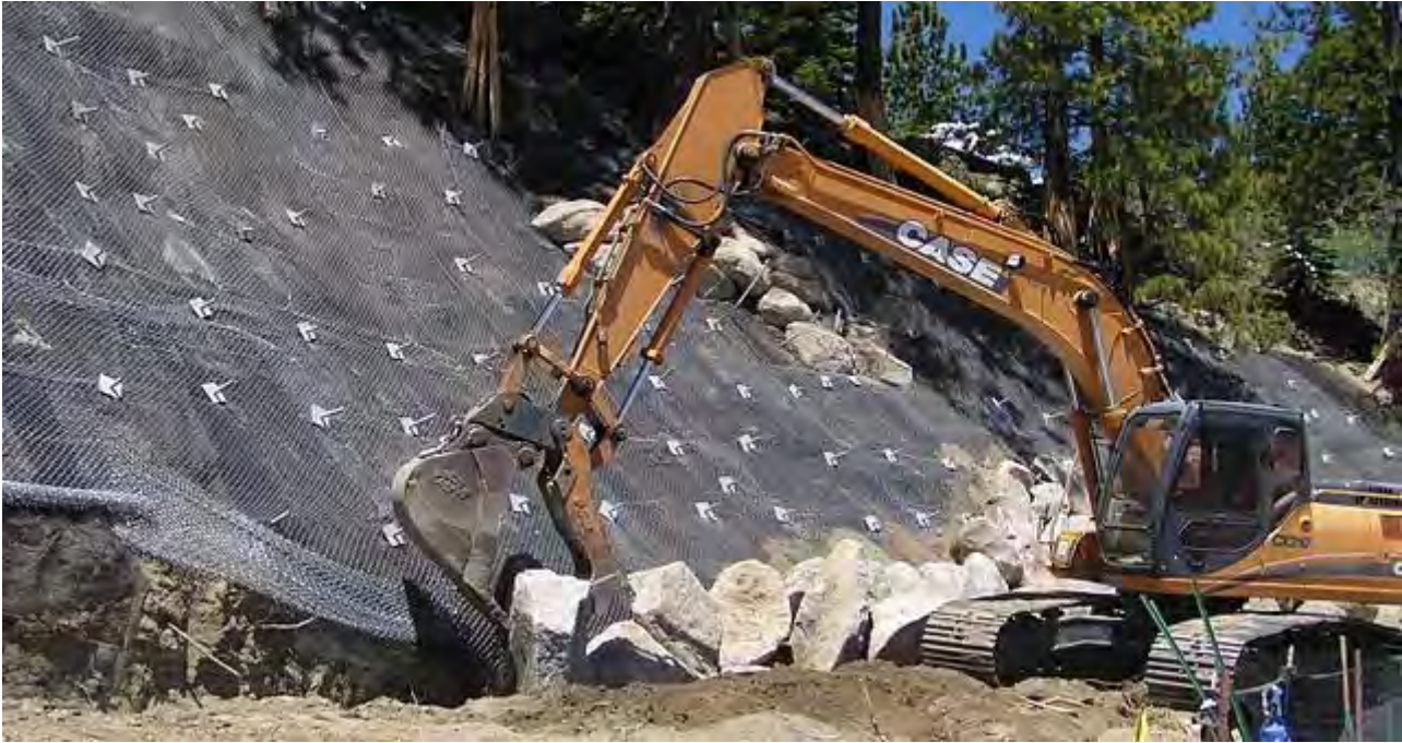
Figure 6 - Native boulders to protect the toe of slope from wave action.
