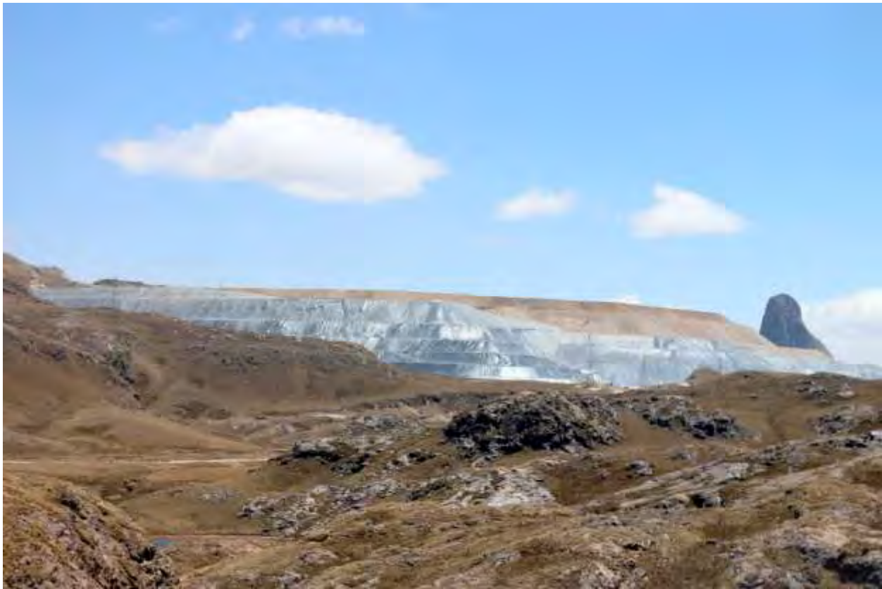
Figure 9. Currently the largest use of raincoats is at the Lagunas Norte gold mine in northern Peru with approximately 30 ha installed (Sept. 2012).
