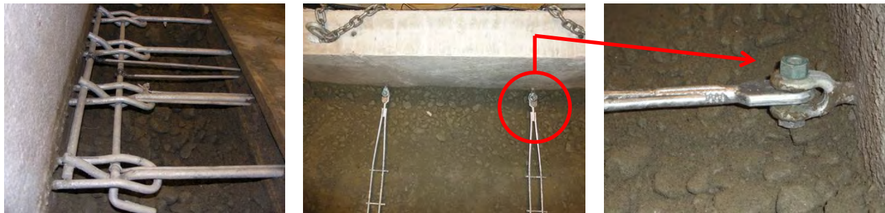
(a) Loop-Crimp connection
