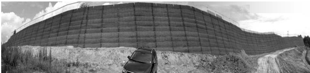
Figure 1. View in construction phase (without piled noise protection wall).
