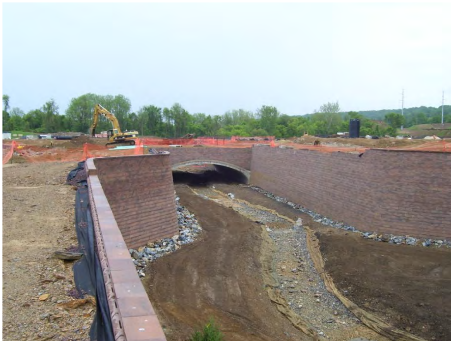
Figure 7- Completed retaining walls along the proposed stream.
