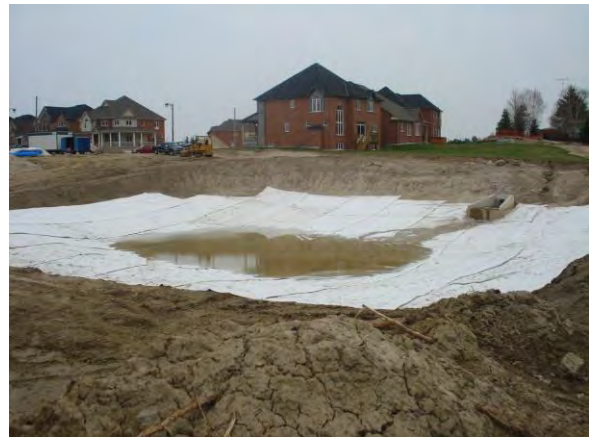
Figure 15. GC leaving the site once the GCL has been deployed. No cover soil.
