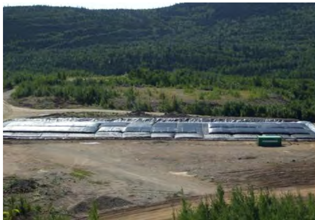
Figure 6. Two layer pyramid to maximize available area.
