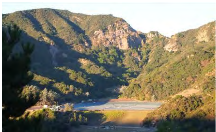
Figure 1: The completed reservoir blends nicely with its surroundings.
