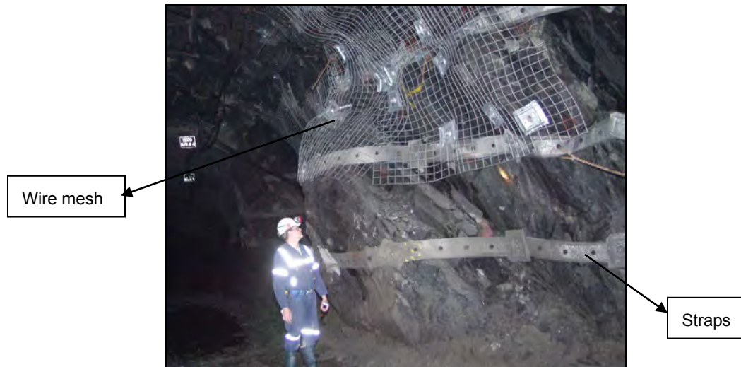
Figure 6: Wire mesh and straps application.
