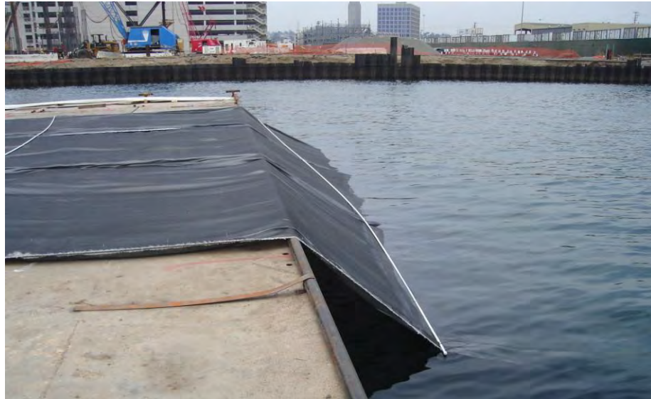
Figure 5. Rebar Attached to Woven Panel Being Deployed.
