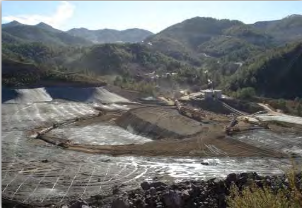
Figure 6. View of heap leach pad being stacked with portable grasshopper conveyors.
