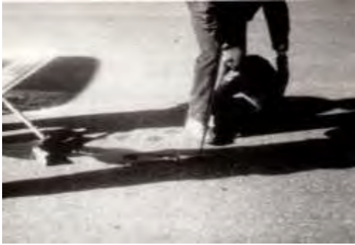
(a) Filling cracks in existing bituminous pavement
