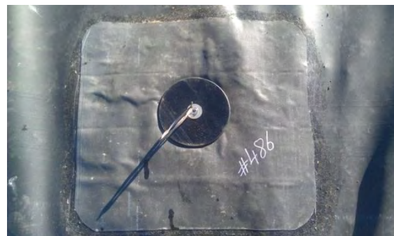
Figure 8. Anchor installed to EPDM Geomembrane
