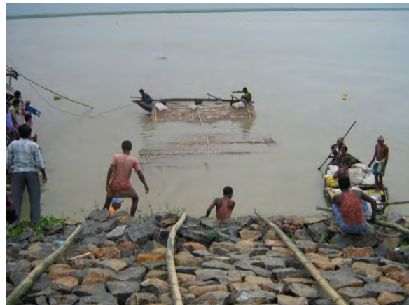
Tarza mat being laid in river bed
