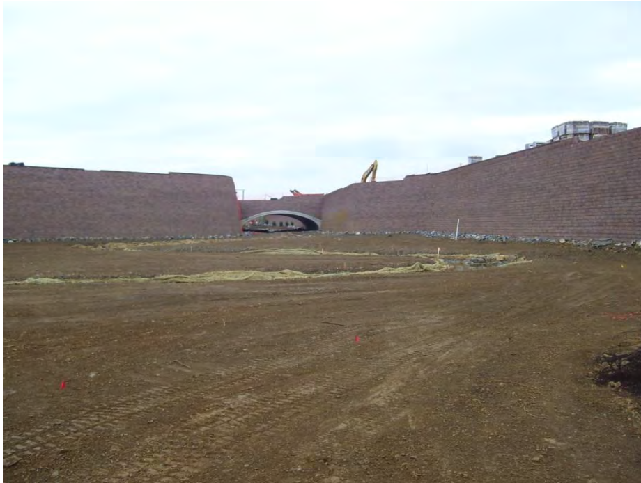
Figure 8- Completed retaining walls along stream, view from stream.
