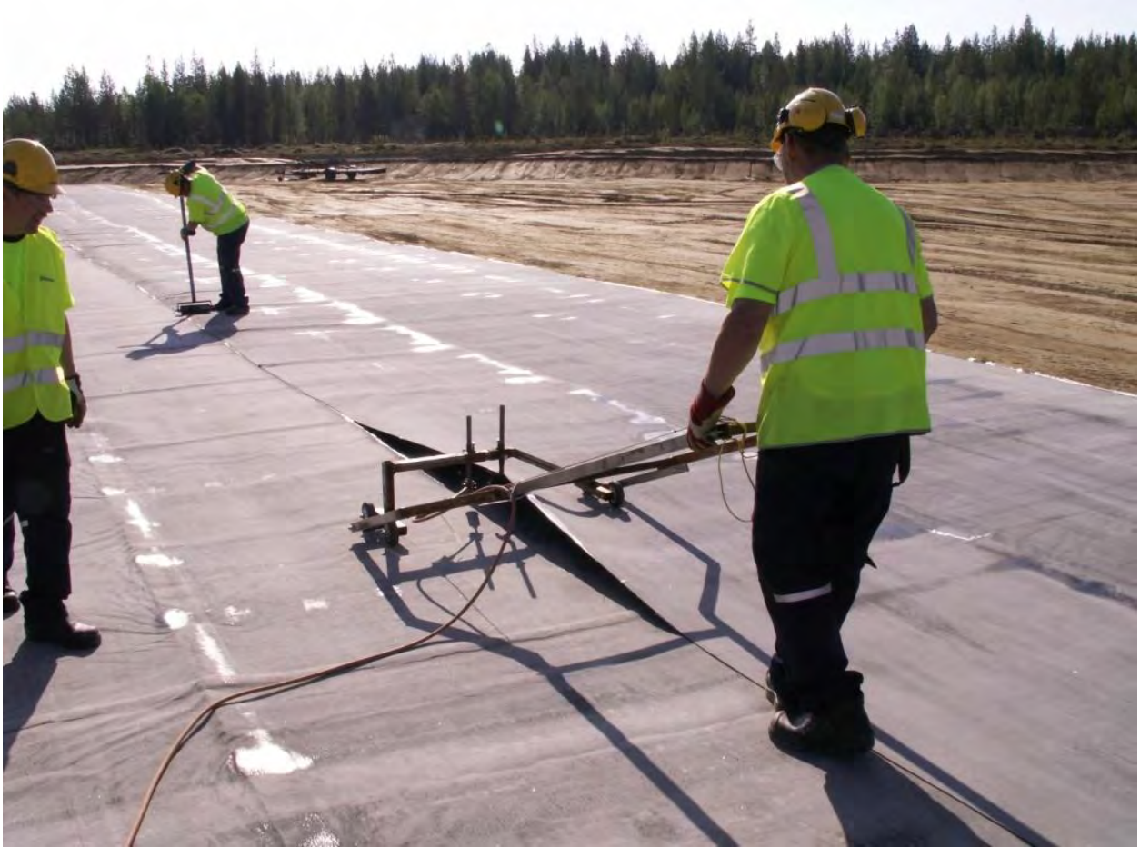
Figure 8: Welding of adjacent panels of bituminous geomembrane
