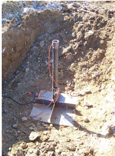
Figure 5- Settlement plate and pore pressure transducer cable.
