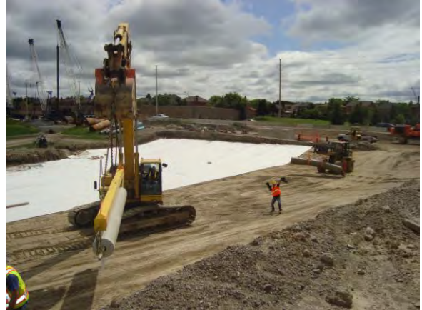
Figure 5. Placement of the cover soil for any lining projects should always be supervised.
