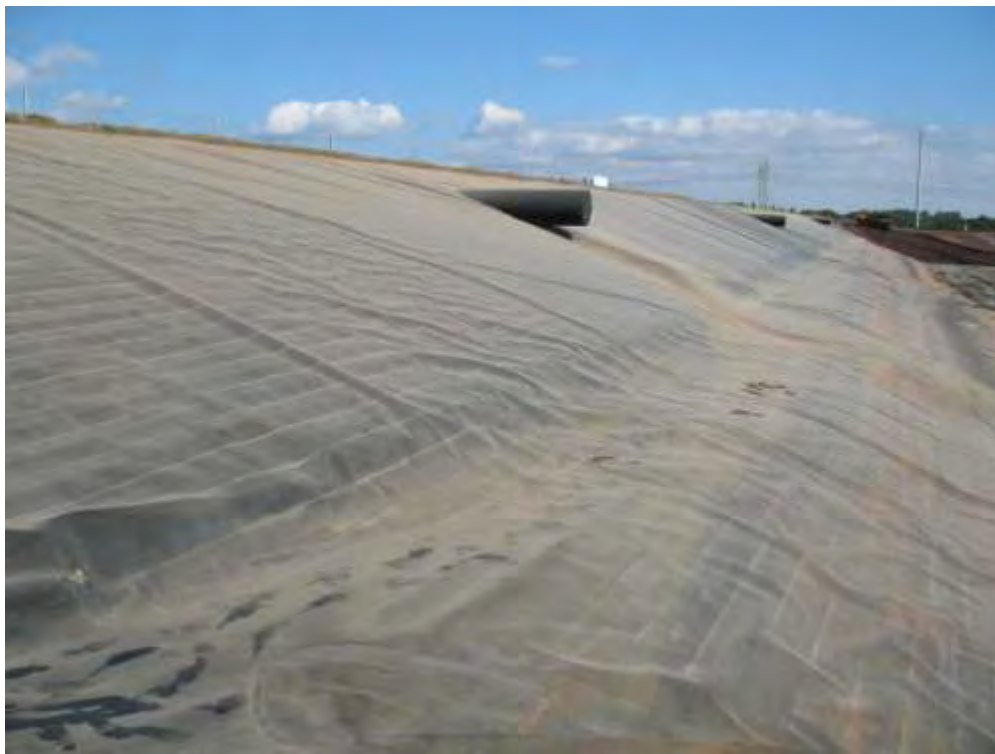
Figure 4. Thirty year old Schlegel HDPE geomembrane with frequent horizontal welds.
