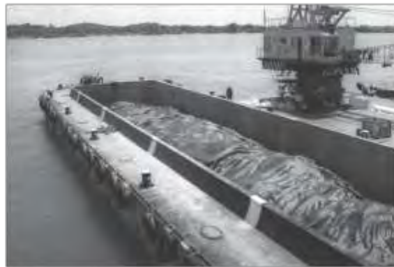
c) Geotextile containers
