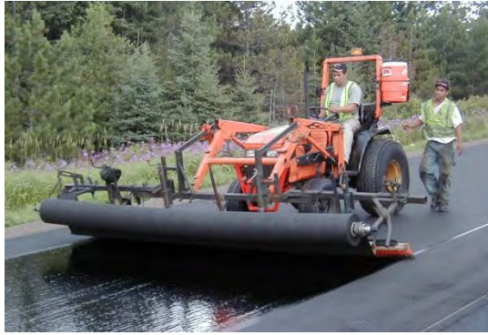
Fig. 1 Paving fabric placed into fresh tack coat
