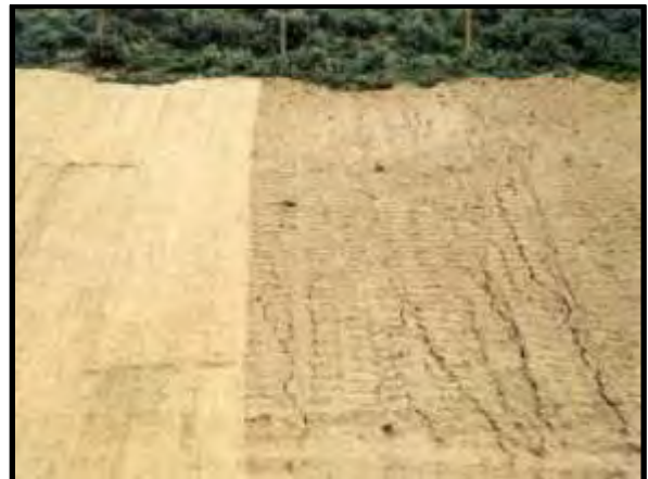
Figure 4 – ECB (left) vs. HMG (right)
