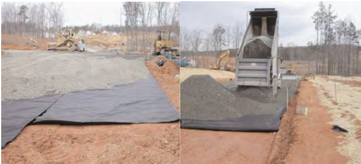
Figure 2. Pavement construction in 2003 showing placement of the woven base reinforcement geotextile.
