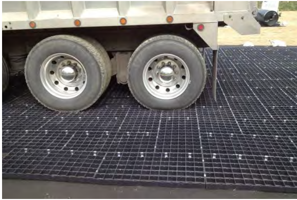
Figure 5. Photographs of a potential well pad system that consists of, from the bottom upwards: a 1.5 mm (60 mil) HDPE textured geomembrane, a 340 g/m 2 (10 oz./yd 2 ) cushion geotextile, a 50 mm (2 in.) recycled foam product, and a durable, reusable specialty mat product.
