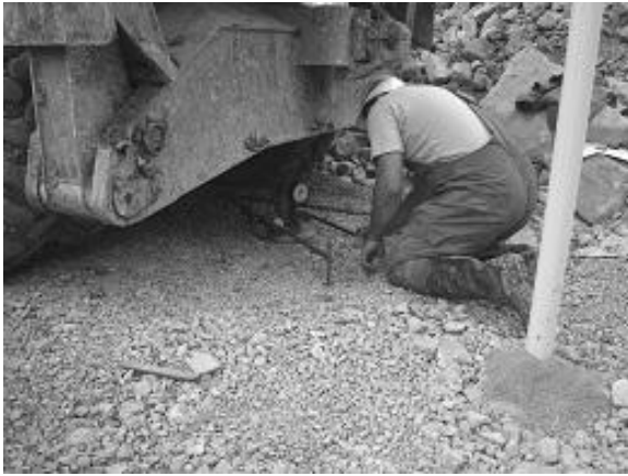
Figure 5. Static load plate test
