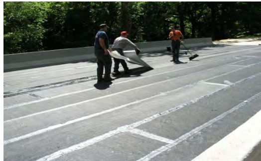
Fig.6 Strip membranes for a bridge deck waterproofing
