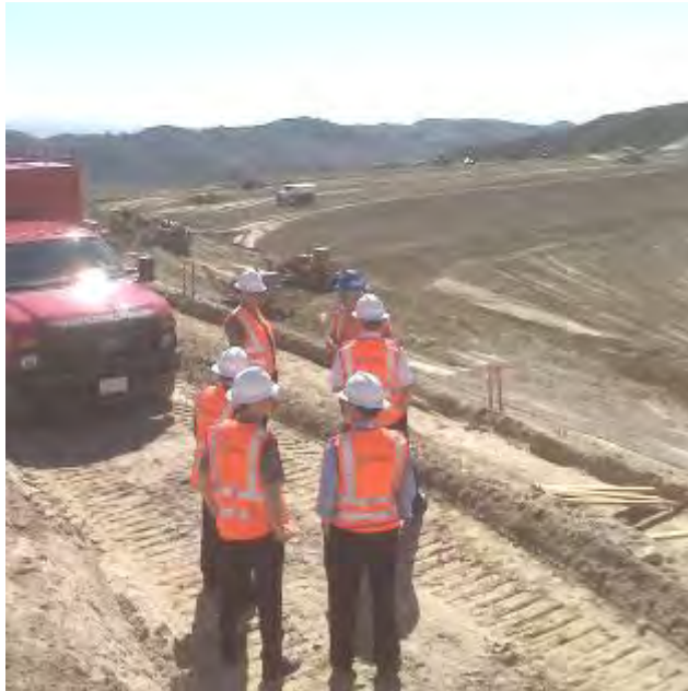
Figure 2: Site visit during the construction of the dam.
