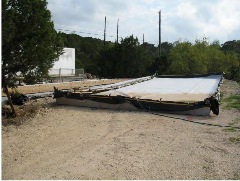
Figure 3. Exposed liner test cell.
