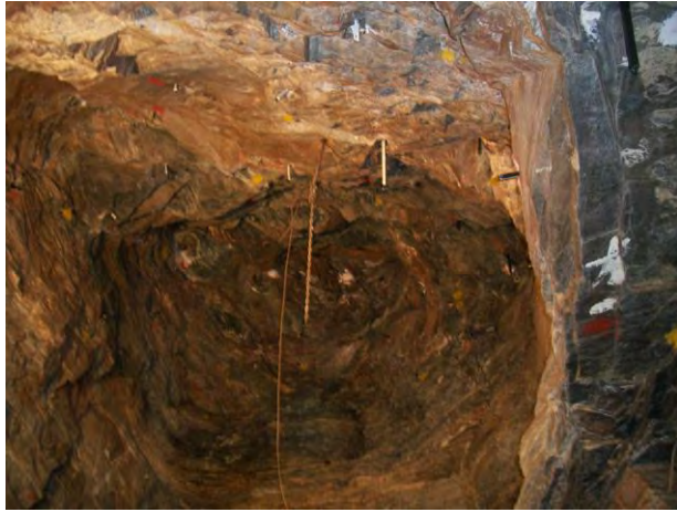
a) Area for geogrid application.
