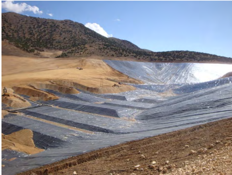
Figure 2. Example stability berm configuration from a heap leach pad liner project (photo courtesy of Comanco)
