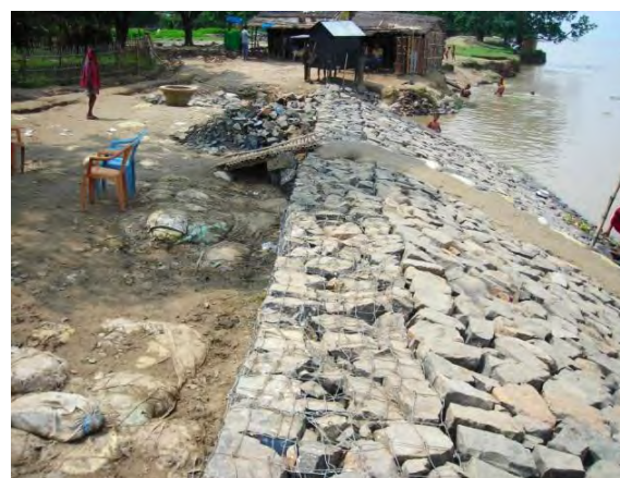
Protection work using Geotextiles and GI wires
