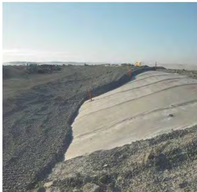
Figure 2: Bituminous geomembrane liner exposed for long term weathering assessment
