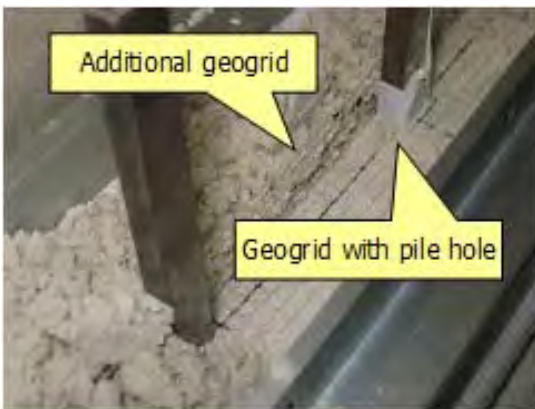
c) Geogrid installing
