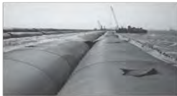
c) Installing base geotextile tube layer
