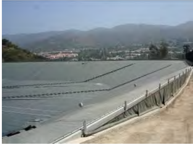
Figure 12: View of the overflow swale.
