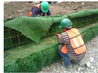
Figure 9. Field-bent black steel wire basket form.
