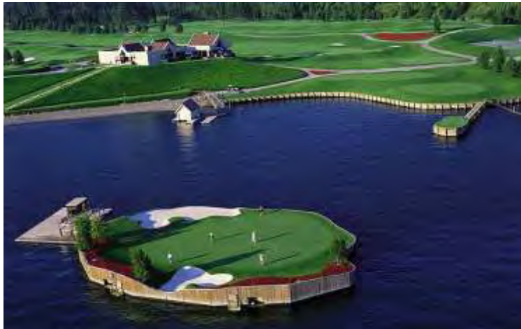
Figure 3 – A geofoam floated golf course green (Courtesy of WorldGolf.com).
