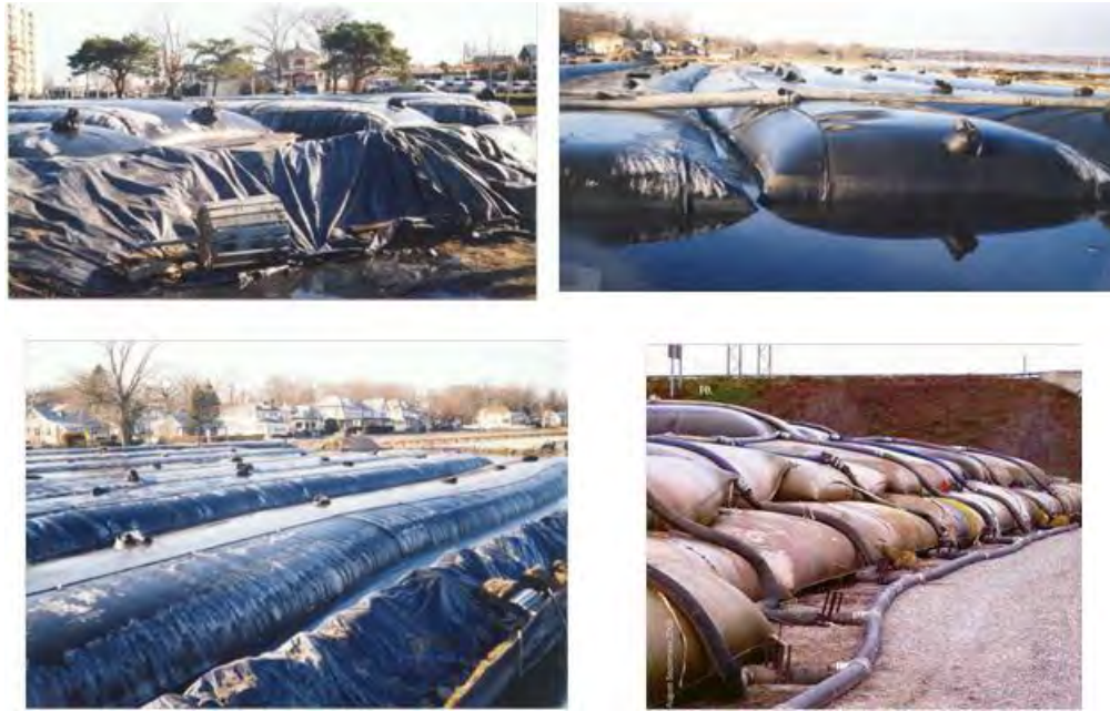
c) Geotextile tubes for harbor sediment dewatering (authors)
