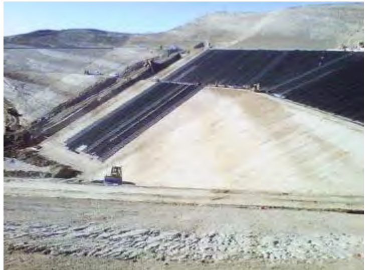
Figure 3: Placement of the geocomposite underdrain.
