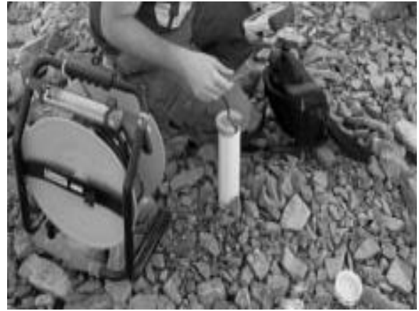
Figure 6. Inclinometer deformation measurements
