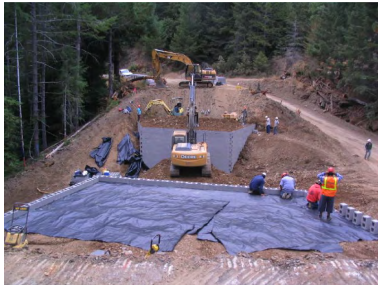
Figure 9. Abutments during construction. Using two crews cut construction time in half.
