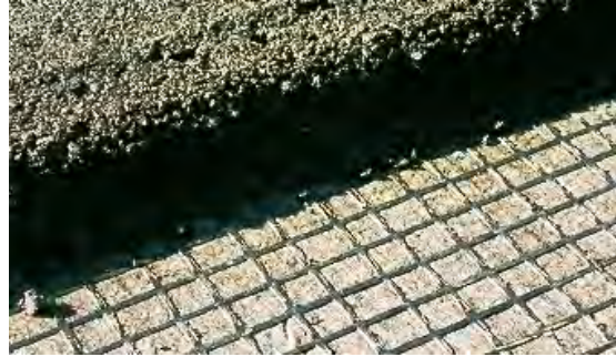
Fig. 4 Paving grid/paving fabric composite and overlay
