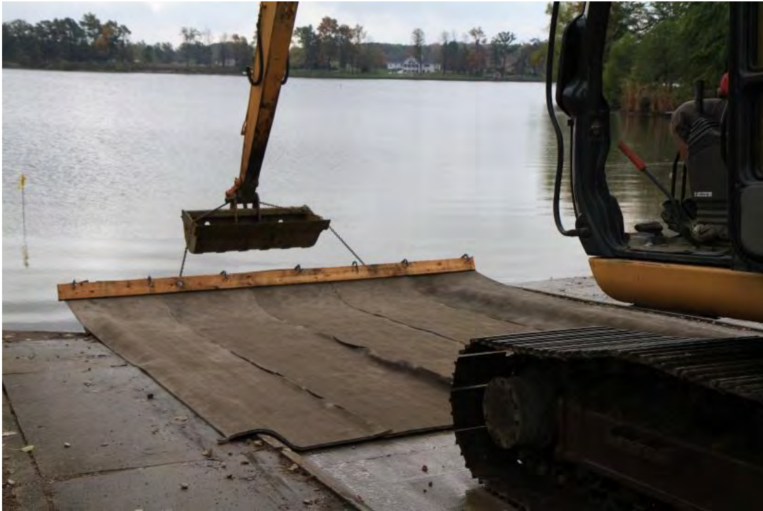
Figure 4– Panel Installation Concrete Cloth Composite Mat
