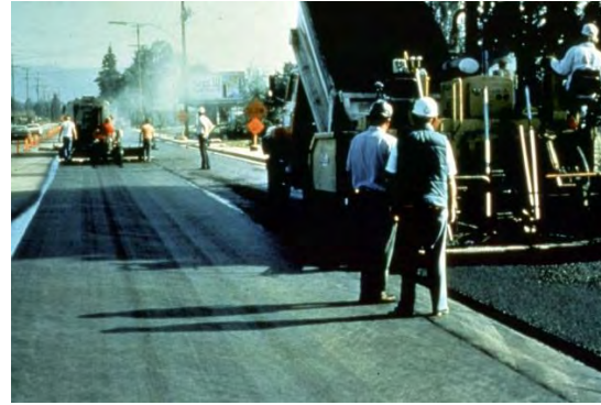
Fig. 2 Asphalt concrete placed over paving fabric
