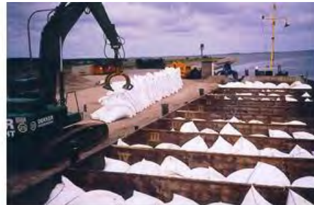
a) Large geotextile bags for coastal erosion control (compl. NAUE).
