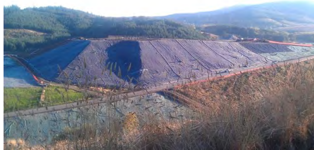
Figure 6. Picture of Northwestern US exposed cap (Case History #4)
