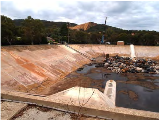
Figure 2: 130 Ton crane used to remove old liner
