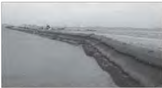
d) Final filling of artificial island
