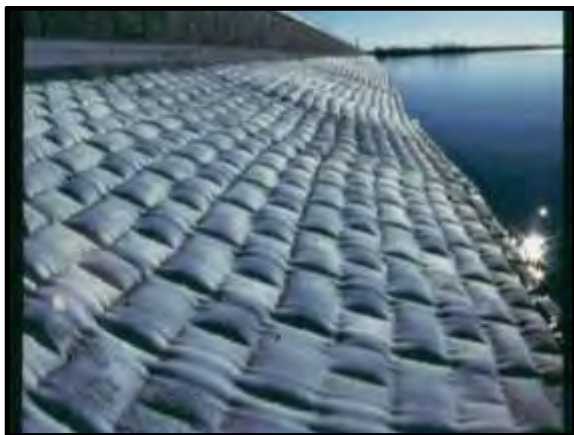
Figure 7 – FFR Installed in Wave Zone
