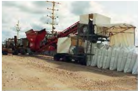
a) Large geotextile bags for coastal erosion control (compl. NAUE).
