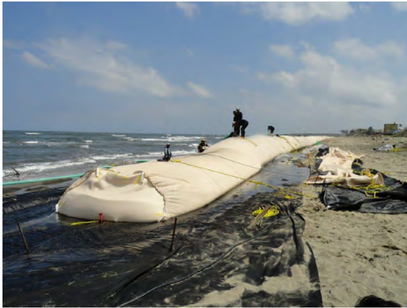
Figure 9. Installation and filling of Geotextile tubes
