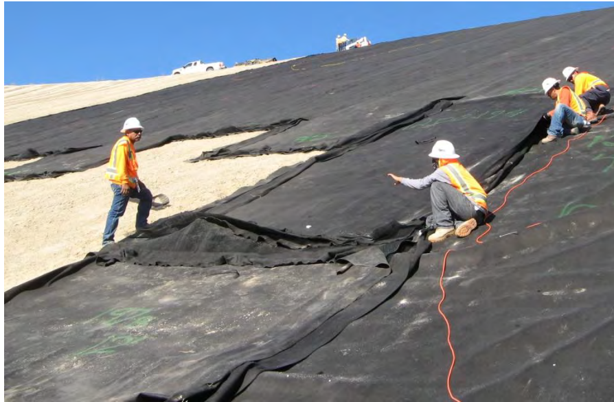
Figure 6. Installation of geonet composite panels and horizontal seams.
