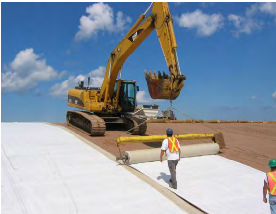
Figure 1. GCL being used in a landfill cap application.
