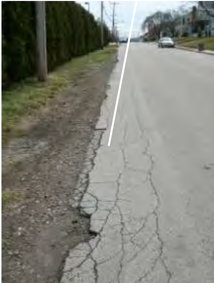
Figure 13. Longitudinal pavement cracking on unrestrained (left) pavement edge and none on curb retained (right) pavement edge.
