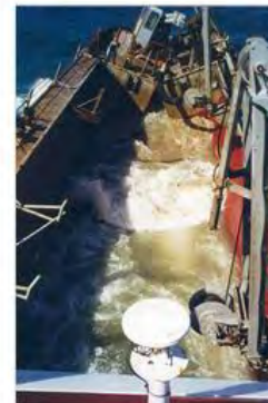
b) Geotextile containers for removal of harbor sediment (compl. TenCate)
