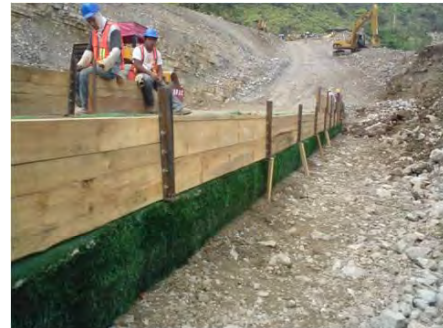
Figure 11. Wood forms used at wall face.
