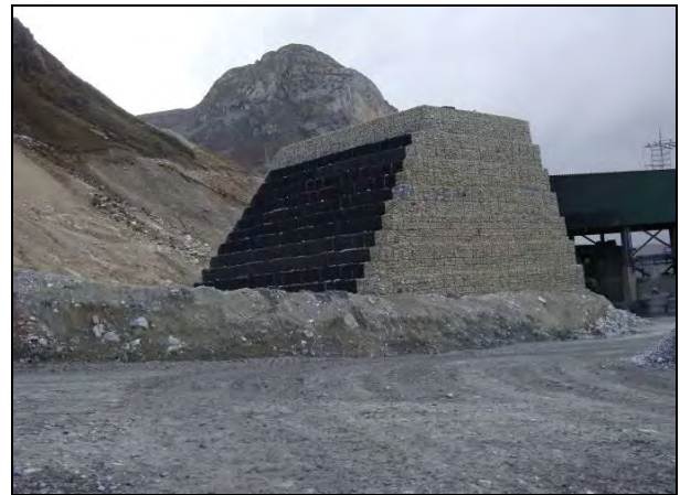
Figure 14. DTSW mesh/ Geosynthetic reinforcement System rockfall embankment for protecting the primary crusher and conveyor belts ( h_{\max} = 20.00\text{m} - Peru).
