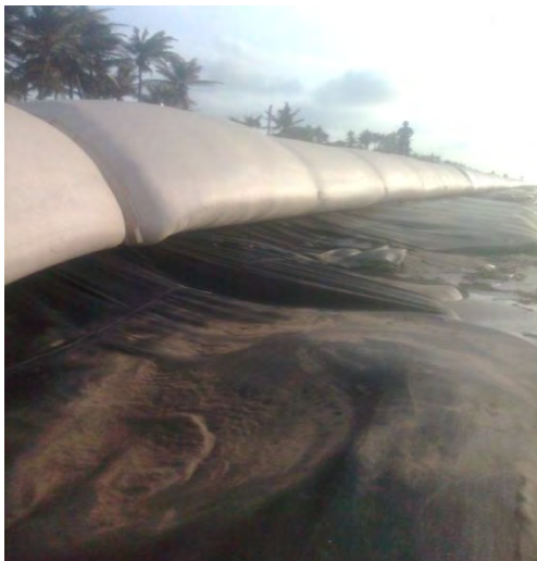
Fig. 10 Scour aprons in operation
