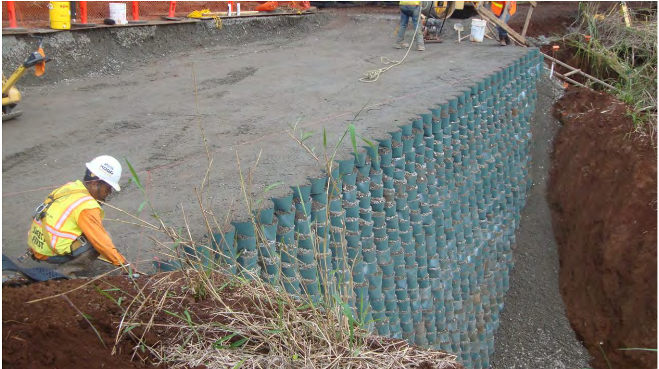
Photograph 4. Site 4 Near the End of Construction.
