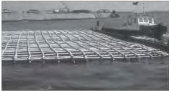
c) Towing fascine mattress into place
