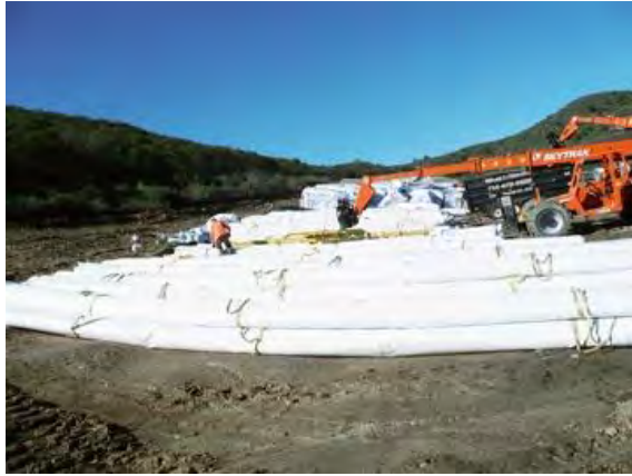
Figure 4: 36 ft wide prefabricated liner panels
