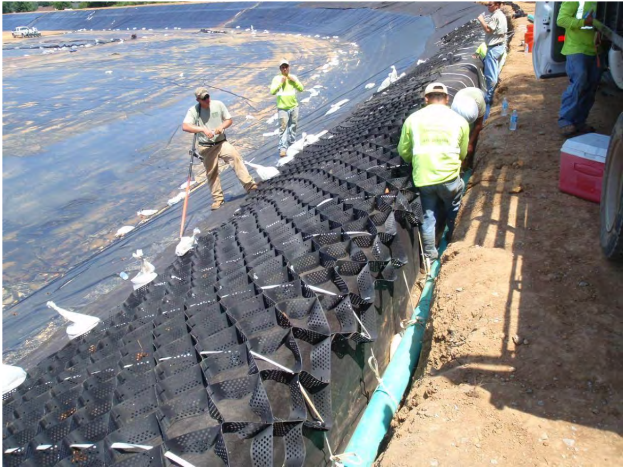
Figure 5: Installation of geoweb along the side slopes
