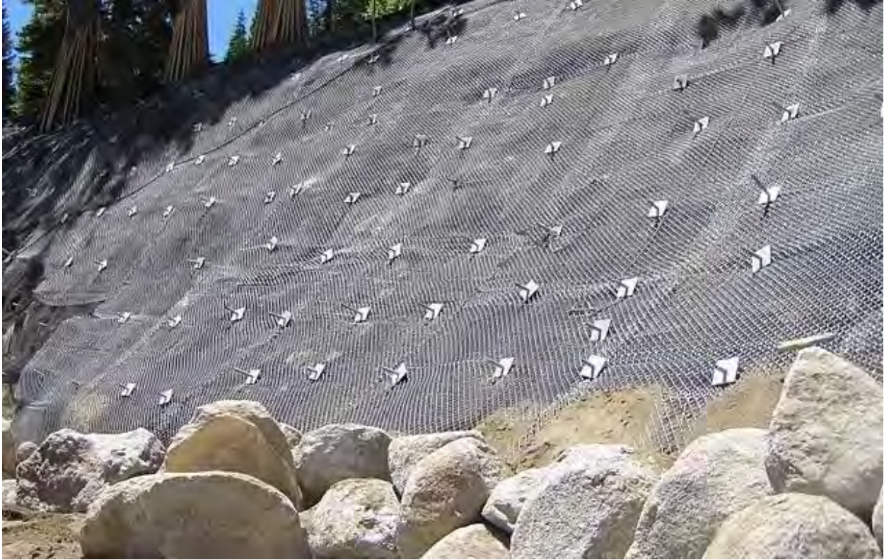
Figure 3 - Tensioned Galvanized Wire Mesh
