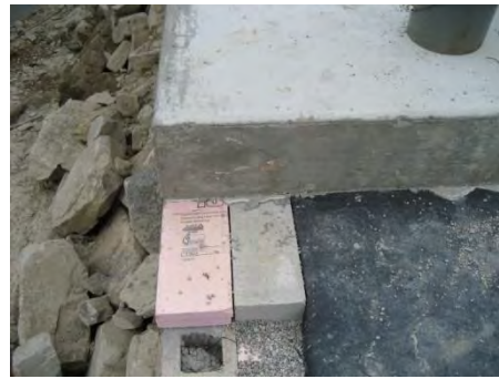
b) footing placement on GRS abutment
