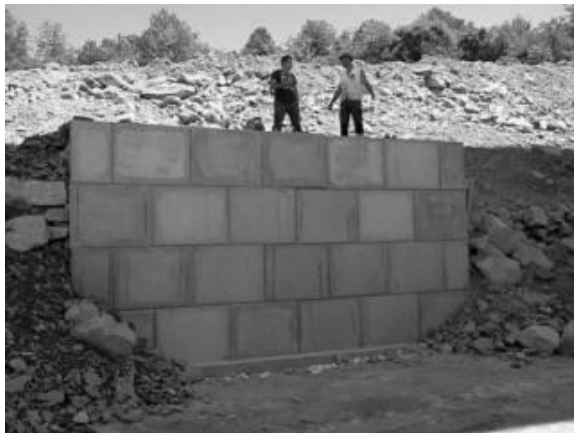
Figure 1. Erected MSE test wall
