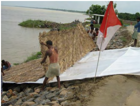
Fixing of the Geotextile on Tarza mat
