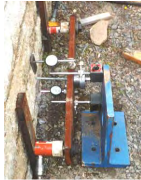
Figure 2. Block pull-out test on a GRS wall (Adams et al. 2011a).
