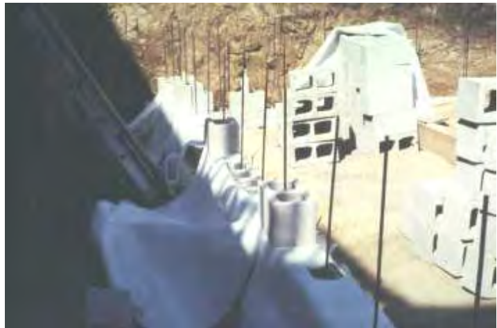
Figure 1. First geosynthetic reinforced soil, block-faced wall constructed in the late 1970s (Courtesy of Professor J.R. Bell)
