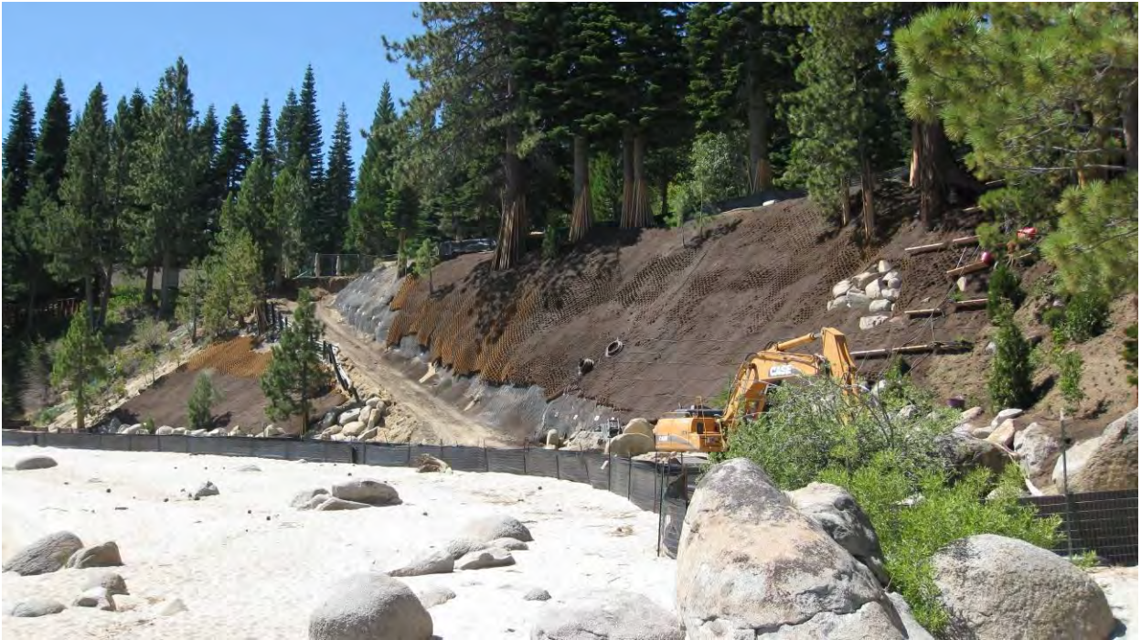
Figure 5 - 75% of the cellular confinement has been filled and planting has started.
