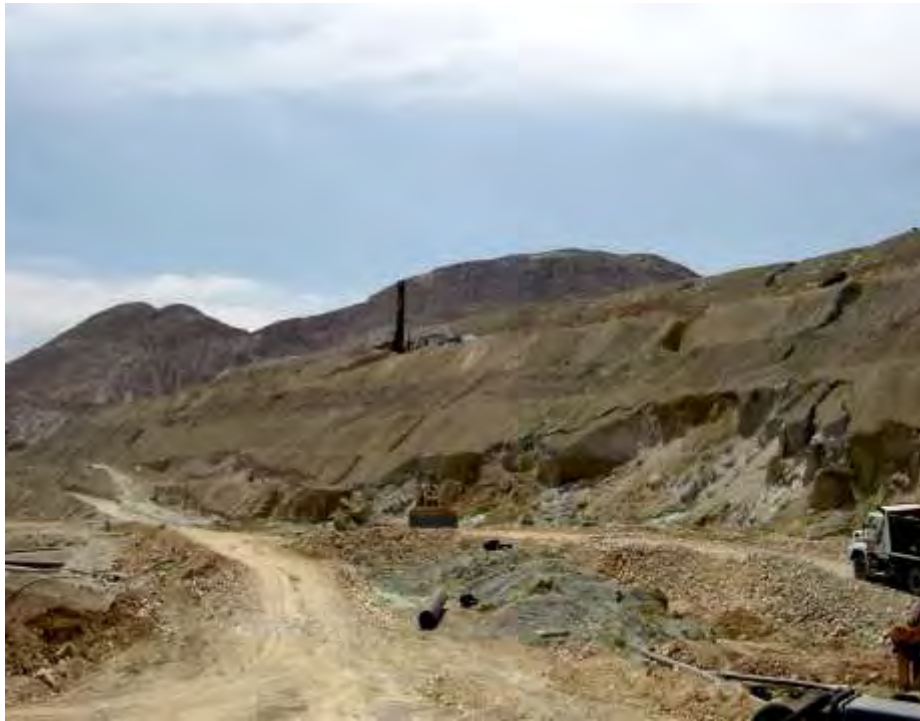
Figure 3. Local liquefaction failure at the Cerro Verde copper heap leach, triggered by high solution levels. For scale, the benches are separated vertically by 7 m.
