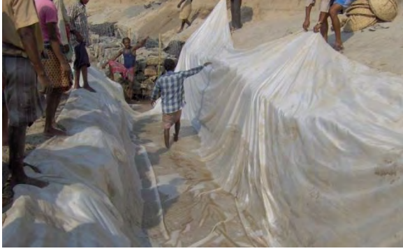
Anchoring the Geotextile on the river bank
