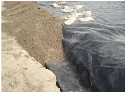
Figure 9 Ballast Trench Under Construction
