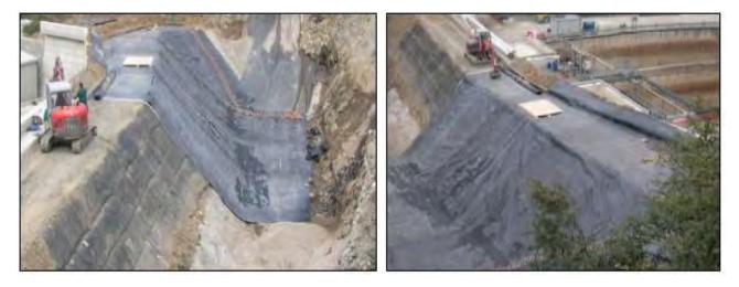
Figure 5 Reinforced earth embankment behind the wall and connection to the old lining system
