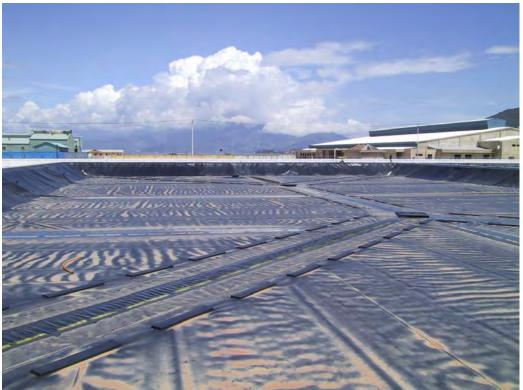
Figure 4. A combined defined sump and gas harvesting cover – HDPE
