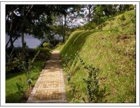
Figure 11. Another example of a "Green" Reinforced Soil Wall four months after construction was finished
