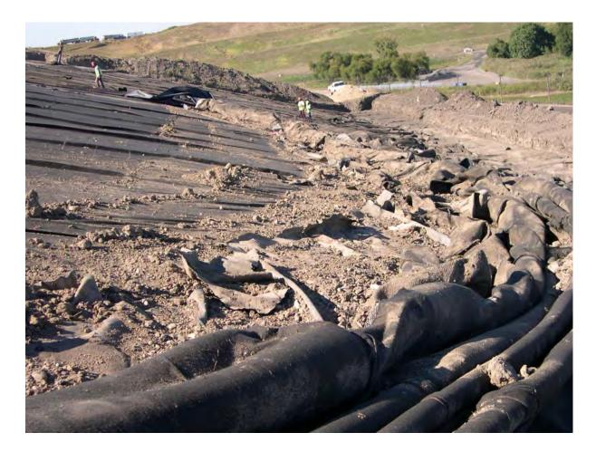
Figure 6. Typical removal of final cover system in failure area.
