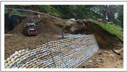
Figure 5. Installation of the woven Geotextile and spread of the fill soil
