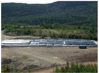
Picture 1: Pad with geotextile containers
