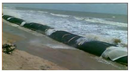
Figure 12. Protection of seashore with geotextile tube at Shankarpur, West Bengal, India
