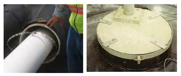
(c) Thin band clamp that has loosened and come off. (d) Heavy wide custom clamp around end of a penetration.
