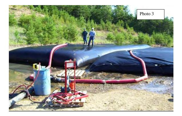
Once all the needed data was collected from the containers, they were split, the material loaded out with a front end loader into trucks and hauled to the coarse refuse disposal area. The material had a consistency of fine, wet sand.
