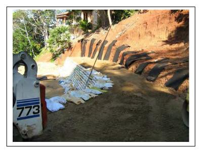
Figure 4. Installation of sacks (filled to a 1/3 of their volume with organic soil) in the façade
