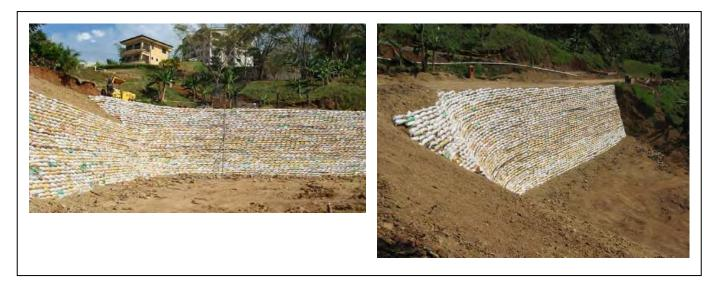
Figure 7. Facade of the wall with sacks filled with organic soil
