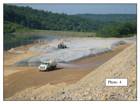
In order to maximize utilization of bag field areas, bags can be stacked on top of each other in a pyramid fashion once the water runs out and the bags have stabilized. Containers were to be placed on top of each other overlapping the line between them. The first field (Bag Field # 1) was approximately two acres in size. The design called for a total of four levels of bags to be filled. Containers were ordered for the field as follows:
