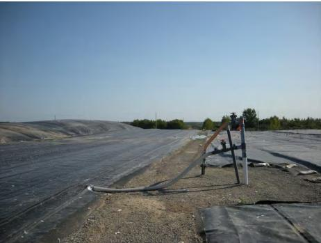
Figure 5 Inflated Area and Trial Landfill Gas Extraction Connection
