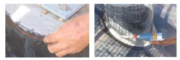
(e) Embedding copper wire before weld for spark test.
