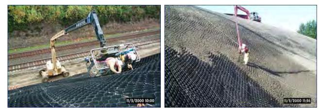
Figure 4. Site 1 geocell anchoring and filling cells with crushed rock.
