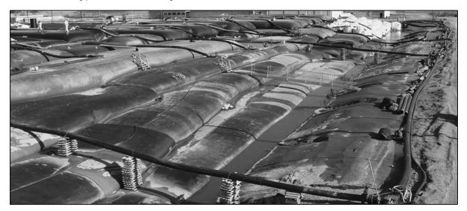
Figure 7. Ramps and stairways constructed to allow personnel safe access to the top of the stacked tubes (May 2008).
