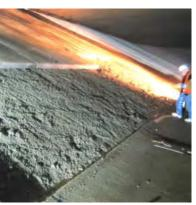
Figure 12. Once the concrete was removed an engineer determined how much of the saturated subgrade to remove.
