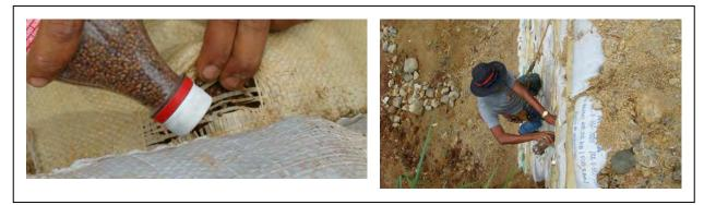
Figure 8. Vegetation seeds installed in each sack
