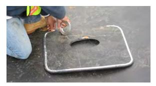
(b) Applying aluminum tape to bottom of plate for spark test.
