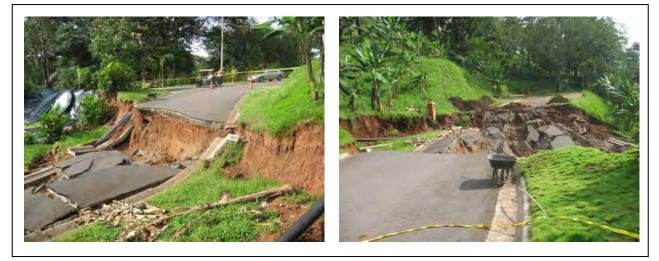
Figure 1. Initial state: Failure of the existing soil and road
