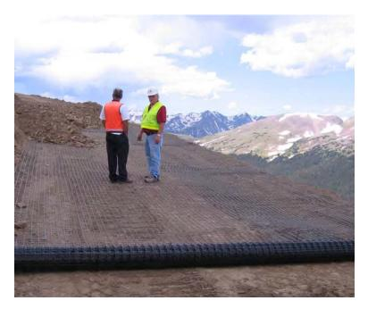
Figure 7. Placement of Biaxial Geogrid
