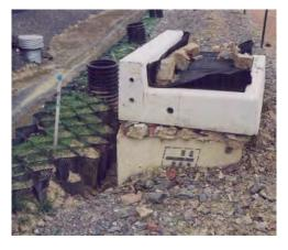
Figure 7. Washouts around inlet structures.
