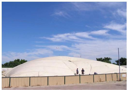
Figure 5. Inflatable Gas Cover – Flexible fPP-R Scrim Reinforced
