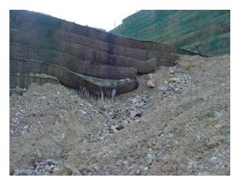
Figure 5. Adverse results arising from a stormwater detention basin above the wall.
