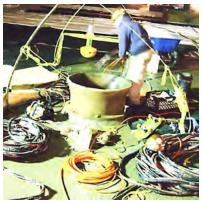
Figure 14. Diving set up at primary drain. Note the bell-shaped standpipe installed on the drain.
