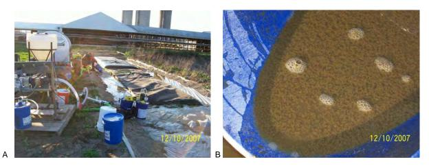
Figure 4. Randy Goettemoeller site after several pumping events (October 12, 2007). An agricultural weight geotextile tube container (background) was pumped to 26 inches over 8 weeks and an industrial weight geotextile tube container (foreground) was pumped to 28 inches (A). Samples collected to verify inline chemical conditioning (B).
