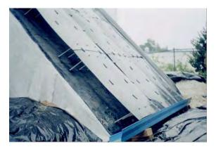
Figure 2. Photograph of field installation of geosynthetic separation box of HDPE(2)
