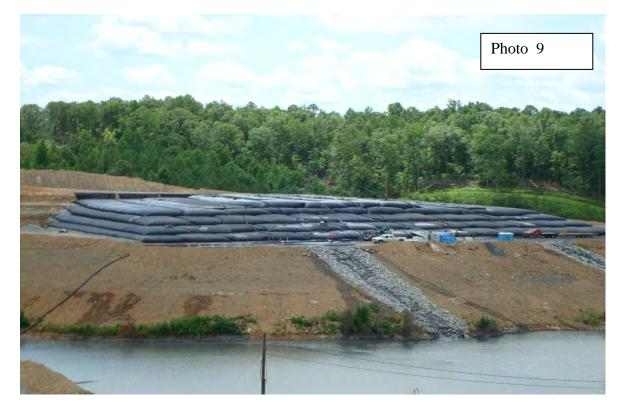
Once all the bags in the field were full and dewatered, the site was then ready for reclamation. First a layer of sand was used to cover the sides of the bags to provide a filter medium and then a layer of limestone for drainage. The bags were then covered with earth and finally topsoil. A low ground pressure bulldozer was used to cover the containers. All the bag field sites were very stable and no problems were encountered during the covering operation with the equipment. (Photo 10)
