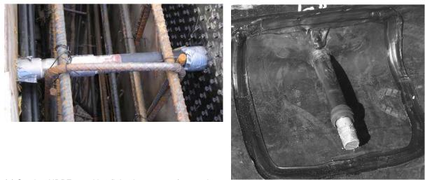
(a) Steel-to-HDPE transition fitting in concrete formwork through studliner.
