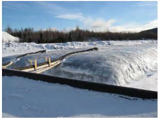
Picture 3: Geotextile containers in operation during winter
