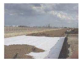
Figure 12 Installation of composite base course reinforcement
