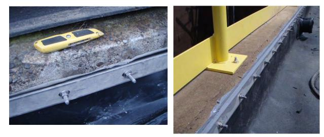
(a) Thick fuel-resistant moldable sealant used to provide leak-resistant seal against rough concrete.
