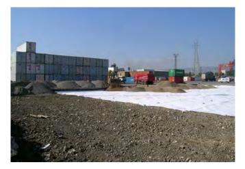
Figure 10. Installation of composite base course reinforcement
