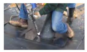
(d) Welding the pipe to the plate. Ideally another welded boot will be installed over this.
