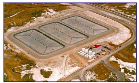
Figure 8. Salt Lake City Airport Deicing Covers (2000) with Double-Y Channels
