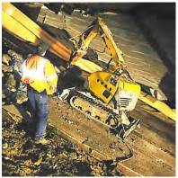
Figure 11. Remote controlled concrete breaker working on reservoir slope.
