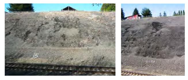
Figure 9. Gravel missing from geocells as a result of soil erosion below geocell slope protection system, Site 1.
