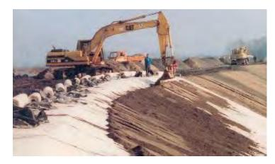
Figure 2. Lippe River levee reconstruction (1994): Installing Bentofix<sup>®</sup> GCL as a levee seal (Saathoff et al. 2003).
