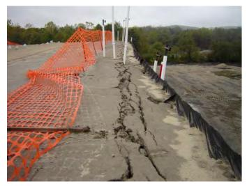
Figure 6: Tension Cracks From Heavy Rain
