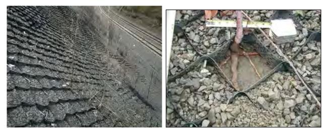
Figure 7. Sparse vegetation and root system spread across top of geotextile, Site 1.
