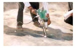
(c) Seaming the membranes by extrusion welding
