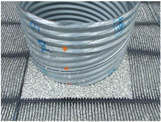
Figure 1 Cut geogrid around CMP metal forms.
