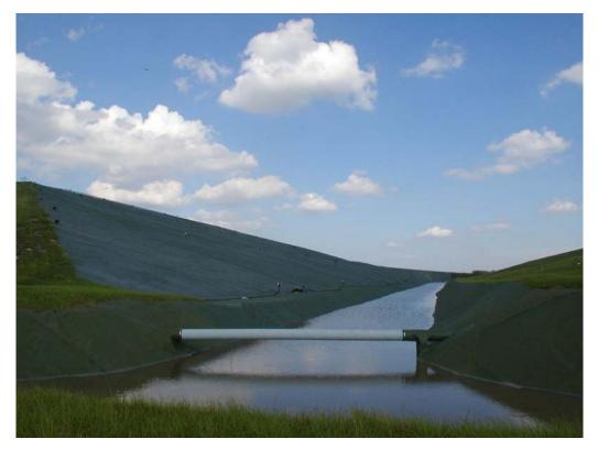
Figure 3. Stormwater sheet flow off of the EGC and into perimeter ditch.
