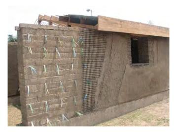
Figure 3. Construction process of geogrid reinforcement
