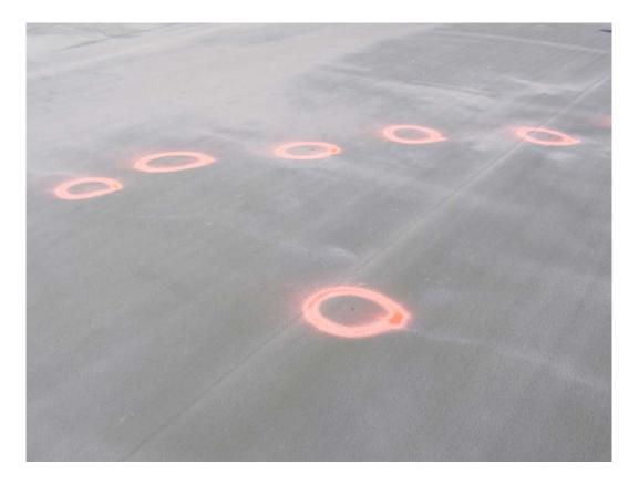
Figure 6. Odd holes in EGC.
