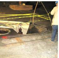
Figure 5. Surge tube leading into a small bypass outlet that connects to the main drain (circular opening on the left)
