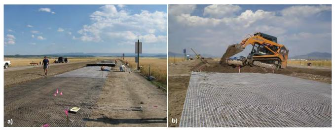
Figure 9. Construction of base course: a) prior to placement of aggregate, b) during placement of aggregate.
