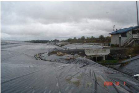
Figure 4 Drainage Ditch Showing Ballast Tubes
