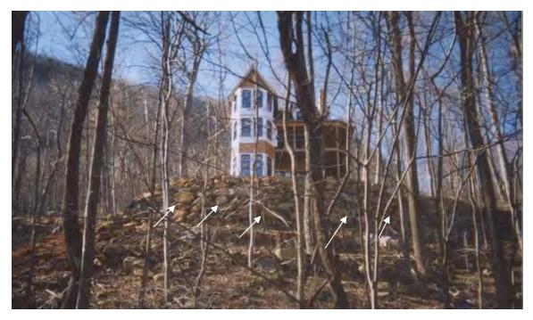
Figure 1. Photograph of Wall "A" (arrows show either apparent poor boulder-to-boulder contact or apparent seams in the wall).
