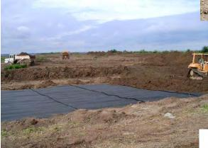
Figure 10 - Placement of harvested material in lifts to not exceed bearing capacity of the sub-soil
