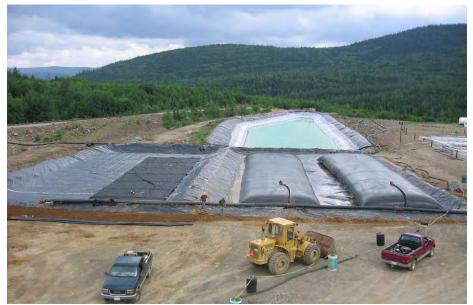
Picture 2: Geotextile container set up for filtration in a flow process
