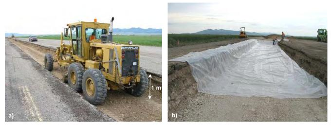
Figure 5. Construction of the test pit: a) final grading, b) installation of liner.
