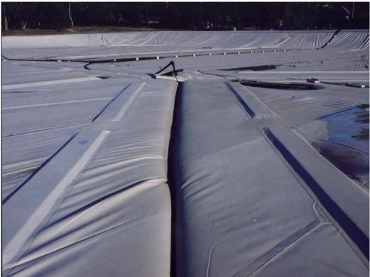
Figure 2. Ballasted trenches and floats - fPP-R defined sump floating cover
