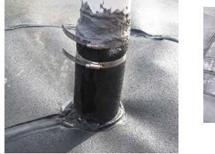
(a) Gasketed and banded boot with polysulfide coating on the end of the boot.
