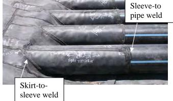
(b) Boot sleeve welded to pipe. This is commonly preferred by many installers for leak resistance.
