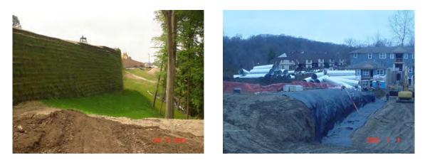
Figure 6. Underground stormwater management system behind 10m high MSE wall
