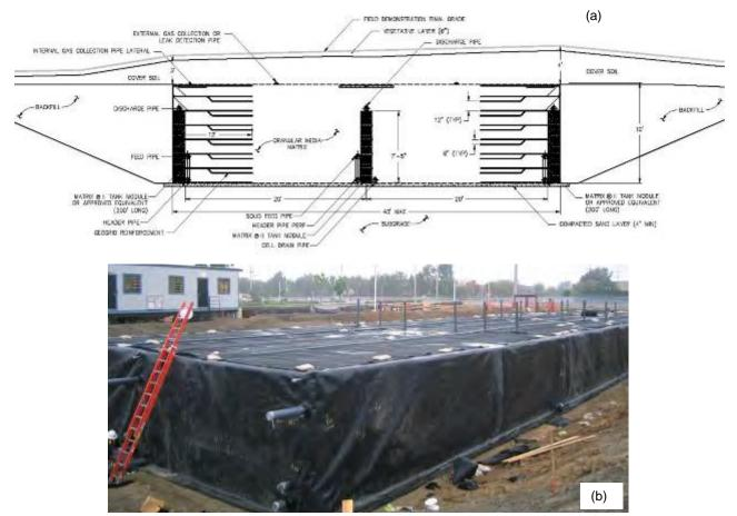
Figure 4. Cross section of the filter cell ((a) construction drawing and (b) photograph during construction)
