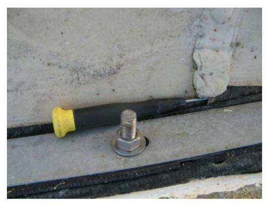
Figure 7. Extrusion weld stopped short of batten strip allowing liner overlap to leak as indicated by the pointer.
