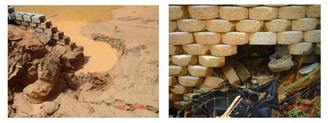
Figure 4. Uncontrolled rainfall runoff creating undermining and wall instability during construction.
