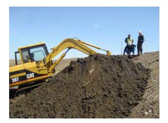
Figure 14 - Excavation of test trenches to reveal location of geofabric reinforcement
