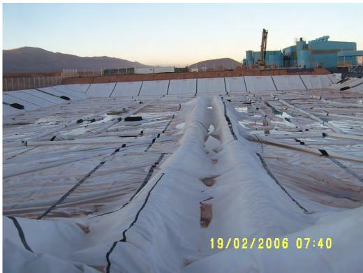
Figure 7. Cover to PLS pond with twin 750 mm diameter inlet pipes floating under cover.
