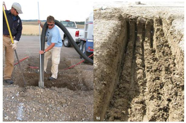
Figure 12. Forensic investigations: a) air and vacuum removal of base course, b) excavation of subgrade.
