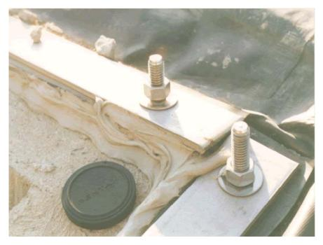
Figure 3. Improperly fastened batten strip.
