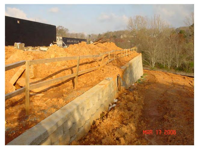
Figure 2. Top of wall being used for storage thereby applying a surcharge loading.
