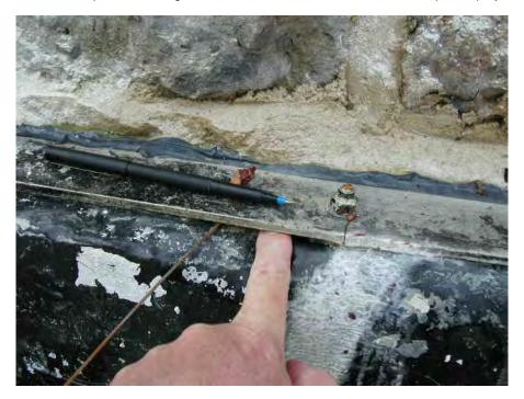
Figure 1. Inadequate sealing of geomembrane beneath batten strip.
