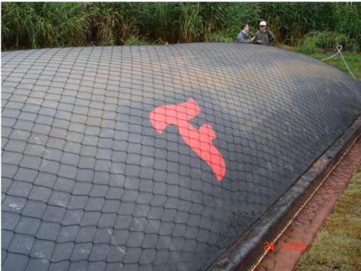
Figure 6. Inflatable / Expanding EPDM Rubber Gas Cover with Restraining Net
