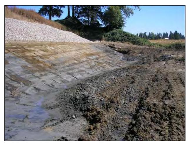
Figure 4. Lower slope immediately prior to placement of sand bedding and geocomposite.
