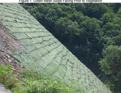
Figure 1. Green Mesh Slope Facing Prior to Vegetation
