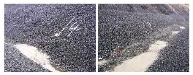
Figure 8. Silt deposits in ditch at slope toe, Site 1.
