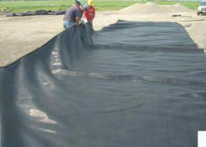
Figure 6 - Folding the completed unit - two sections sewed together to allow the connecting seam to be completed on location.
