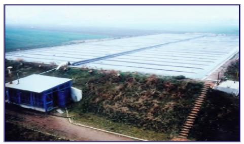
Figure 1. Anaerobic cover system in Harnes, France (1981)
