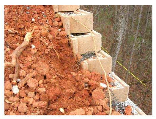
Figure 1. Stress concentration of geogrid layer over sharp back-edge of masonry block.
