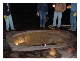
(b) Sinkhole at bottom of reservoir caused by failed pipe boot.
