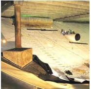
Figure 4. Surge tube (beige tube in foreground) directing surge water to the primary drain. Note the 1.2m (48") pipe boot and sloped column support in the background.
