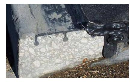
Figure 15. Cut section through actual concrete embedment strip with welded geomembrane.
