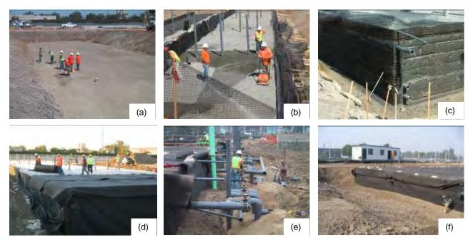
Figure 9. Construction procedure of the filter cell
