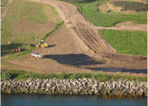
Figure 12 - Aerial view of operation, note interior haul road constructed to provide ORT access to berm construction. Note pile of material in the right side of the picture ready to be pushed onto the fabric. Dewatering pump in the top right of the picture.
