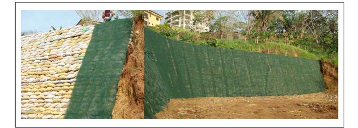
Figure 9. Installation of the permanent erosion control mat: TRM435
