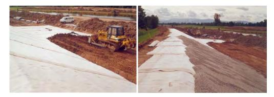
Figure 3. Kinzig River levee reconstruction (2001): Covering Bentofix<sup>®</sup> GCL with locally available fine gravel to ward off burrowing animals (right).
