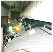
Figure 9. Sealing the liner under multiple small inlet pipes.
