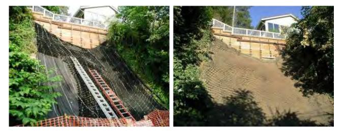
Figure 5. Site 2 geocell installation and completed slope after hydroseeding.
