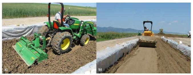
Figure 6. Subgrade construction: a) tilling, b) compacting.
