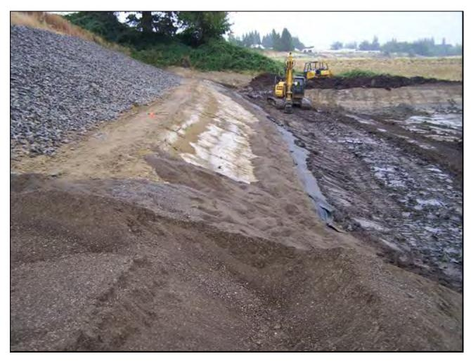
Figure 5. Geocomposite installation, showing sand bedding and CCL fill.
