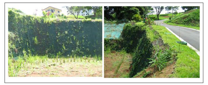
Figure 10. Vegetative state of the facade two months after construction
