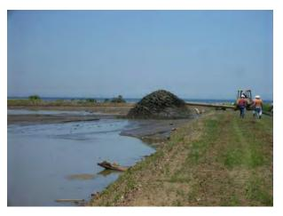
Figure 1- Hydraulic deposition of dredged material Into CDF 12
