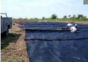
Figure 8 - Fabric units in placed and a field seam installed
