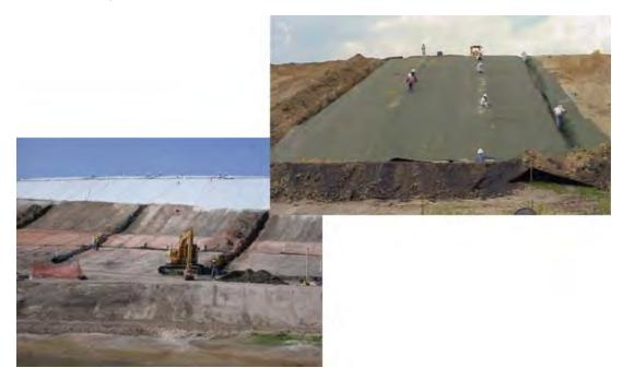
Figure 2. Construction sequencing illustrating side achorages.
