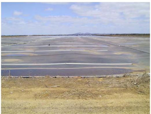
Figure 3. A fixed level floating HDPE cover for gas collection from an anaerobic lagoon
