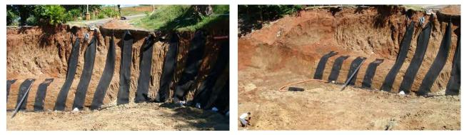
a) Strips of Geodrain at the rear of the wall
