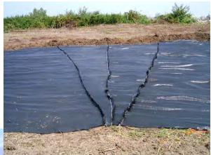
Figure 9 - Pie-shaped sections going around a curve
