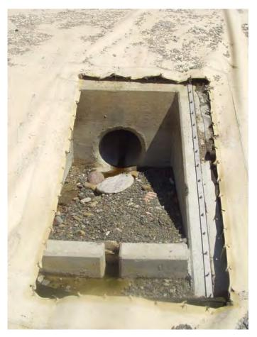
Figure 2. Liner pulled from batten strip by adjacent wrinkle.
