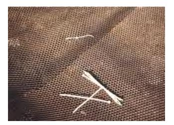
Figure 3. Plastic ties joining sides of a biplanar geonet.
