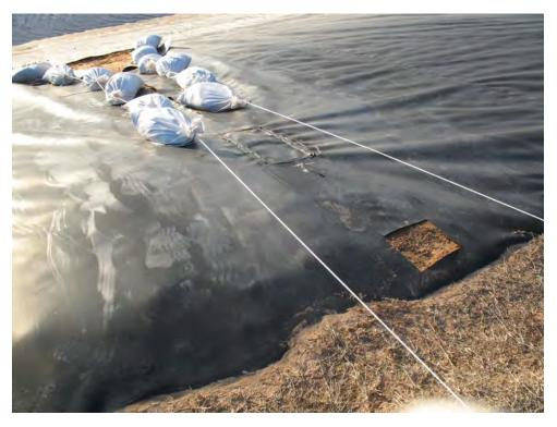
Figure 3. Stress cracks in apex-down fold (arrowed).
