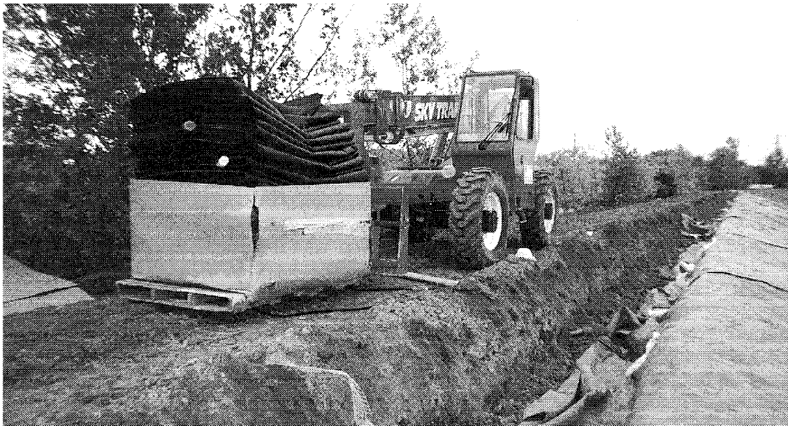
Figure 2. Photograph of PP panel carried to the site
