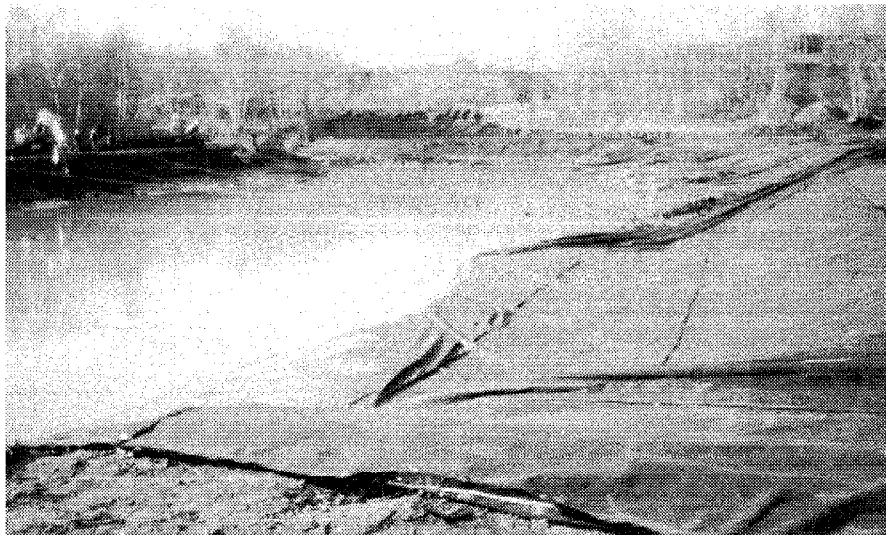
Figure 5. Installation of Geotextile Fabric.
