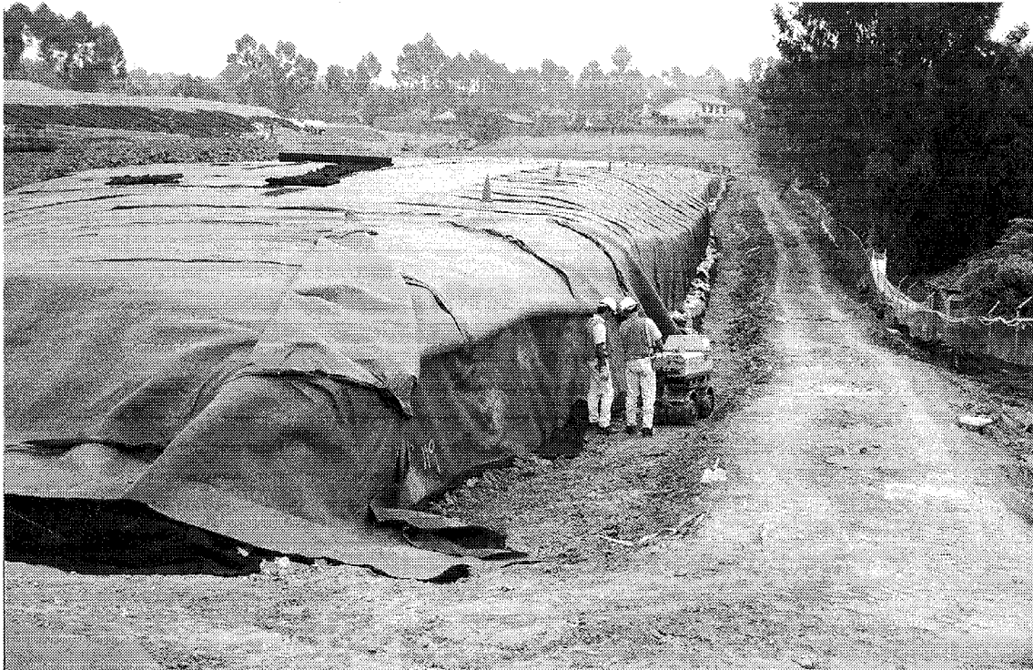
Figure 5. Completed Cover Installation over the Soldier Pile Wall
