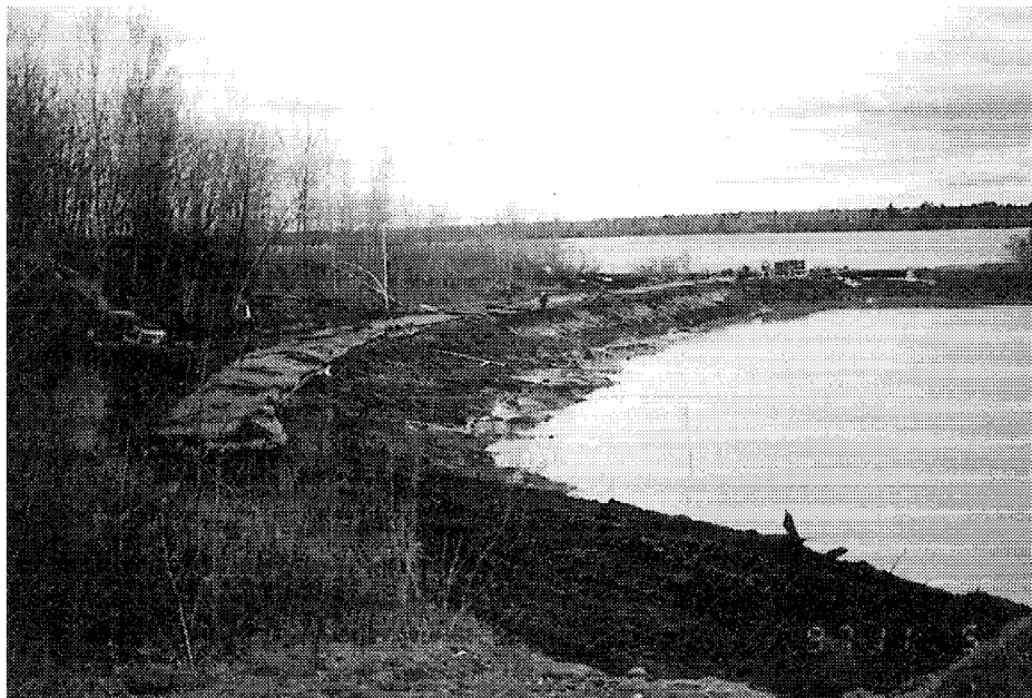
Figure 4. Geotextile on bank.
