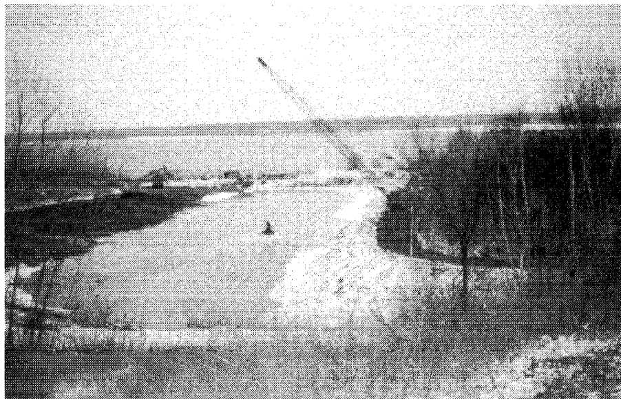
Figure 8. Photograph of Pond Backfilling.
