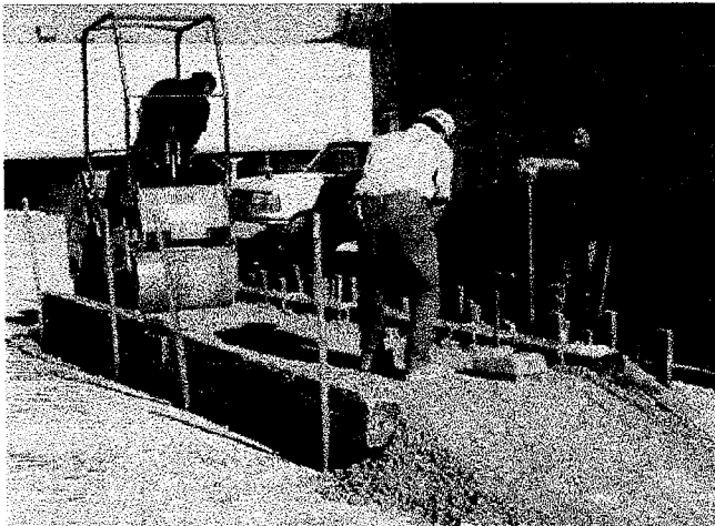
Figure 4: Secondary Compaction and Quality Control Testing
