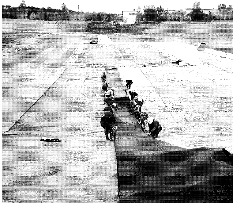
Figure 3. Photograph of PP geomembrane panel deployment
