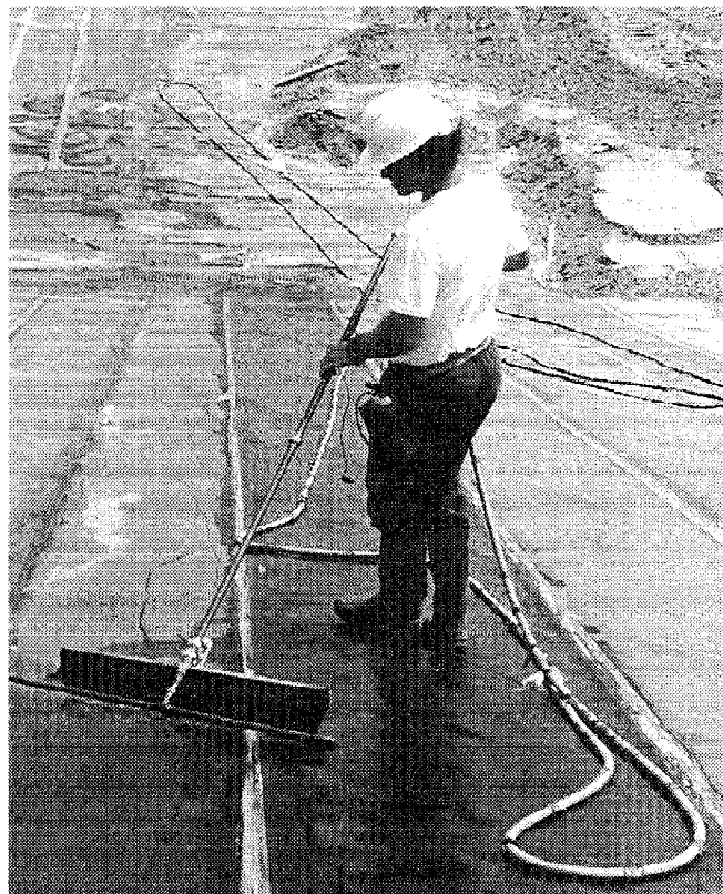
Figure 6. Photograph of an operator surveying the pond liner
