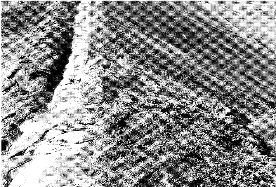
Figure 1. Trench dug to isolate cover stone from subgrade soil
