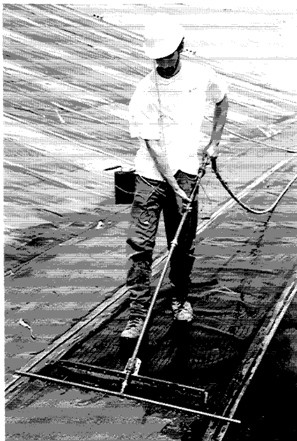
Figure 3. Geo-electrical leaks survey on uncovered geomembrane
