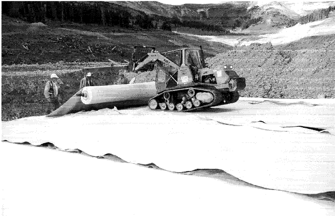
Photograph 2. Installation of capping system using rubber tracked low ground pressure vehicle operating directly on geosynthetics.
