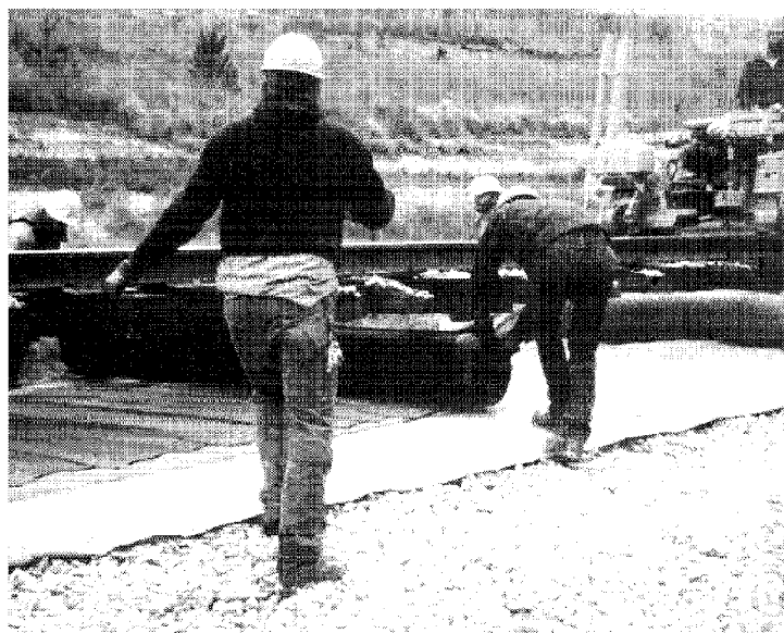
Figure 14. Geogrid Reinforcement of a Ballasted Railway Track.
