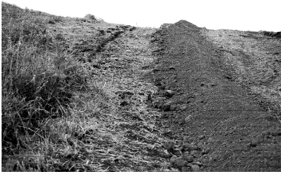
Figure 6. Earthen Berm Construction
