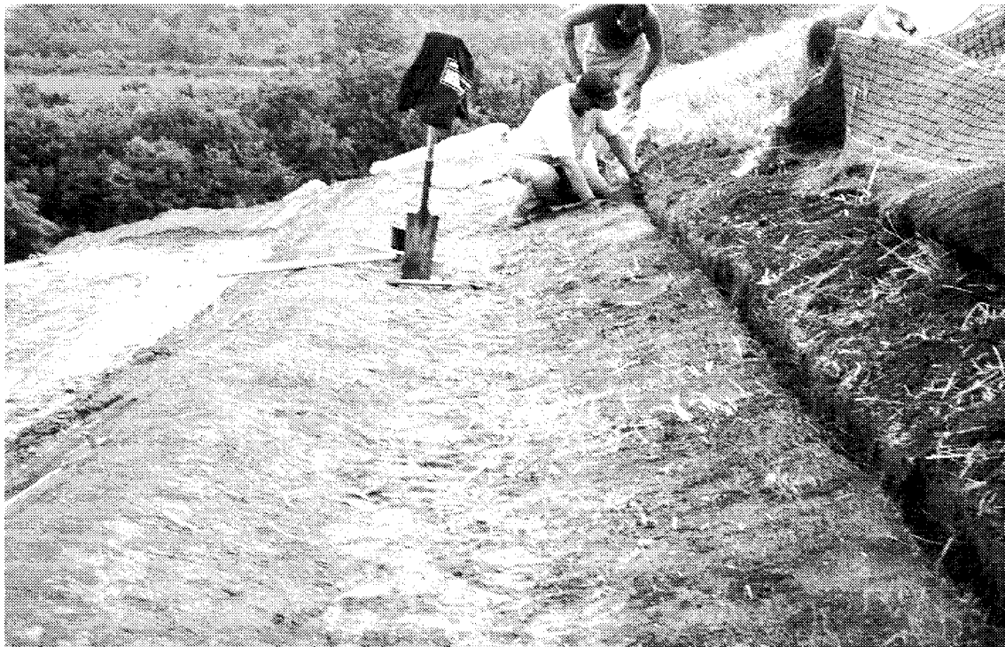
Figure 7. Turf Reinforcement Mat Installation
