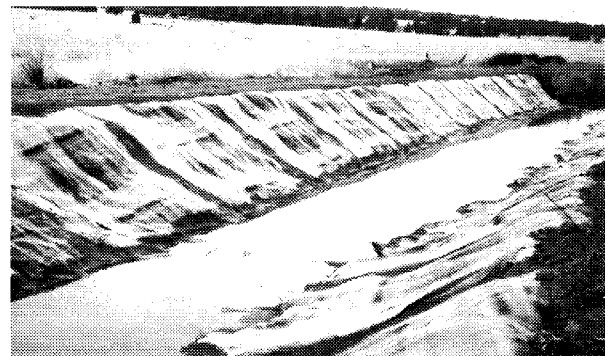
Figure 31- View of completed canal
