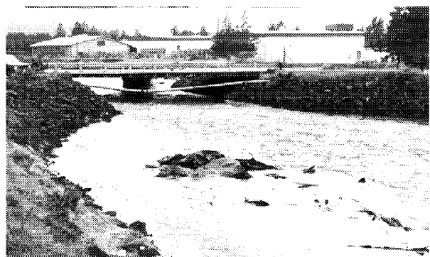
Figure 21- Lining floating downstream
