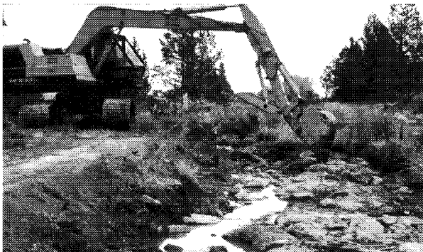
Figure 30- Trackhoe trying to excavate basalt
