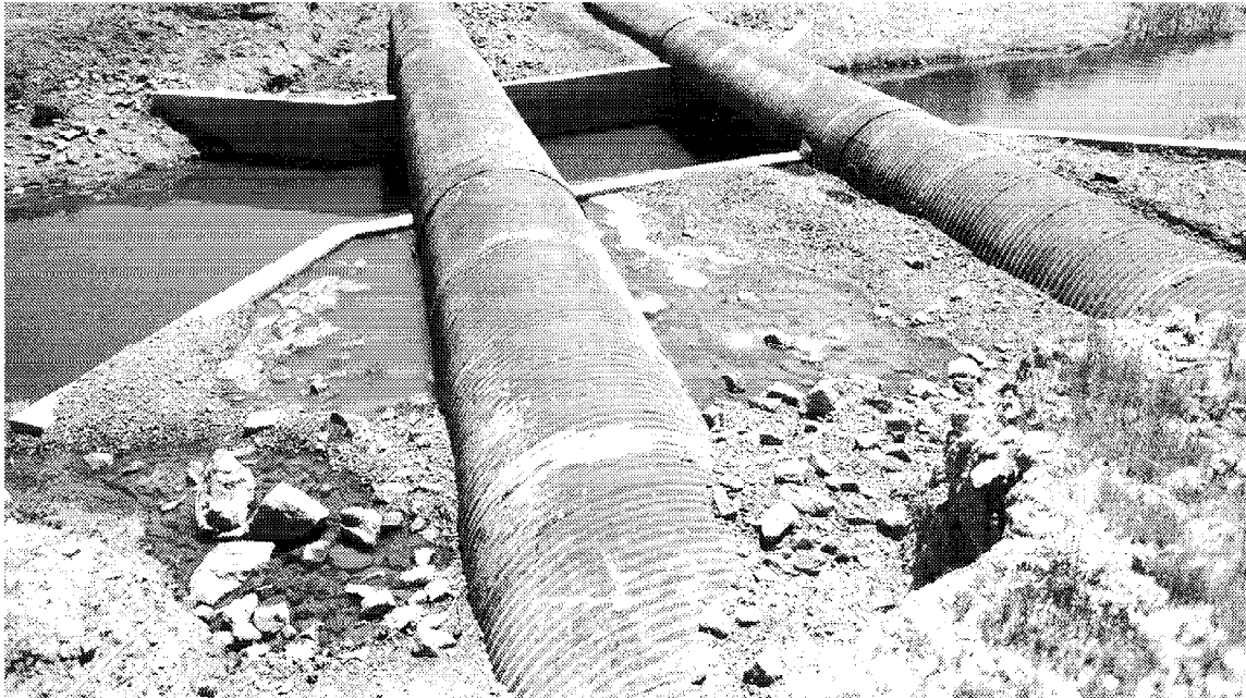
Figure 4. Pipe Bridge and Retaining Walls
