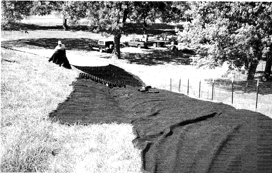
Figure 9. Construction of Temporary Roadway
