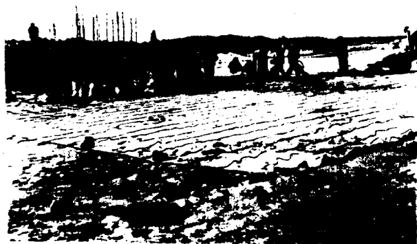
Figure 1. Sinking mattresses on ice cover
