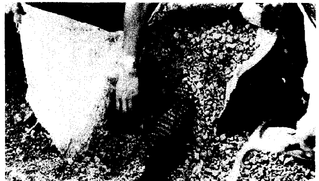
Figure 4. Open graded aggregate and pipe within geotextile.
