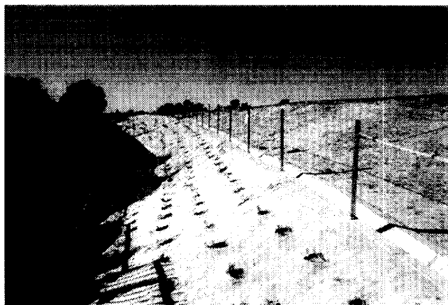
Figure 4- One of the reinforced earth structures completed during construction. Galvanized wire baskets were used to form the geogrid wrap-back earth structures.
