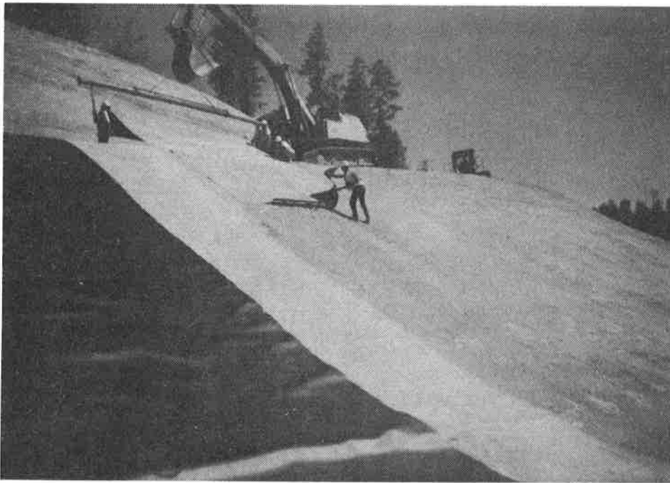
Figure 7 - Cummings Road Landfill side-slope GCL installation
