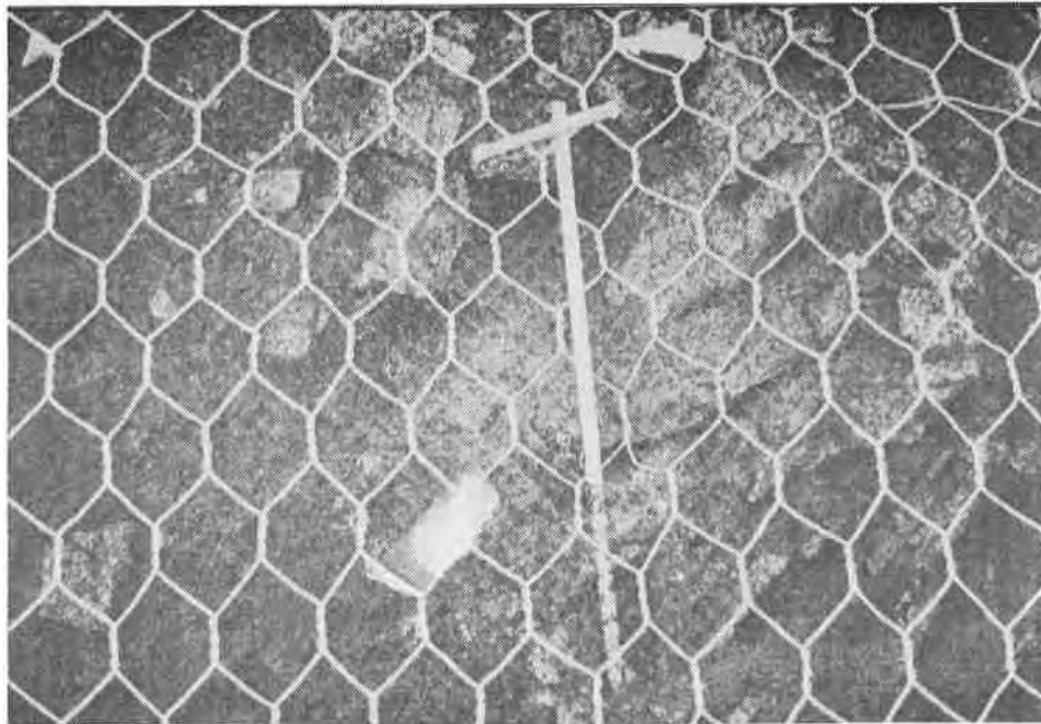
Figure 3: Rebar tee shaped anchor pins
