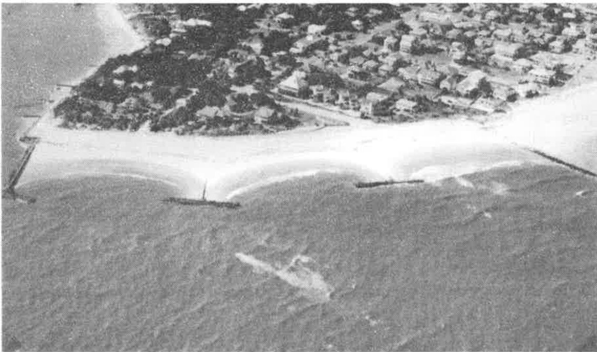
Figure 12 Groin Field (Post-Beach Fill)
