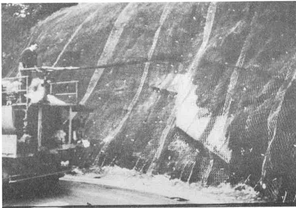
Figure 4: Hydroseeding slope face
