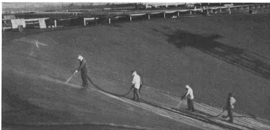
Figure 2. Application of the Polyurea Topcoat
