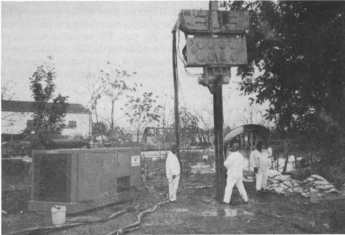
Figure 7. Installation of HDPE barrier wall utilizing conventional pile driving equipment.
