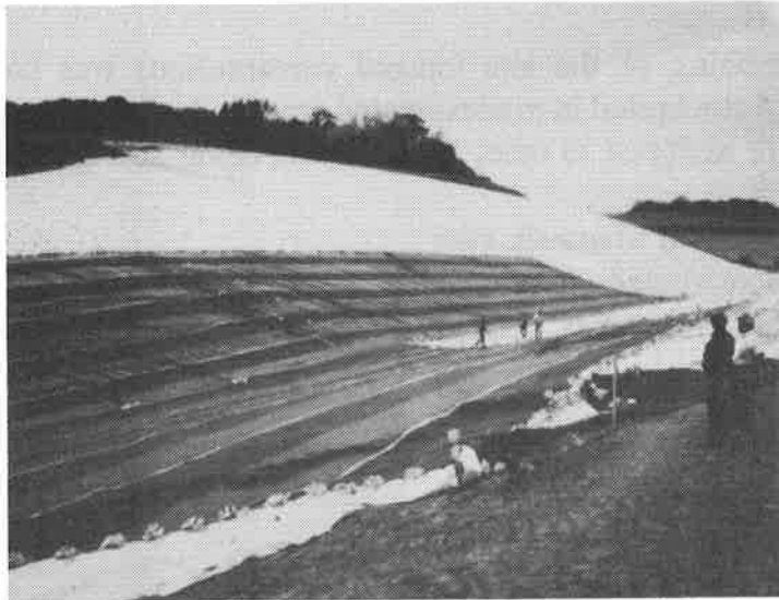
Photograph 3. Completed Sand Blanket Covered with Geotextile Followed by PVC Liner Installation.
