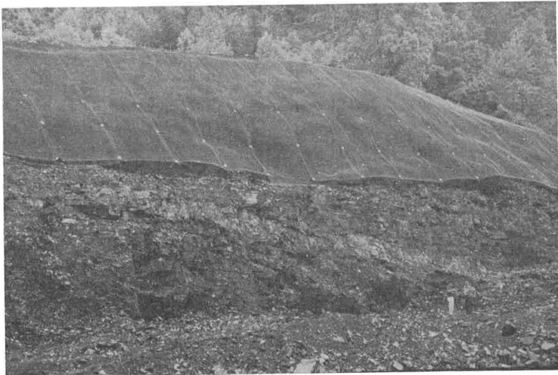
Figure 7. Partially Vegetated Slopes Three Months After Installation
