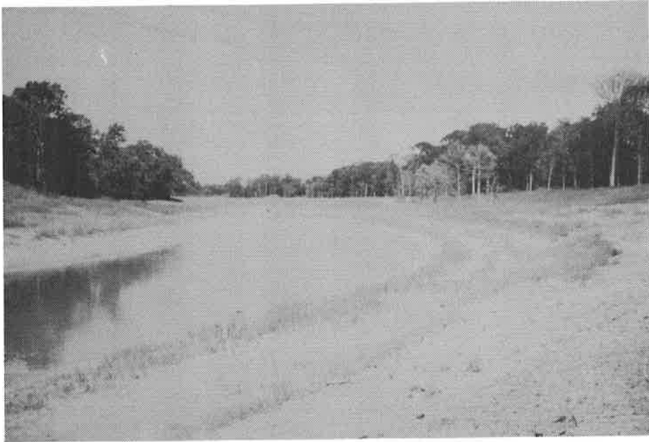
Figure 4. Photograph of Sims Bayou Channel Three (3) Months After Installation
