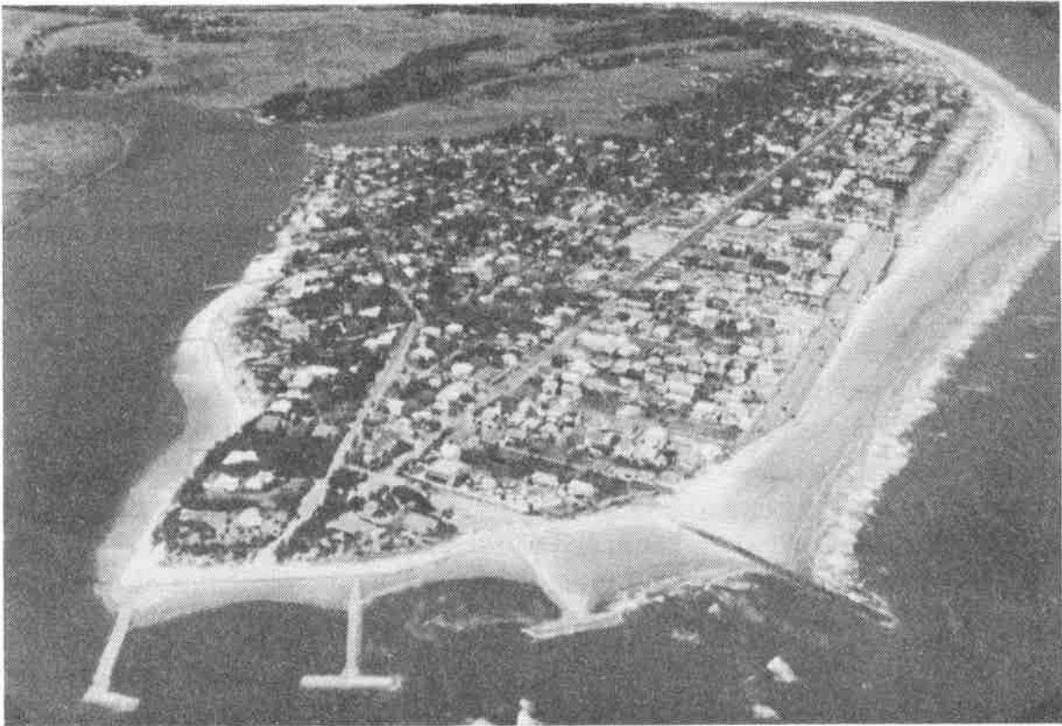
Figure 11 Groin Field (Pre-Beach Fill)
