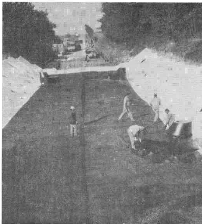
Figure 7: Installation of the first geogrid layer
