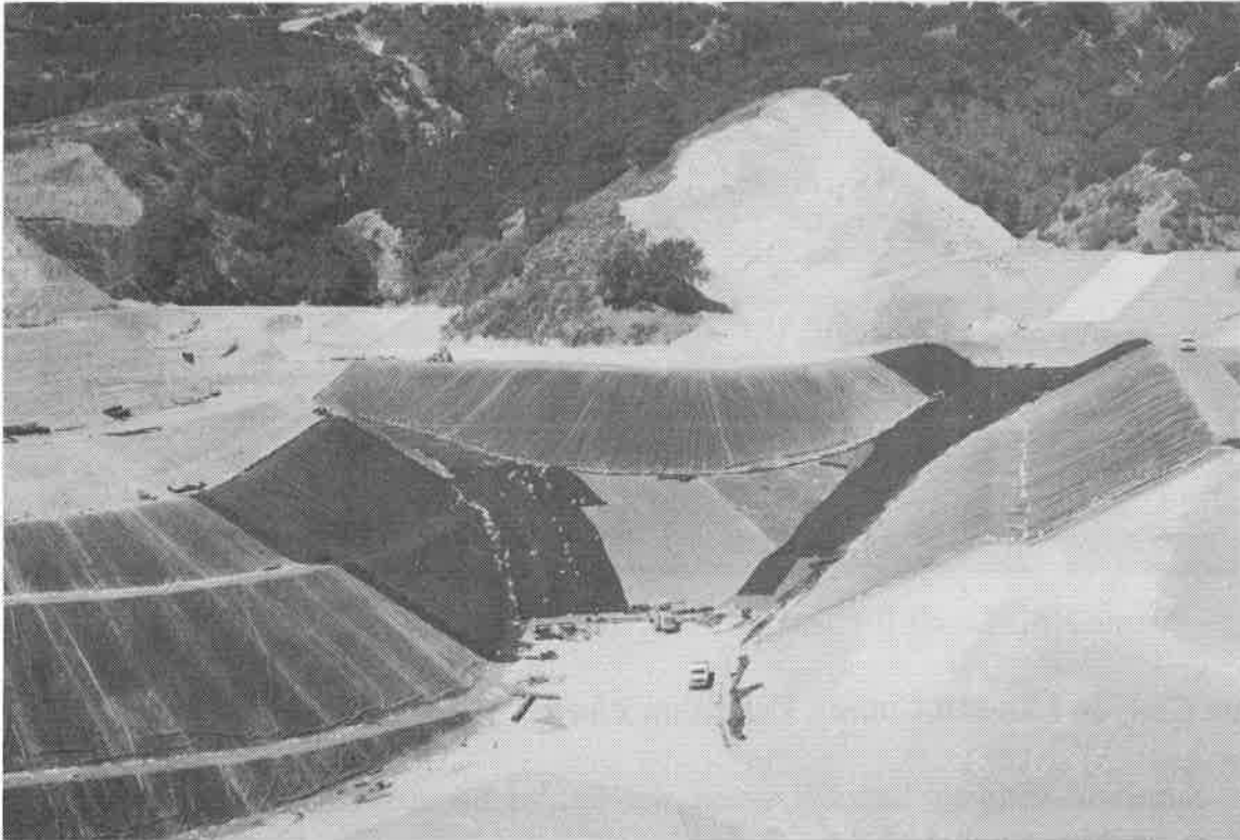
Figure 4 - Sunshine Canyon Landfill Phase I Stage 1 GCL installation
