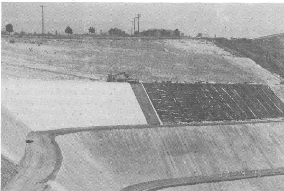
Figure 1 - Lopez Canyon Sanitary Landfill Area "C" side-slope GCL installation
