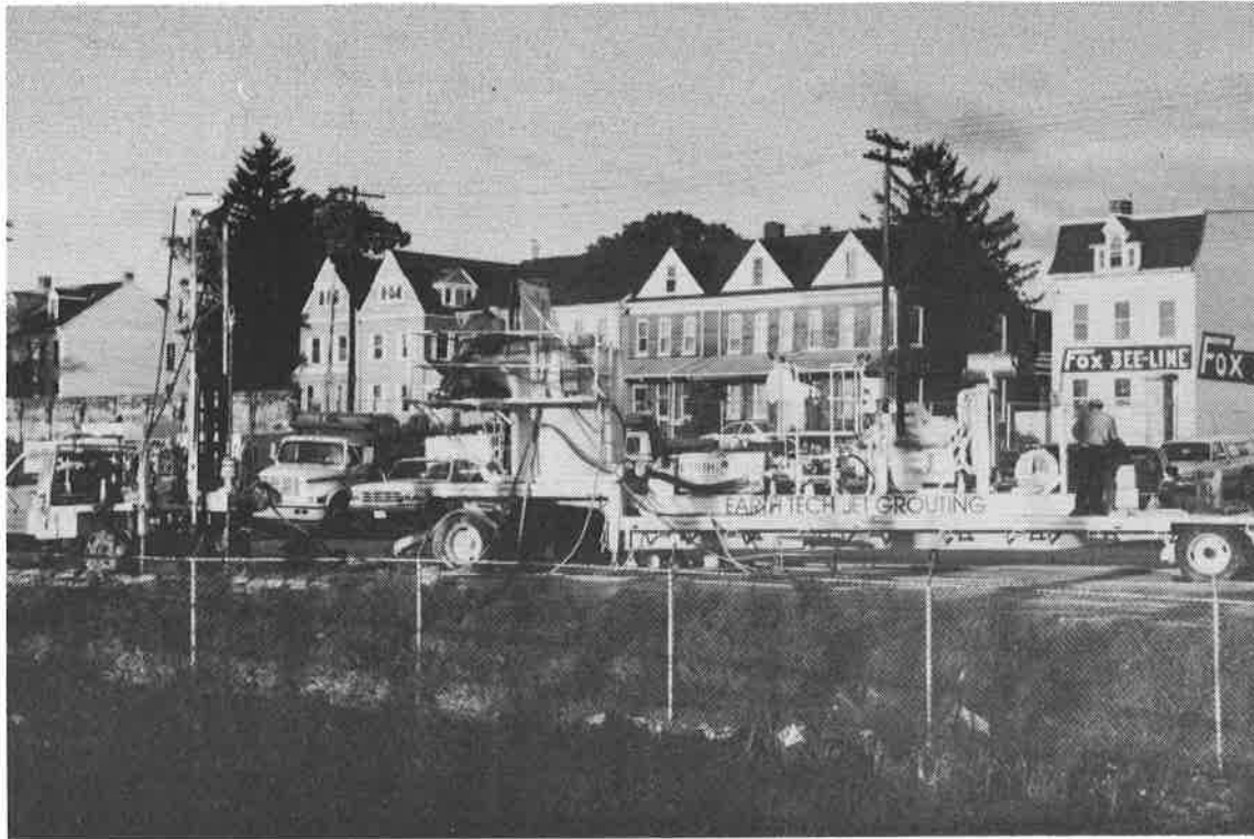
Figure 6. Trailer mounted pump and mixer.
