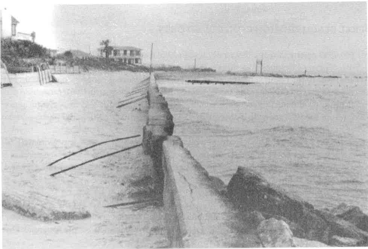
Figure 4 Pre-project Seawall Conditions (Looking Northeast)
