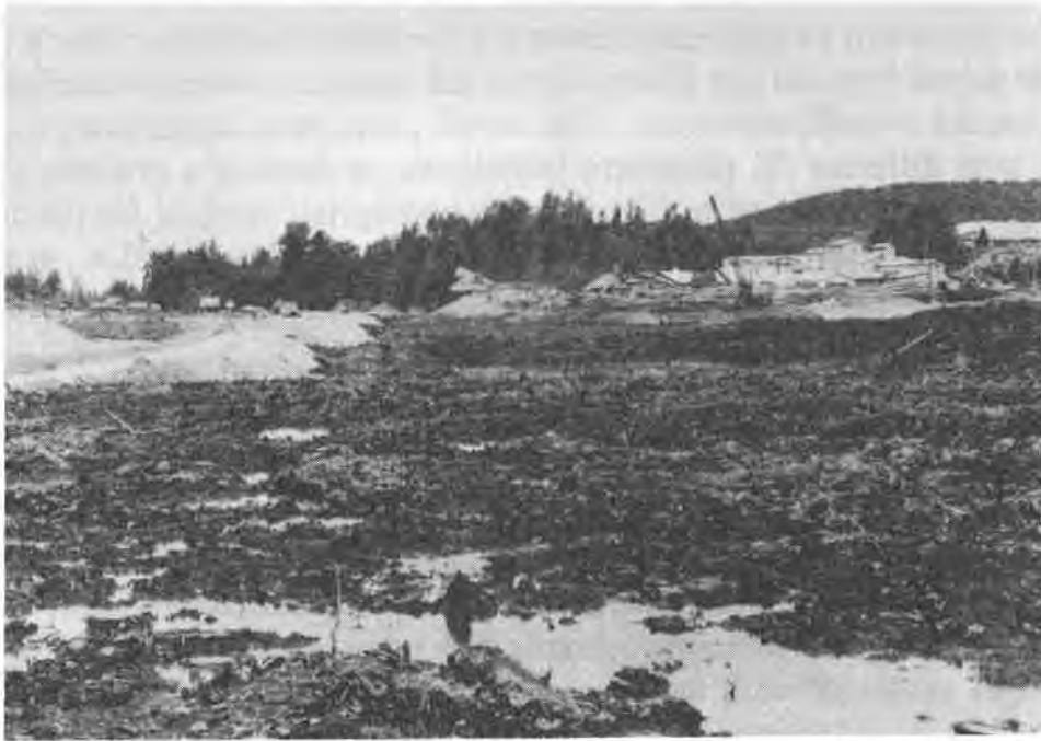
Figure 5. Condition of completed muck surface prior to geotextile placement.
