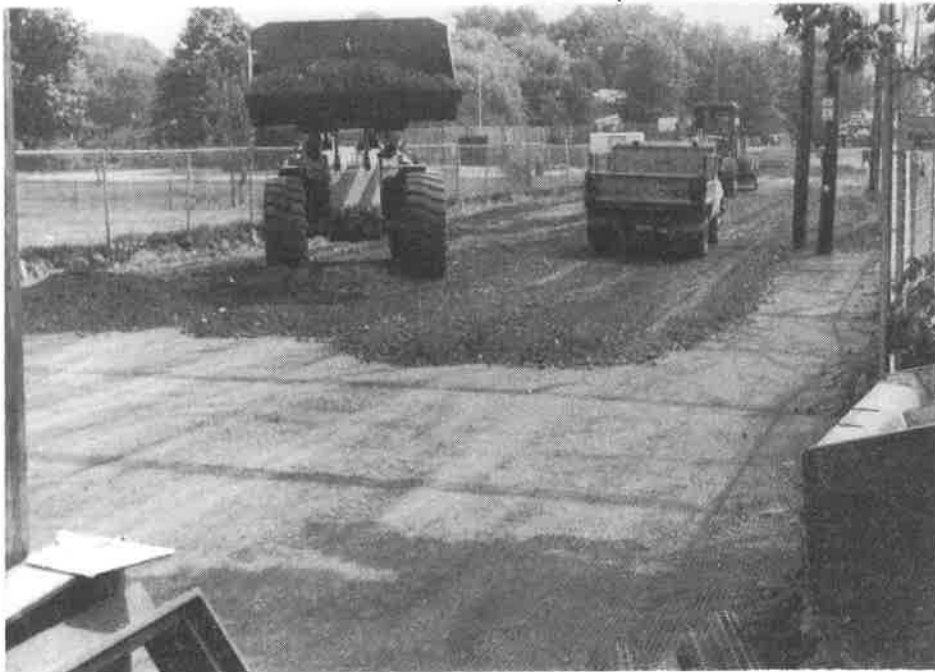
Figure 10. Fill Spread on Second Geogrid Layer
