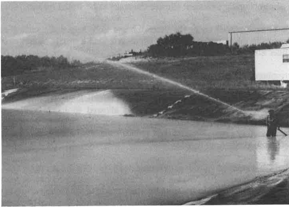
Figure 9. Spraying the Clay Slurry on the Pond
