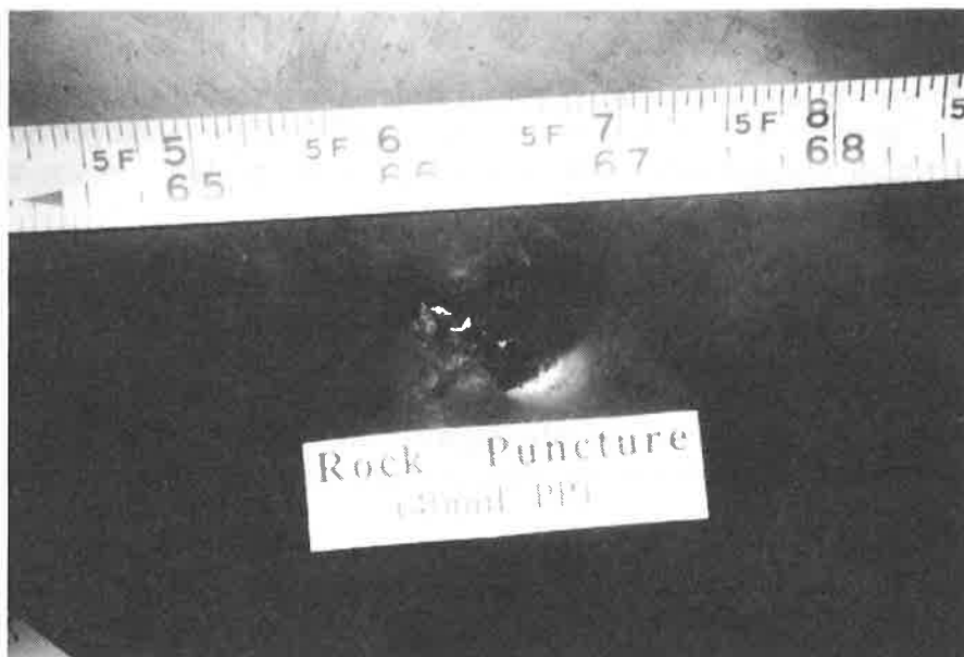
Fig. 6. Photograph of Stone Puncture in PP Geomembrane.
