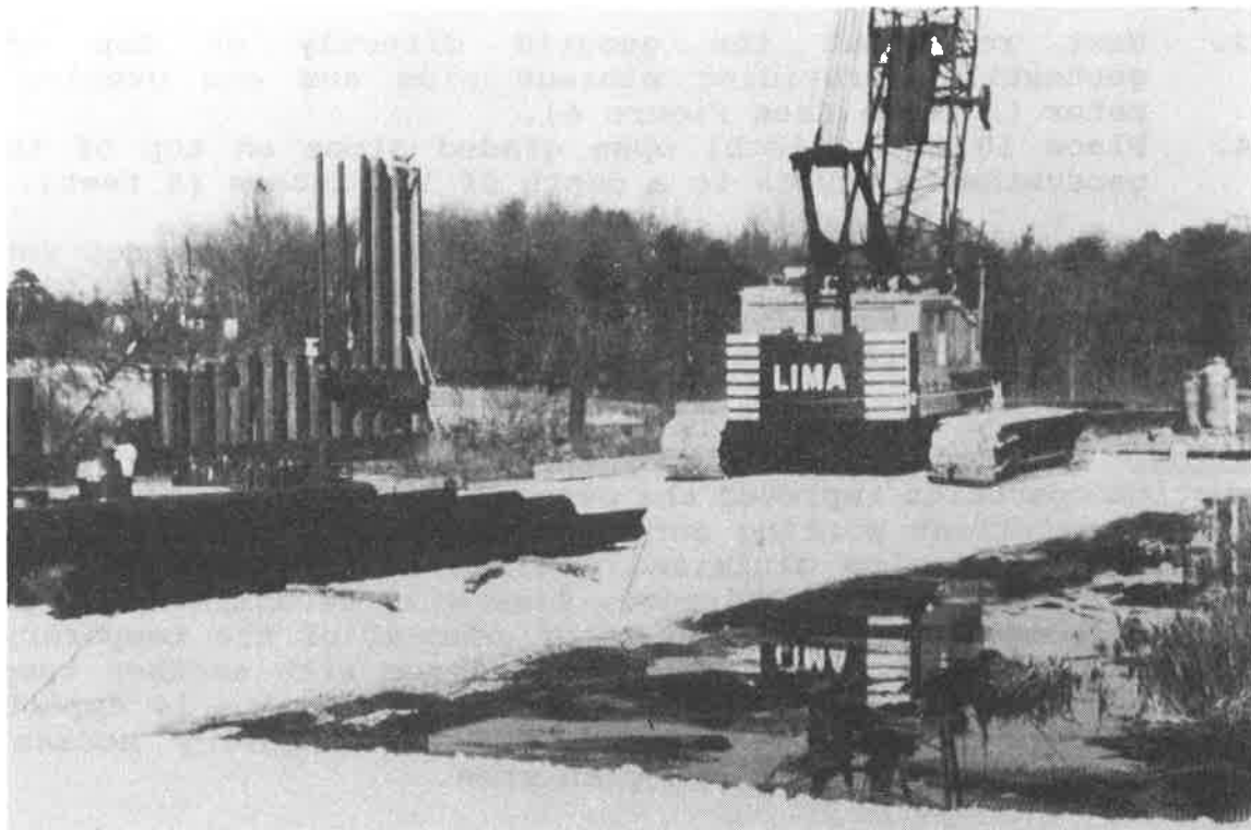
FIGURE 7. PHOTOGRAPH OF CRANE ON TEMPORARY ACCESS ROAD
