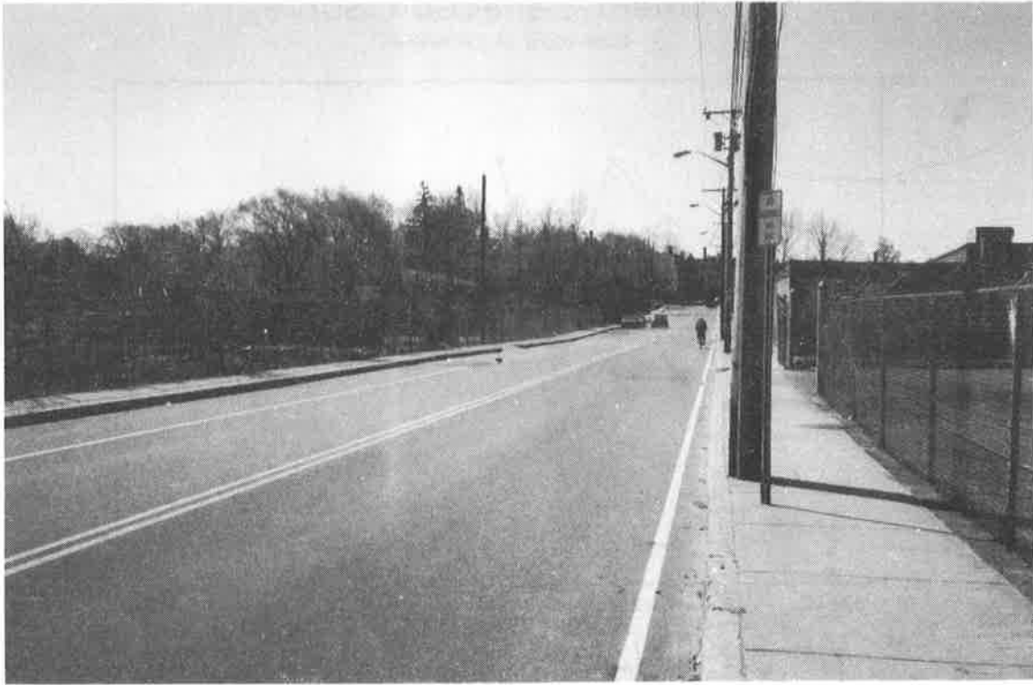
Figure 14. STA 23+00 After Construction (4/94)
