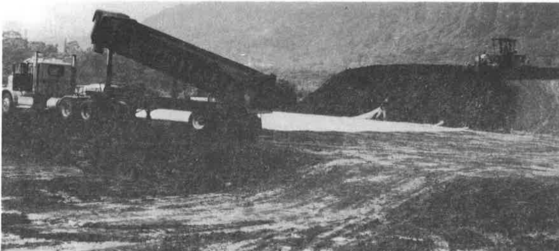
Photograph 1. Placement of Geotextile
