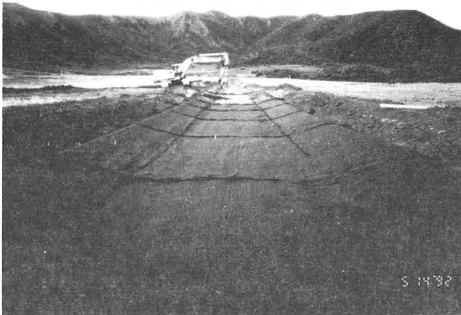
Figure 5. Upstream view of TRM installation in main drainage channel.
