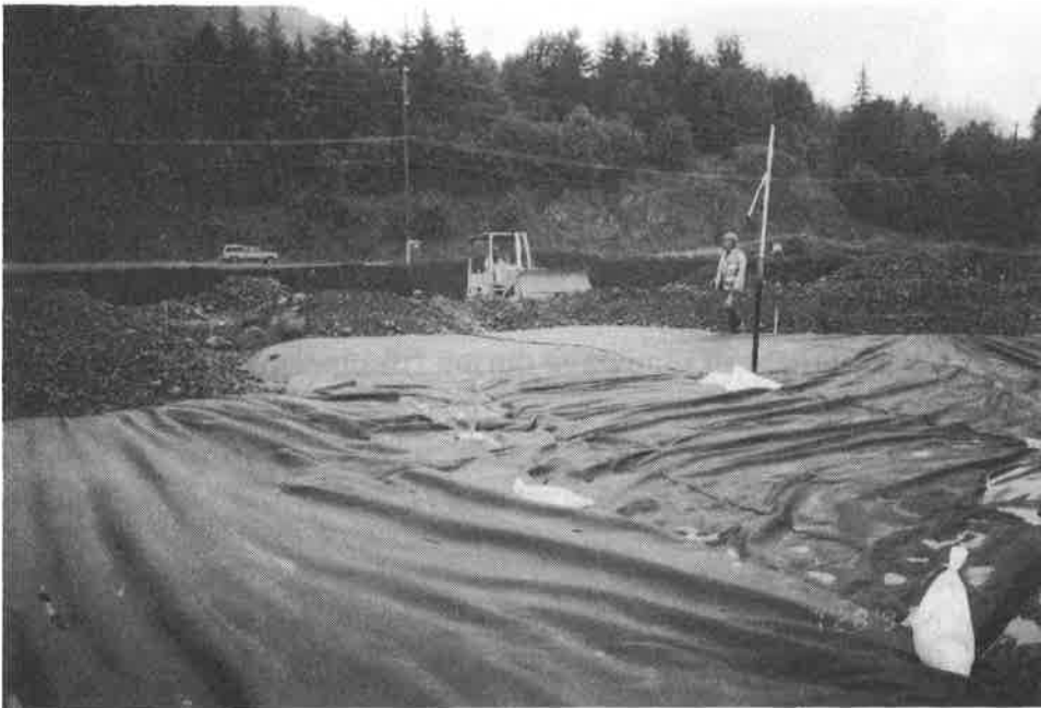
Figure 6. U-shaped fill placement technique used to contain the mudwaves.
