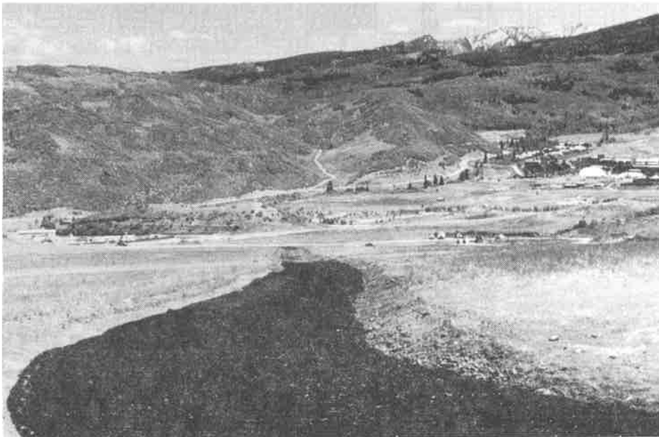
Figure 7. Main drainage channel after installation (May 1992).
