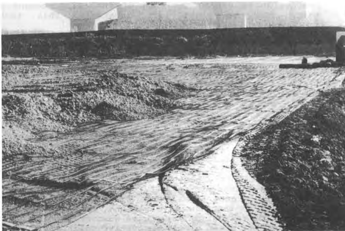
FIGURE 10. PHOTOGRAPH OF GEOGRID REINFORCED SLOPE DURING CONSTRUCTION
