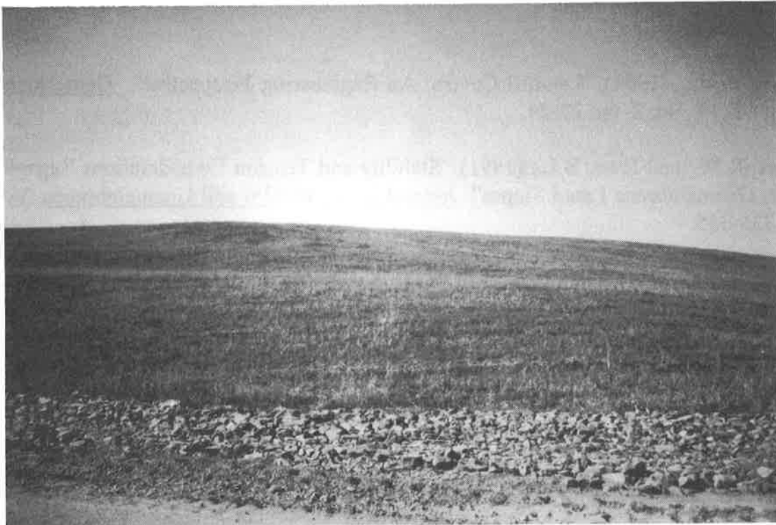
Figure 10. The Auburn, NY Landfill Number 1, South Slope Closure
