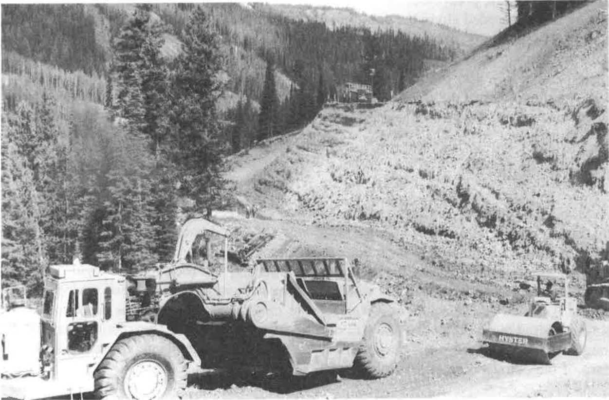
Figure 3. Rock shear key under construction
