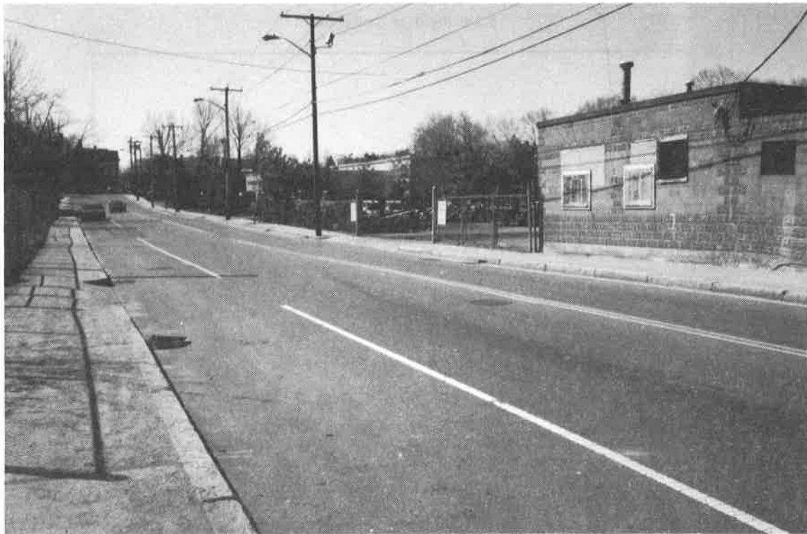
Figure 15. STA 25+25 After Construction (4/94)
