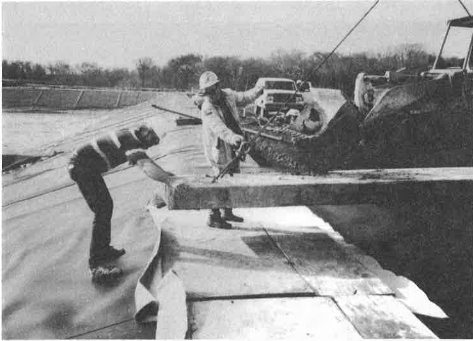
Figure 4. Protective Geofabric, Plywood, and Timber Mats Placed Over Anchor Trench
