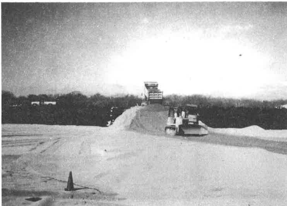
Figure 7. Spreading Gravel
