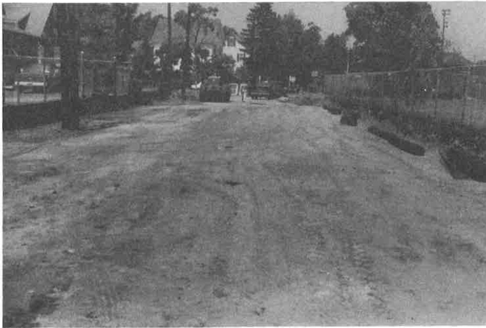
Figure 7. Prepared Subgrade
