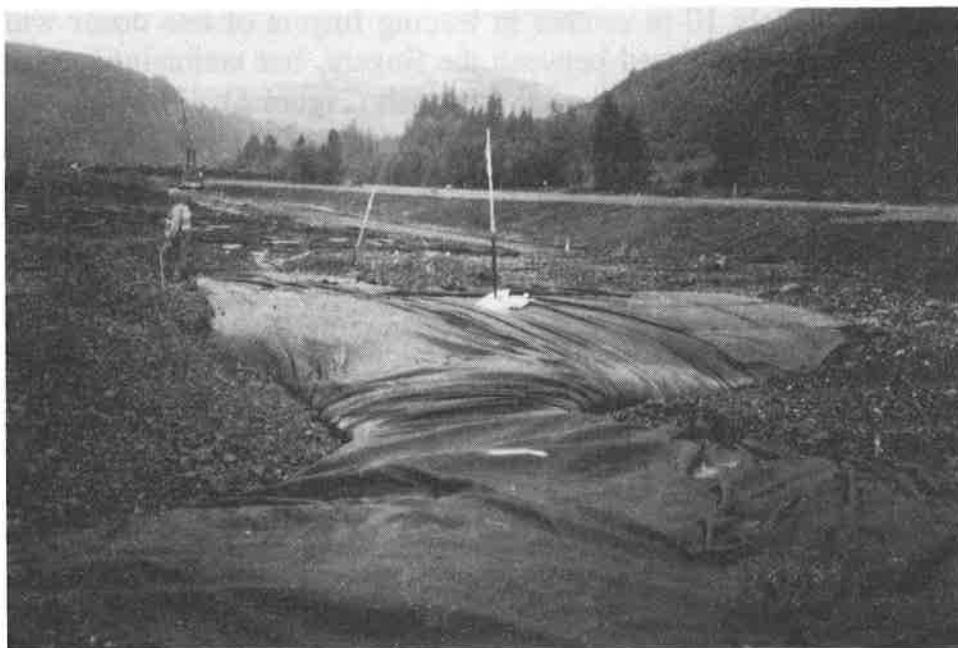
Figure 7. Development of mudwave during fill placement in the test section.
