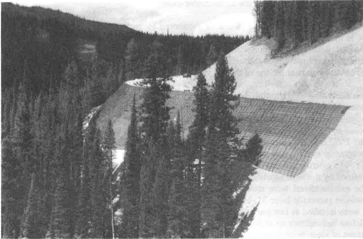
Figure 4. Finished reinforced slope with erosion matting in place
