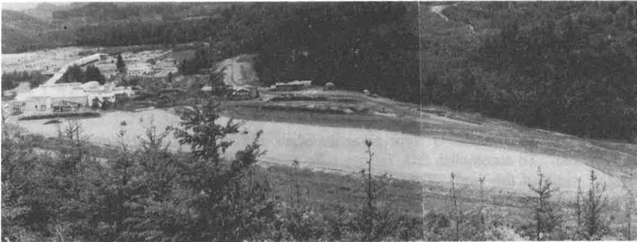
Figure 9. Completed log storage yard.
