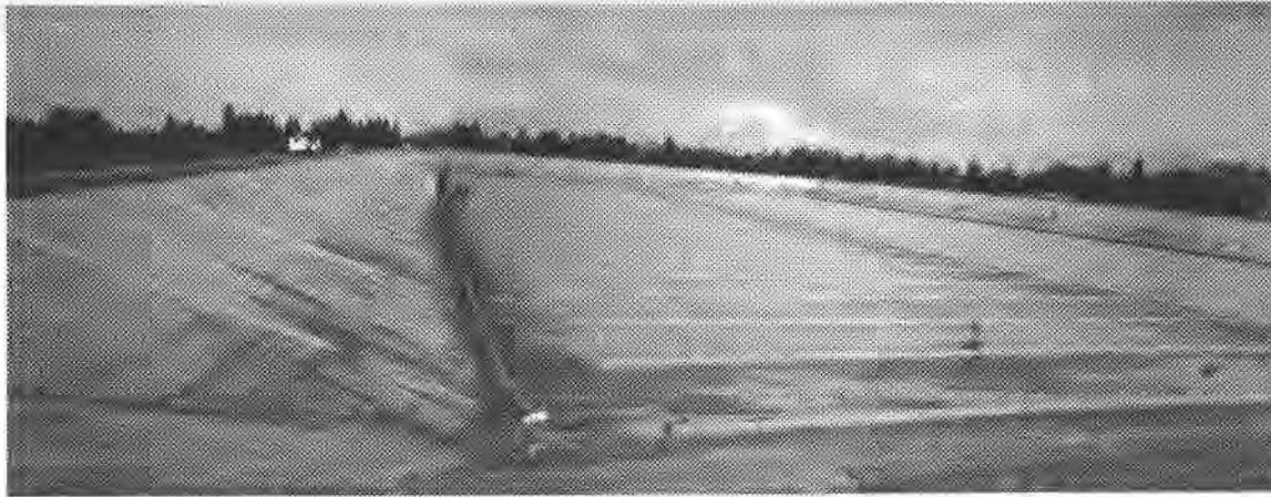
Figure 2. The Eugene reservoir, emptied for inspection.
