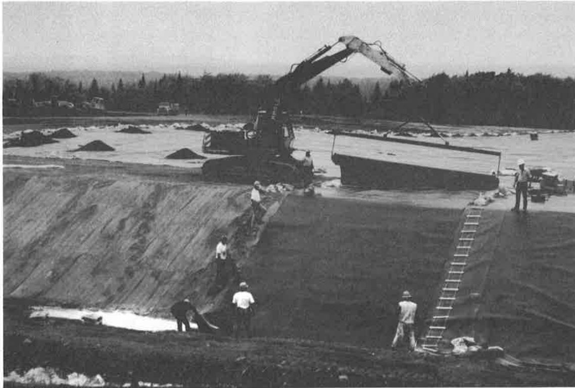
Figure 3. Placement of the geomembrane.
