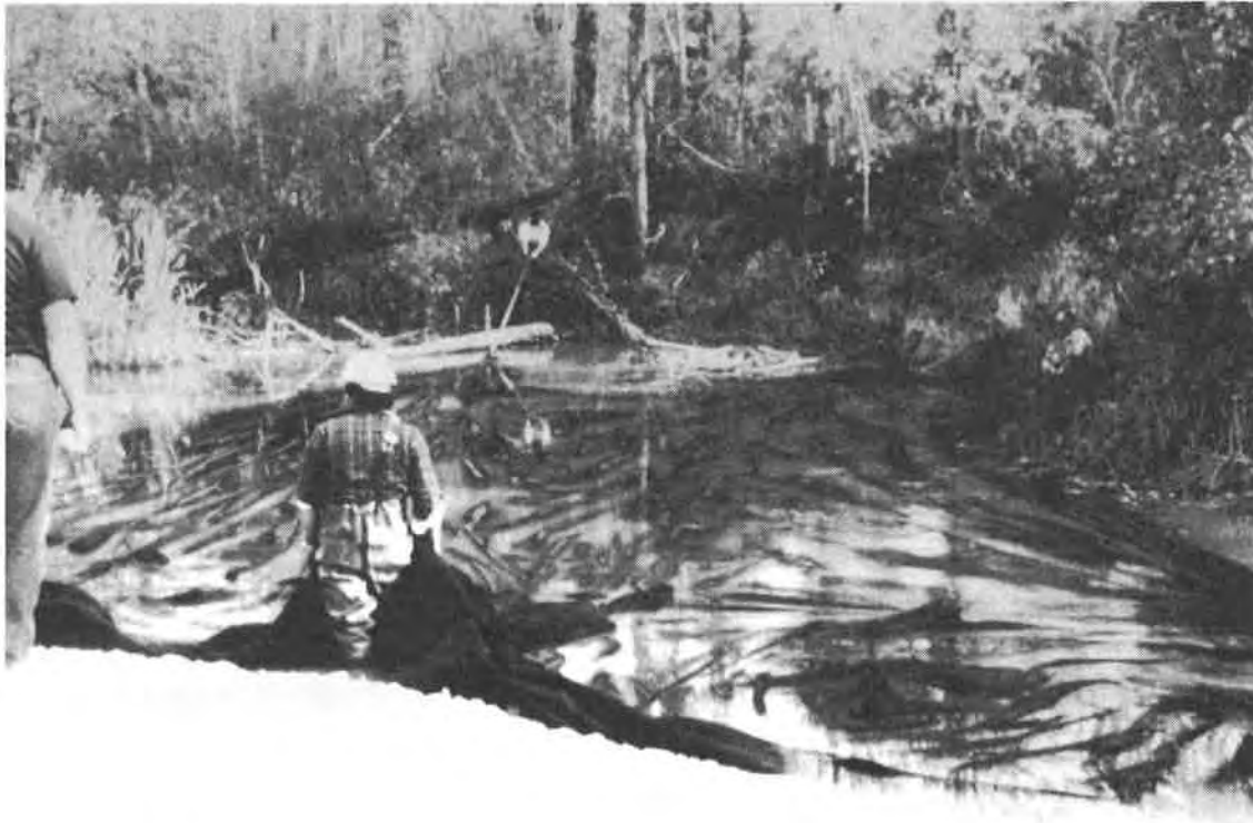
FIGURE 5. PHOTOGRAPH OF PULLING GEOTEXTILE INTO PLACE
