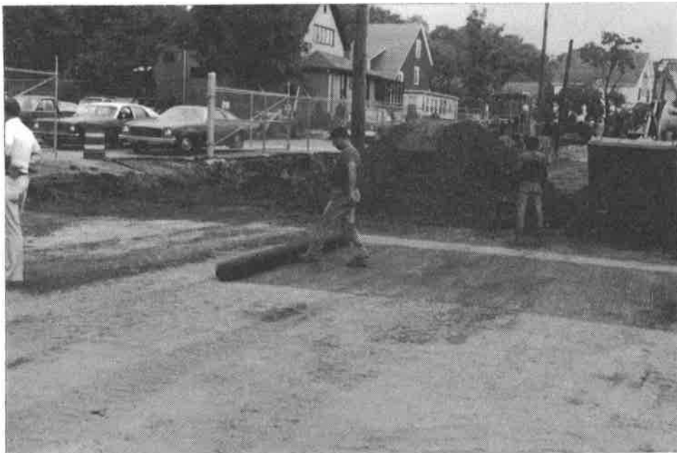
Figure 8. Placement of Geogrid
