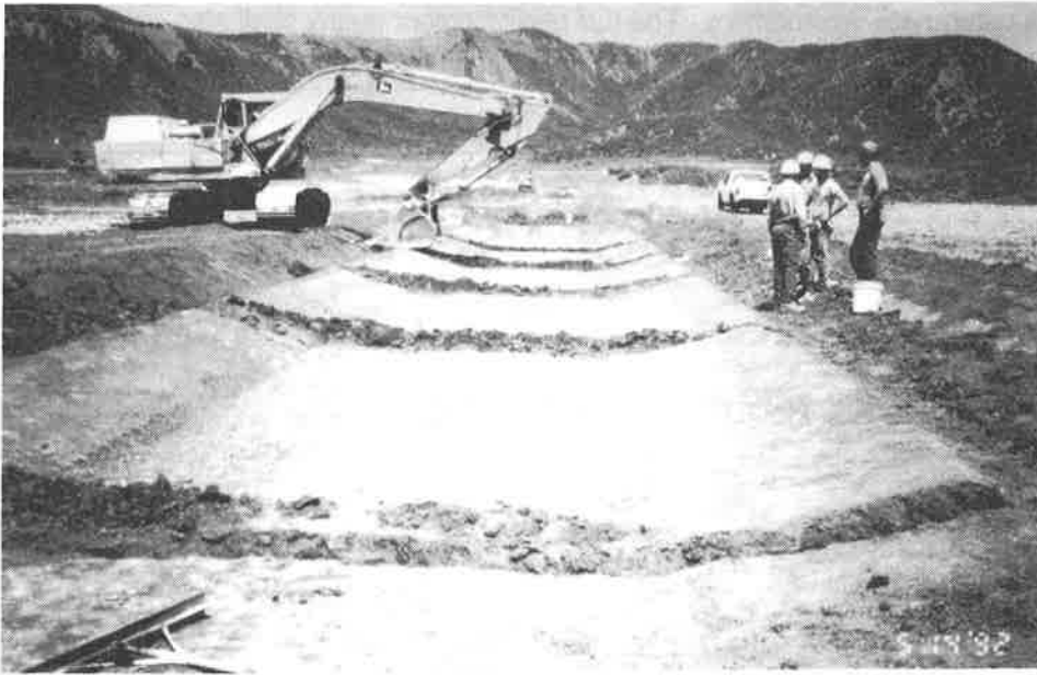
Figure 4. Construction of check slots and anchor trenches.
