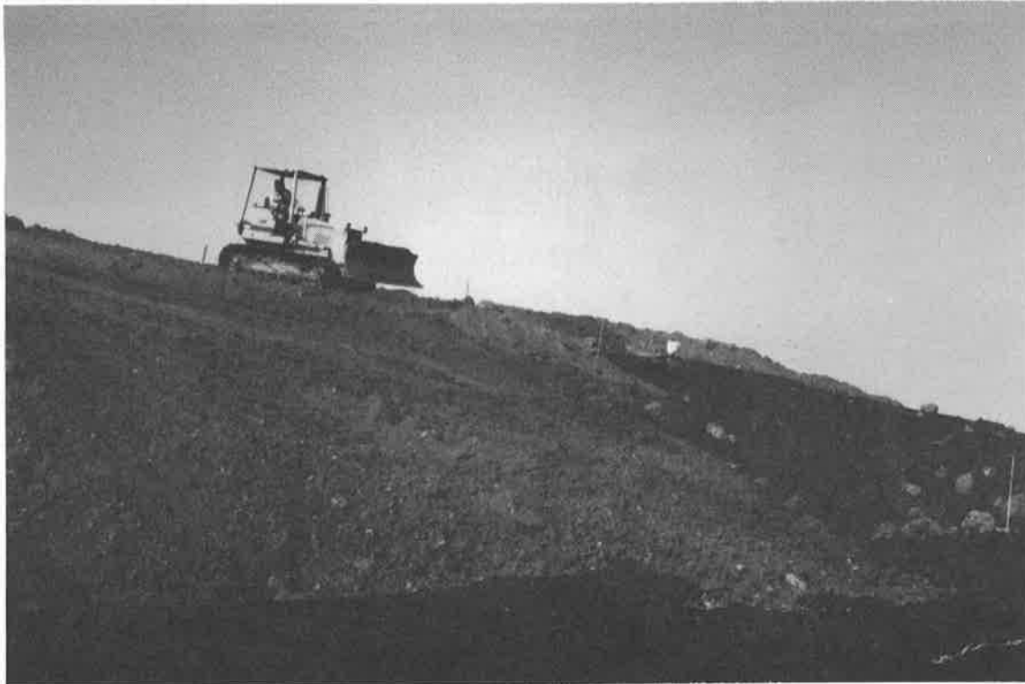
Figure 7. Placement of the barrier protection soil over the geogrid
