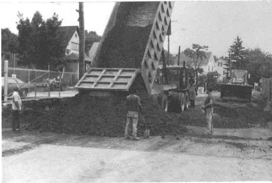
Figure 9. Placement of Fill on First Geogrid Layer
