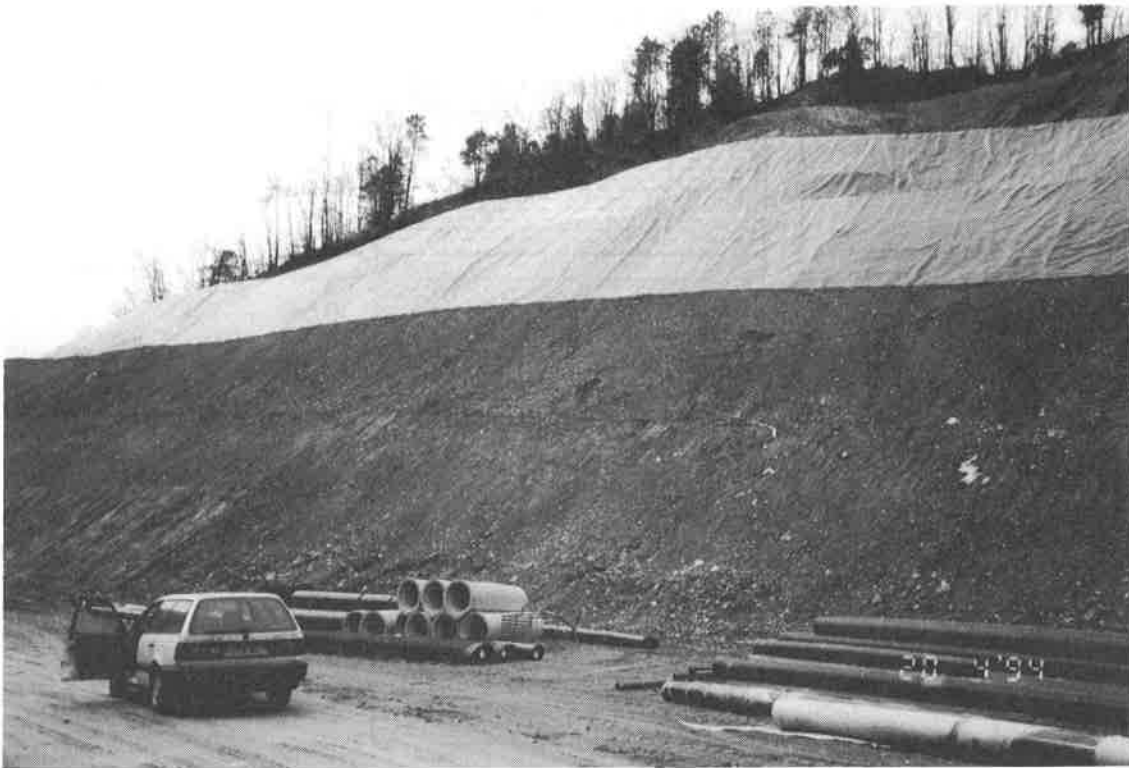
Figure 4 : SCARPINO LANDFILL - VIEW OF EMBANKMENTS DURING INSTALLATION
