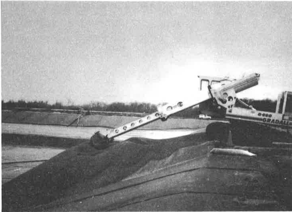
Figure 6. Push Gravel Down Side Slope to Form Temporary Ramp
