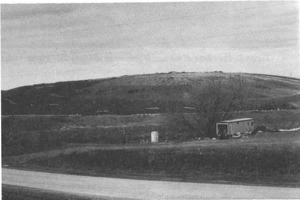
Figure 9. Overview of the Auburn Landfill barrier protection soil installation
