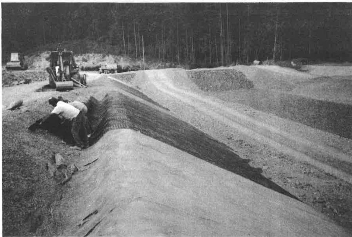
Figure 8. Installation of Geogrid Reinforcement System in Lagoon
