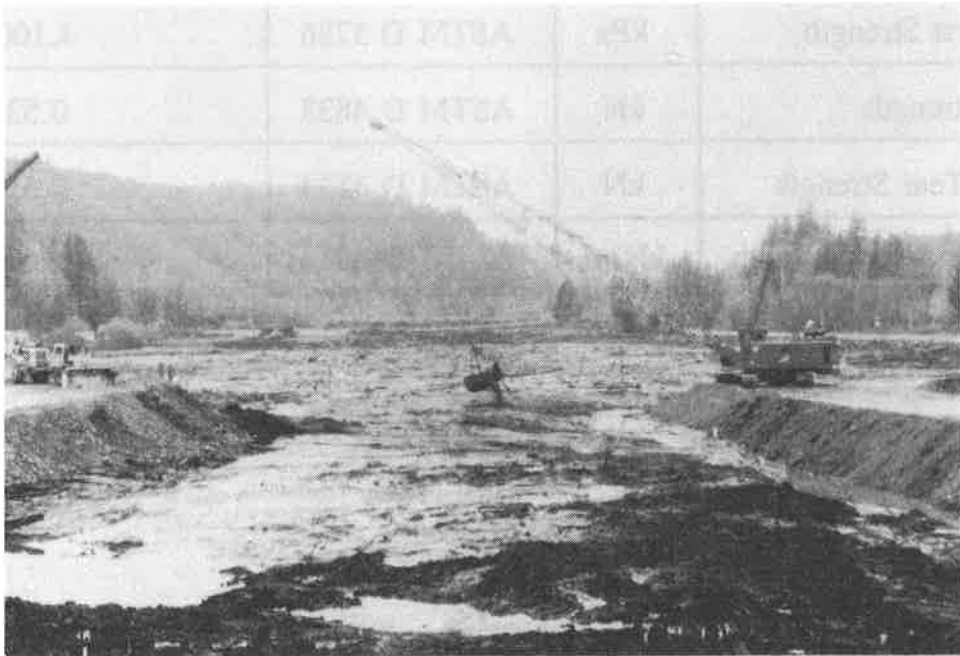
Figure 4. Condition of muck during dredging operations.
