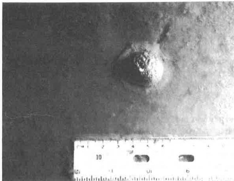
Figure 7. Clay Accumulation on 15 mm x 19 mm (0.59 x 0.75 in.) Ellipse Leak
