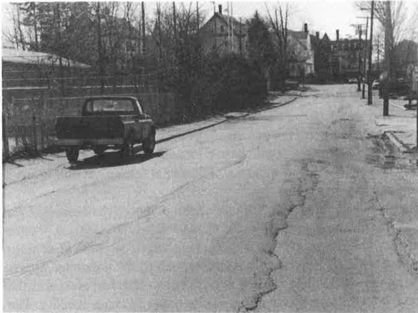
Figure 3. STA 26+50 Before Construction
