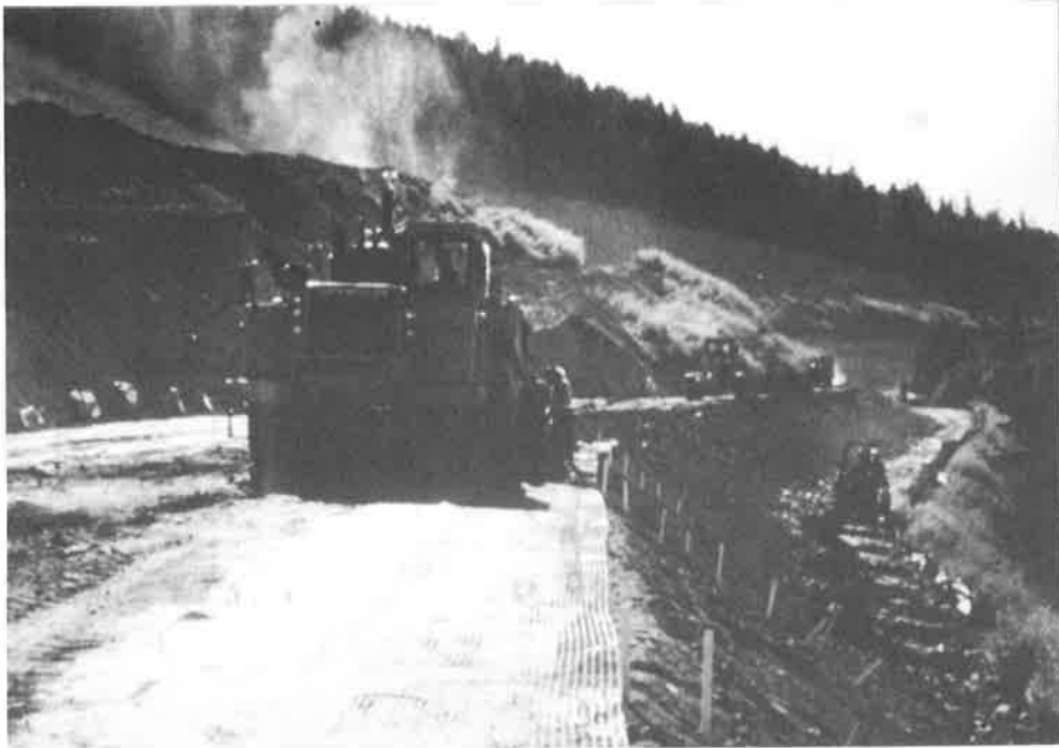
FIGURE NO. 8 - GEOGRID REINFORCED EMBANKMENT UNDER CONSTRUCTION AT DICKEY LAKE
