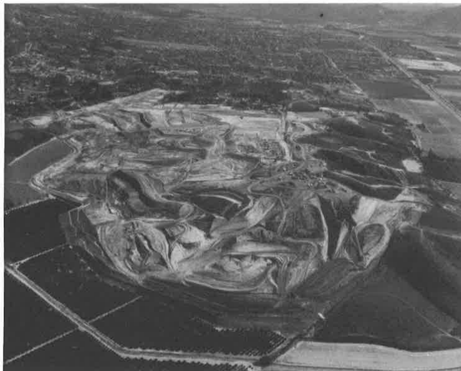
Figure 1 - Aerial View of Project Site During Construction
