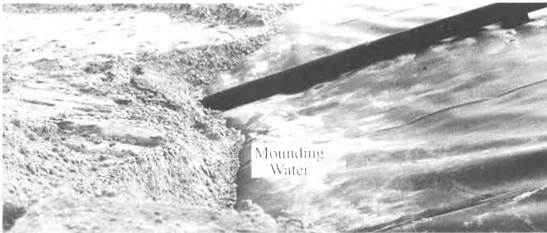
Figure 5. Area of Water Retention between the Geomembrane Liner and the Underlying Clay
