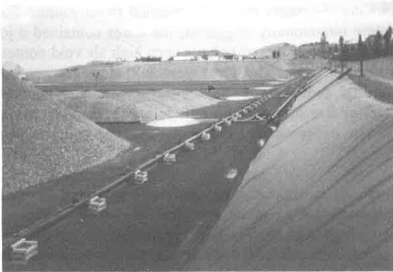
Photo 1 View of Leach Pad and Heap
