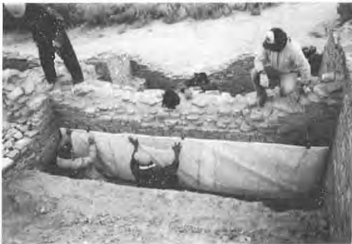
Fig. 3. Vertical Geodrain: Backfilled room during installation of geodrain (left) and cross-section through test room (right).
