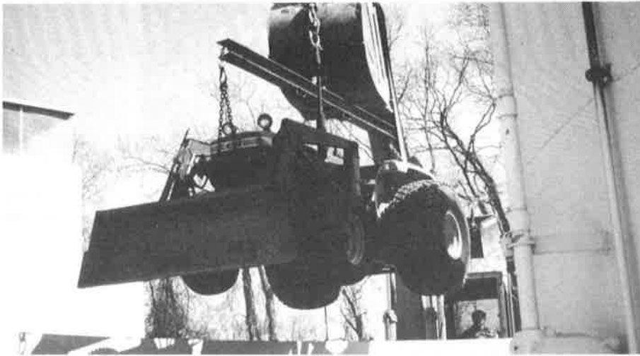
Figure 7. Crane lifting tractor into site
