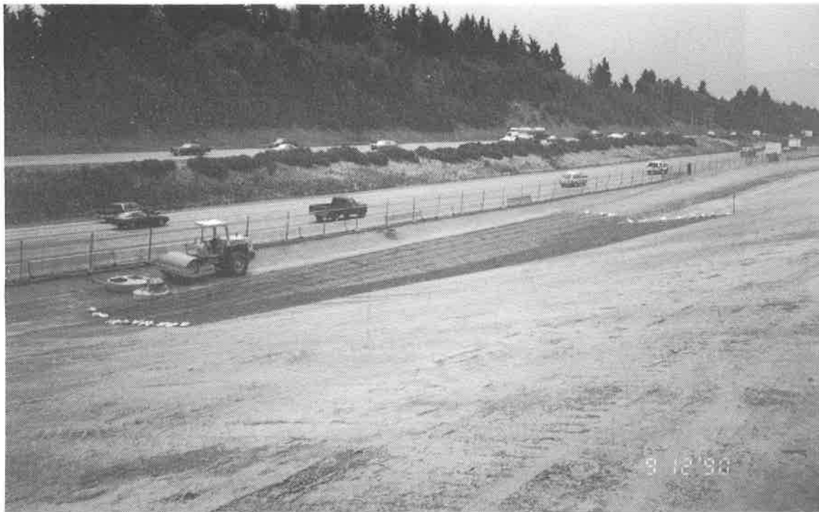
Figure 12. Geogrid Placed Parallel to Access Road Centerline
