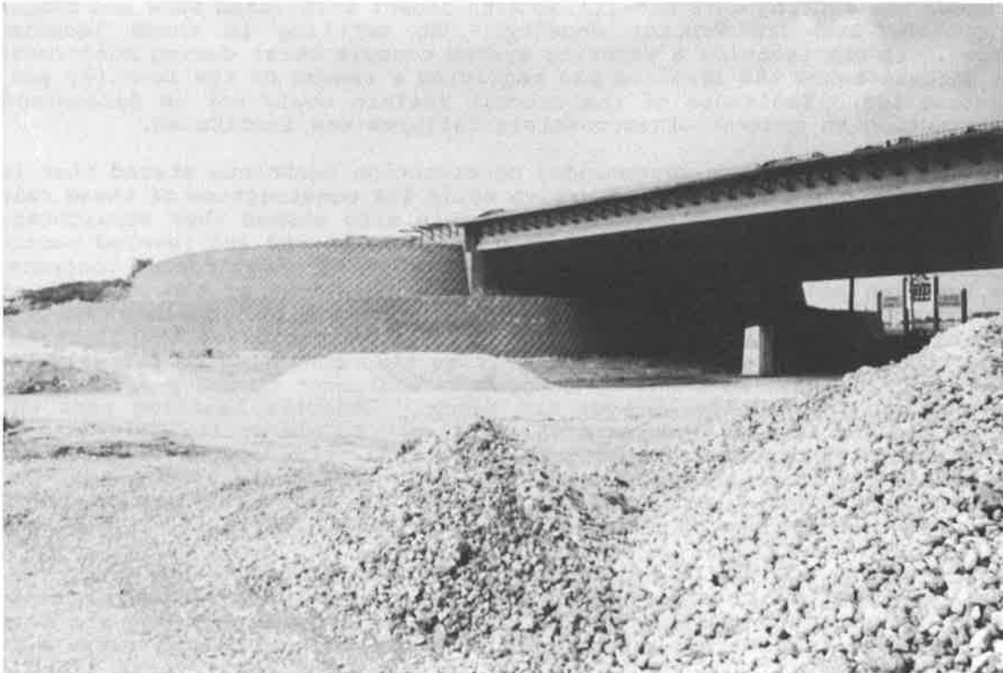
Photograph Taken Near the End of Construction at 'Fiesta Texas'
