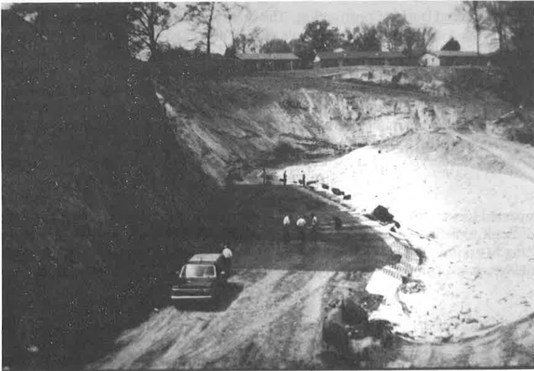
Photograph 1. Placement of Primary Geogrid
