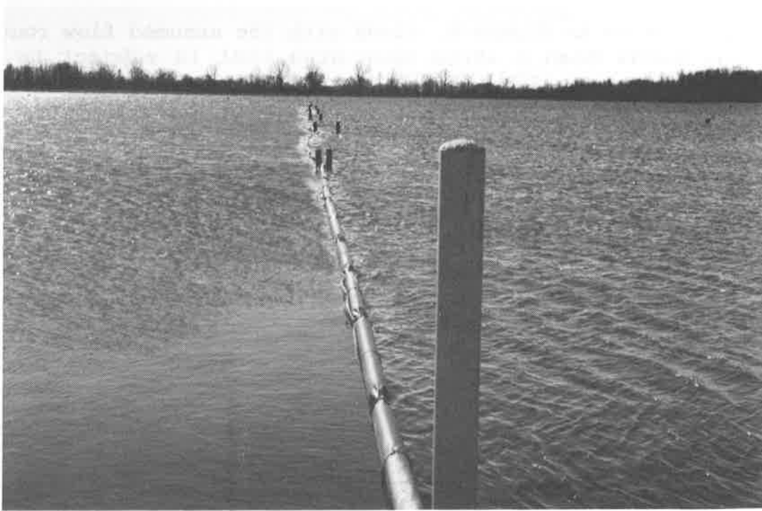
Figure 9. FDB in Municipal Wastewater Treatment Impoundment
