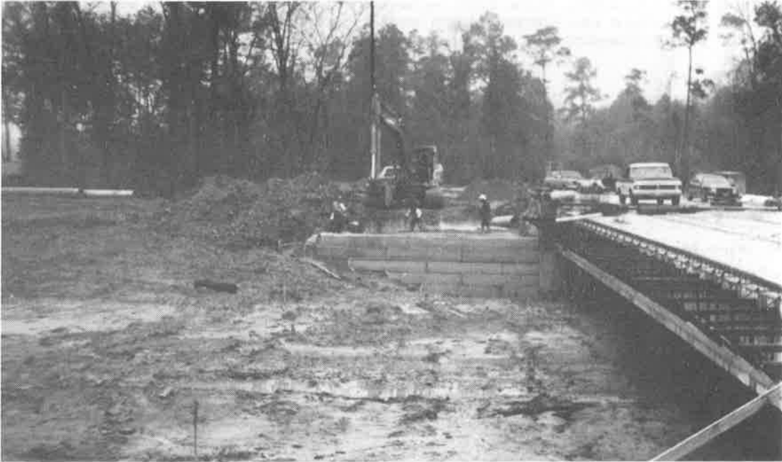
Photo 1: MSE Wire Basket Faced Wall During Construction
