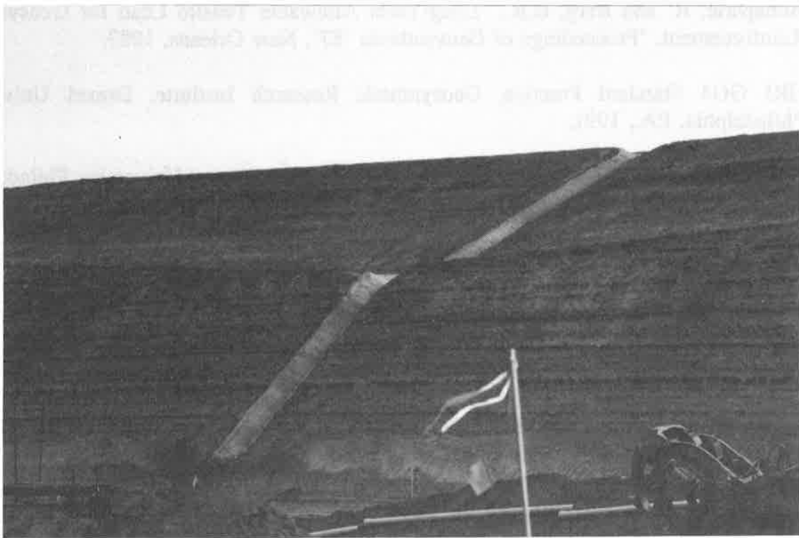
Figure 9. CONSTRUCTED SLOPE SHOWING LAYERS OF PRIMARY AND SURFICIAL REINFORCEMENT
