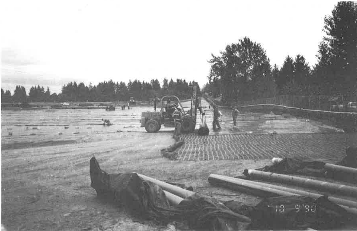
Figure 9. Geomembrane Being Placed Over Geogrid
