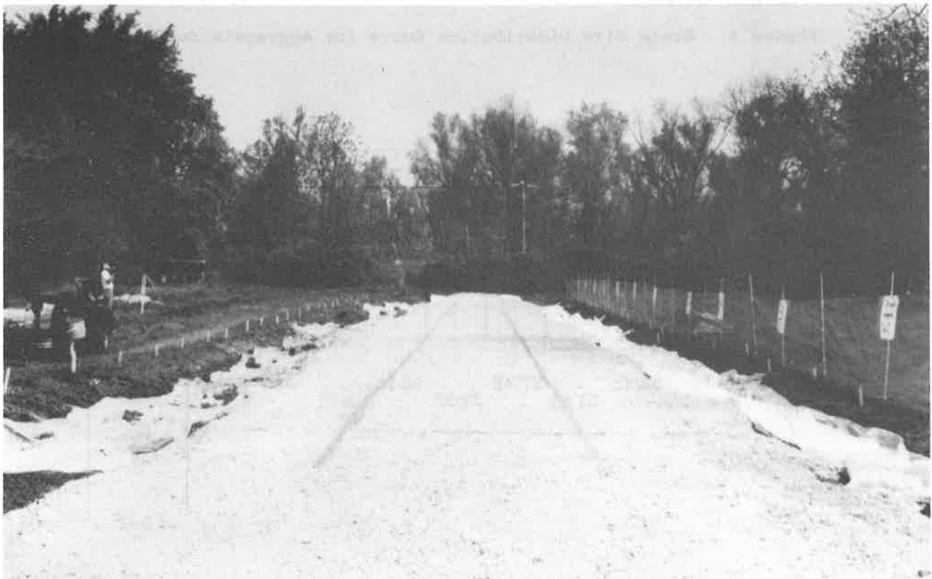
Photograph 1. Completed Test Road
