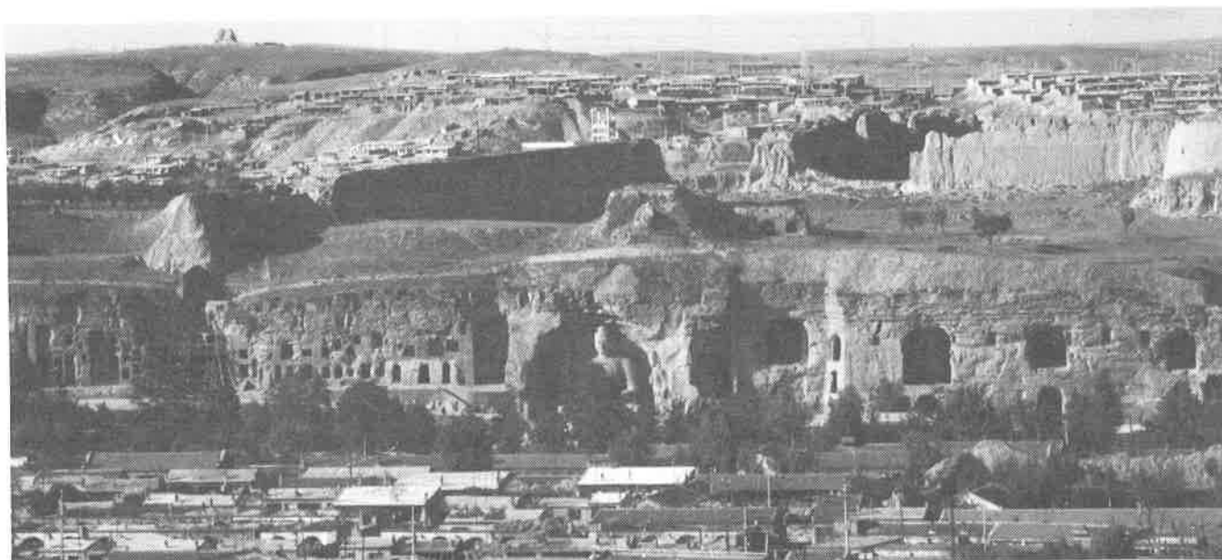
Fig. 9. The Yungang Grottoes carved in the sandstone cliff face and the Ming Dynasty fort on the plateau above.
