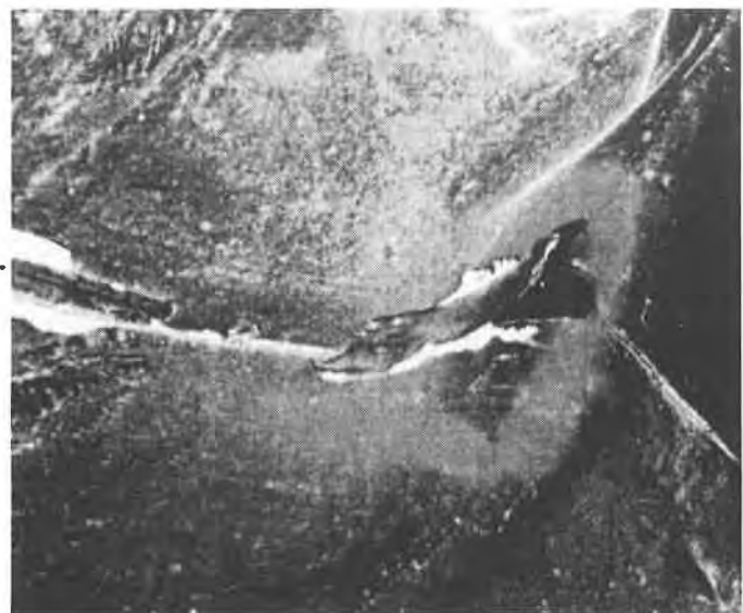
Figure 2. General view of secondary liner; note wrinkles and ponding.
