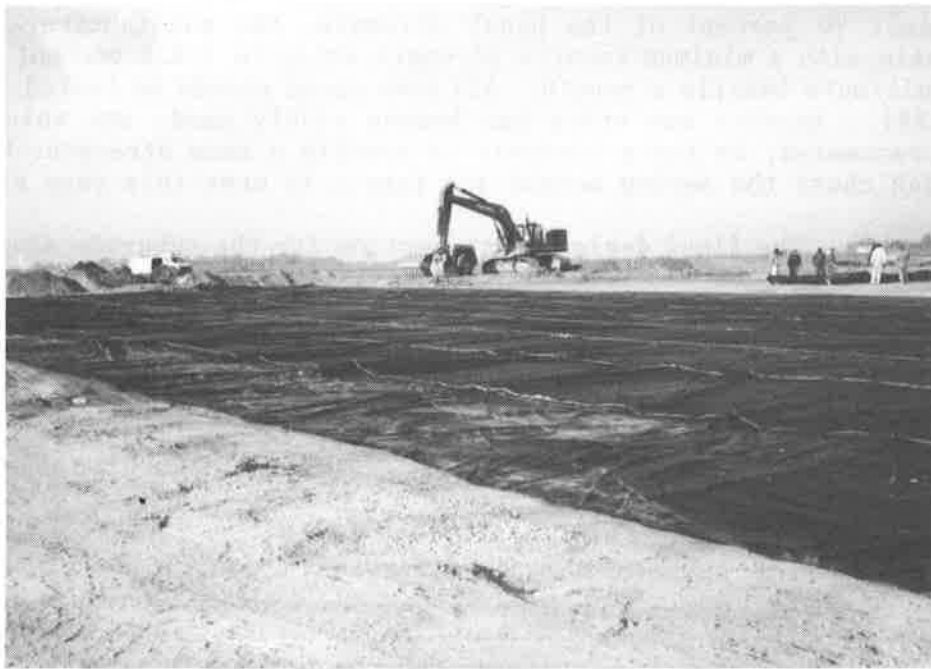
Photo 2. Pre-Sewn Geotextile Sheet In-Place.
