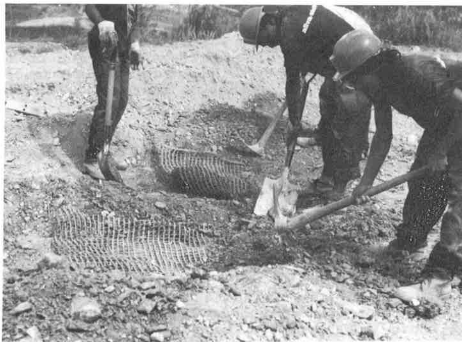
Figure 6. Hand Excavation of Geogrid using Pick Axes and Shovels
