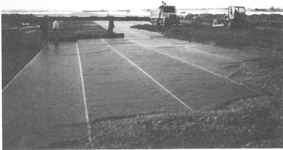
Photo 4. Installing and Backfilling Geogrids.
