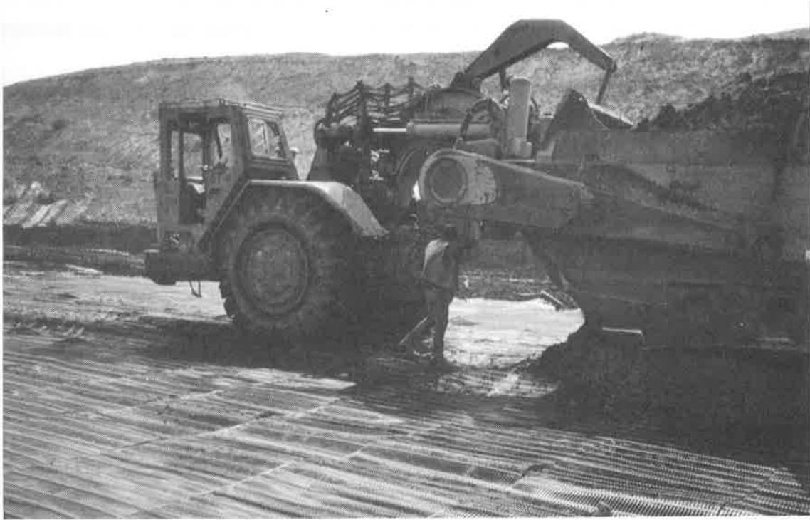
Figure 6. SCRAPER DUMPING FILL SOIL ONTO GEOGRIDS
