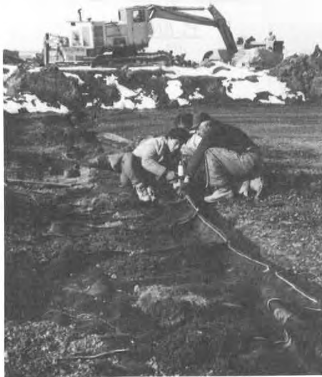
Photo 3. Attempting to Sew Perpendicular Seam Between Geotextile Sheets.
