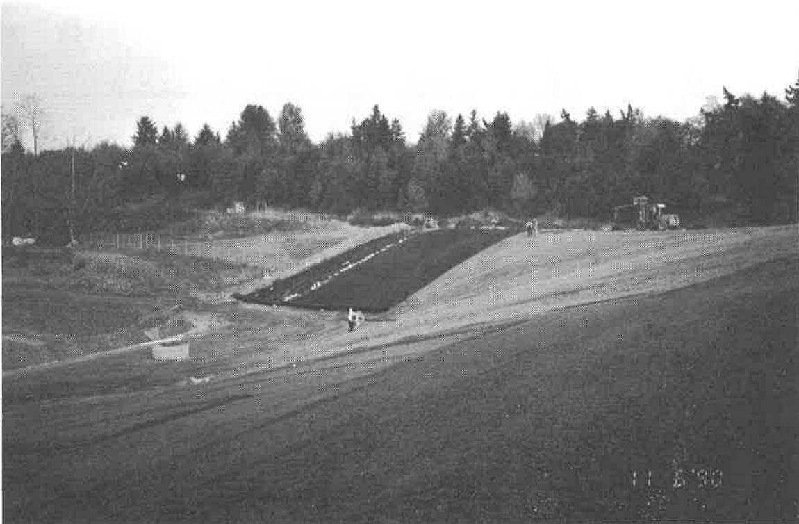
Figure 5. Geomembrane Was Placed First
