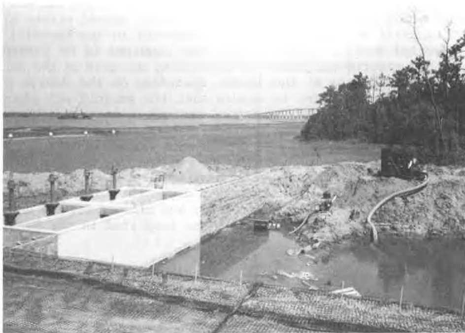
FIGURE 6. The Main Outfall Structure and the Geogrid Reinforced Wing Walls
