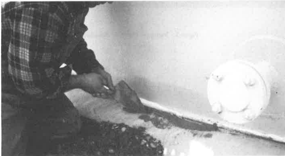
Figure 5. Repair of seal around tank wall
