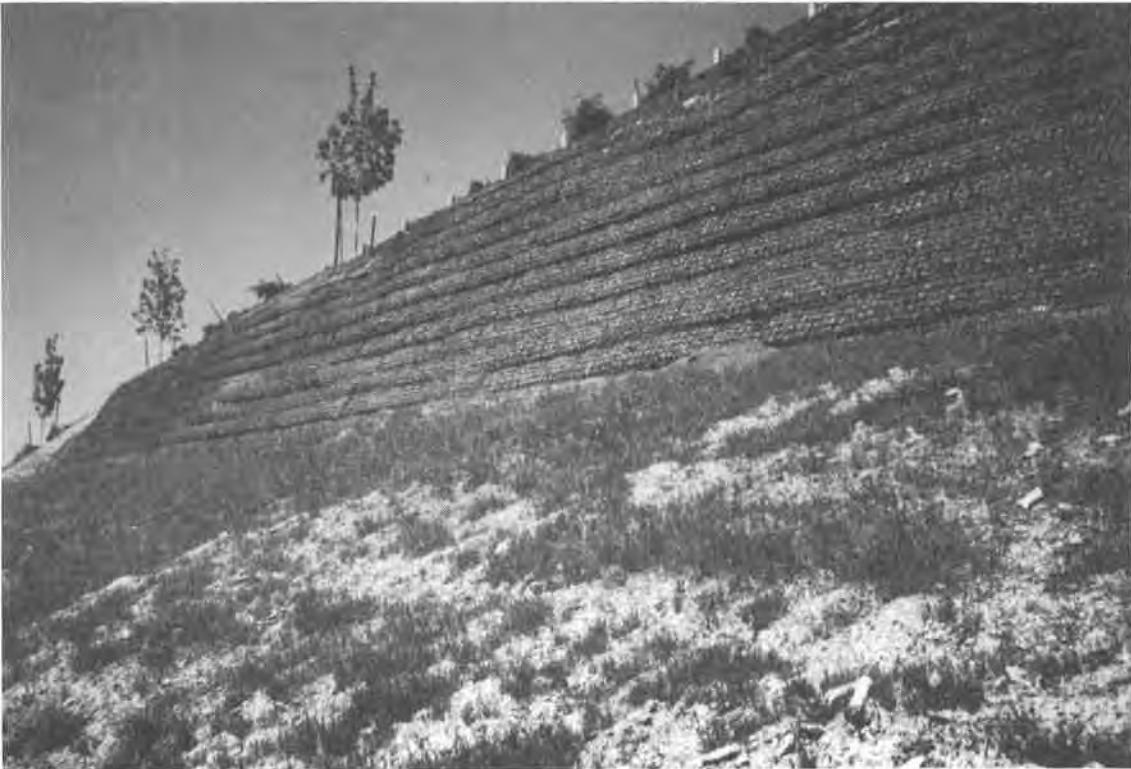
Figure 13. Completed Geogrid Wrapped Rock Faced Slope
