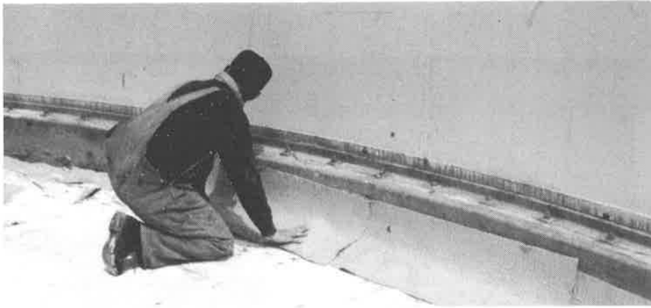
Figure 4. Repair of seal around perimeter wall
