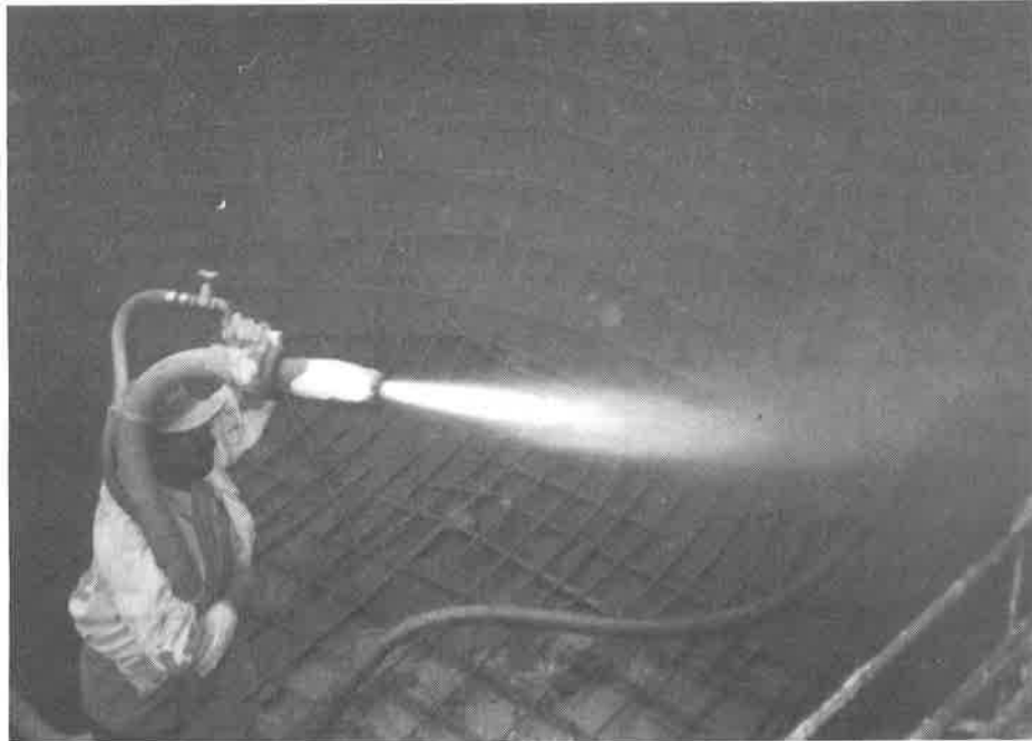
Photo 2: Shotcrete Application Operation
