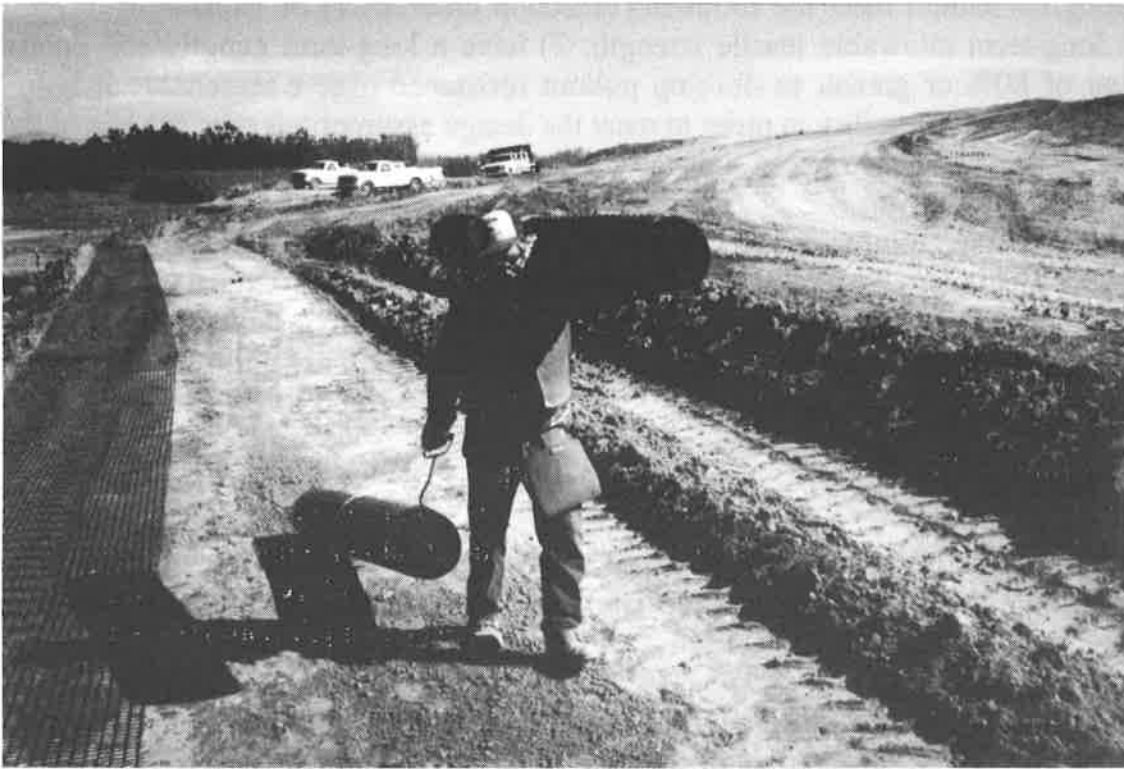
Figure 7. SURFICIAL GEOGRID REINFORCEMENT PLACED AT A SLOPE FACE
