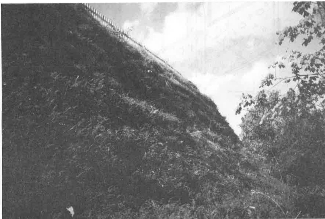
Figure 10. Vegetated Slope Face Eight Months After Construction
