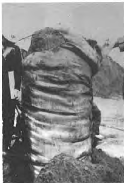
Fig. 3 Fabri-Packed Sand Drain
