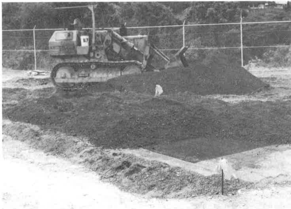
Figure 4. Placement of Slope Drain Material on Installation Damage Test Pad
