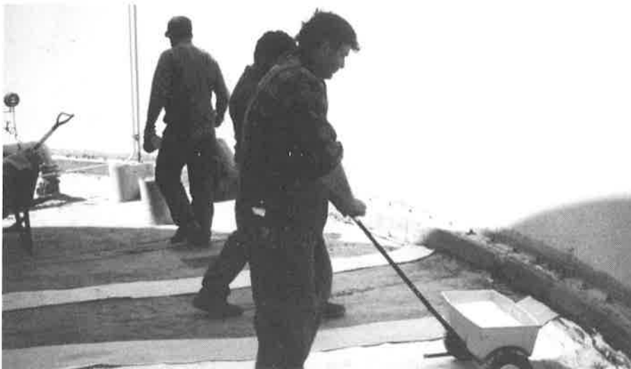
Figure 6. Soda Ash application using standard drop spreader
