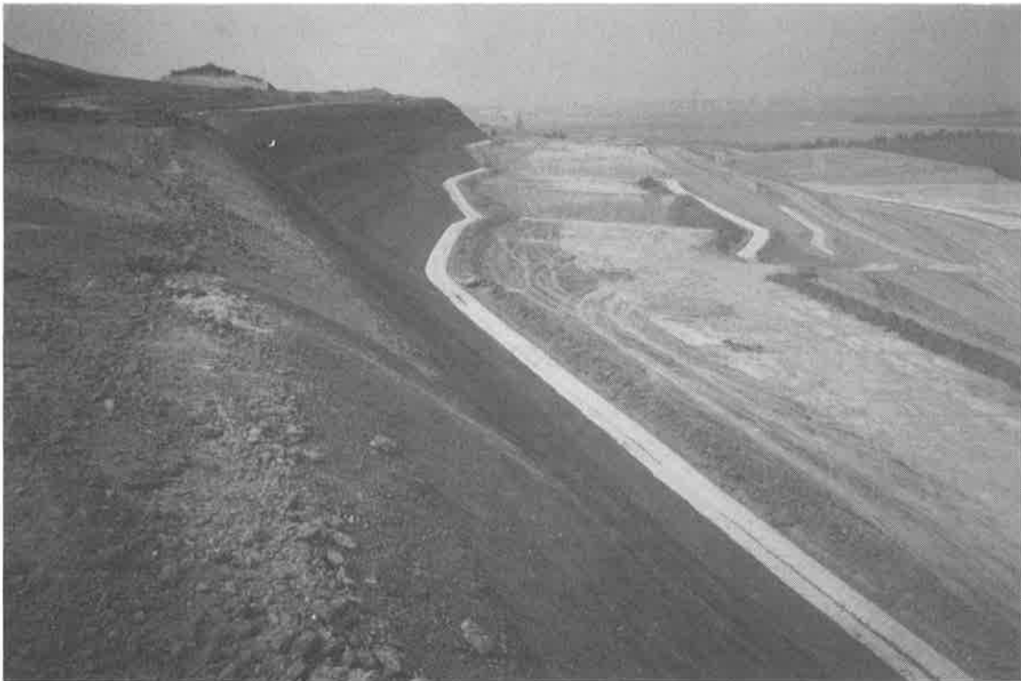
Figure 8. COMPLETED LANDFORM GRADED SLOPE PRIOR TO REVEGETATION
