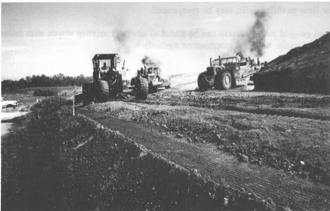
Figure 8. PLACEMENT AND COMPACTION OF FILL OVER SURFICIAL GEOGRIDS
