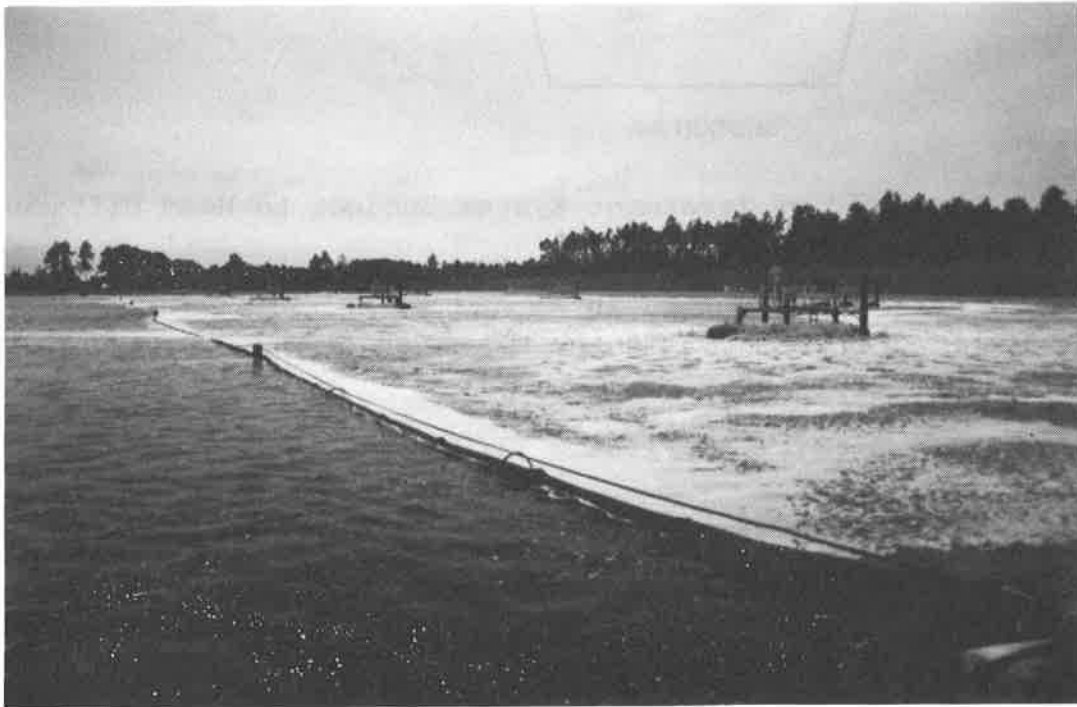
Figure 5. FDB System at Paper Mill Wastewater Treatment System
