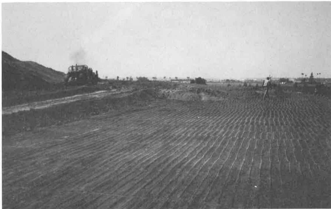
Figure 7. FILL SOIL SPREAD ONTO GEOGRIDS
