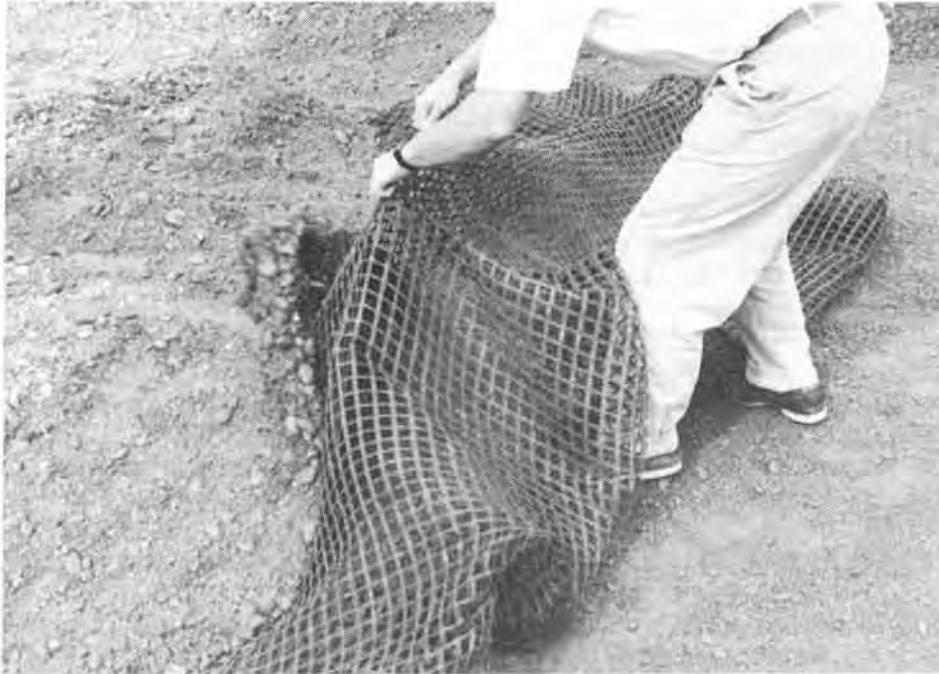
Figure 7. Lifting of Geogrid to Remove Loosened Soil from Partially Excavated Geogrid
