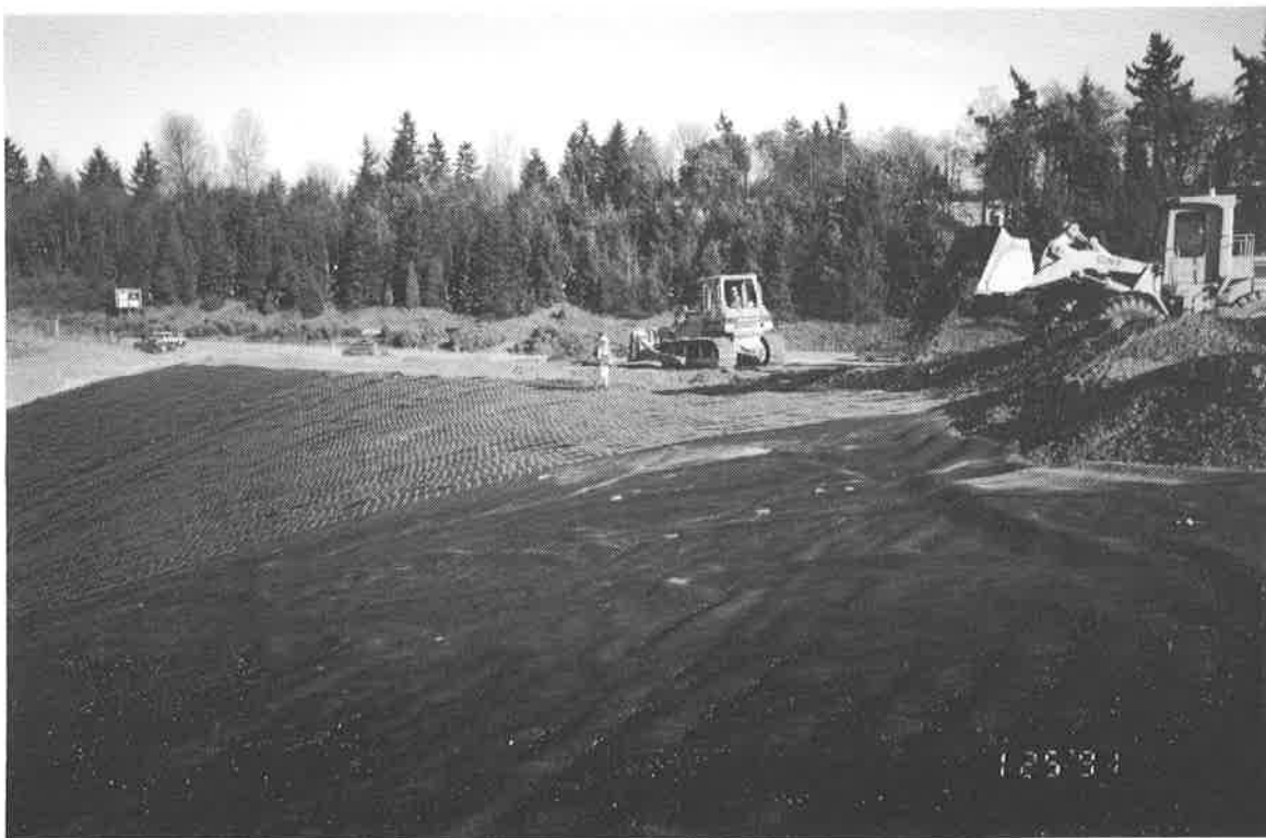
Figure 7. Drainage Sand Being Placed Over Geogrid
