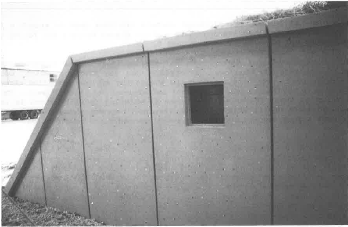
Figure 8 - Completed Polyfelt Lite Wall System
