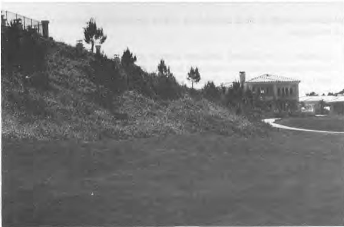
Figure 2. REVEGETATED 21 METER HIGH LANDFORM CONTOUR GRADED SLOPE HAVING A 1H:1V REINFORCED SECTION IN THE UPPER 9 METERS.
