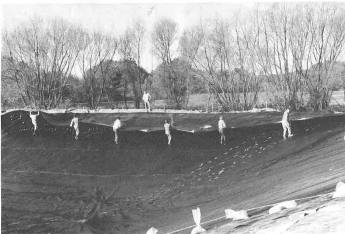
Figure 6. Panel Deployment.
