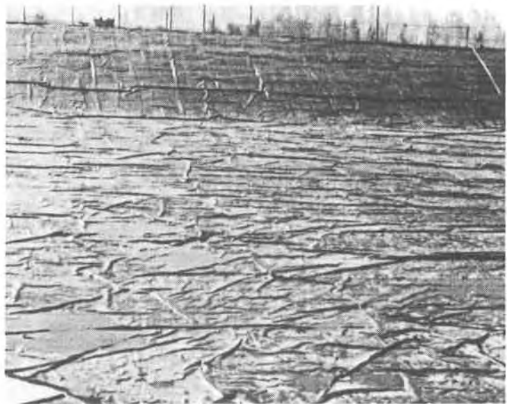
Figure 2. General view of secondary liner; note wrinkles and ponding.
