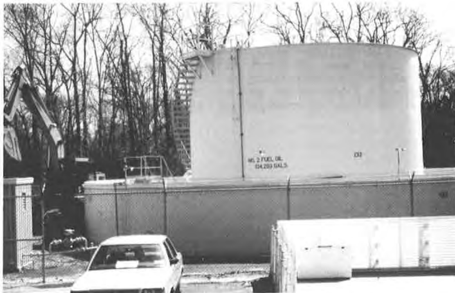
Figure 1. Overview of Site
