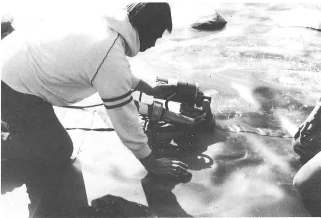
Figure 7. Hot Air Thermal Seaming of Panel Field Seams.
