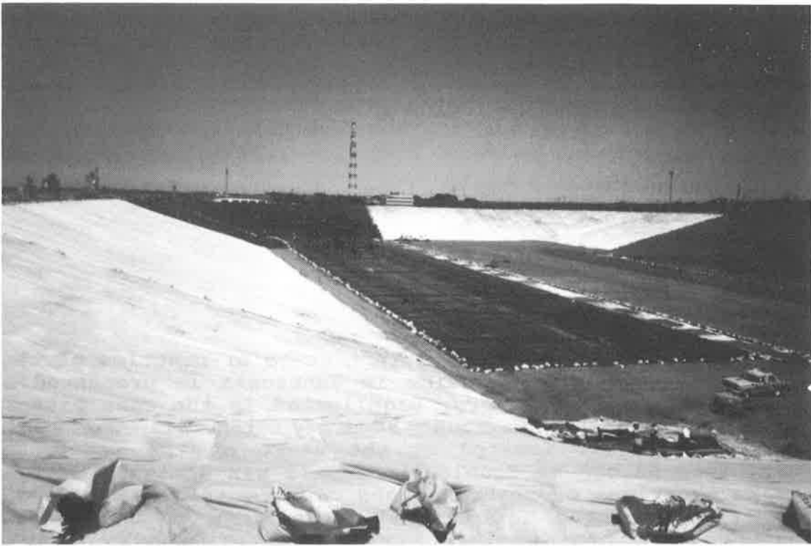
Figure 1. Primary Liner Deployment
