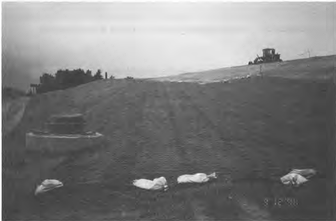
Figure 11. Geogrid Placed on Subgrade
