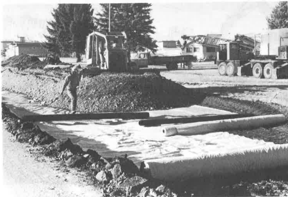
Figure 5. Spreading A-1-b material over geogrid.
