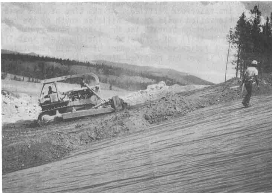
Figure 3. Placement of protective soil material on geomembrane.
