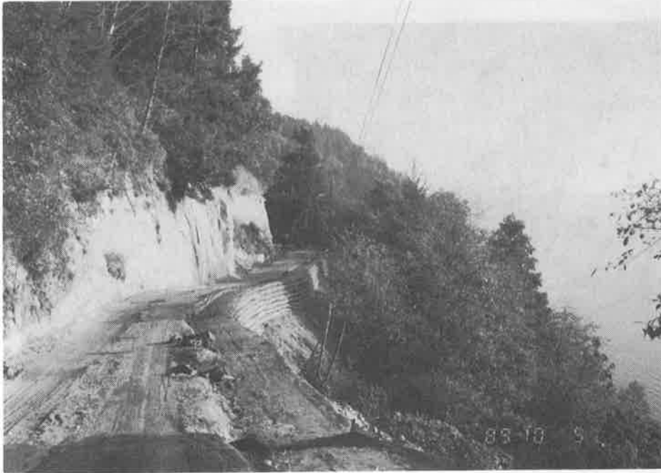
Photo 5. Before paving and shotcreting (October 1989).
