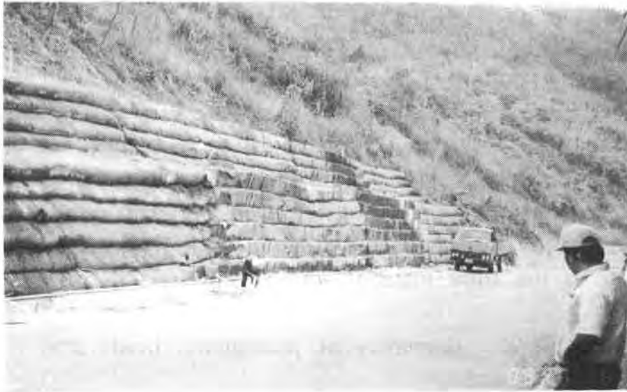
Fig. 9 Finished test wall
