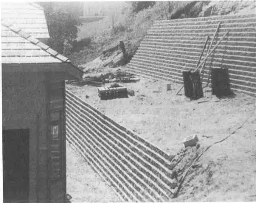
Figure 3 Retaining Wall Under Construction
