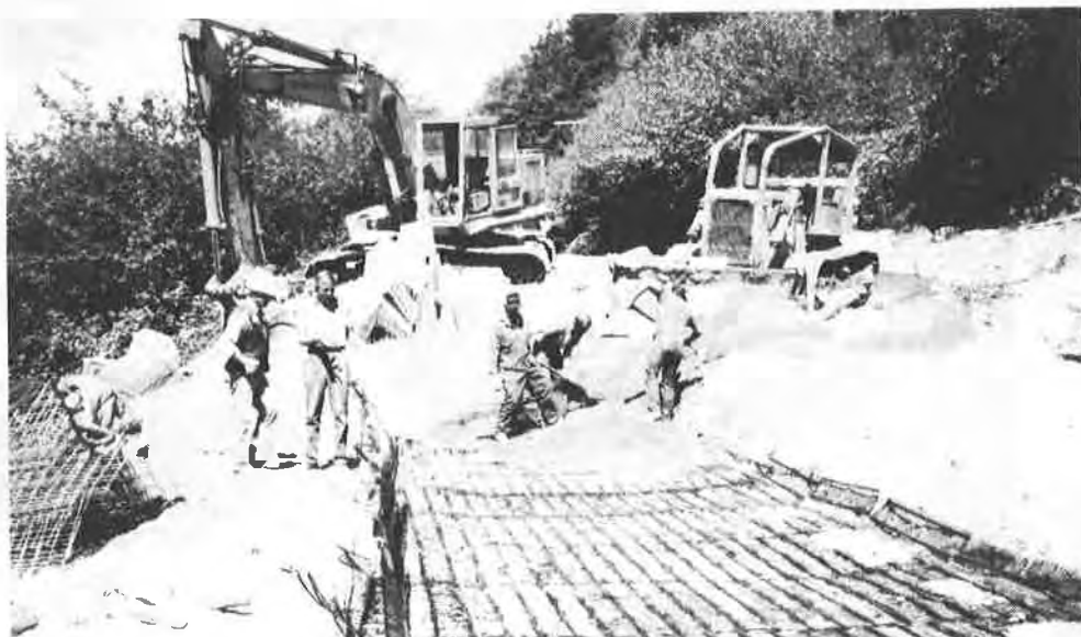
Figure 8. Beginning Wall Construction
