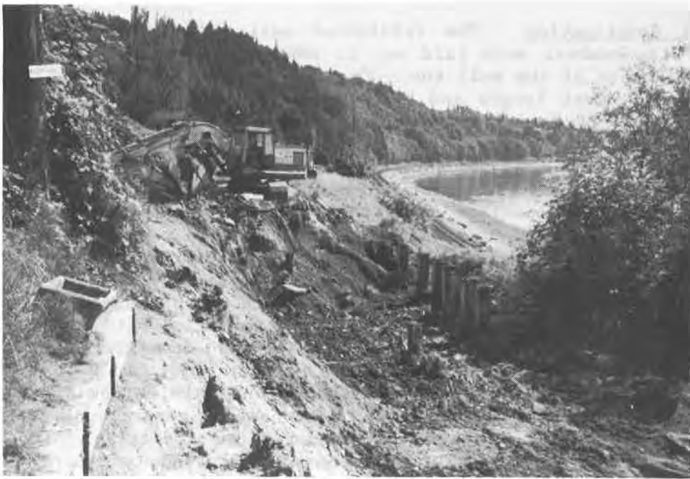
Figure 6. Bridge Demolition and Excavation
