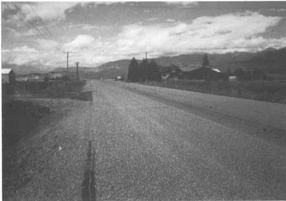
Figure 7. Completed installation. Pavement surface has recently been chip-sealed.
