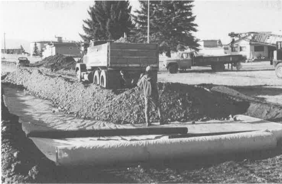
Figure 6. Initial compaction of surface A-1-b material.
