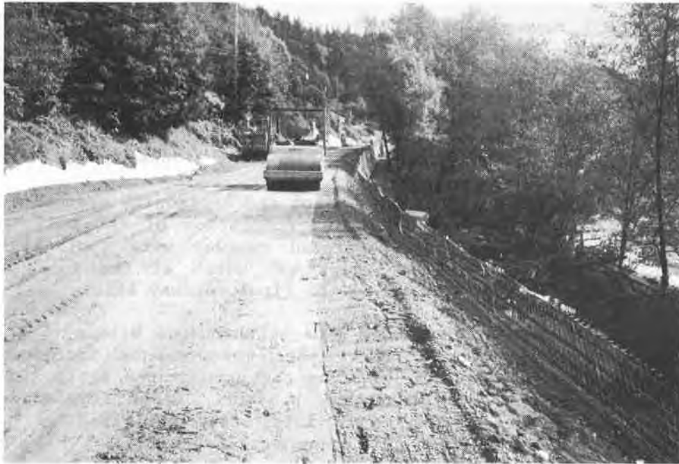
Figure 9. Compaction Was Performed Using a Vibratory Steel Drum Roller
