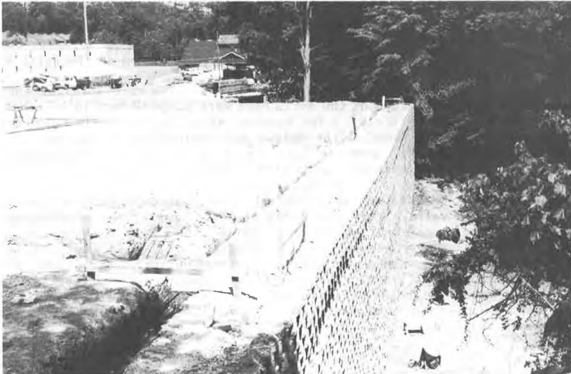
Figure 5 South Wall With Spread Footing in Place
