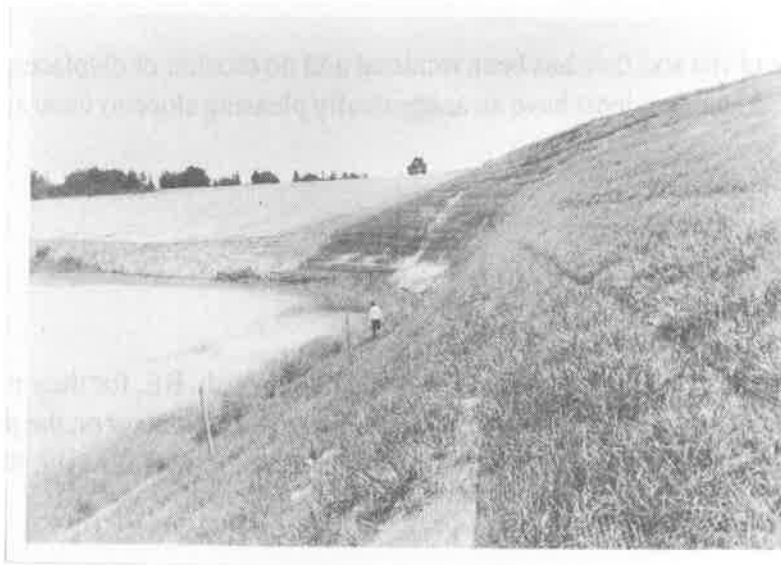
Figure:10 Embankment thirty days after construction
