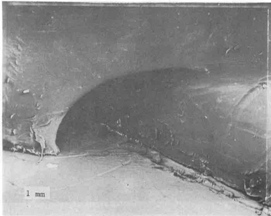
FIGURE 13. SEM IMAGE OF 0.04 INCH DIAMETER LEAK SHOWING BREAK IN FACTORY SEAM WELD
