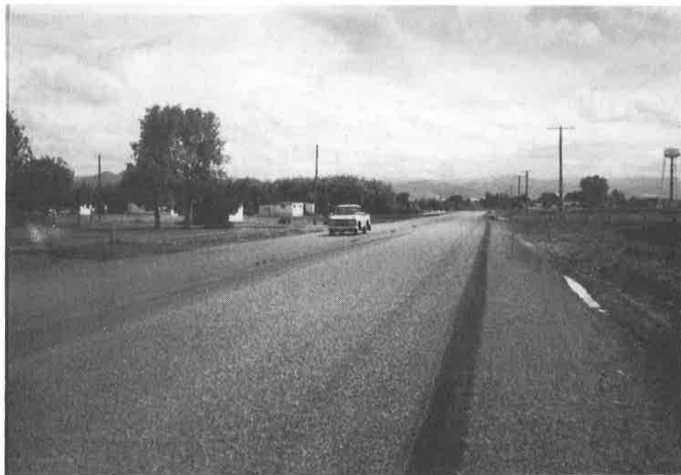
Figures 8 & 9. Completed installation. Note presence of water in side ditches.
