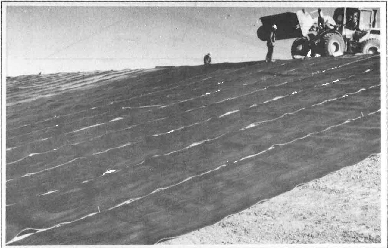
Figure 9 Construction of the Geonet Decant
