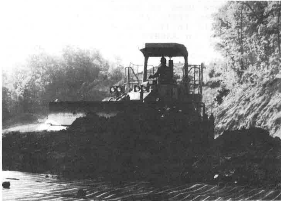
Photo 2: Clay Fill Being Placed over Primary Geogrid Reinforcement
