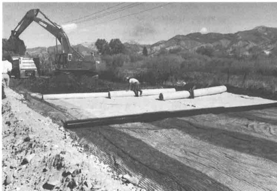
Figure 3. Excavation operations and installation of geotextile and geogrid.
