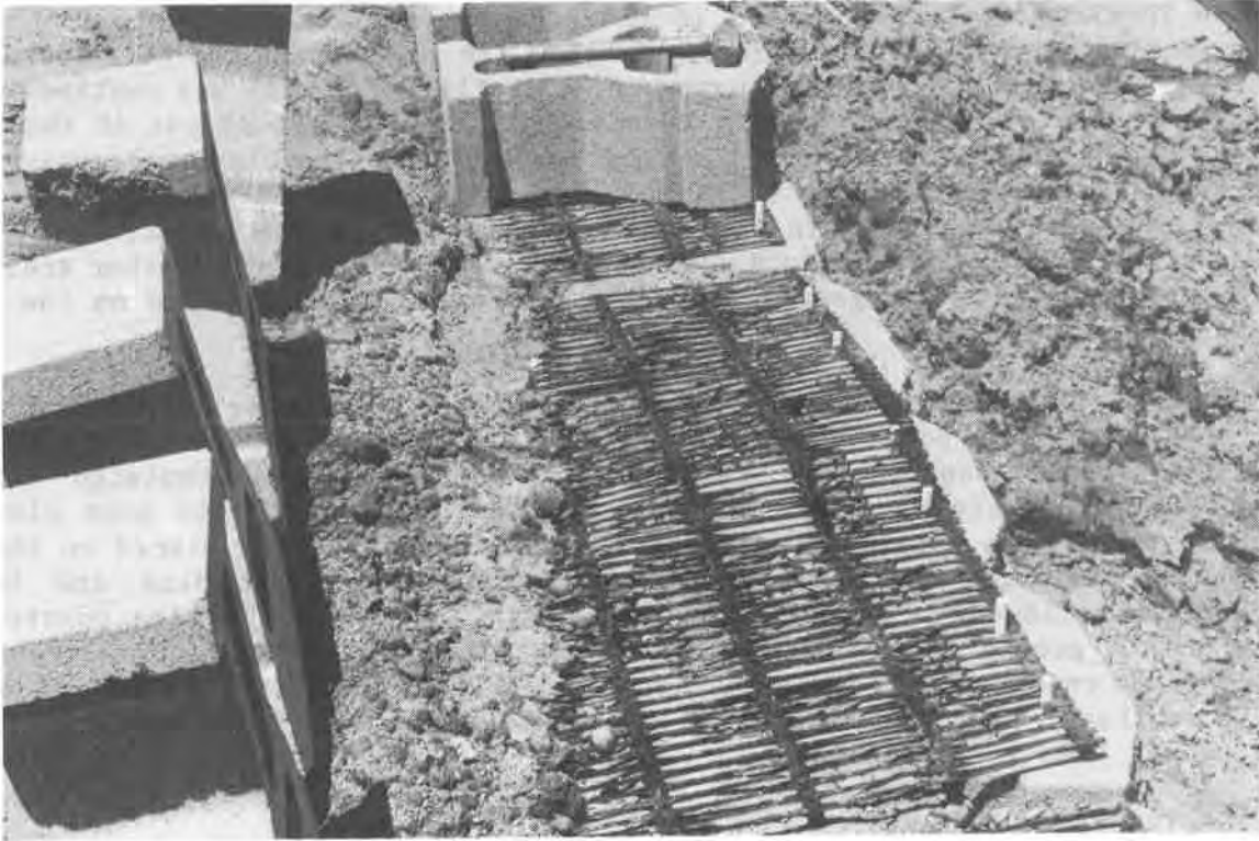
Figure 5 South Wall With Spread Footing in Place
