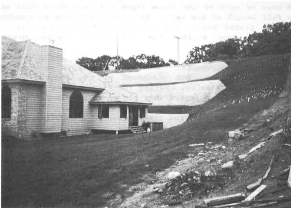
Figure 4 Completed Retaining Wall
