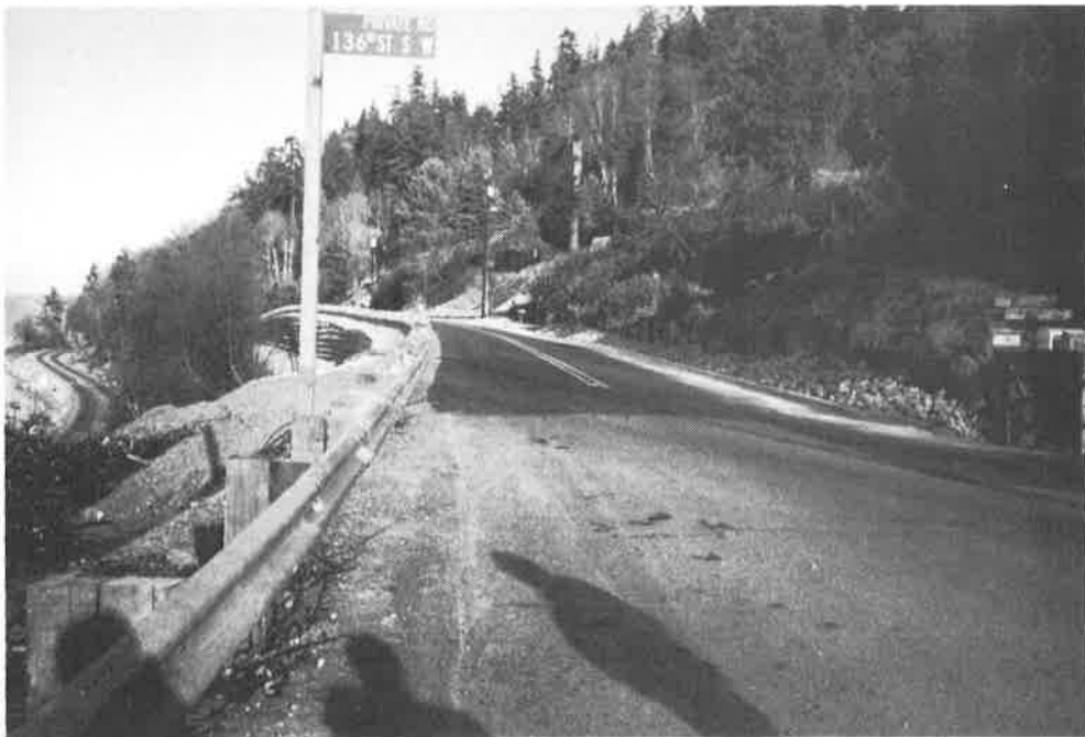
Figure 11. View to the North After Completion of the Project
