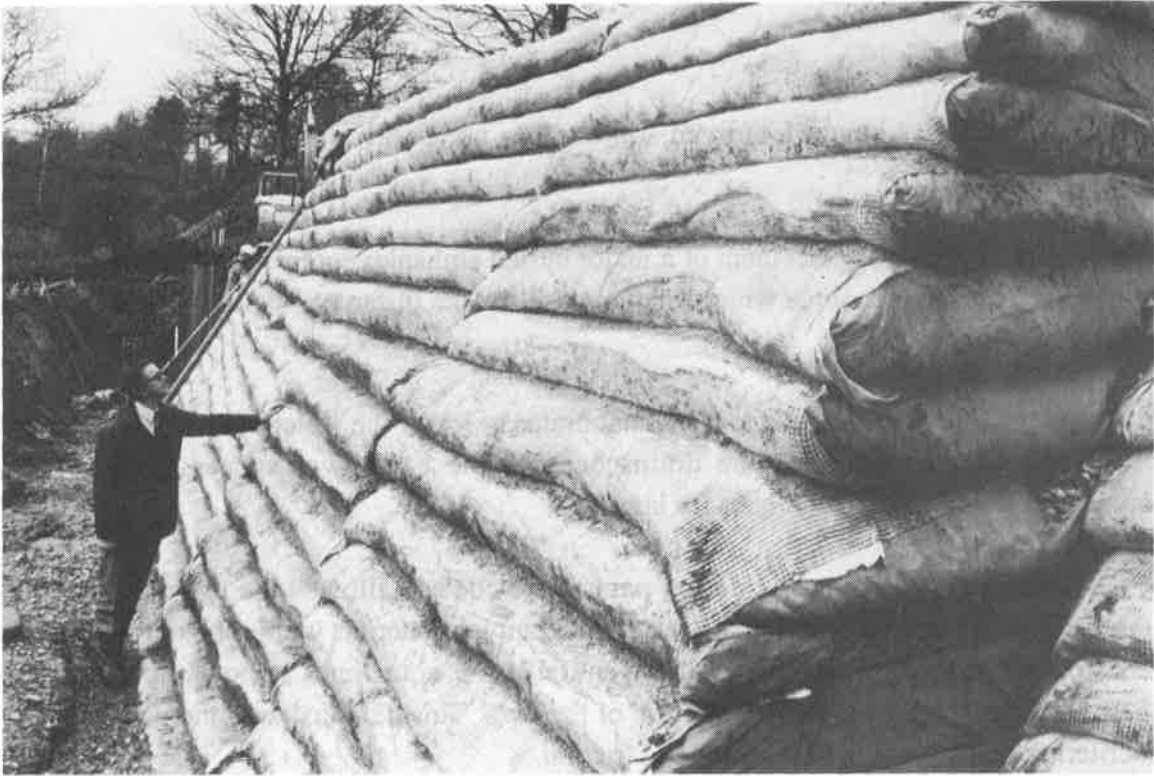
Fig.13. View of Reinforced Soil Bank Being Built in Modular Units.
