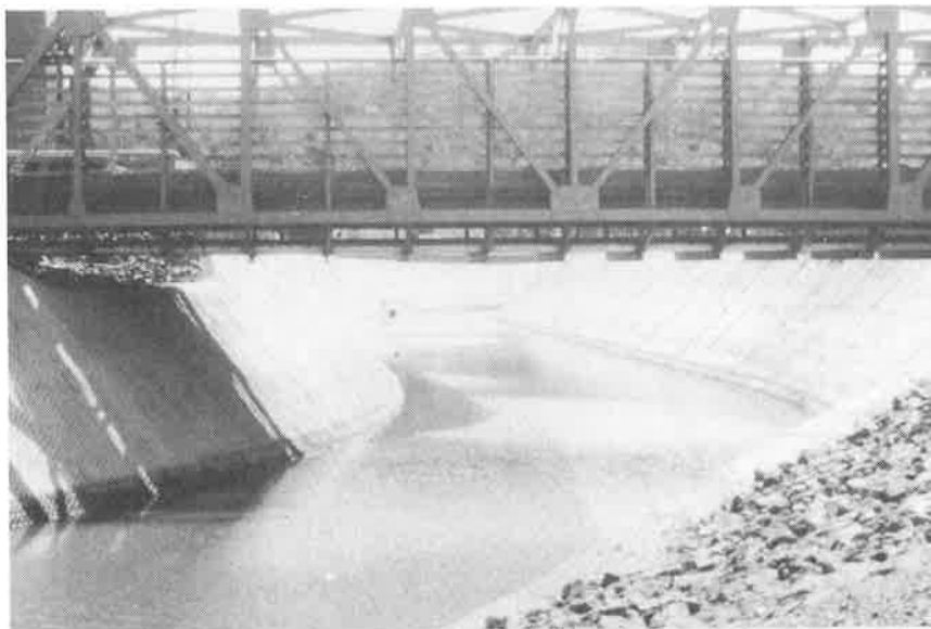
Figure 10: Flow in the diversion channel at the bridge crossing.
