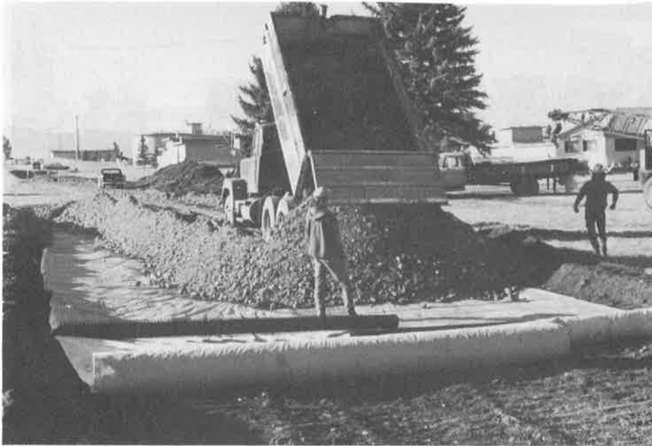
Figure 4. End-dumping A-1-b borrow on geogrid.
