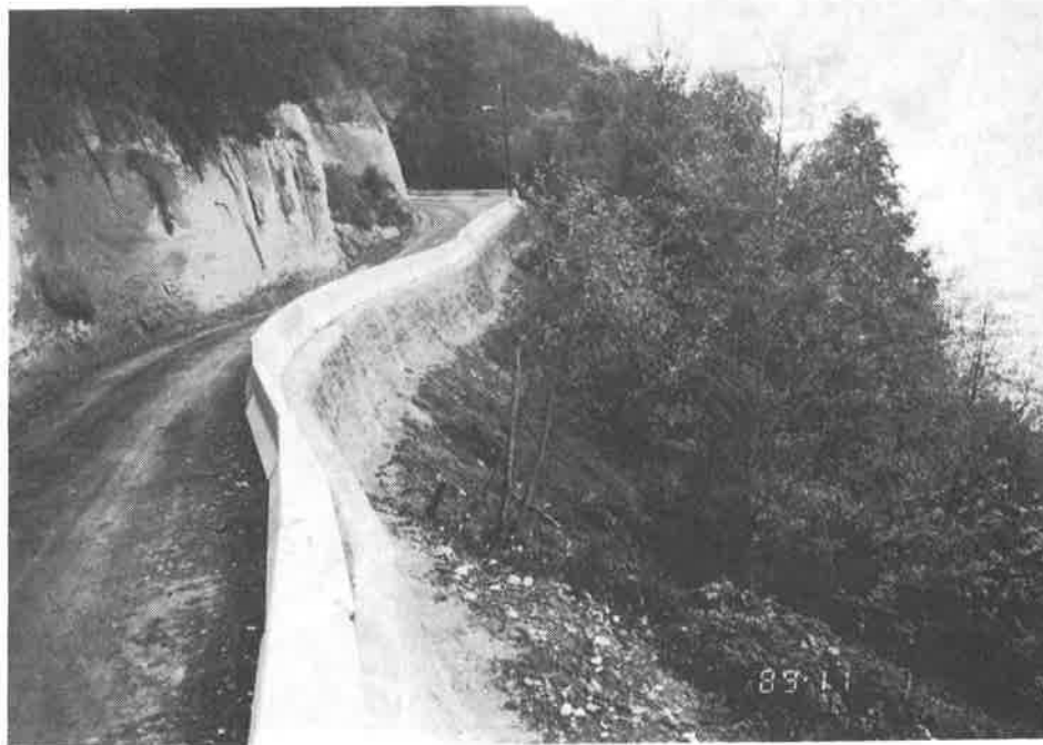
Photo 6. Substantially completed wall (November 1989).
