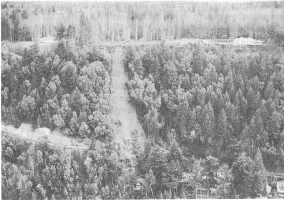
Photo 1. An aerial view of the Sunny Shores Road after a landslide closed the road (March 1989).
