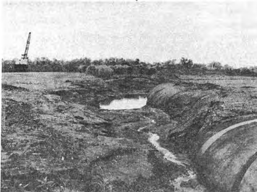
FIGURE 5. VIEW OF THE SITE SHOWING GEOTEXTILE BUBBLE
