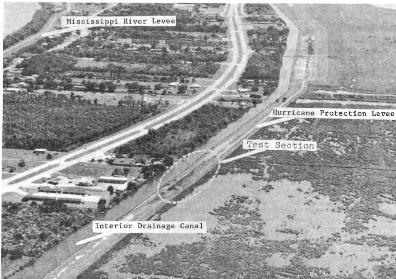
Figure 1. Aerial view of construction site.
