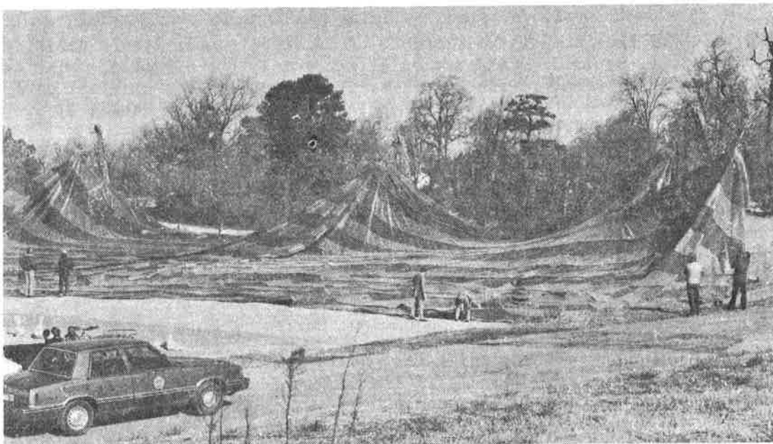
FIGURE 6. FABRICATED GEOTEXTILE PANEL BEING PULLED ACROSS SOFT AREA
