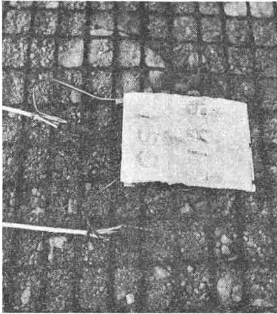
Photo 1: Installation of Strain Gauge for Tensar SS-2 Grids
