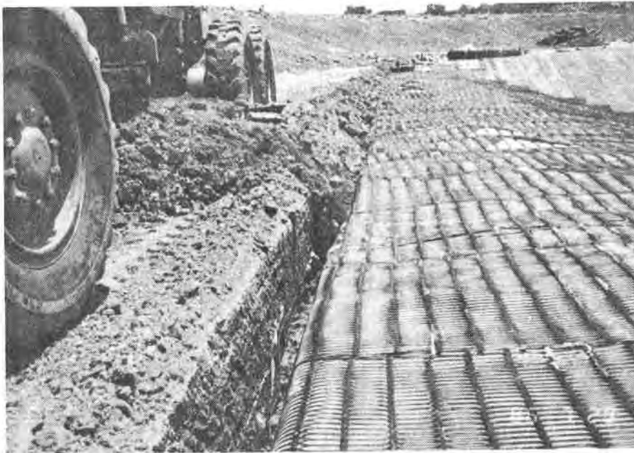
Figure 5. Anchorage of the Geogrid. In this project, the geogrid was placed in the same anchor trench as the lining system.
