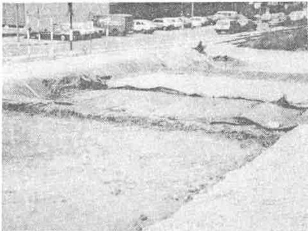
Photo 3: Installation of subsoil material, test fields 1 (front), 2 and 3
