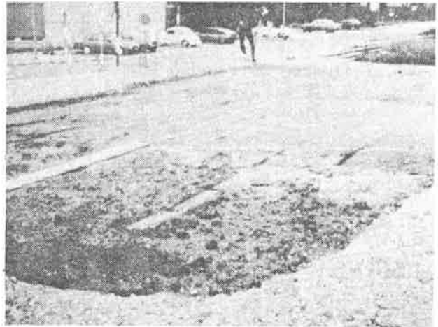
Photo 4: Surface of installed subsoil
