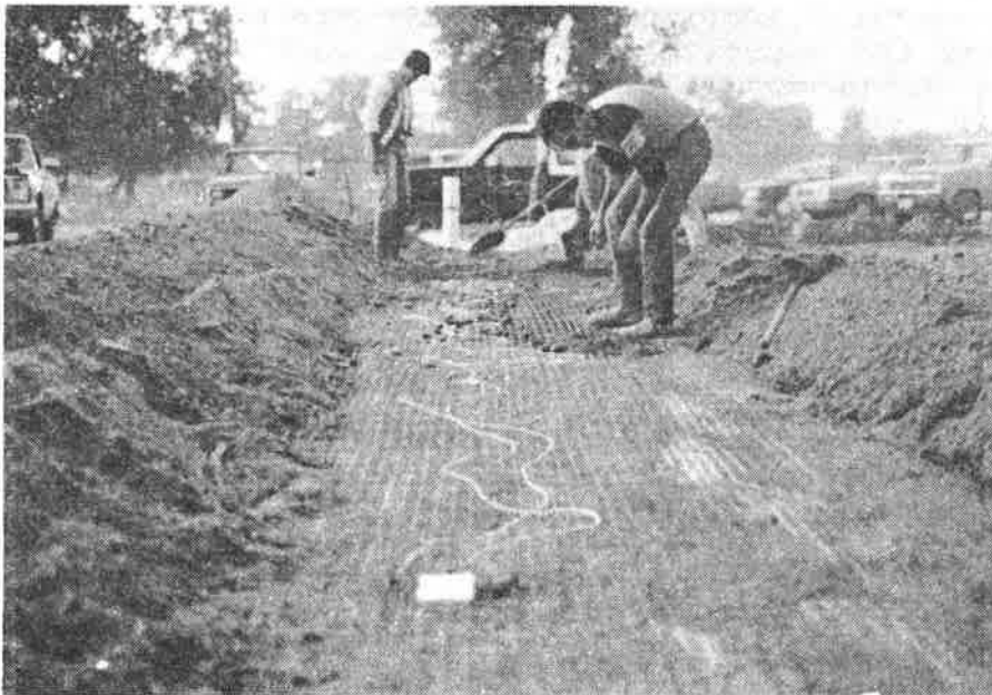
Photo 3 : Alignment of Strain Gauges for Geogrids
