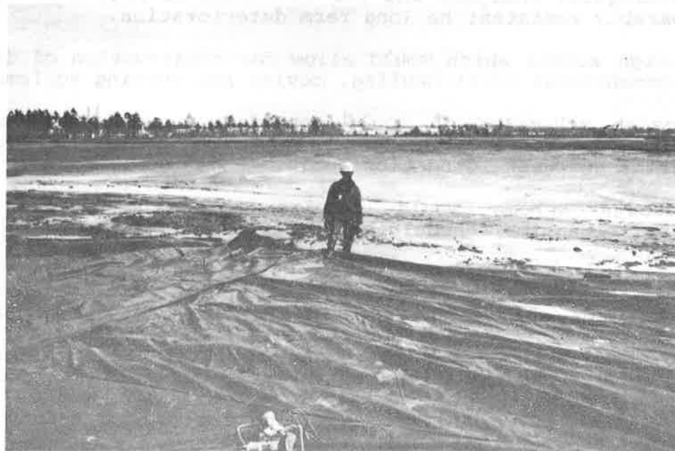
VIEW OF PRE-SEWN GEOTEXTILE LAYER APPLICATION
