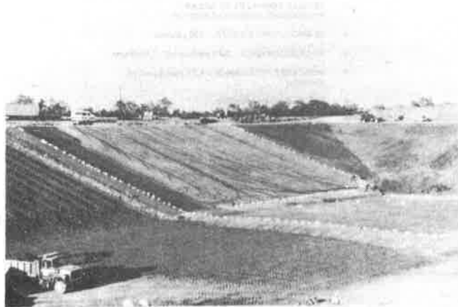
FIGURE 8 - Geomembrane Liner Placement - Slope and Bottom
