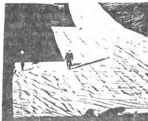
Figure 6. Installation of Geotextile
