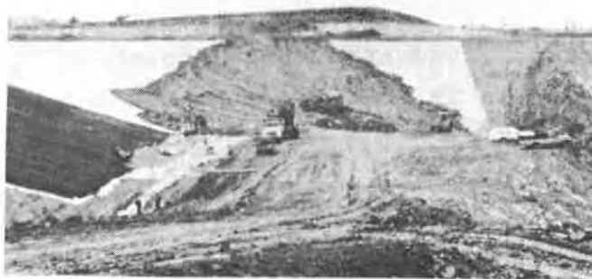
FIGURE 4 - Clay Liner - Initial Placement and Spreading
