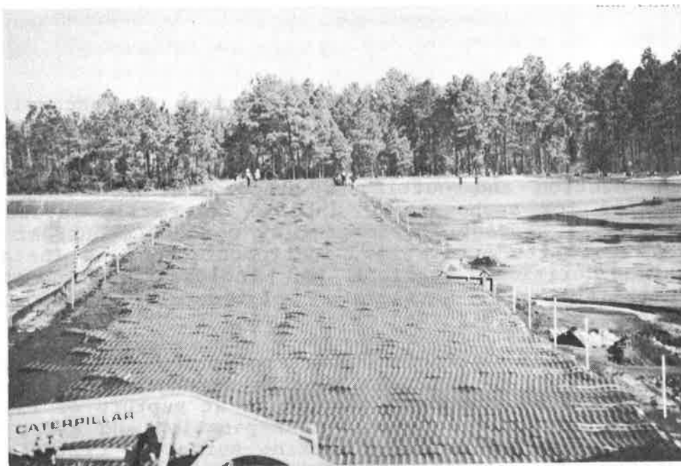
GEOGRID SR2 APPLICATION AT COMMON DIKE (PLACED TRANSVERSE TO DIKE CENTERLINE)
