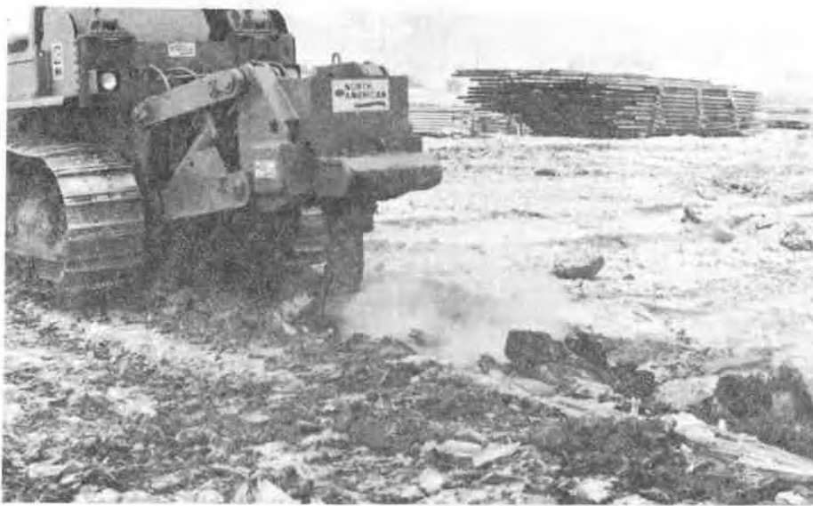
Figure 3: Ripping of frozen subgrade necessitated by the very low freezing temperatures
