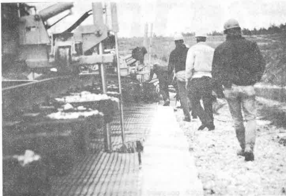
Figure 5 Installing geogrid and geotextile on top of existing subballast.
