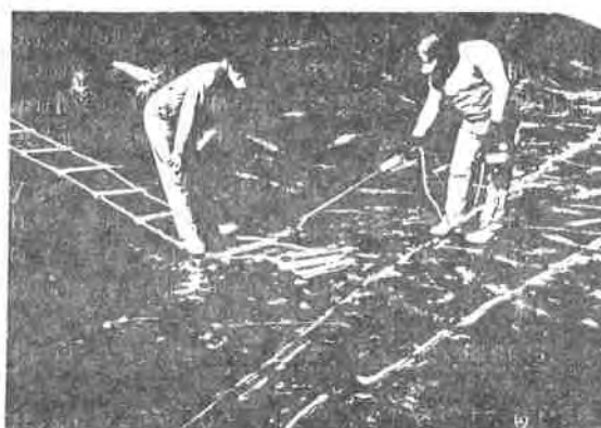
Figure 10. Spark Testing of Seams
