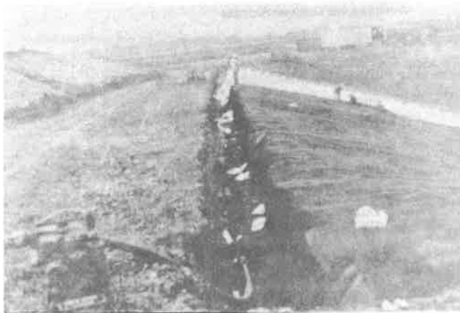
FIGURE 9 - Geomembrane Liner Placment - Anchor Trench
