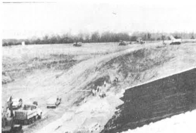
FIGURE 3 - Pressure Relief System - Installation of Gravel Collection Laterals
