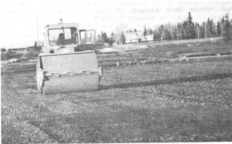
Figure 4: Finished surface prepared prior to the cold weather work
