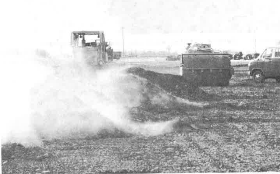
Figure 5: Gravel placement during -40 degree C. weather
