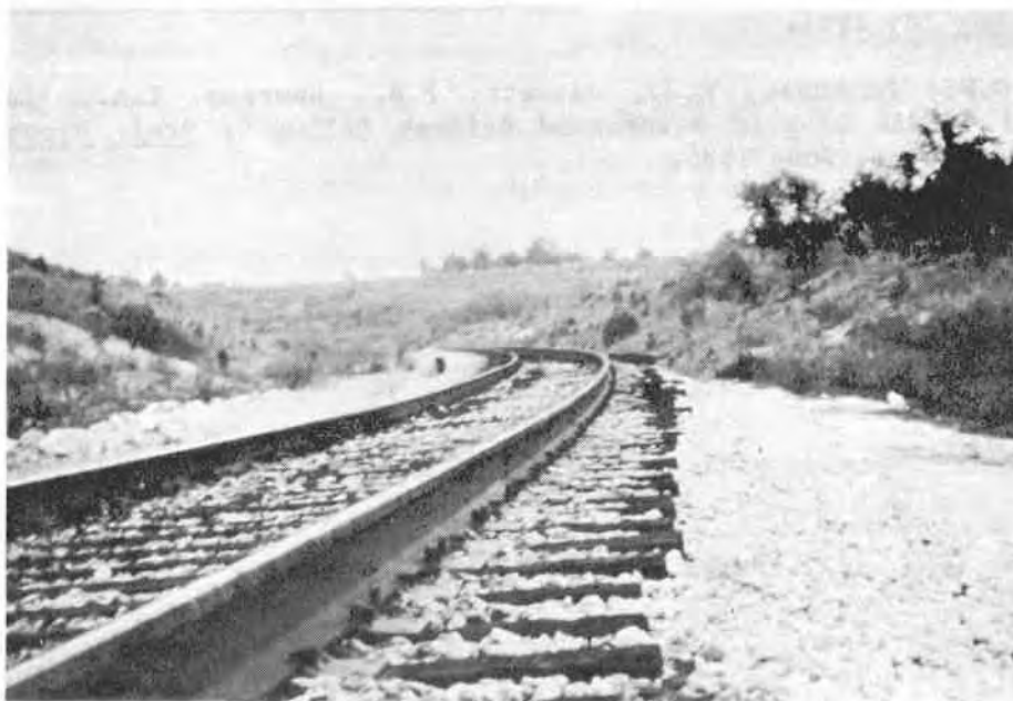
Figure 7 Track structure after construction.
