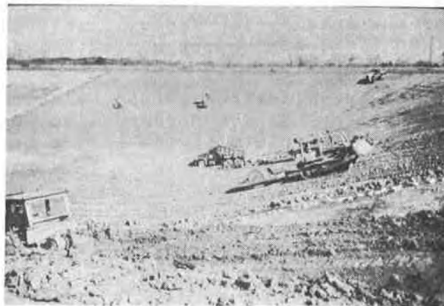
FIGURE 5 - Clay Liner - Placement, Compaction, Fine Grading, and Testing
