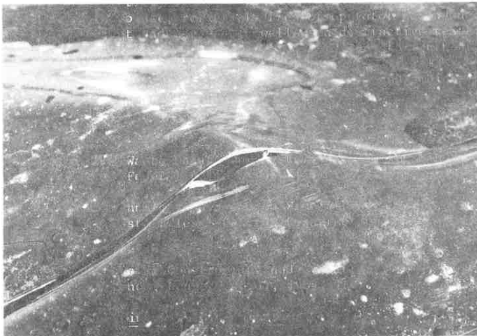
Figure 1 Brittle fracture adjacent to an extruded lap seam prepared in the plant
