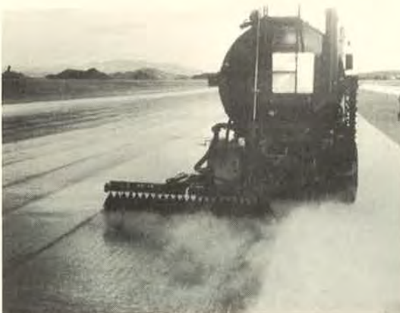
Figure 8. Applying a bottom.
