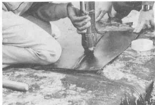
Fig. 2 Startup Seam Test Weld
