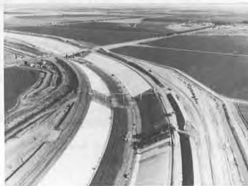
Figure 5 - Full Section Canal Construction Machinery Courtesy - R.A. Hanson Co., Inc.
