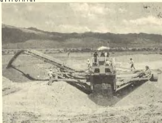
Figure 1 California Aqueduct Under Construction
