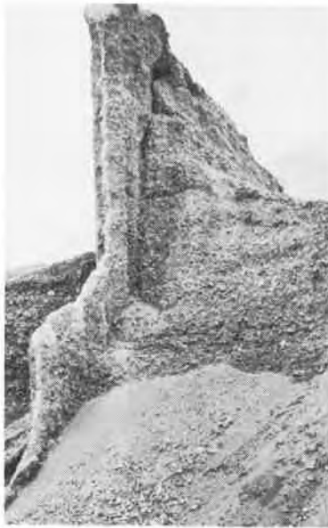
Fig.7: Excavated diaphragm wall from test driving
