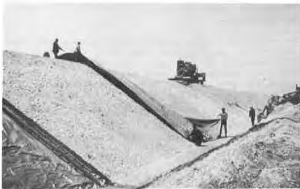
Fig.3: Placing of foils on the slope
