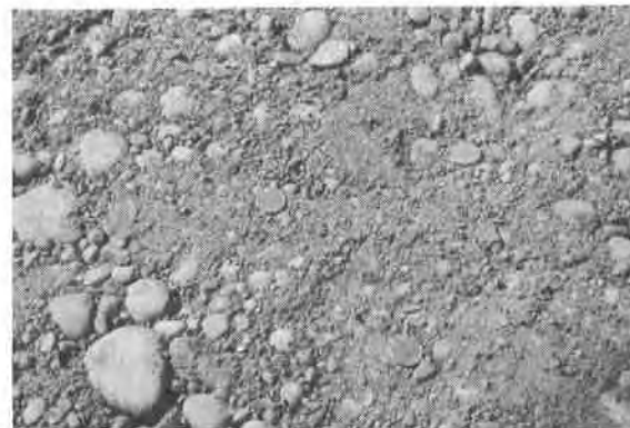
Fig.4. Photograph of test area subgrade surface.
