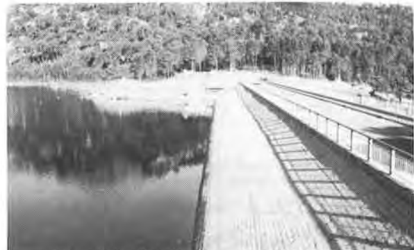
Fig. 3 Ospedale dam. View of upstream slope.
