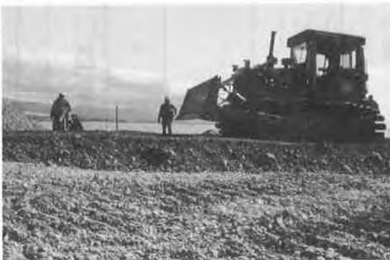
Fig.7. Fill being placed over test area by D-6.
