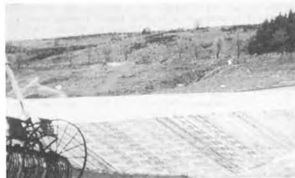
Fig. 8 Mas d'Armand dam - General view.
