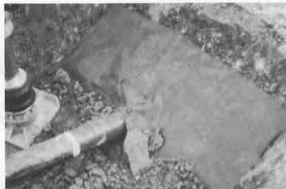
FIGURE 4: ANTI-SEEP COLLAR CONSTRUCTION
