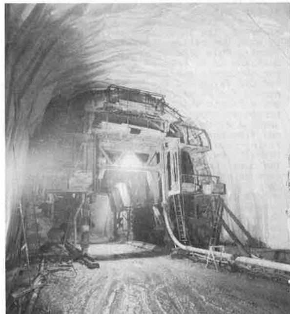
Fig. 4: Section of a tunnel after fastening of the plastic sheeting
