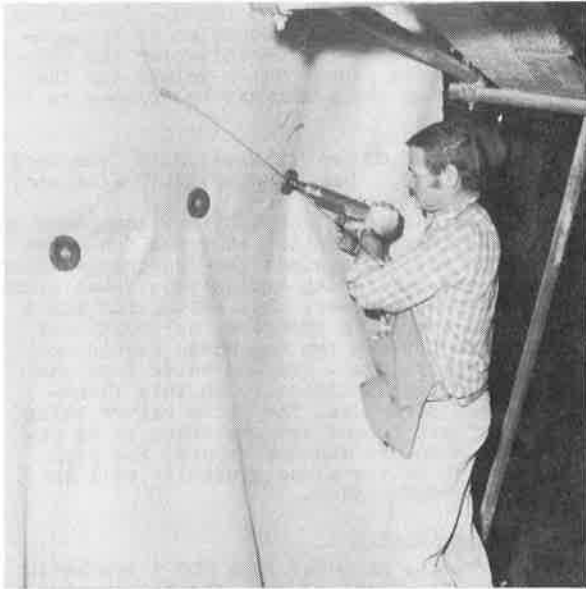
Fig. 1: Fastening the non-woven protective layer to the tunnel wall
