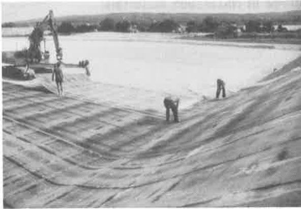
Photograph n° 1 .Placing of Geomembrane. (West Germany)
