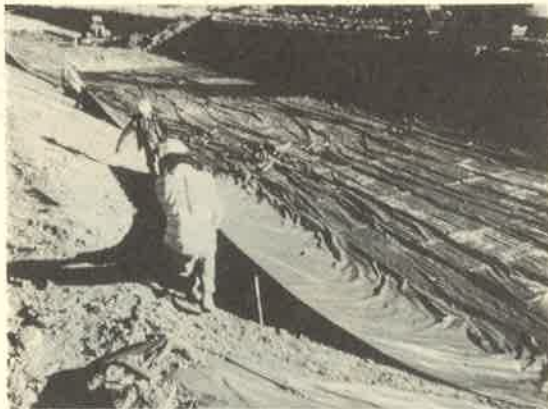
Figure 8 Courtesy of U.S. Bureau of Reclamation
