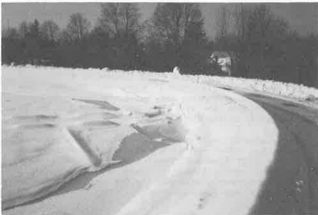
Fig. 2 - Hypalon Floating Cover at 20 MG Reservoir March, 1983
