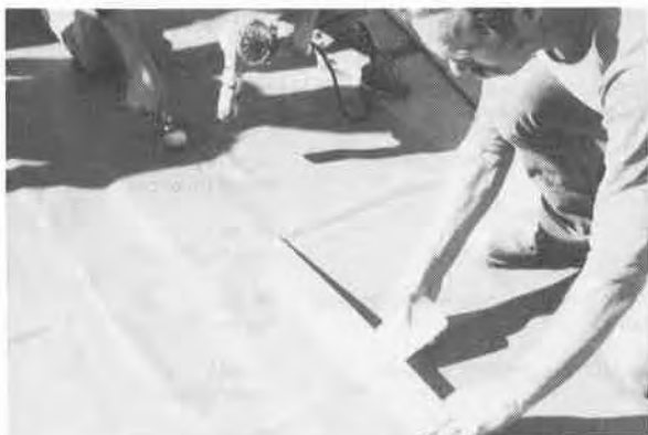
Figure 1. Fabrication of a typical seam section
