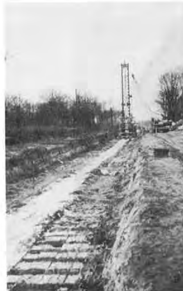
Fig.5: Manufacturing of a diaphragm wall for building pit-dam
