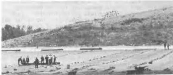
FIGURE 5: HDPE LINER PLACEMENT
