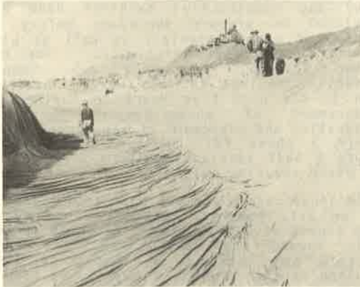
Figure 7 Courtesy of U.S. Bureau of Reclamation
