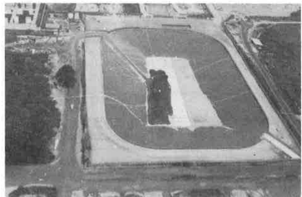
Fig. 9 - A general view of the second basin
