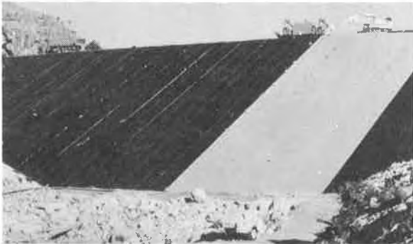
Fig.4 Ospedale dam. Laying the upstream facing.
