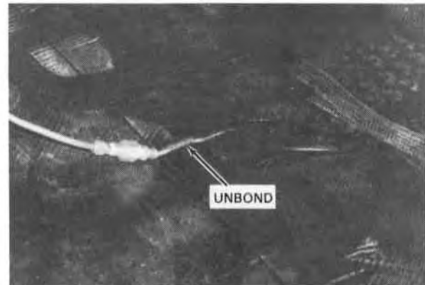
Fig. 1. Air lance detecting an unbond in a chlorosulfonated polyethylene seam.
