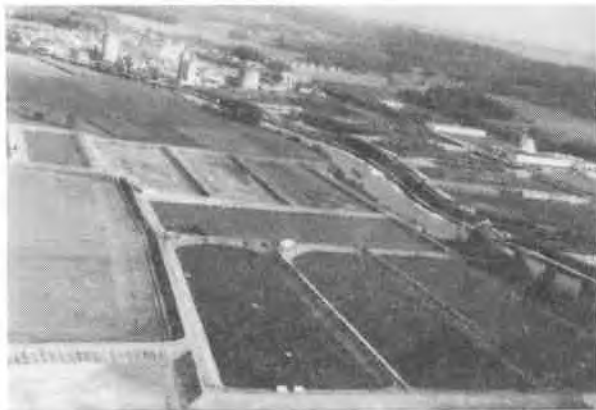
Photograph n° 6 : Aerated lagooning in Vic-sur-Aisne (France)
