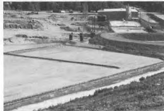
FIGURE 8: FINAL LEACHATE COLLECTION DRAINS AND COVER
