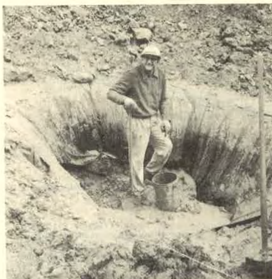
Figure 7. THE GEOMEMBRANE STRETCHED BEFORE RUPTURING IN ONE OF THE 1962 SINKHOLES
