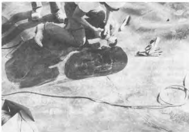
Fig. 8 Grinding a Patch Weld for Rewelding
