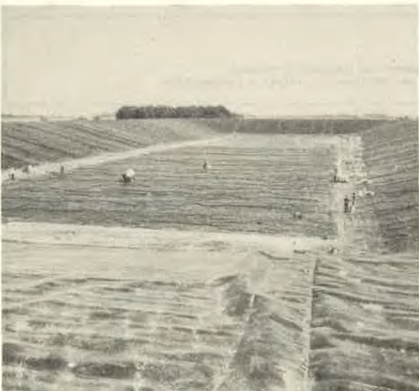
Figure 6: In-place high density polyethylene (HDPE) liner.
