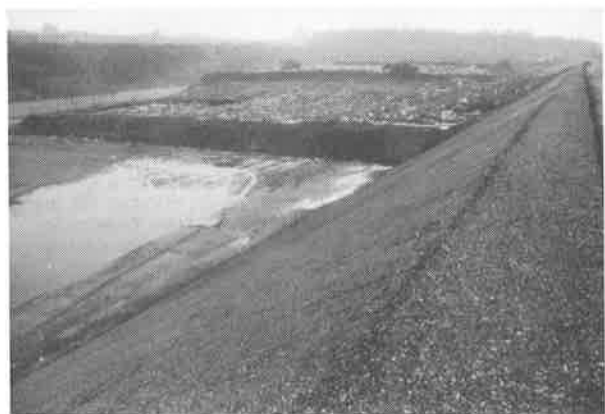
Photograph n° 3 : Landfill operation phase one and gravel emulsion protection on the slope
