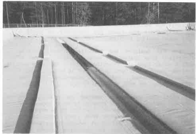
Fig. 3 - Photo of typical rainwater collection channel at 4 MG reservoir October, 1982
