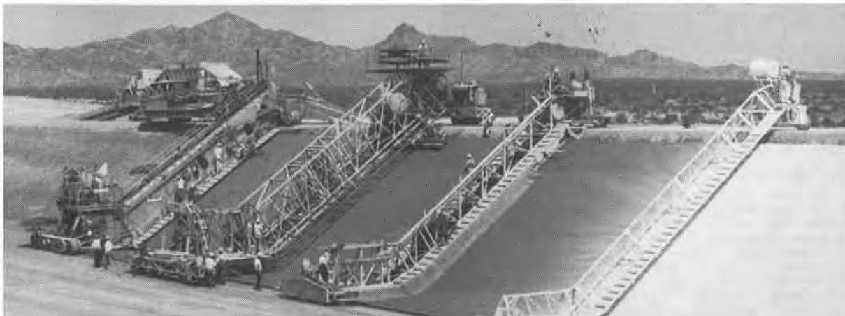
Figure 6 - Half Section Canal Construction Machinery Courtesy - R.A. Hanson Co., Inc.
