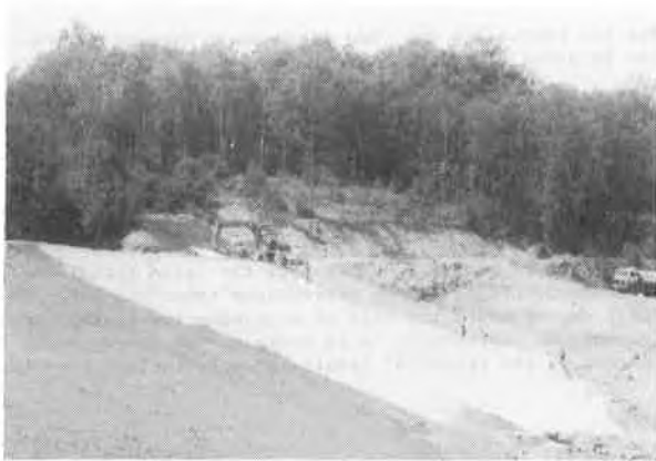
Fig.7 Lanouaille dam - Laying the membrane.
