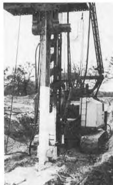
Fig.6: Driving plant pulling the H-pile
