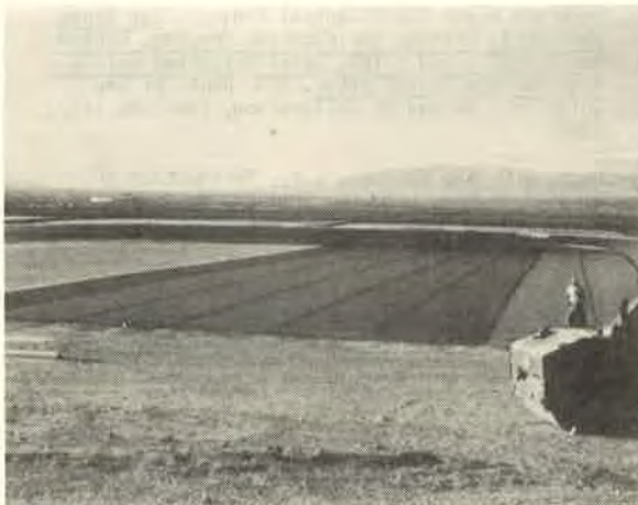
Figure 7. Partially complete bottom.
