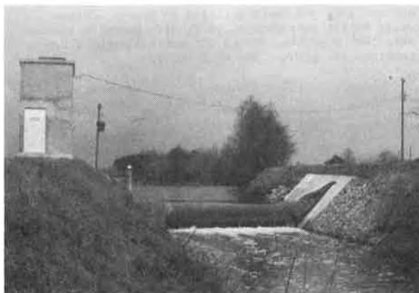
Figure 1. The Water Inflatable Fabric Dam on Mitchell Creek near Tarboro, North Carolina, U.S.A.
