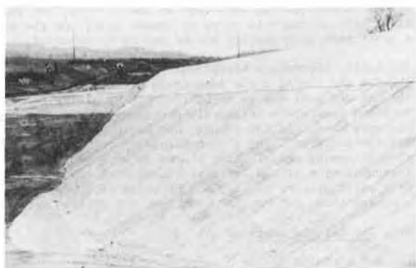
Fig. 9. Mas d'Armand dam - Upstream slope facing.
