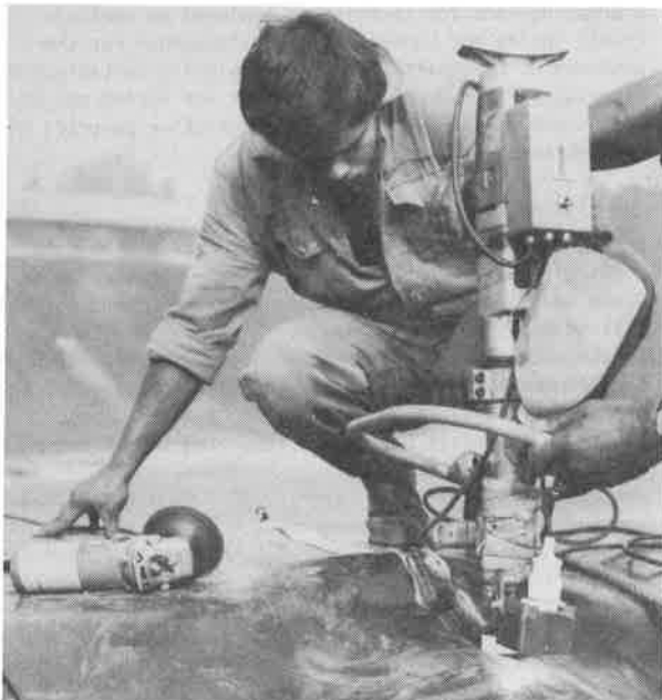
Fig. 6 - The geomembrane welding in the first basin (by extrusion system)
