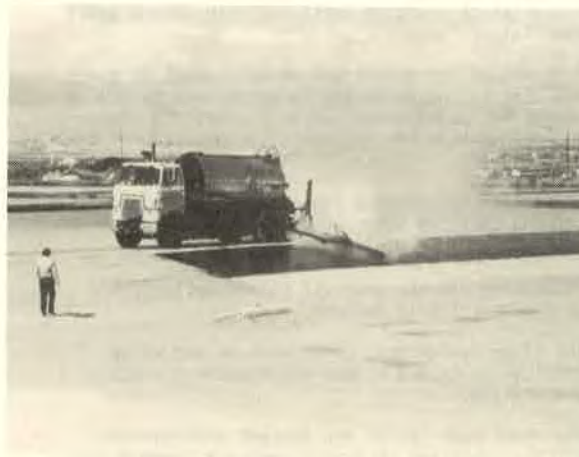
Figure 6. Applying second coat to a slope.
