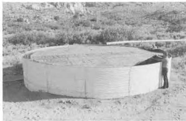
Fig. 3. Floating cover on water storage tank near Safford, Arizona. The inflow pipe conveys water from a water harvesting catchment. The tank is notched (upper left side) to provide an overflow. This floating cover was constructed and installed in 1974.
