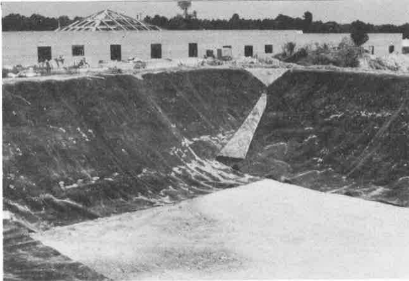
FIGURE 3 - A salt gradient solar pond at Louisiana Tech University was lined with a 2.5 mm high density polyethylene geomembrane. The pond is 75' x 75', 1:1 side slope, 12' vertical depth. Capacity of the pond is 350,000 gallons of brine.
