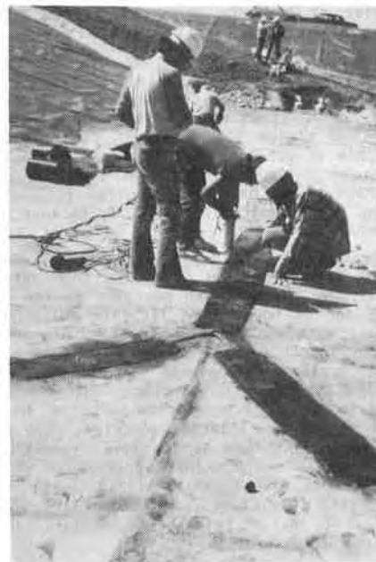
Fig. 3 Cap Strips Being Applied to a Wrinkle Removal Seam
