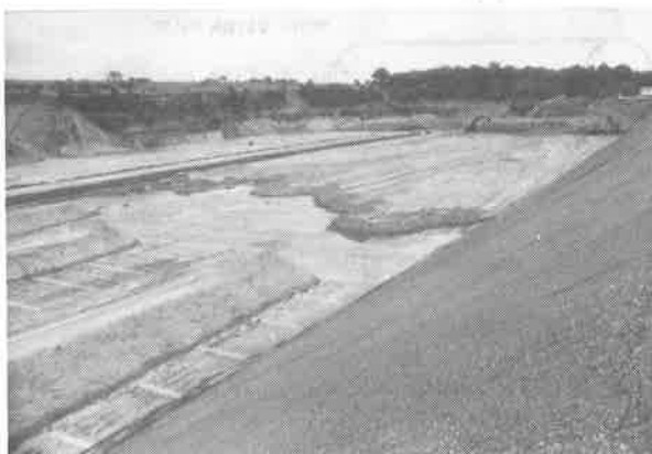
Photograph n° 2 : Protecting sand layer on Geomembrane - Fosse Marmitaine Landfill (France)
