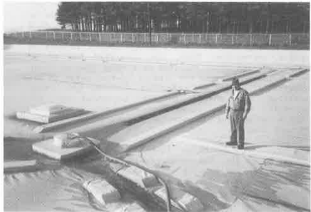
Fig. 4 - Photo of 4 MG reservoir cover and dewatering system October, 1982
