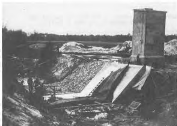
Figure 5. Reverse filter downstream of the Fabridam.
