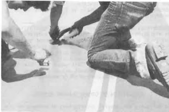
Fig. 1. - Making a solvent seam on PVC.
