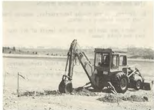
a. Removal of earth cover.
