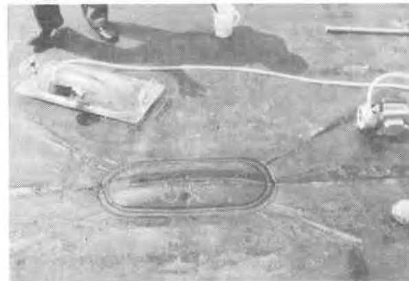
Photograph n° 5 : Vacuum Test Saint Augustin Landfill (West Germany)
