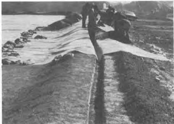
FIGURE 6: ANCHORAGE OF HDPE INTO PERIMETER BERM
