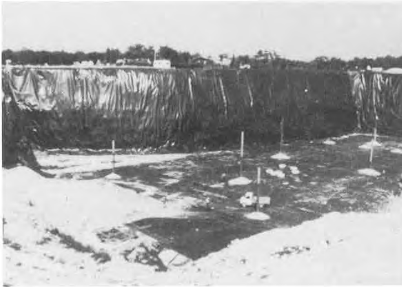
FIGURE 4 - The Osio Sotto landfill was lined with 35,000m 2 of HDPE geomembrane.
