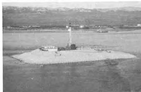
Fig.1. View of constructed artificial drilling island
