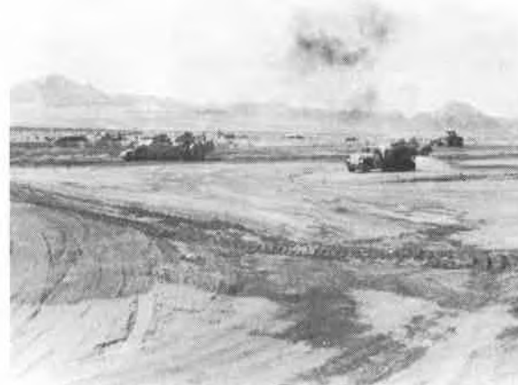
Figure 3. Earthmoving for a crystal harvesting pond.
