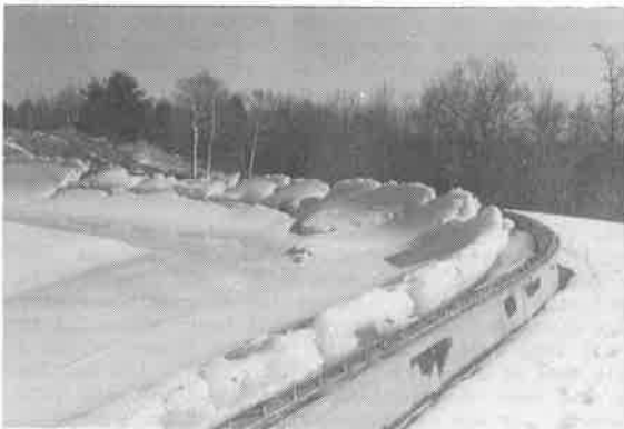
Fig. 1. - EPDM Floating Cover at 20 MG Reservoir March, 1978
