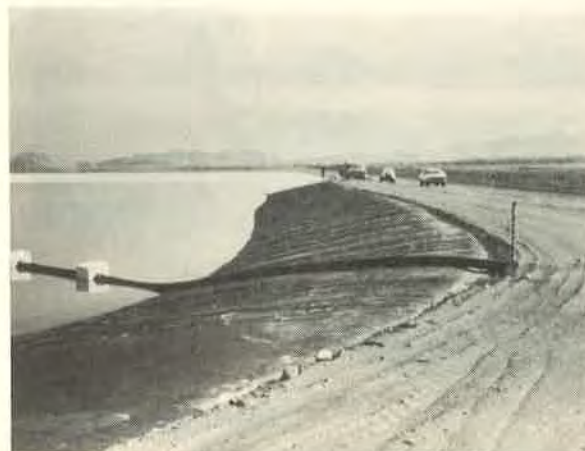
Figure 9. Applying U.V. protective coating.
