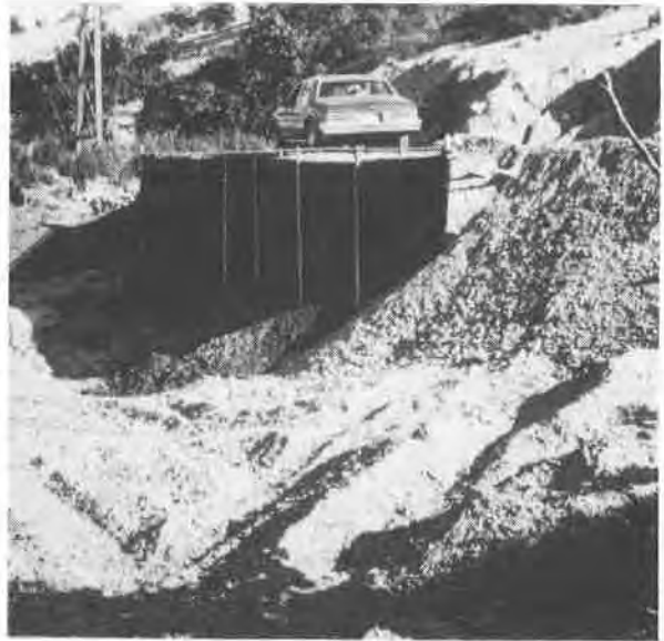
PHOTO 3 TEST WALL NO. 3, BACKFILLED
