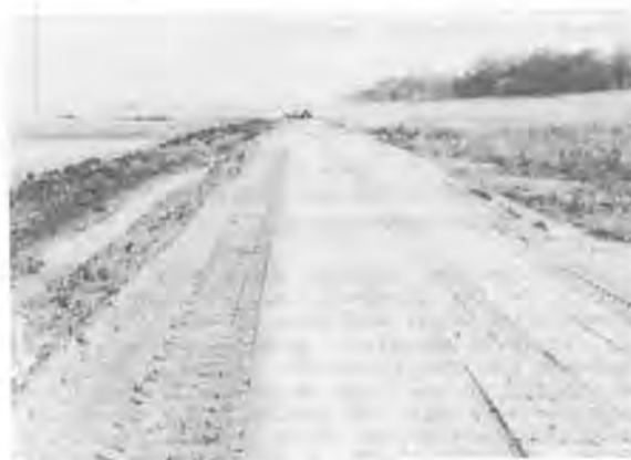
Figure 1 Site and Embankment
