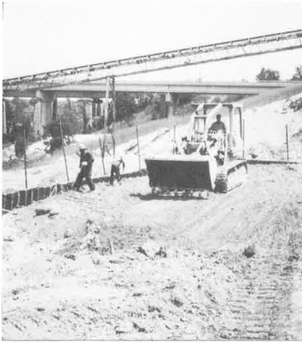
PHOTO 10 COMPACTING BACKFILL, TEST WALL NO. 2
