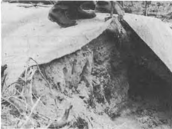
Figure 6 - Cut section of sausage showing filling material already settled.
