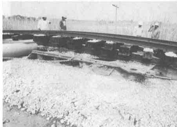
Figure 5. Geotextile Inserted Behind Sled
