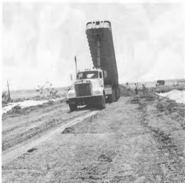
Photo 2 Fill material for construction of the working pad is back-dumped.
