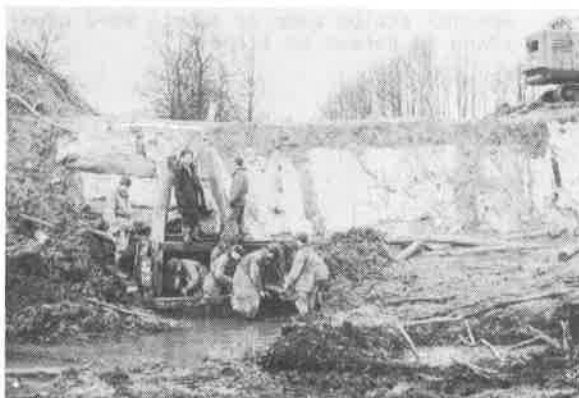
Phot.2 Earth dam during construction, with aid of geotextiles.
