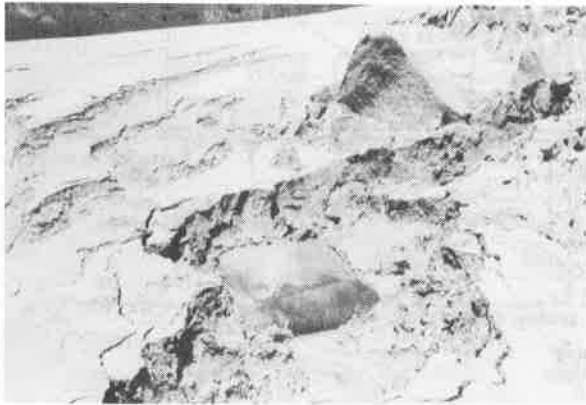
Photo 1 : ERGO Tailings dam - Exposed filter drain, no physical damage to fabric.
