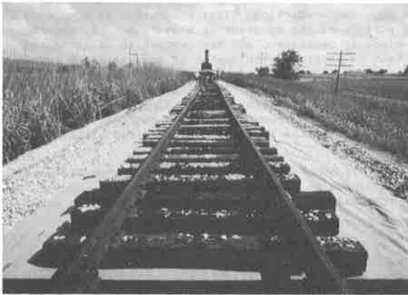
Figure 6 Track Structure on Geotextile After Insertion Behind Track Sled
