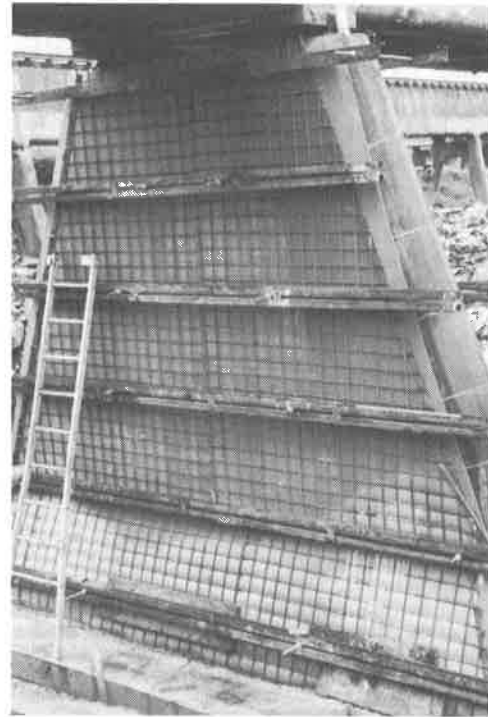
Figure 4b the flexible formwork being filled
