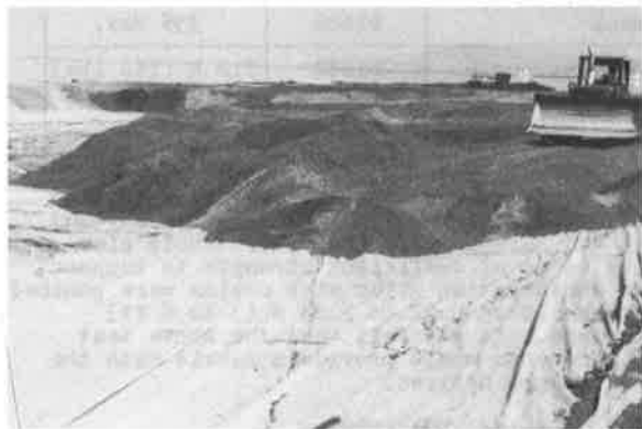
Photo 2 Lightweight fill (sawdust) placement on reinforcing fabric for main embankment.
