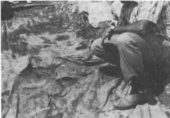
Fig. 7 Typical Test Section Showing Tears and Punctures
