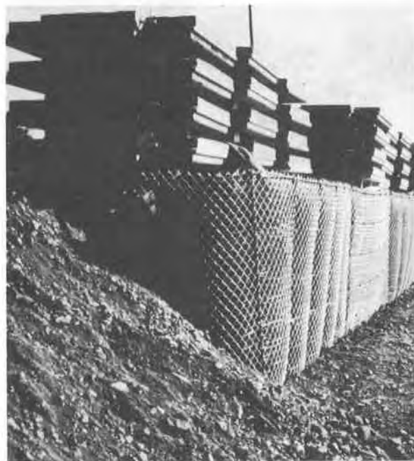
PHOTO 5 LOAD TESTING TEST WALL NO. 1
