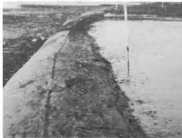
Figure 7 - Final phase of hydraulic construction.
