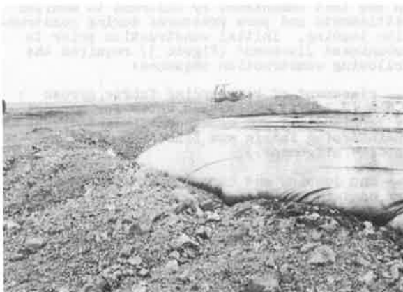
Photo 3 Soft mud contained by reinforcing fabric.
