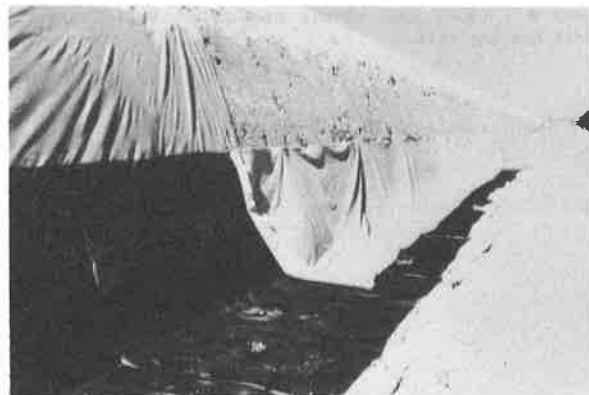
Photo 7 : Placing of laminated filter drain.
