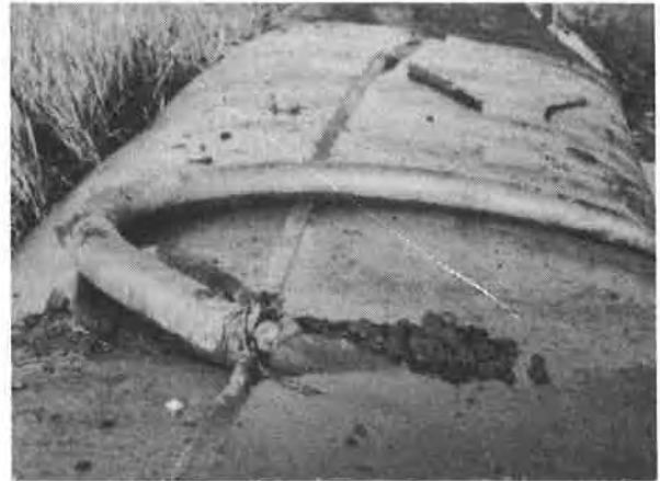
Figure 4 - Sausage filling through a flexible plastic pipe.
