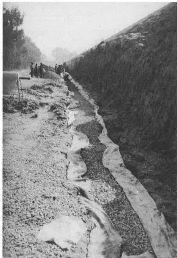
Photo 6 : Toe drain under construction - Trench backfilled with filter stone.
