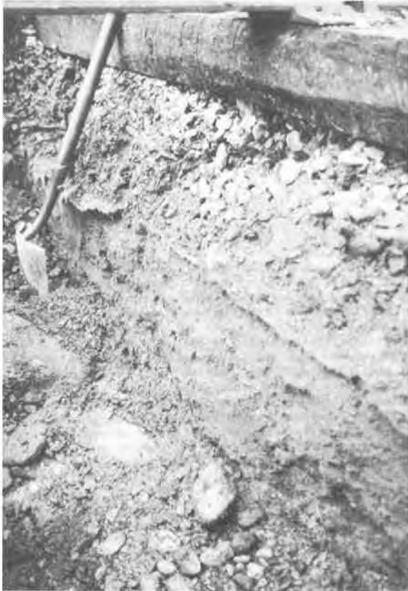
FIGURE 1 TYPICAL GEOTEXTILE EVALUATION EXCAVATION
