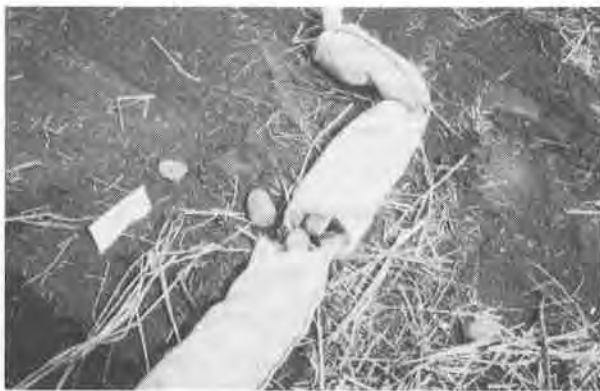
Egypt: Zawia, 100 mm geotextile tube drain.
