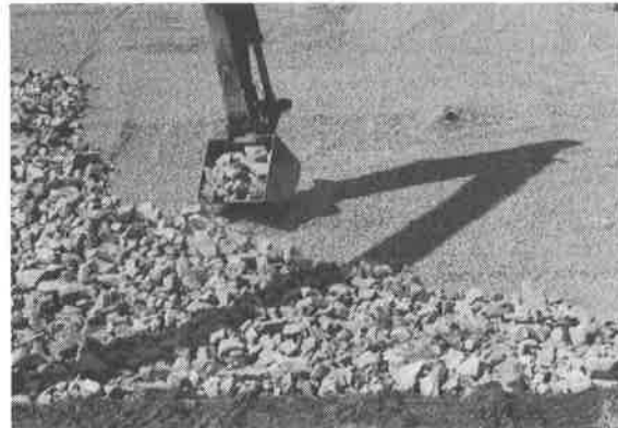
Fig. 8 Crushed Stone Blanket Placed Between Riprap and Filter Cloth
