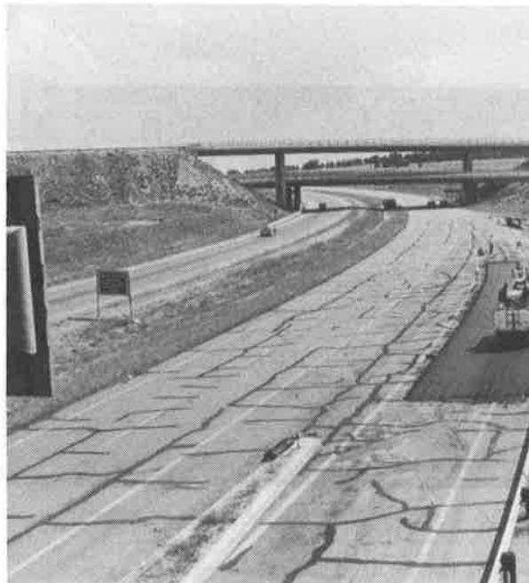
Fig. 4 General View of Site during Construction of Test Section
