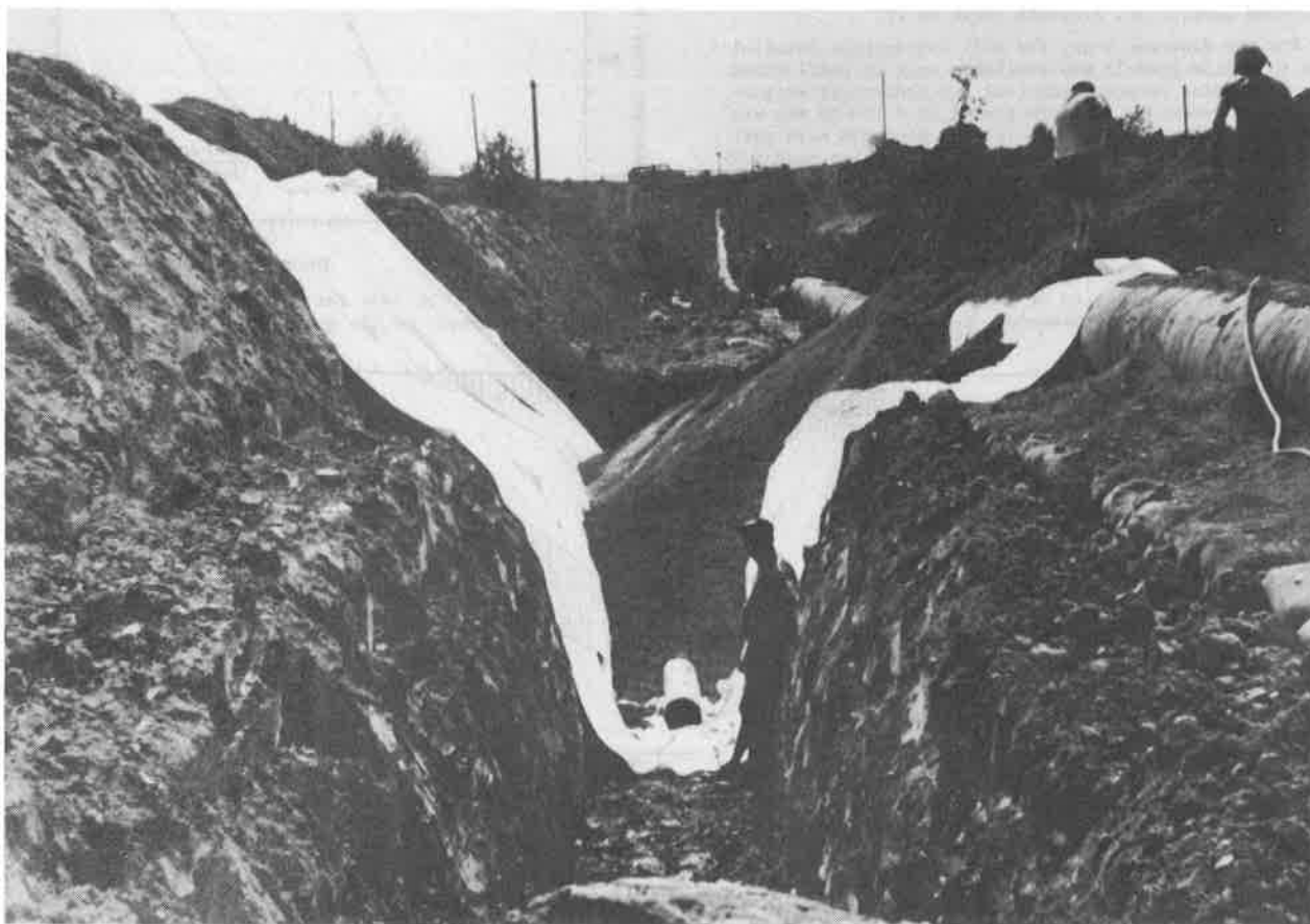
Fig. 5 View of the drainage trench along the pipeline during construction.
