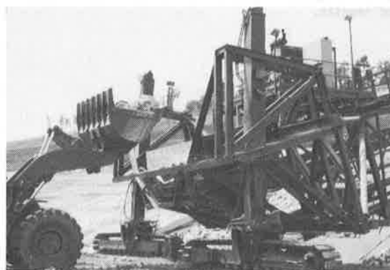
Fig. 11 Riprap Machine Fed by Front End Loader
