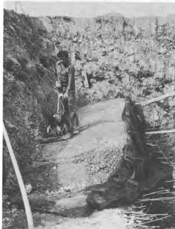
Fig. 6 IGB stability slope, partly constructed
