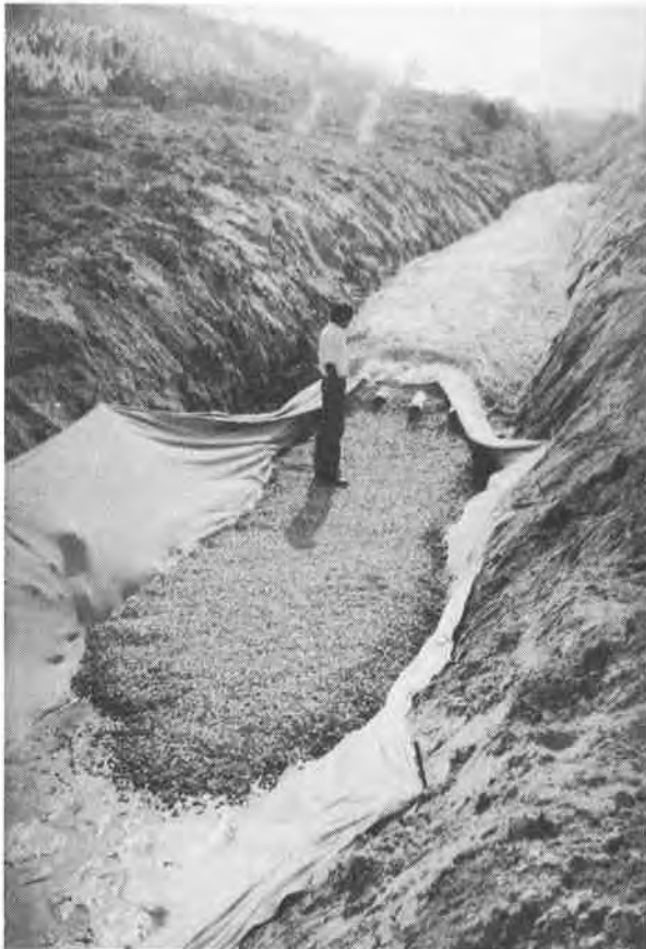
Photo 8 : Crown Sand Slimes Disposal - Filter drain under healing wall.
