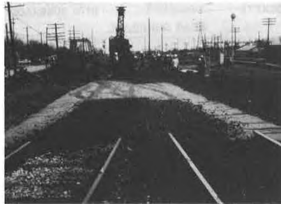
Figure 12. Geotextile Turnout Package Being Installed under switch.
