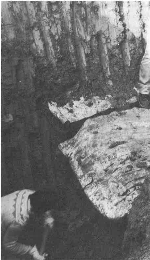
Fig. 6 Excavating the exploration pit.
