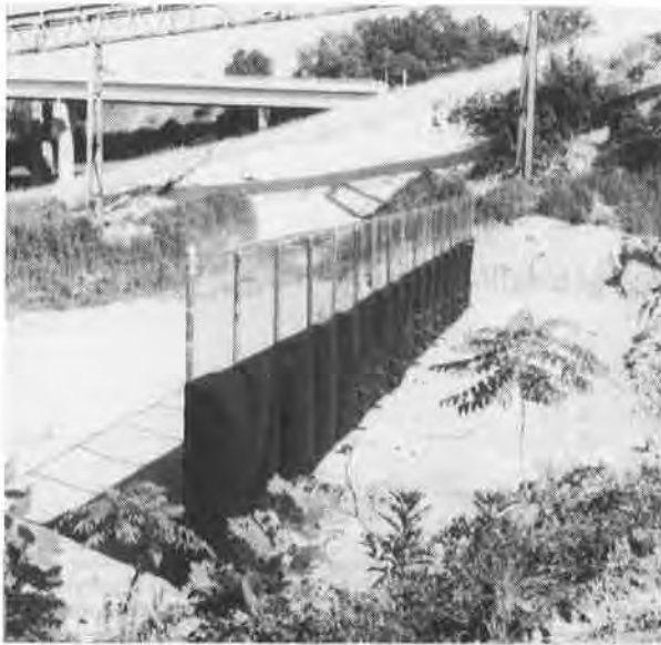
PHOTO 2 TEST WALL NO. 3, BEFORE BACKFILLING
