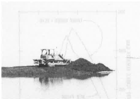
Photo 1 Dike construction in open water
