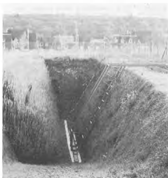
Fig. 10 Travelling framework for control measurements on the slope
