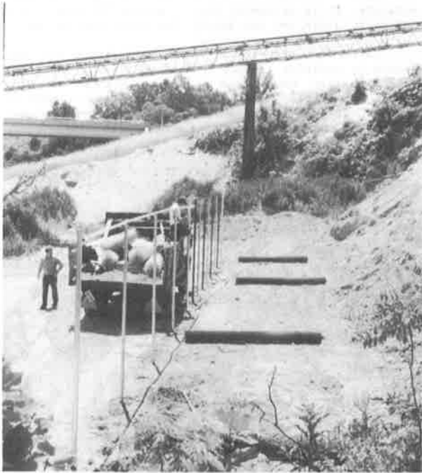
PHOTO 6 HANGING FABRIC FACING, TEST WALL NO. 3
