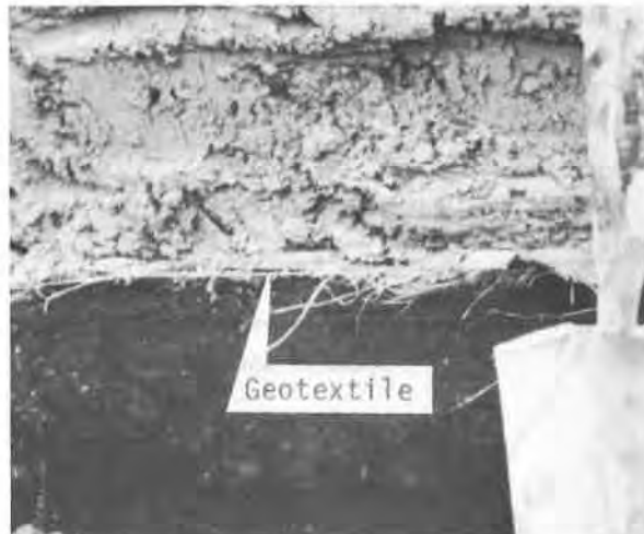
FIGURE 5 - Fill, Peat interface with Geotextile
