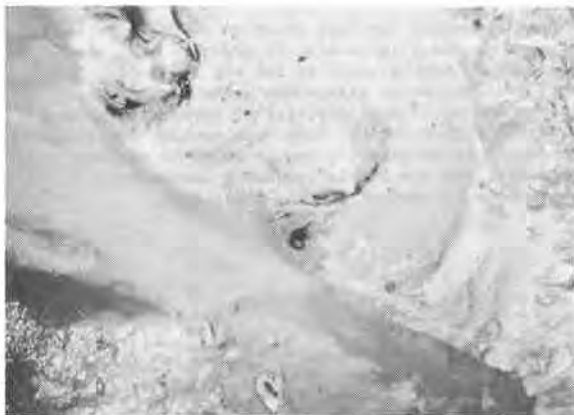
Figure 11. Mud Swirls From Under Track Indicating High Pore Pressures
