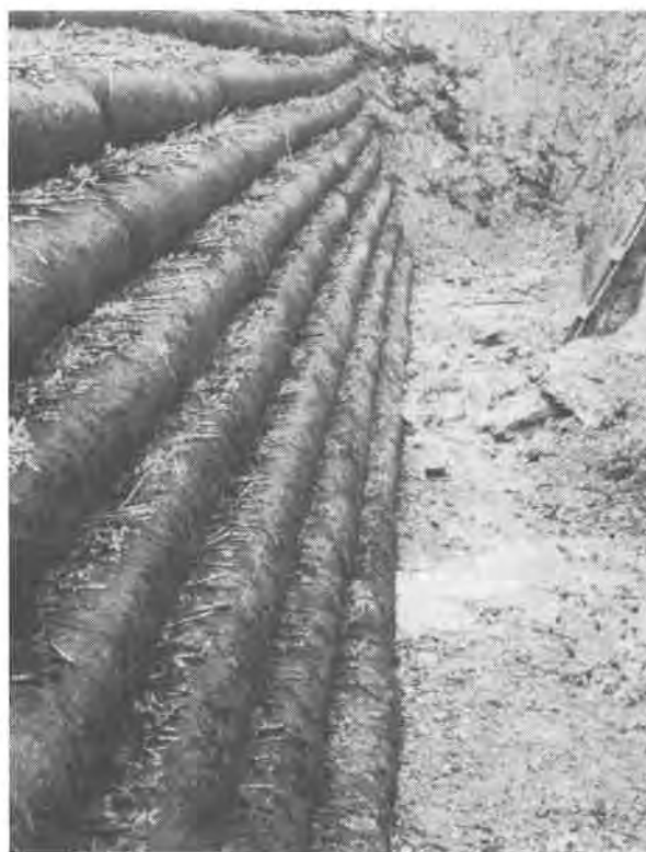
Fig. 8 IGB stability slope, partly constructed
