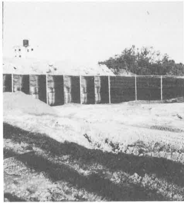
PHOTO 12 TEST WALL NO. 3
