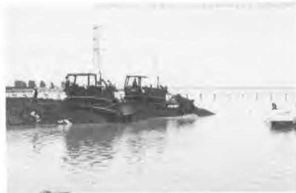
Photo 6 View showing dozers pushing dike embankment forward over fabric in open water. Fabric is being spread by small barge in right of photo.
