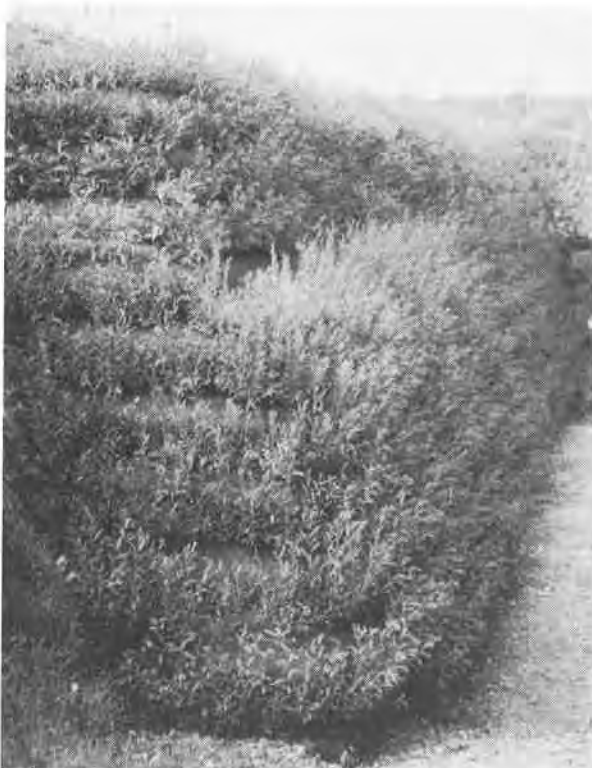
Fig.11 Condition of the IGB stability slope after two months
