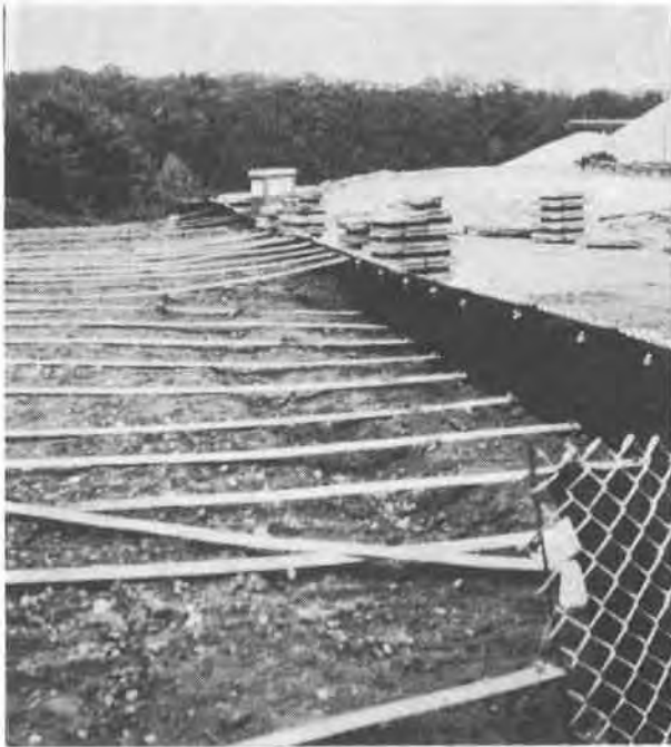
PHOTO 4 REINFORCED EARTH STRIPS, TEST WALL NO. 1
