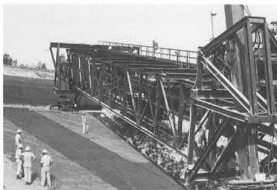
Fig. 10 Closeup of Riprap Machine
