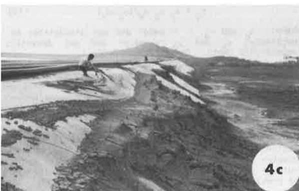
Fig. 4 Phenomena likely to damage a geomembrane by mechanical actions: (a) crack in a cement stabilized aggregate drainage layer (the geomembrane could burst through such a crack); (b) geomembrane wrinkled during the placement of fresh concrete in a full scale test; (c) geomembrane stretched and pulled out from its anchor trench by sediments having slid during a rapid draw-down of the reservoir.
