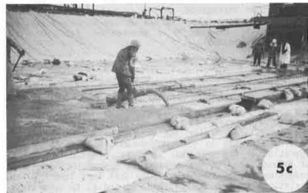
Fig. 5 Use of geotextiles to protect geomembranes: (a) geomembrane (black) placed on a geotextile (white) on a cracked cement stabilized aggregate drainage layer (see Fig. 4a); (b) concrete being poured on a geotextile protecting a geomembrane used to line a canal; (c) concrete being placed on a geotextile (white) protecting a geomembrane (grey).
