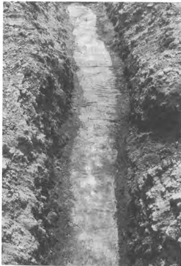
12. View of fabric in trench across section 4A.
