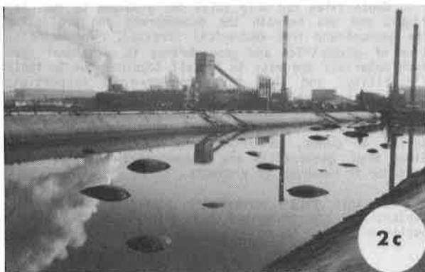
Fig. 2 Detrimental effects of fluids: (a, b) when water is pumped from the ditch, the geomembrane moves inward, pushed by the pressure of water entrapped underneath; (c) geomembrane uplifted by gas; (d) bank deformed by wave action after the dike has been softened by water leaking from the pond (in the middle of the bank, a pipe is protruding under the geomembrane); (e) the sand layer has been displaced by wave action and stones are in contact with the geomembrane; (f) slide under the geomembrane; (g) localized subsidence due to piping.
