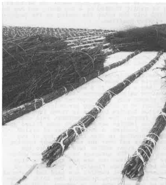
Photograph 2 - Fascines and bush bundles.
