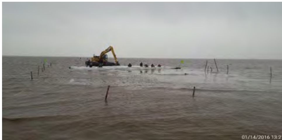
Figure 13. High strength basal reinforcement over bamboo mattress.
