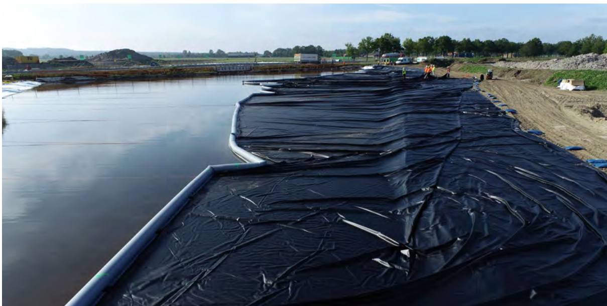
Figure 4. Geomembrane being pulled across the water surface using ropes
