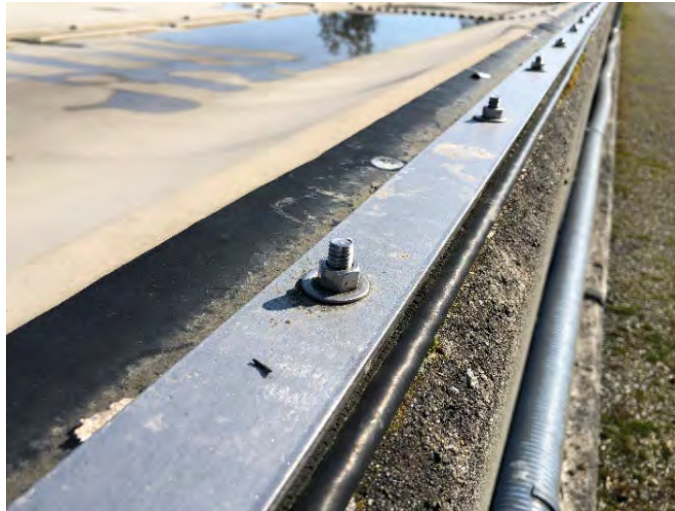
Figure 10 Floating cover mechanical anchorage at parapet wall
