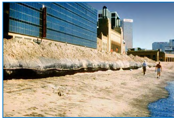
Figure 5. Erosion stopped by geotextile tube sand dune core
