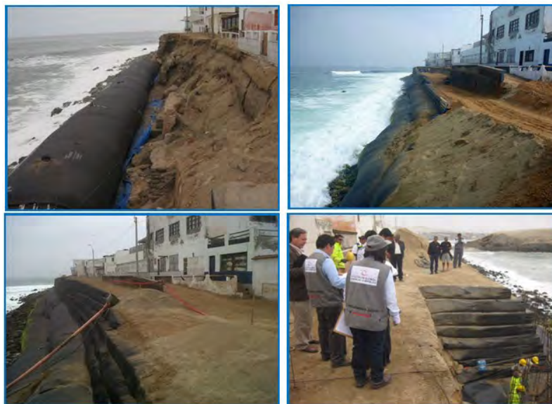
Figure 23. Punta Hermosa erosion protection project construction sequence
