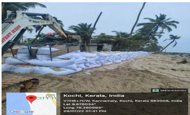
Figure 11. Two Photographs of Geotextile Bags as Temporary Coastal Protection Works. (Source: KID 2021-22)
