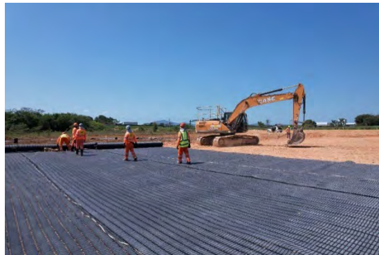
Figure 8 – Installation of the 1750 kN/m Geogrid
