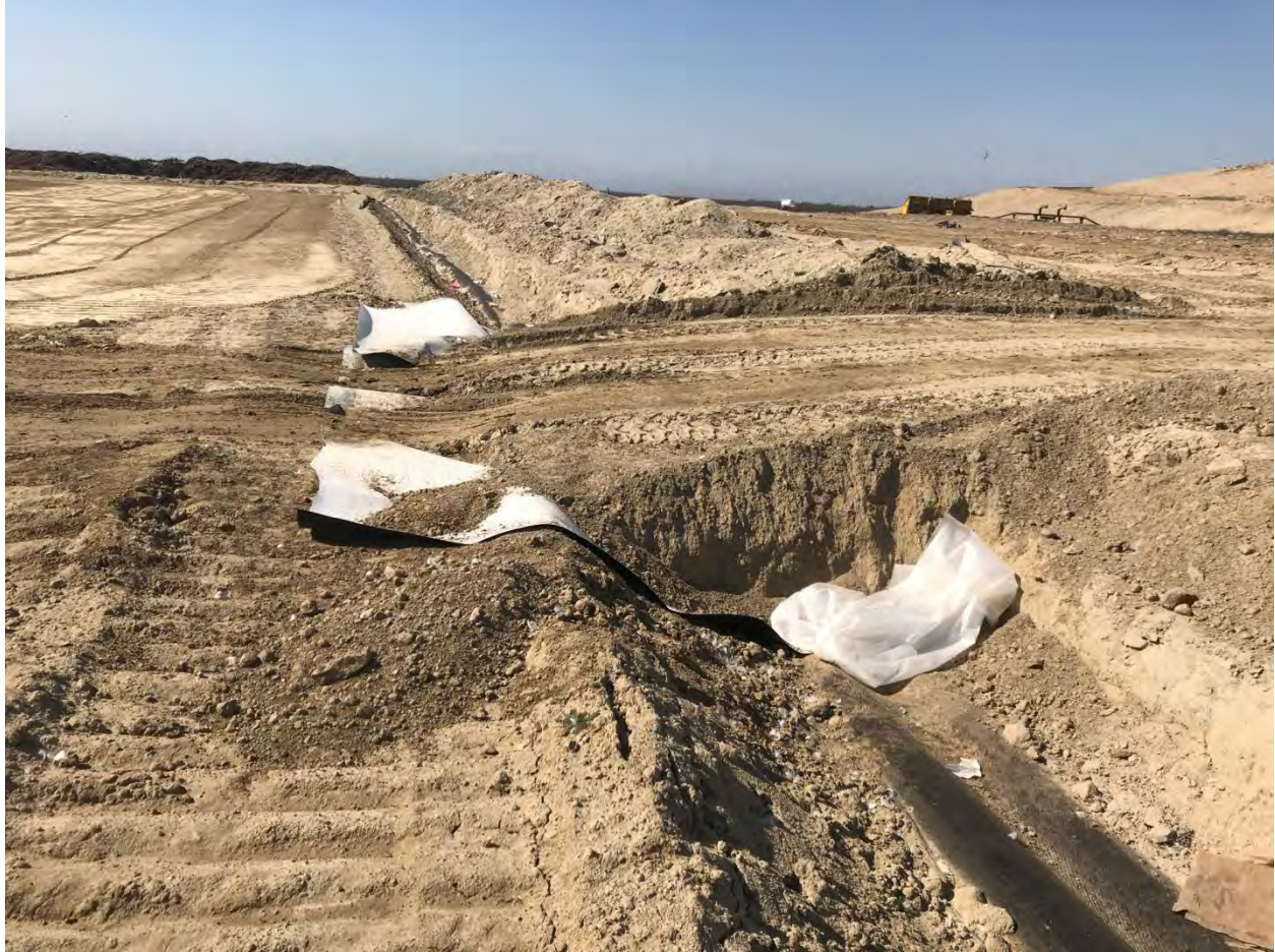
Figure 2. Method of Electrically Isolating Access Roads
