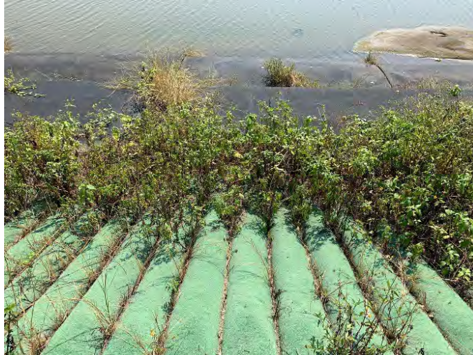
Figure 17. Close up of sand filled mattress covered with vegetation.
