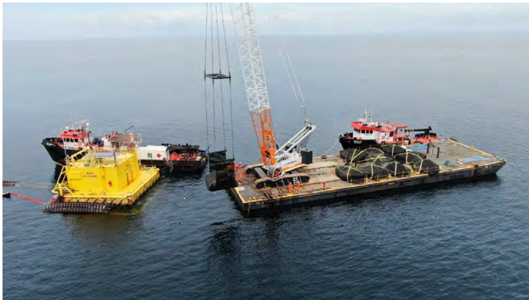
Figure 7 – Geotextile Bag Lifting Harness and Installation
