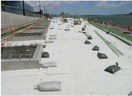
Figure 9. Geofoam with adjacent planters and knee wall construction.
