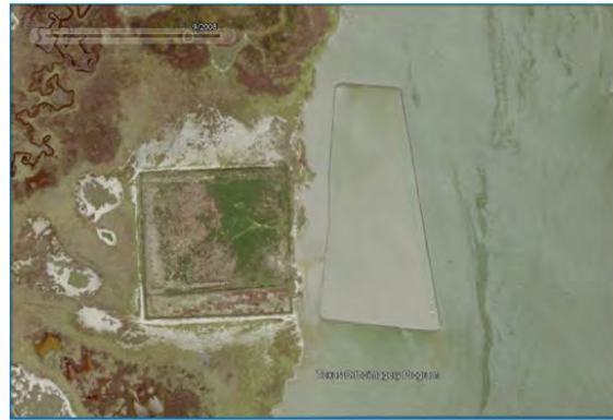
Figure 9. 2006 - Completed disposal site
