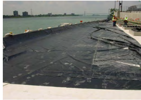
Figure 10. Geomembrane Installation over Geofoam.
