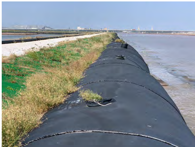
Figure 15. Sand filled mattress covered with vegetation after 9 months.
