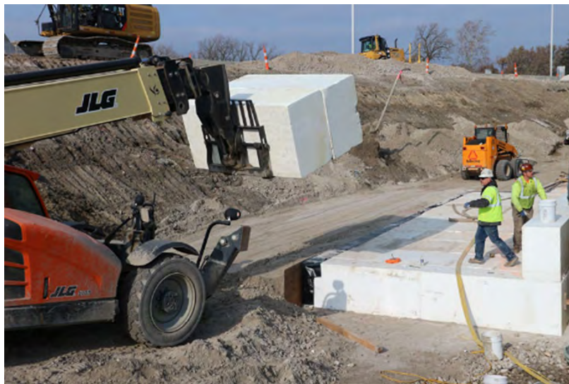
Figure 3. Placement of Geofoam on project site. I75 Toledo OH USA
