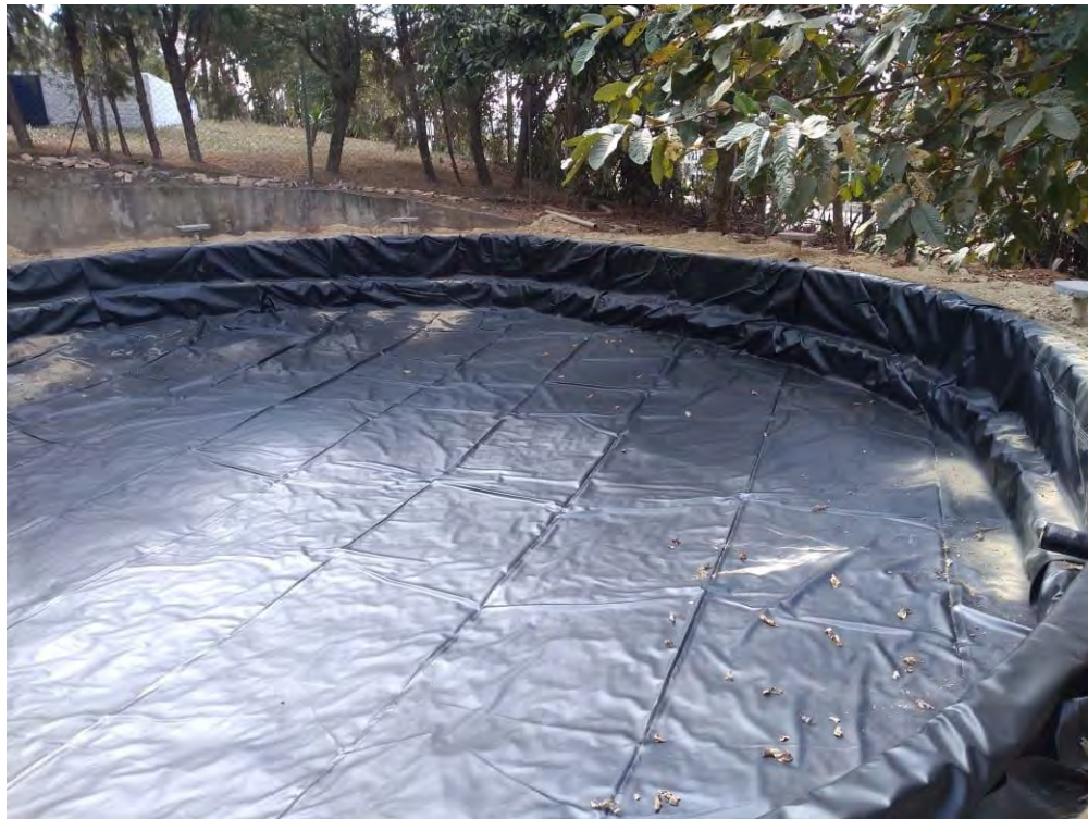
Figure 5: Circular tank coated with PVC geomembrane
