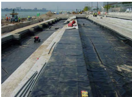
Figure 11. Geomembrane deployed over Geofoam.
