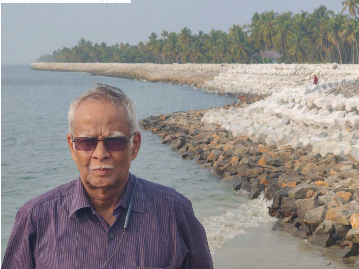
Figure 5. A Rubble-Mound Seawall with Concrete Tetrapod as Armour Layer Reach Under Construction at Challam Coast (Nov 2022). (Source: KID 2022)
