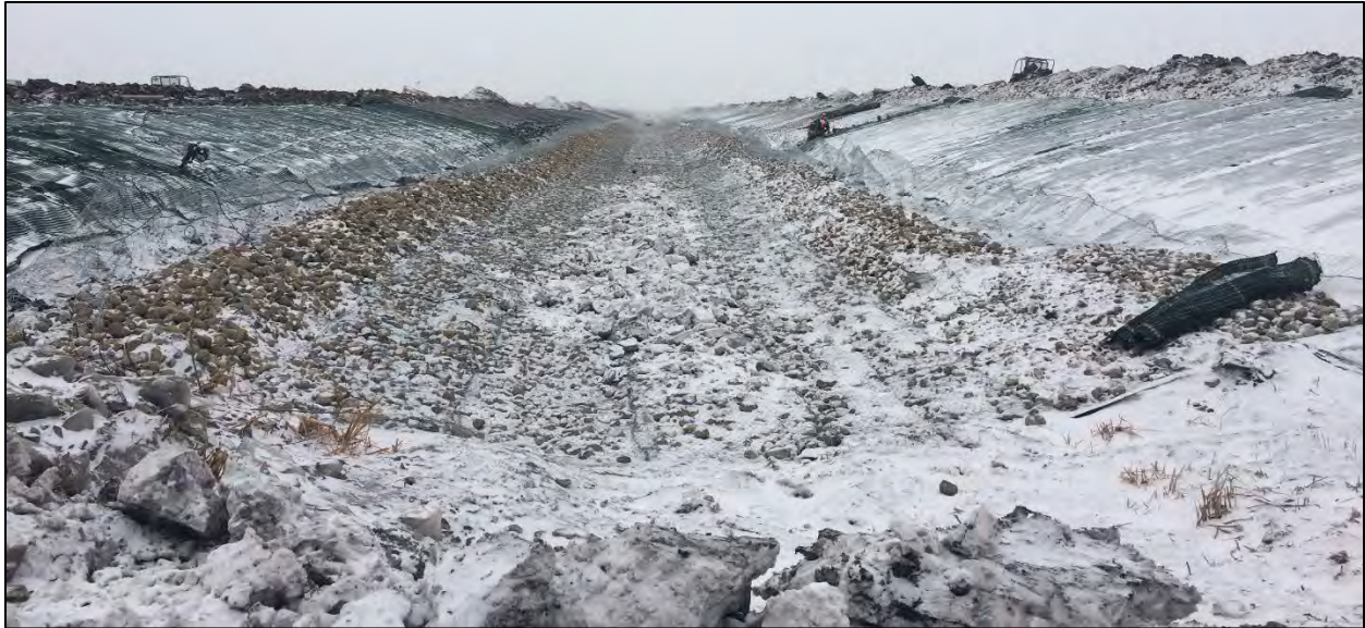
Figure 5. Winter Installation of Gabion Mattress and EEAS (01/2018)
