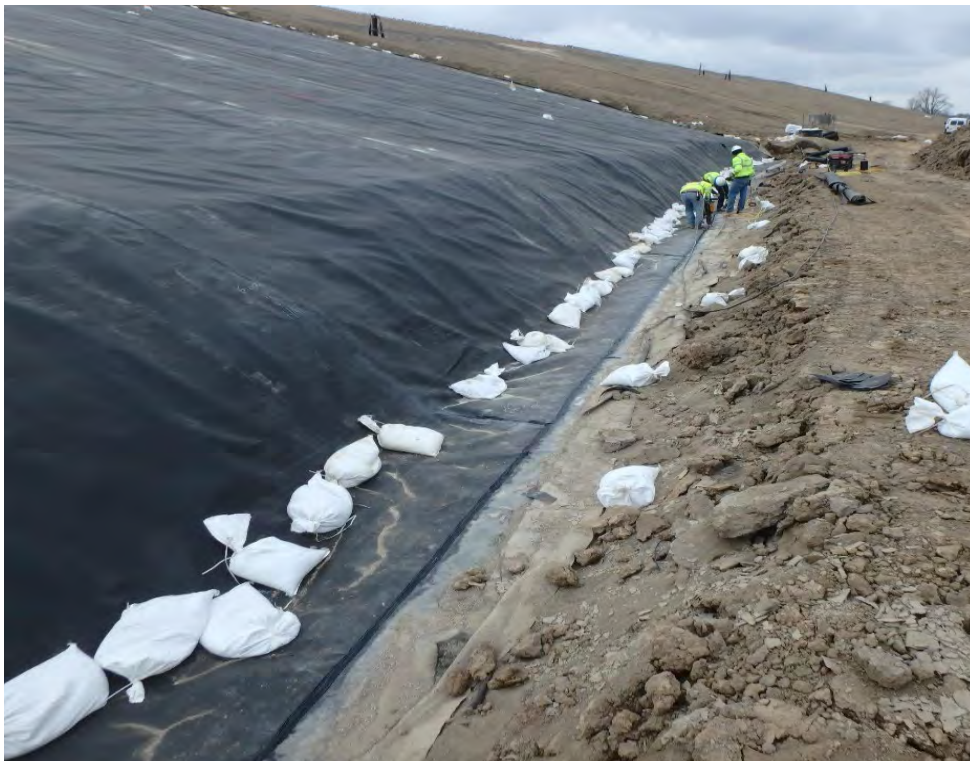
Figure 9 – Welding of EGC to Baseliner at Perimeter of a Landfill
