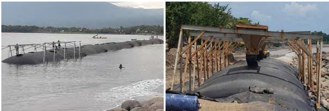
Figure 7. A-frame structure to hold the geotextile tube during filling operation
