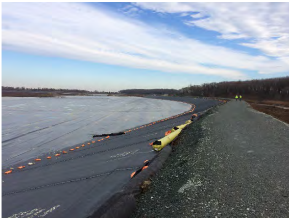
Figure 3. Site photo of deployed geotextile
