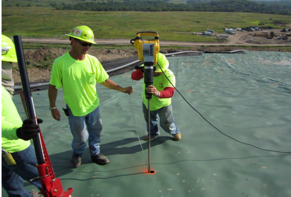
Figure 8 – Platypus Soil Anchors Being Installed to Anchor an EGC
