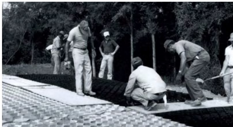
Figure 5. side-by-side testing of HDPE geocells and aluminum geocells at the Waterways Experiment Station, Vicksburg, MS, circa 1979
