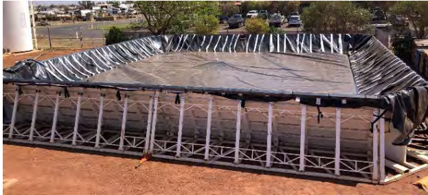
Figure 5. 0.75mm proprietary polyolefin rain cover on a coal seam gas frac storage to eliminate rainfall intermingling with stored fracking liquid. NT, Australia. (Image: MPC, 2018)
