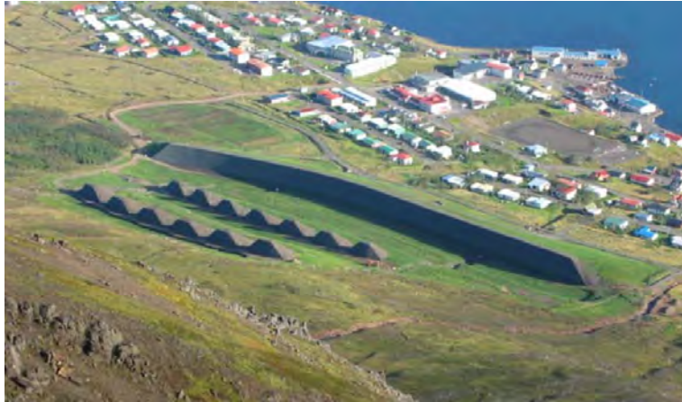
Figure 3. Avalanche control facility in Neskaupstaður, Iceland.
