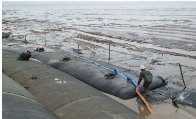
Figure 10. Scour apron pumped to an inflated height of 0.5m.
