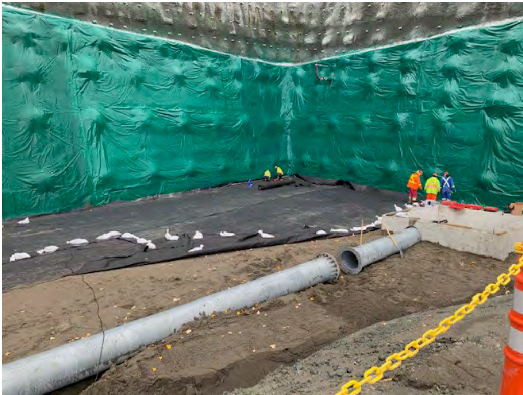
Figure 1. The Finished Floating Liner
