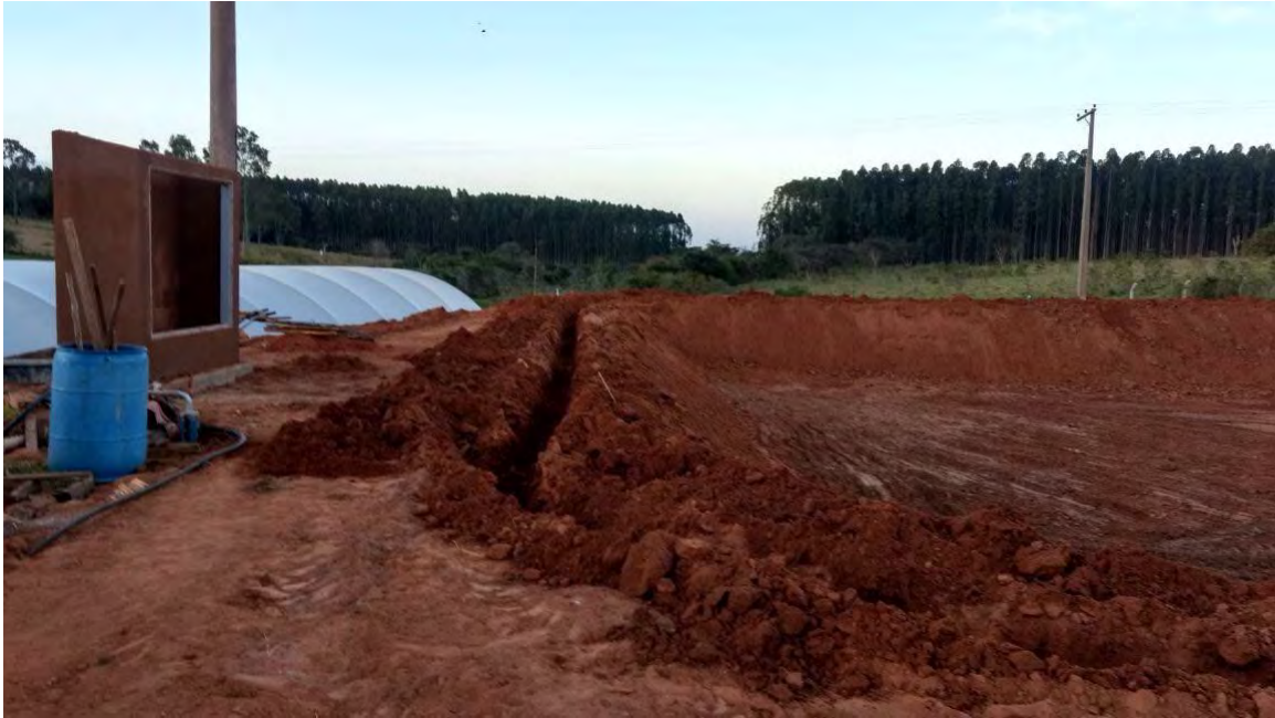
Figure 4: Shape of the excavated tank
