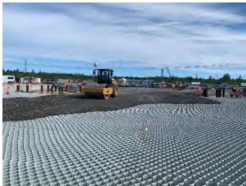
Figure 13. Top layer geocell being built
