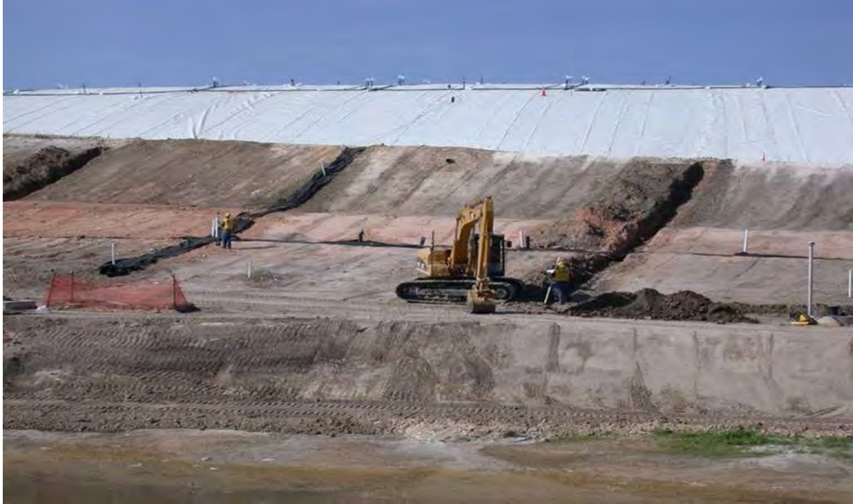
Figure 4 – EGC Anchor Trench Construction
