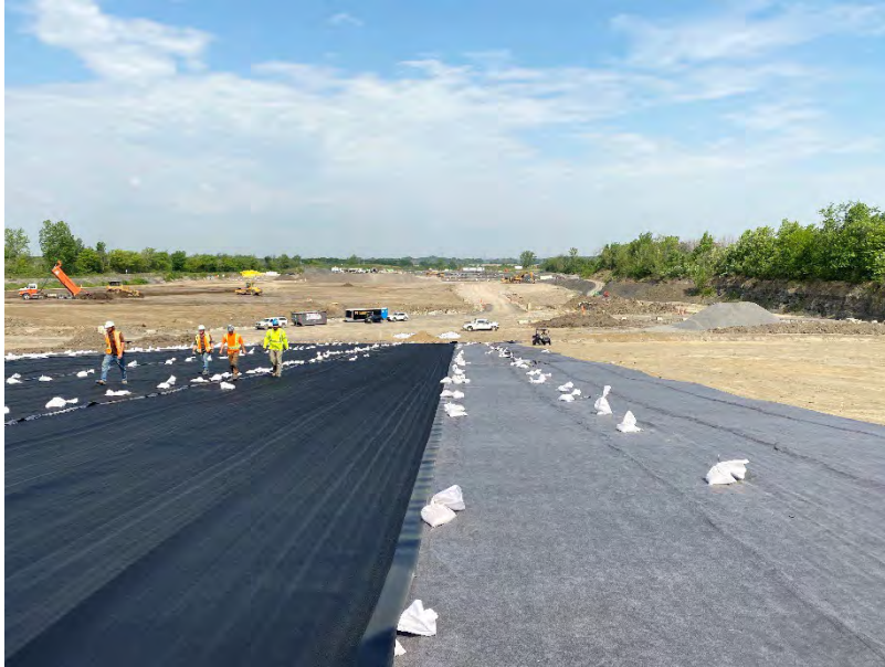
Figure 11. Installation of the geomembrane on the geocomposite
