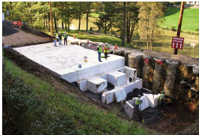
Figure 1. Typical Geofoam Application. Source: EPS Alliance
