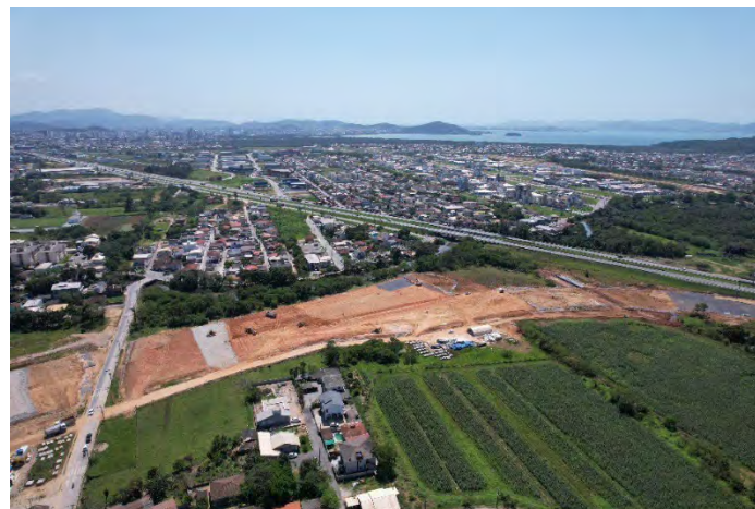
Figure 7 – Construction of embankments along the Florianópolis Ring Road
