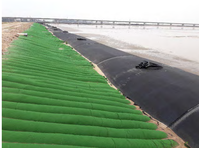
Figure 14. Newly installed sand filled mattress at tube crest.
