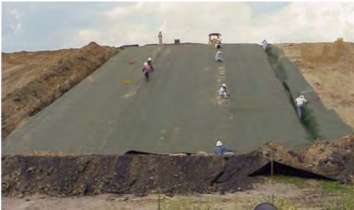
Figure 5 – Placement of an EGC in Prepared Anchor Trenches
