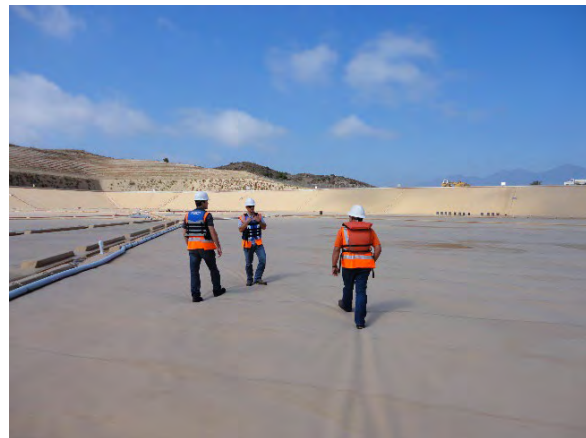
Figure 4. Personnel on cover in full operation
