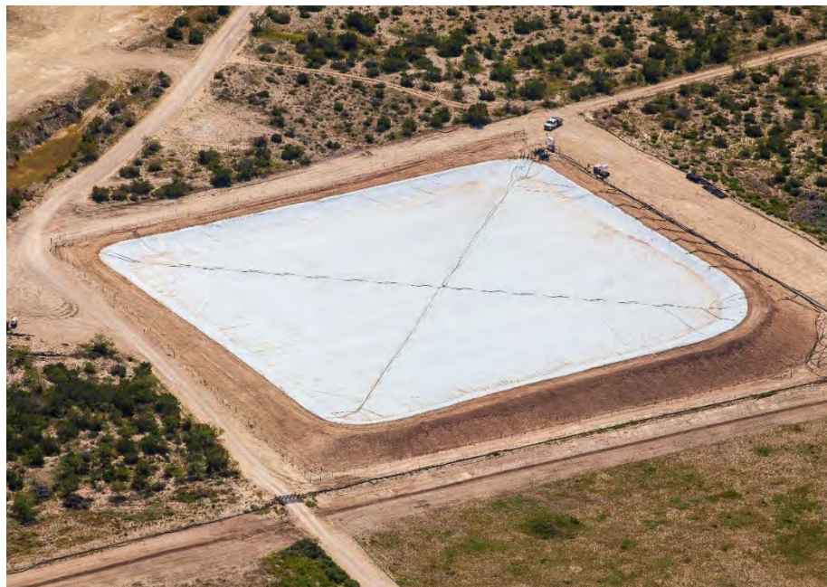
Figure 2. Evaporation control floating cover, West Texas, USA
