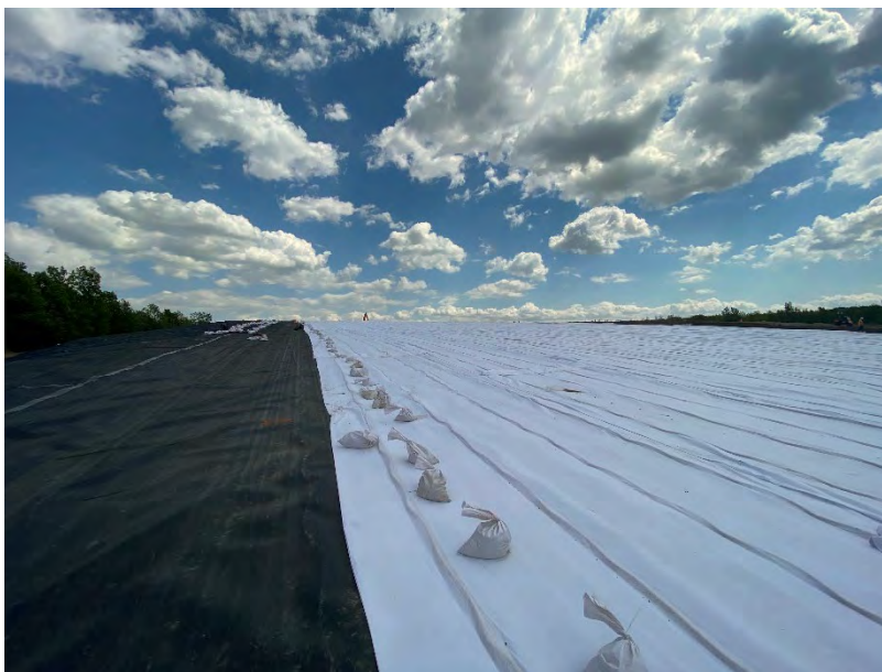
Figure 12. Infiltrated rainwater drainage geocomposite
