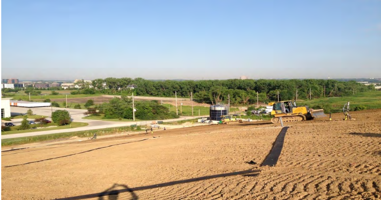
Figure 3 – Installation of EGC Undercap Flat Drains for Gas Control
