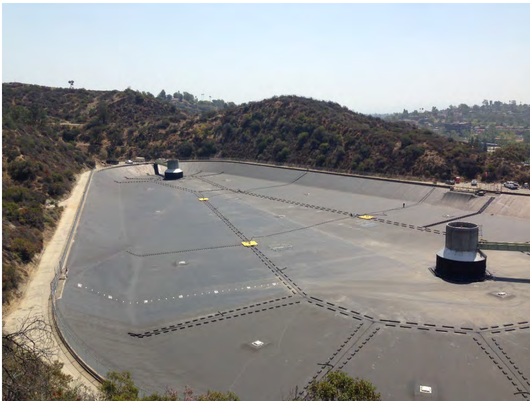
Figure 1. 350,000 ft 2 Floating Cover Eagle Rock Reservoir, CA USA
