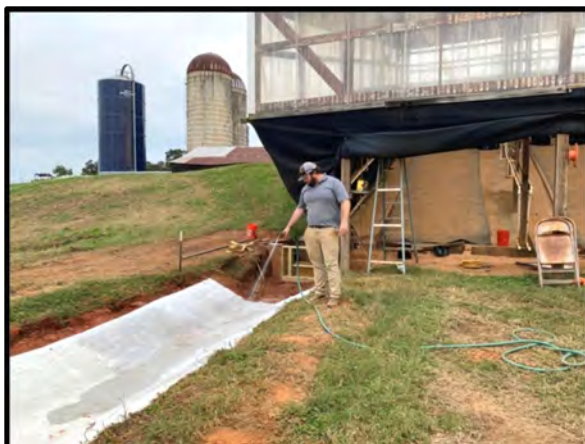
Figure 13. Spraying Water to Hydrate Product
