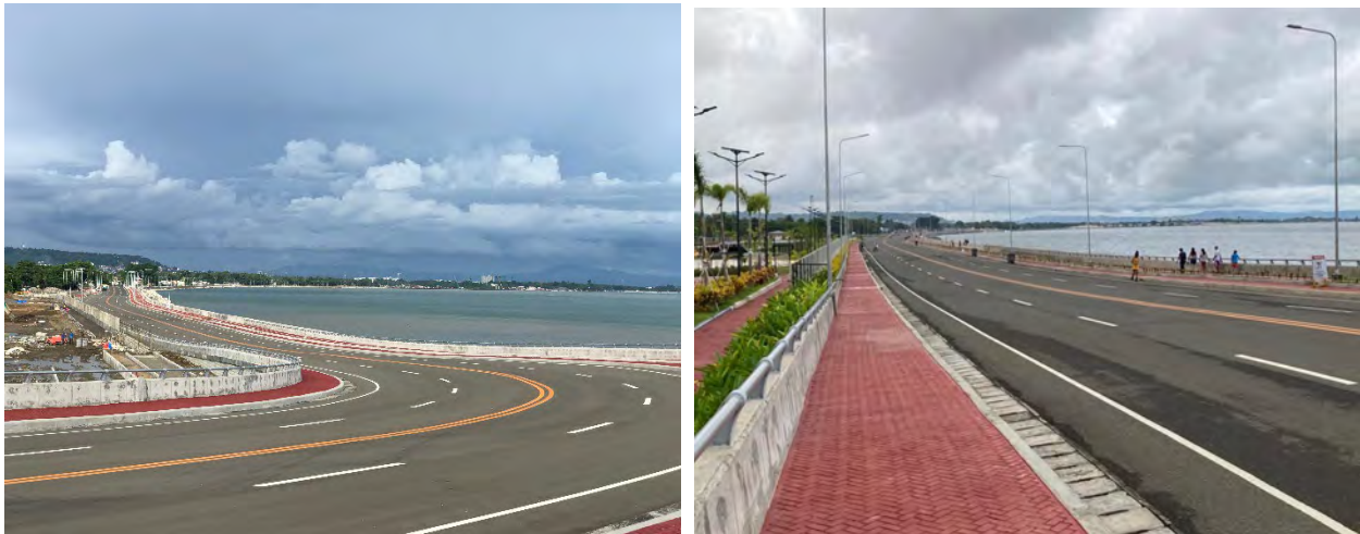
Figure 12. Overview of completed coastal road project
