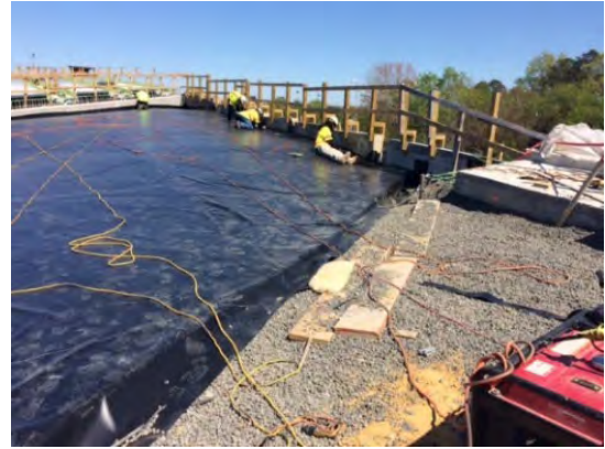
Figure 7. Geomembrane completion over Geofoam. Norfolk VA USA
