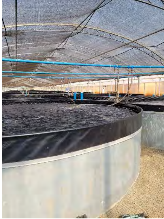
Figure 3: Suspended galvanized sheet tank
