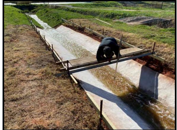
Figure 16. Depth Measurements used a Point Gauge
