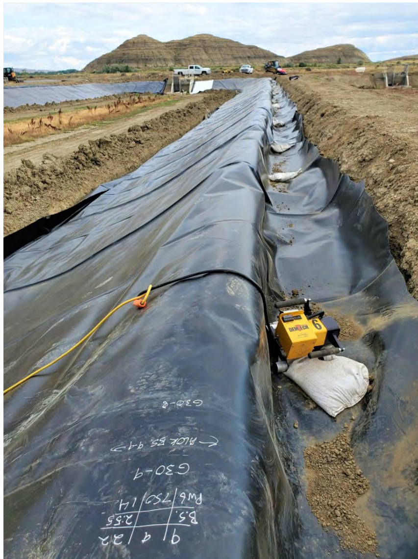
Figure 1. Slopes only liner, trenches top and bottom represent 40% of total liner needed
