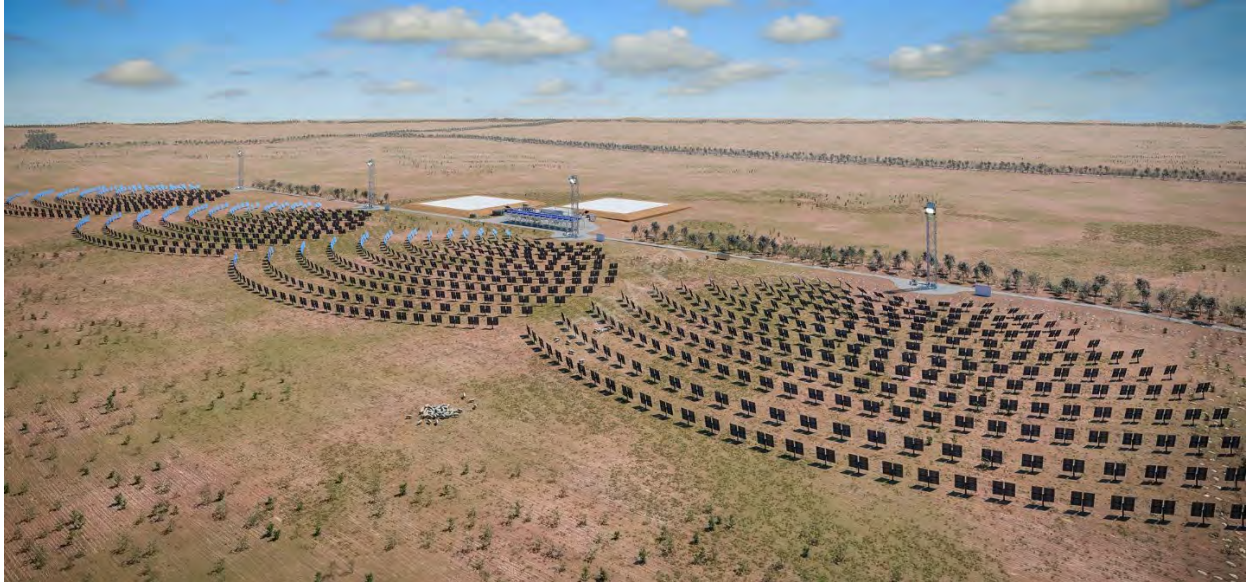
Figure 9. Bi-modal HDPE insulated floating cover on a thermal pit storing hot water for power generation using a thermally driven Organic Rankine Cycle (ORC) engine. Victoria, Australia. (Image: Raygen, 2021).
