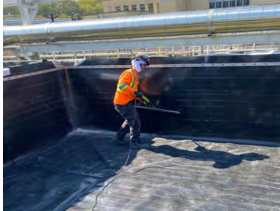
Figure 5. Technician performing arc testing on the primary liner
