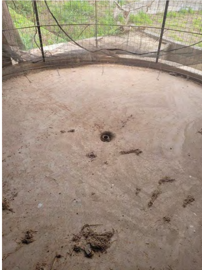
Figure 1: Drainage system for cleaning
