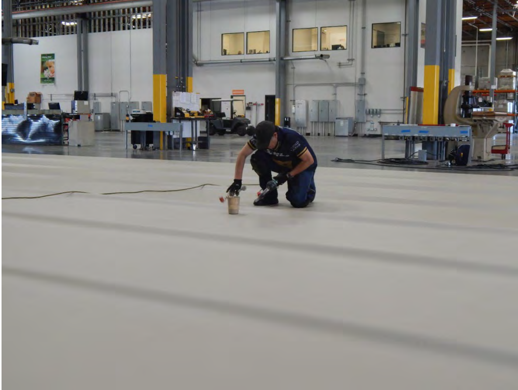
Figure 11. Factory fabrication of CSPE panels in Lakeside CA plant
