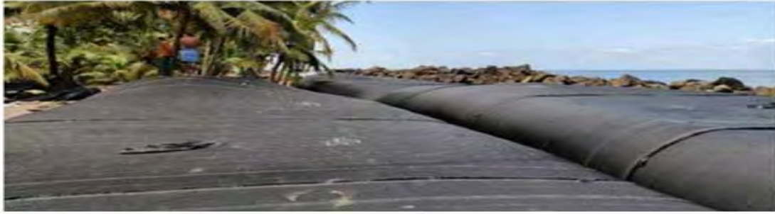
Figure 10. Geosynthetic Tubes as Seawalls for Coastal Protection, Pilot project at Neerkunnam Beach, Alappuzha (2018). (Source: KIIDC)
