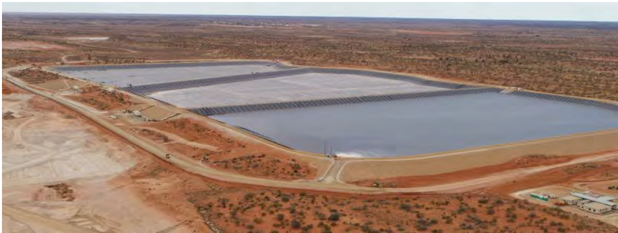
Figure 3. The completed storage facility in operation.
