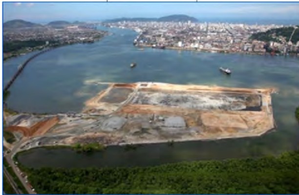
Figure 16. Partially constructed perimeter dike
