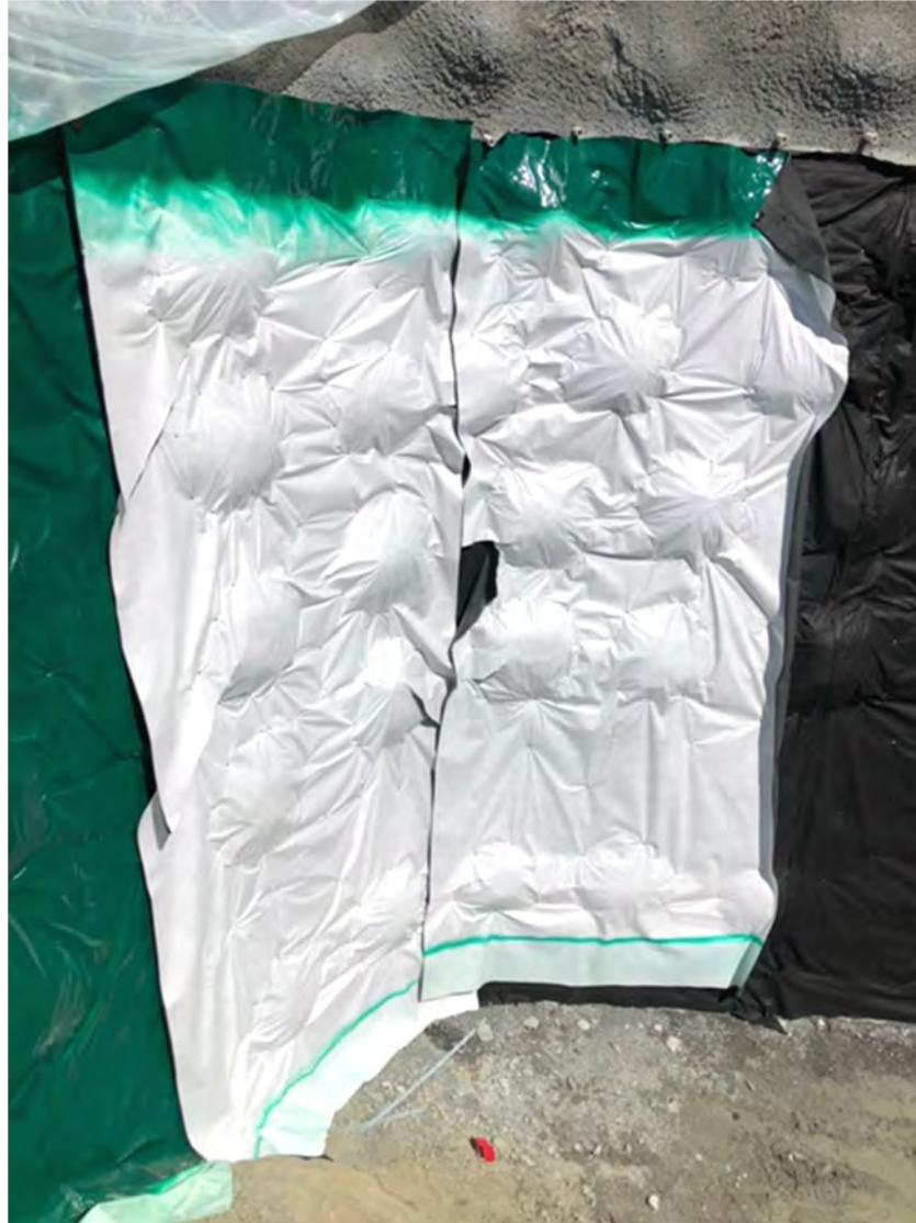
Figure 3. Conforming the Geotextile into A Corner
