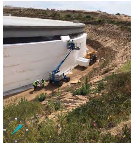
Figure 14. Geofoam Installation. Note Geomembrane behind and under Geofoam.
