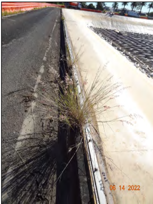
Figure 2. (a) Vegetation growing: (a) under geomembrane batten strip at top of reservoir sideslope and (b) around reservoir instrumentation within bottom liner system.
