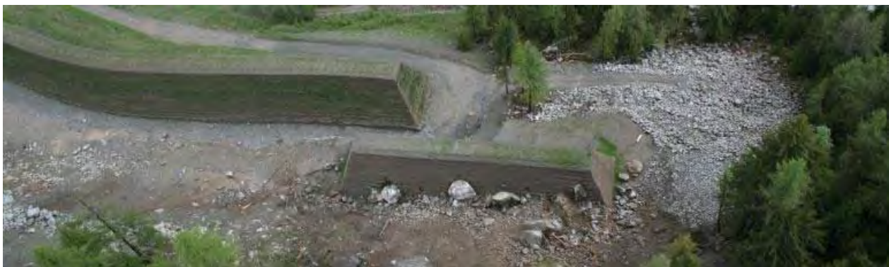
Figure 2. Example of rockfall protection embankment.
