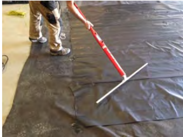
Figure 2. Arc testing on a 3-mil conductive film.
