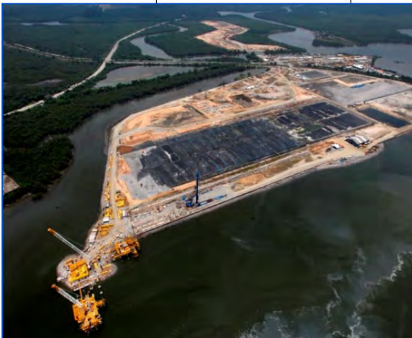
Figure 18. Covering the geotextile tube containers
