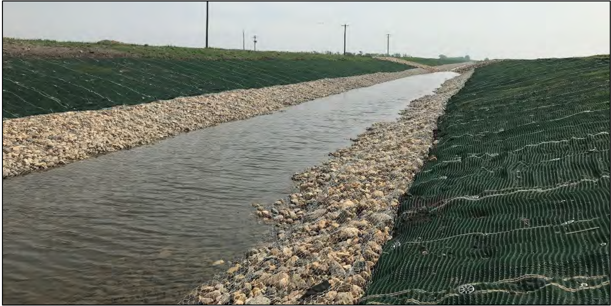
Figure 7. Performance Prior to Vegetation Establishment (05/2018)
