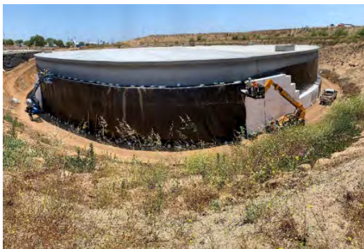
Figure 15. Geomembrane Installation over Geofoam with top closure seam.
