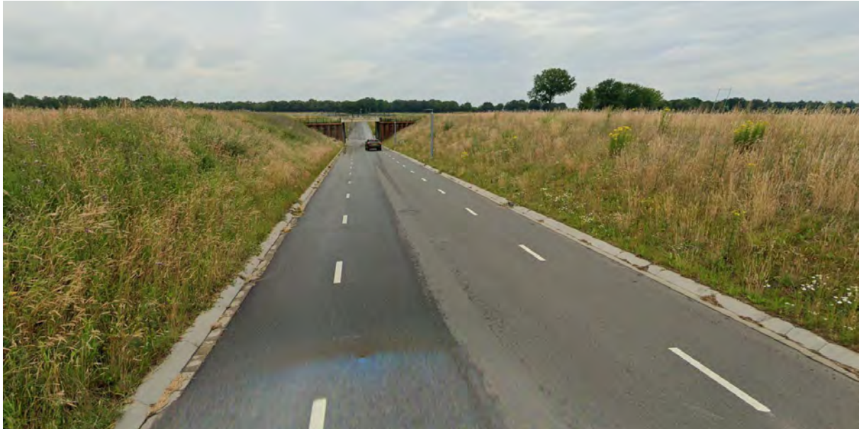
Figure 7. Road view tunnel ramp after 6 months of use
