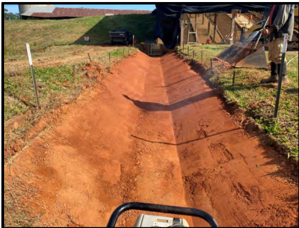
Figure 11. Trapezoidal Channel Prepared
