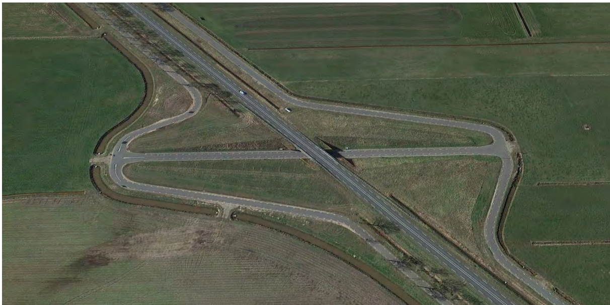
Figure 8. Road aerial view tunnel ramp after 6 months of use
