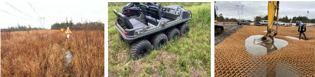
Figure 11. Existing subgrade condition and bottom layer of geocell
