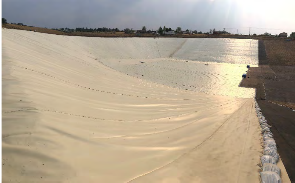
Figure 2. Tan color reinforced geomembrane after installation
