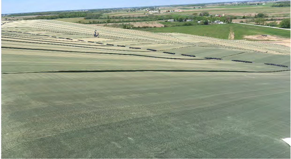
Figure 6 – Installation of a Reinforced Geotextile Windscreen for EGC Anchorage
