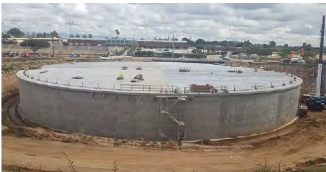
Figure 13. Infiltration Tank Construction.
