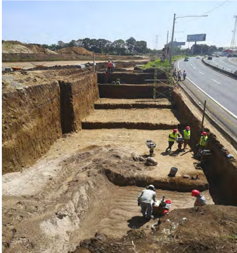
Figure 2. Excavation for the MSME
