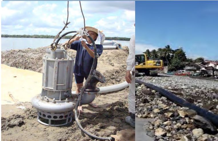
Figure 8. Filling of geotextile tube using slurry pump method
