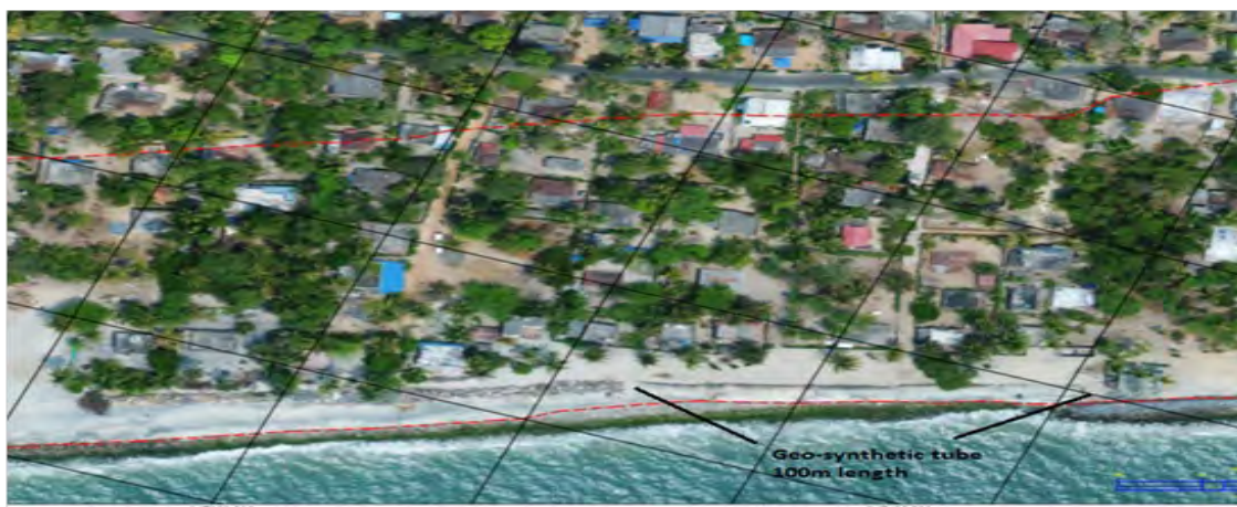
Figure 2. Aerial Photograph of Coastal Reach at Neerkunnam, Alappuzha District, Kerala (Photograph: April 2018) . (Source: KIIDC 2018)
