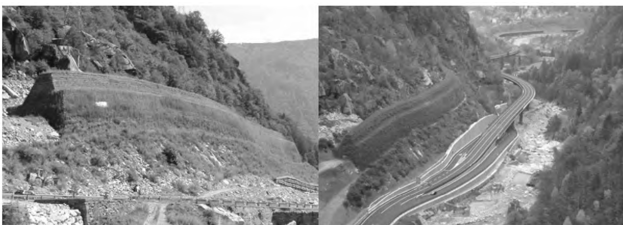
Figure 1. Huge rockfall protection embankment protecting the Simplon road, in Varzo, Italy (Rimoldi et al., 2008).
