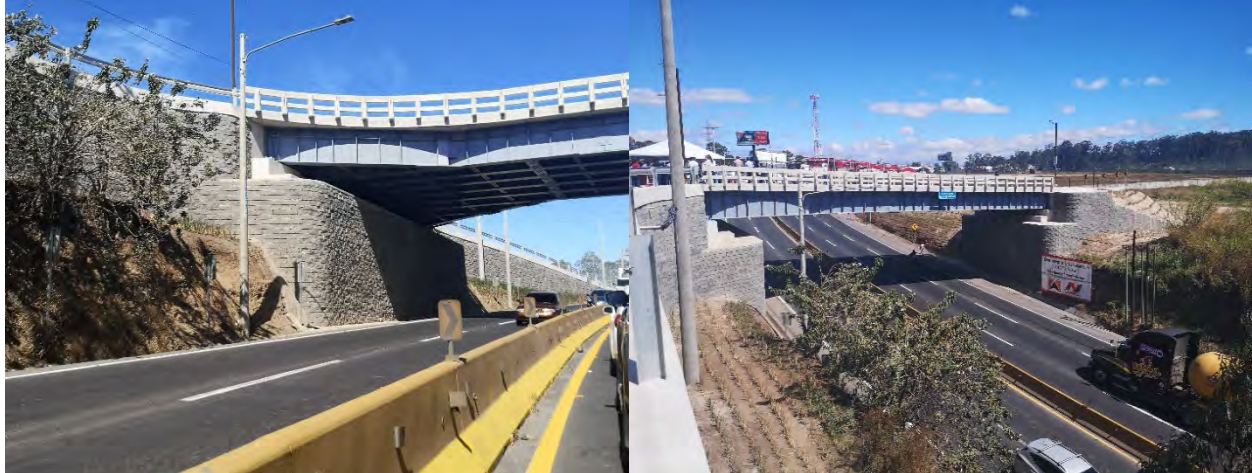
Figure 5: Abutment in service
