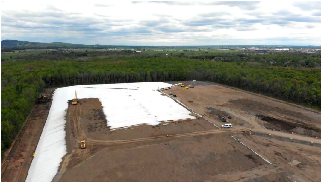
Figure 14. General view of the final cover construction
