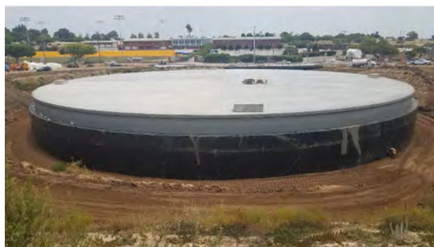
Figure 16. Argo Drain Infiltration Tank Completed Installation.
