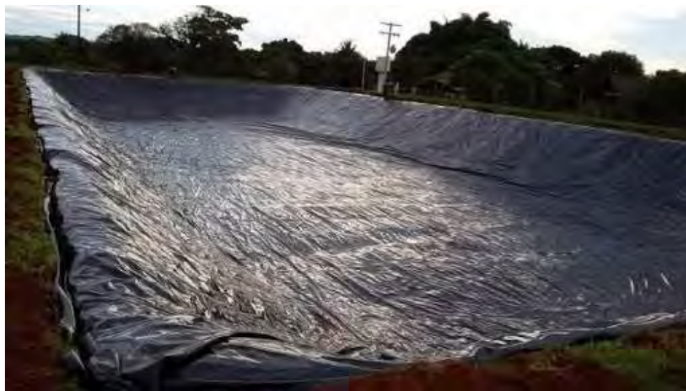
Figure 6: Rectangular tank coated with PVC geomembrane
