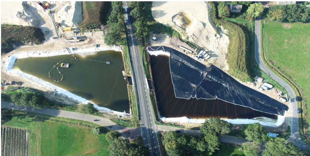
Figure 2. Aerial view tunnel while pulling the geomembrane across the water surface
