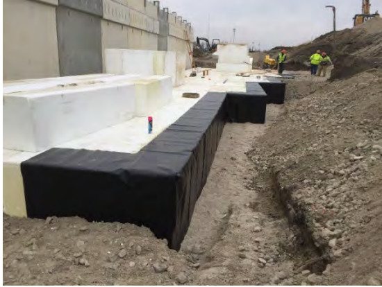
Figure 6. Geomembrane over Geofoam edges. 175 Toledo OH USA
