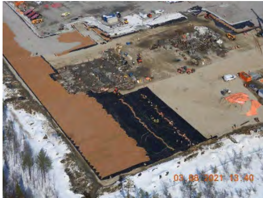
Figure 12. Progress of 3 layers of geocell through winter
