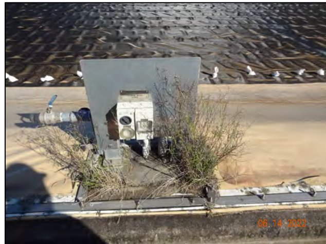
Figure 2. (a) Vegetation growing: (a) under geomembrane batten strip at top of reservoir sideslope and (b) around reservoir instrumentation within bottom liner system.
