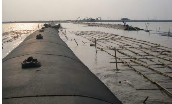
Figure 12. Geotextile tube installation in progress.
