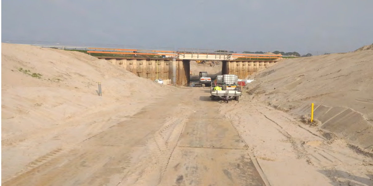
Figure 5. Ramp after backfilling and dewatering
