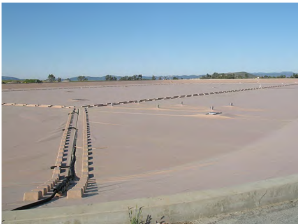
Figure 3. Defined sump cover in operation
