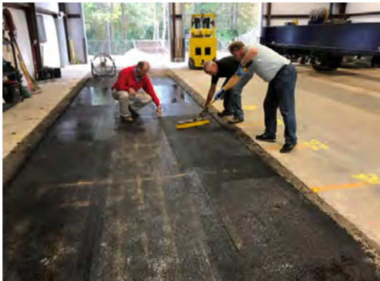
Figure 6: Installation of interlayer fabrics.
