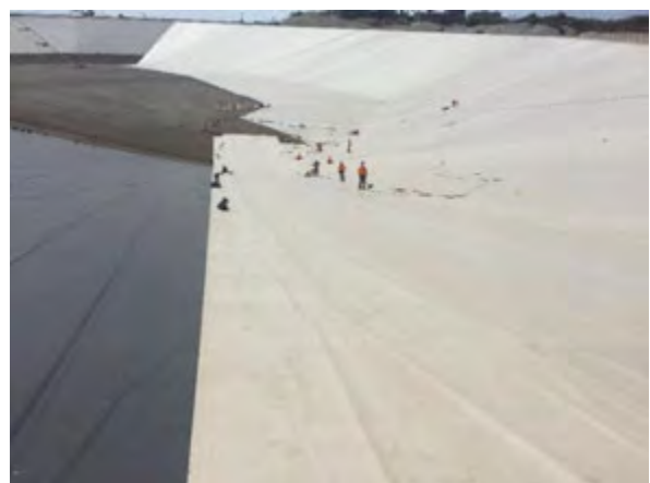
Figure 8. Floating cover and rainwater collection trough progress.
