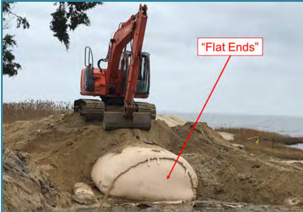
Figure 7: Geotextile tube flat end.
