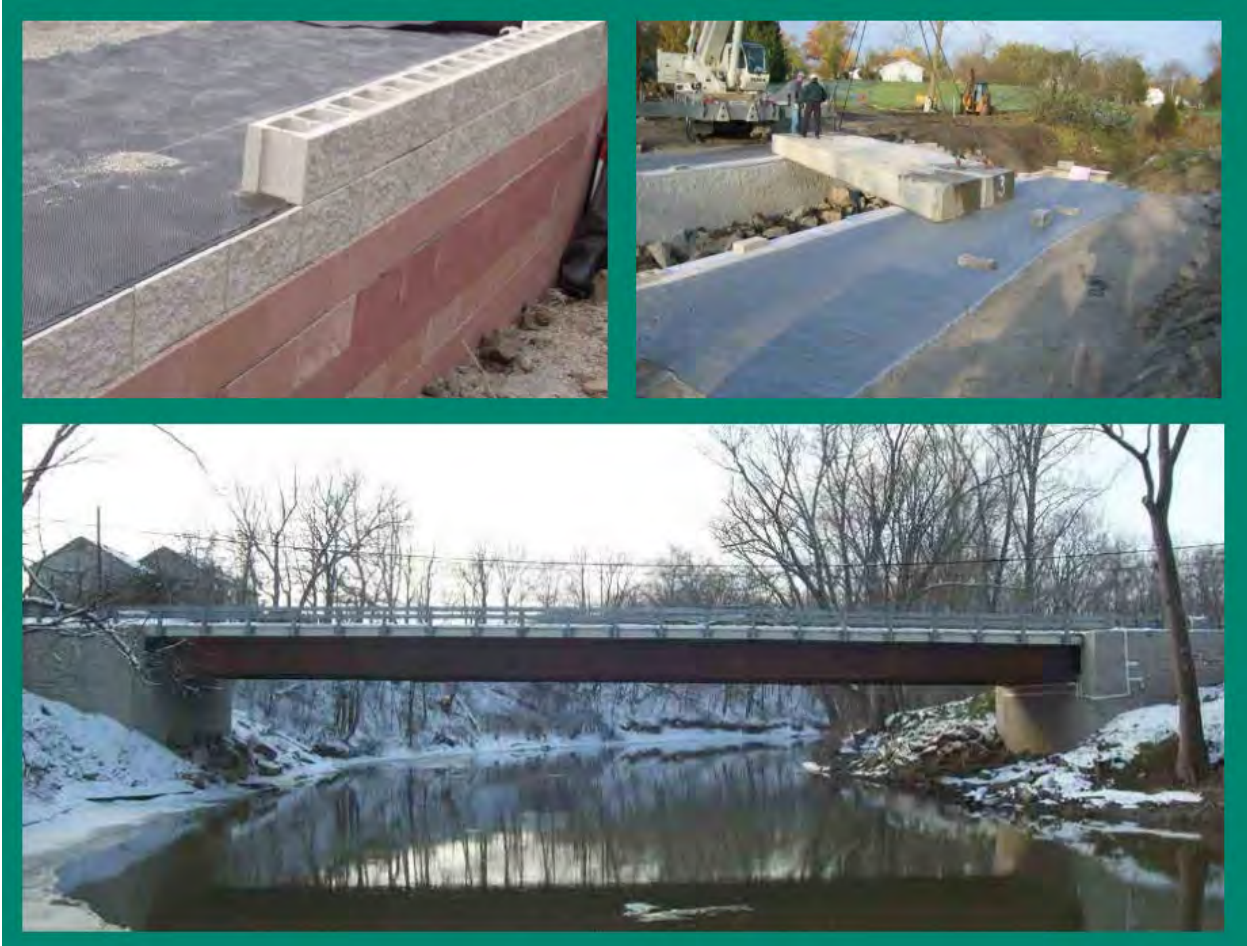
Fig. 1. Geosynthetics Abutments (Courtesy of FHWA (2018 ))
