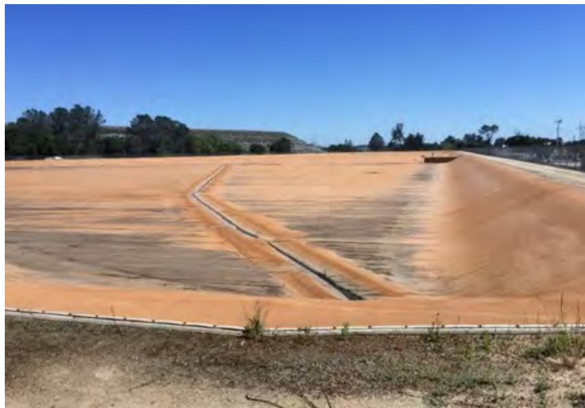
Figure 6. Hinkle Reservoir. 40-year-old cover installed in 1980
