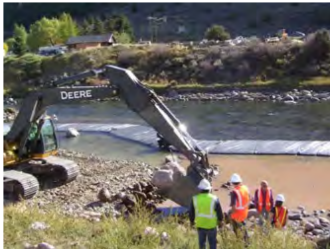
Figure 1. Installation of 6' Cofferdams – Eagle River, CO
