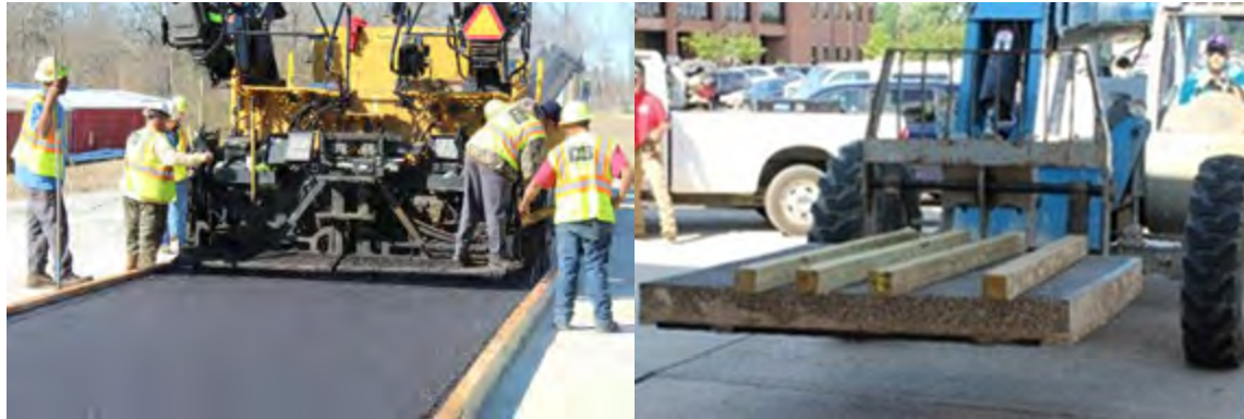
a) Paving HMA on a plywood base. b) Saw cut HMA slabs transported to box.
