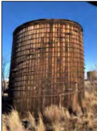
Figure 1. Wooden oil tank near Odessa, Texas. Source Ron MacKenzie
