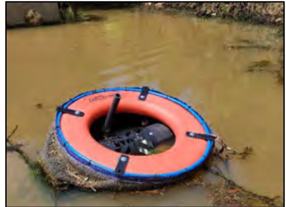
Figure 7. Skimmer in Basin with Siltron
