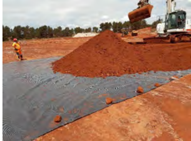
Figure 12. Continued placement of bottom ash soil over geosynthetic
