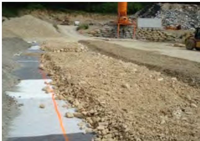
Figure 4. In-situ tests with several types of soil over the geosynthetic
