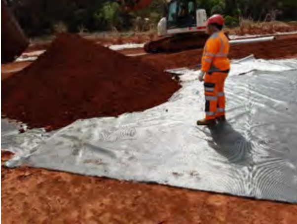
Figure 11. Placement of bottom ash soil over geosynthetic
