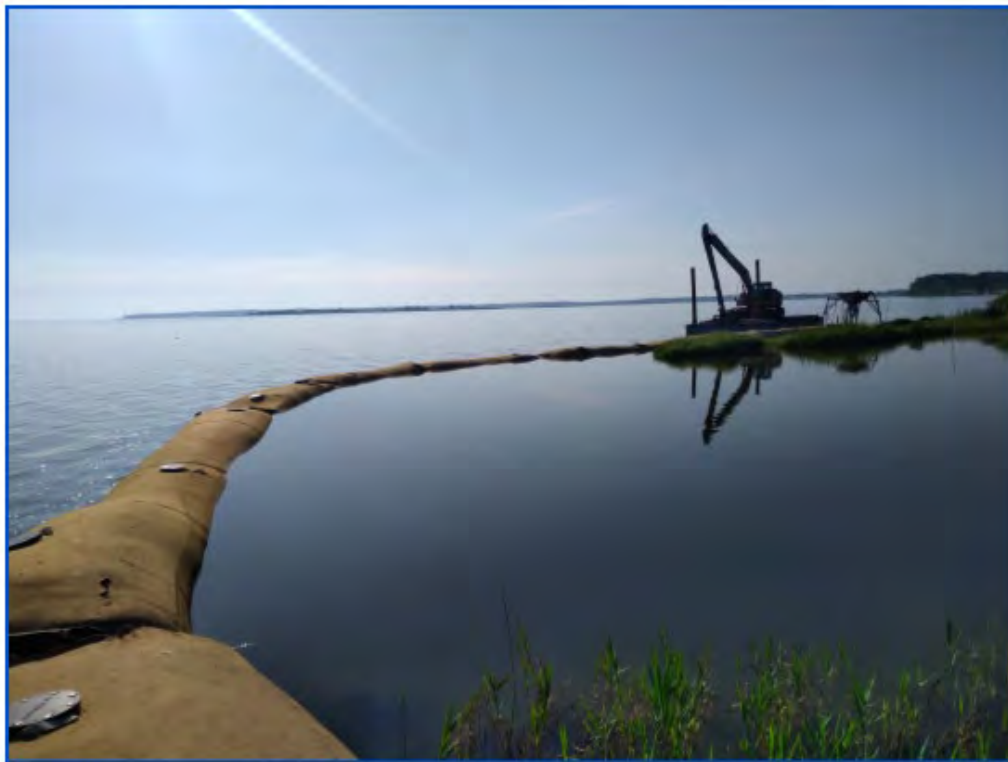
Figure 6 Installation of Geotextile Tube Perimeter Structure
