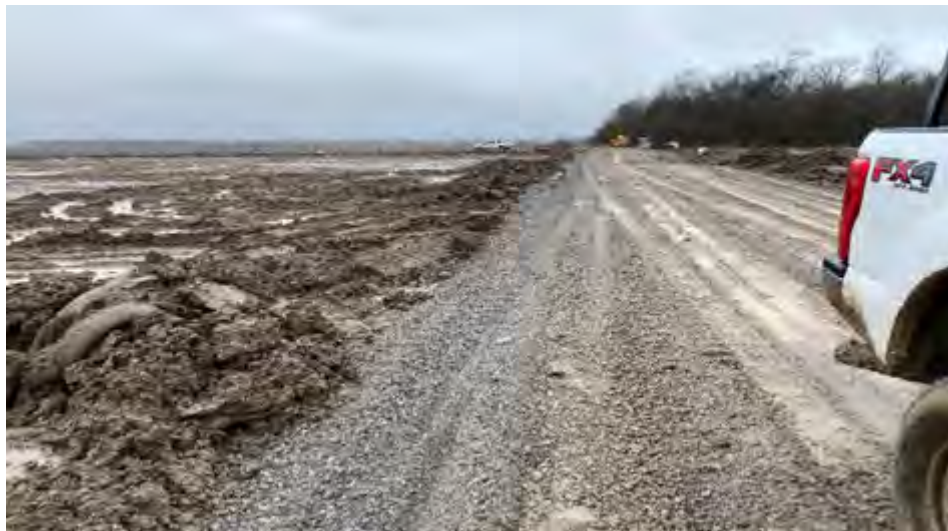
Figure 6. Stabilized Access Road with High-Strength Geotextile
