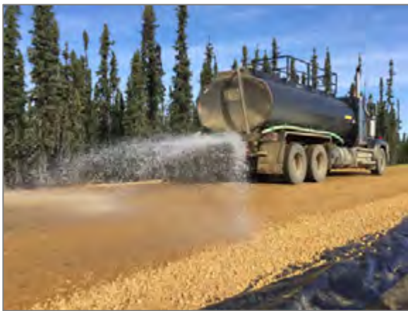
Figure 6. Top layer gravel fill placed in NPA geocell.
