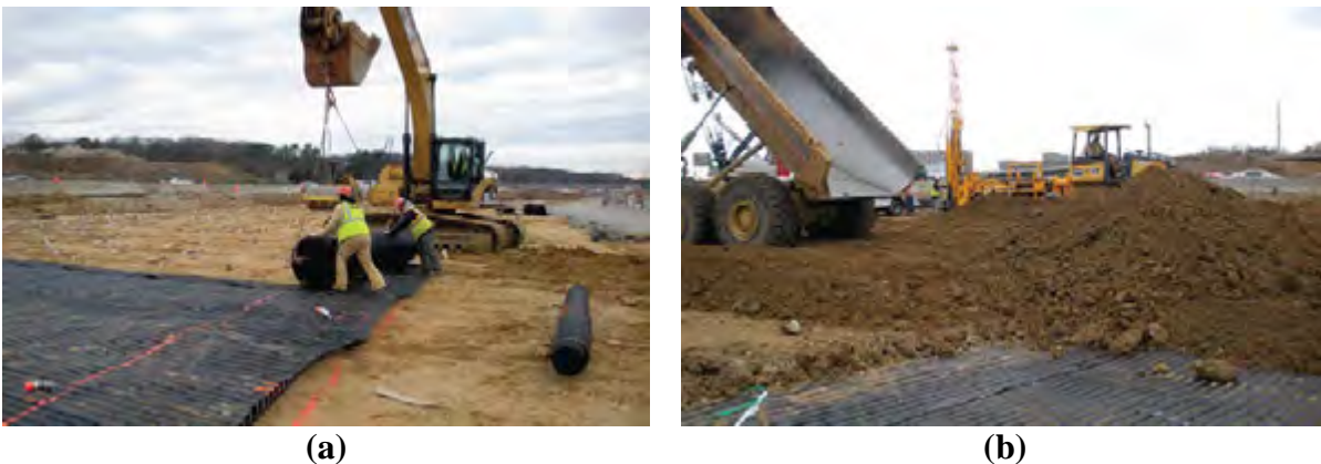
Figure 6. Geogrid installation (a) and laying down of fill material (b).
