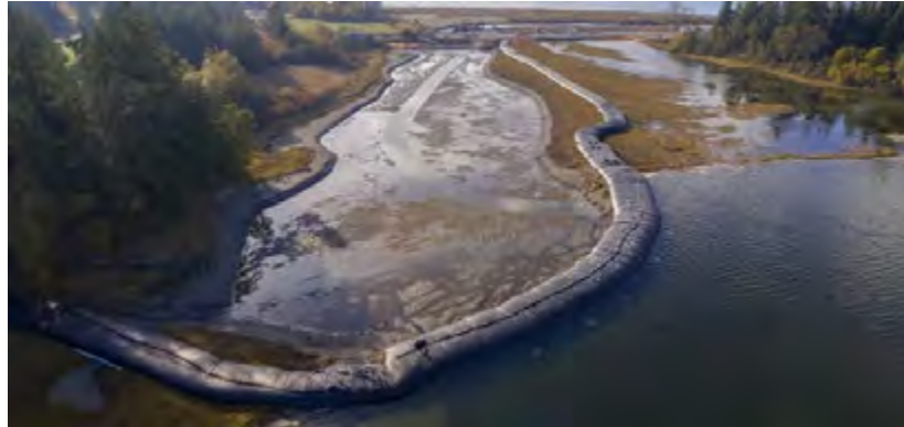
Figure 7. Kilisut Harbor Cofferdams
