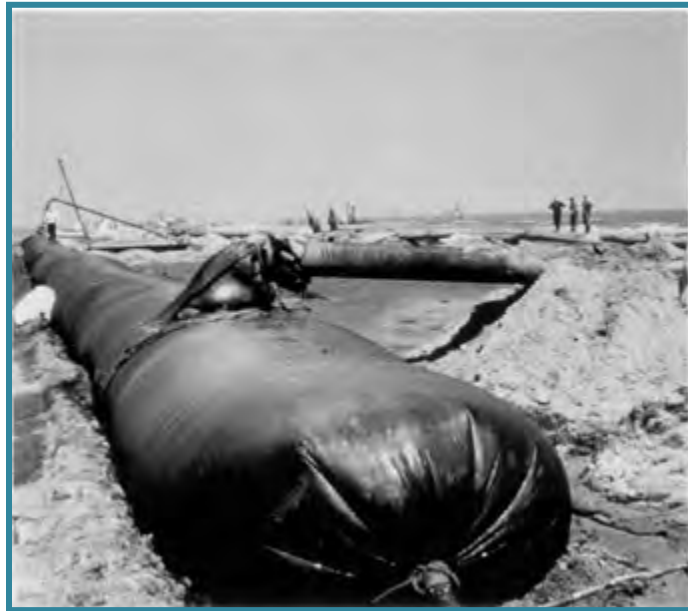
Figure 2: First job using the geotextile tube technology in 1962 (TenCate Geosynthetics)
