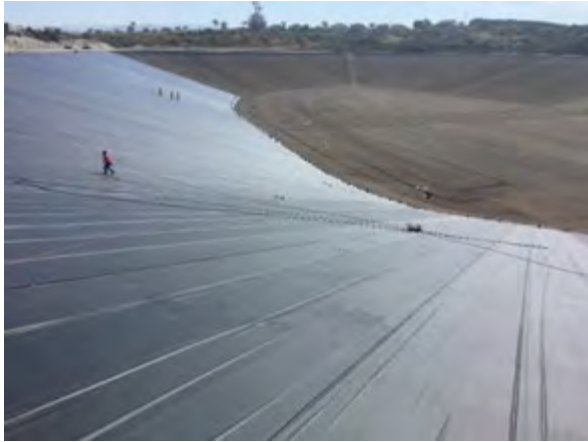
Figure 3. Chafer panel installation progress.
