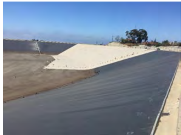
Figure 6. Floating cover fabricated panel deployment progress.
