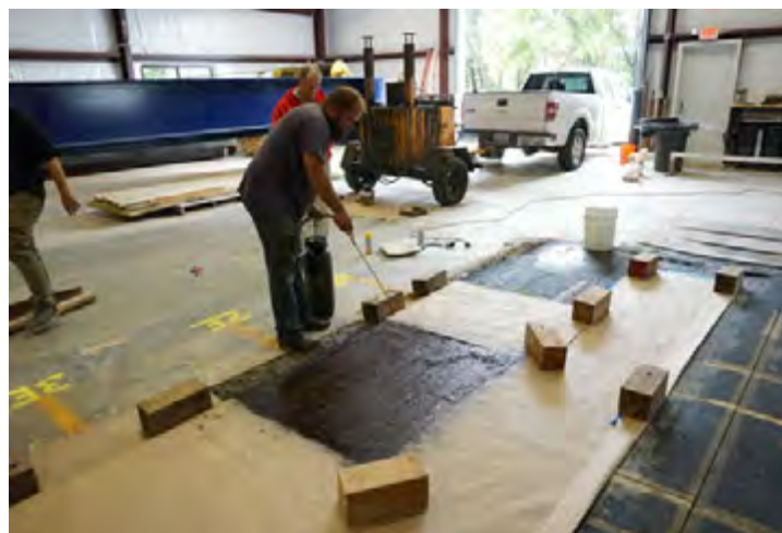
Figure 4: Application of asphalt emulsion onto pavement surface.
