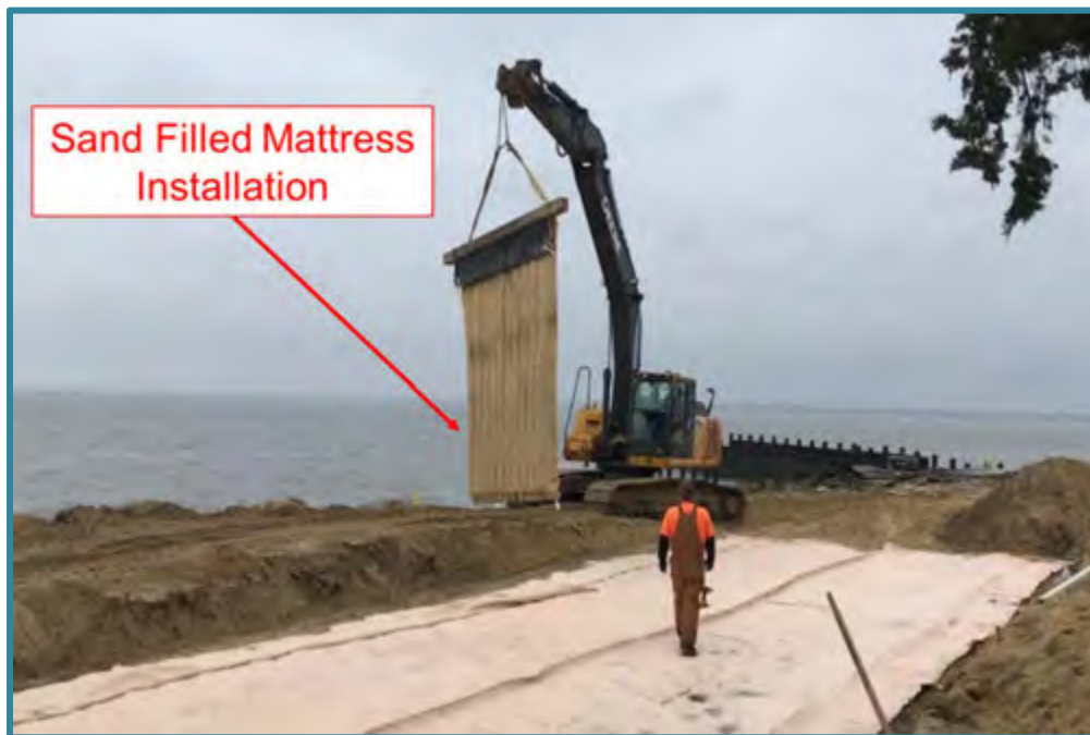
Figure 8: Sand Filled Mattress installation.
