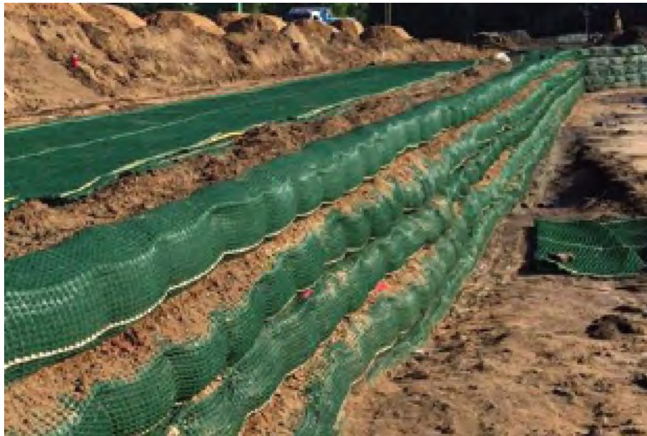
Figure 3. Partially completed GWFV wall at Edgewood MS.
