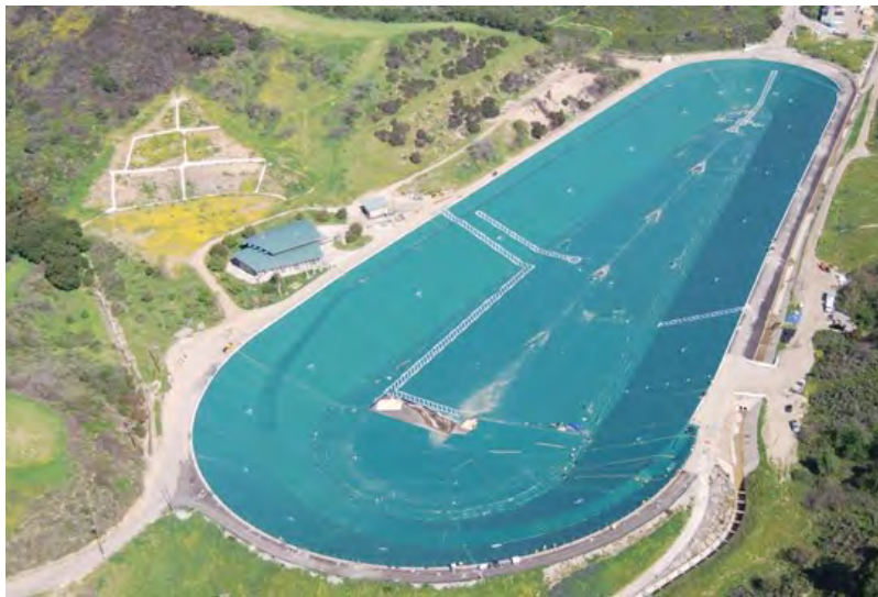
Figure 7. 45 mil CSPE Defined Sump Cover installed in 2019
