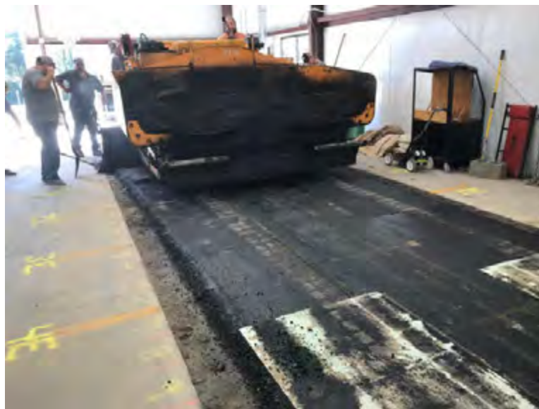
Figure 8: Asphalt overlay paving.
