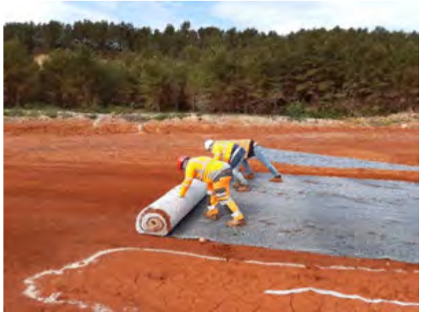
Figure 9. Continued installation of reinforcement geosynthetic
