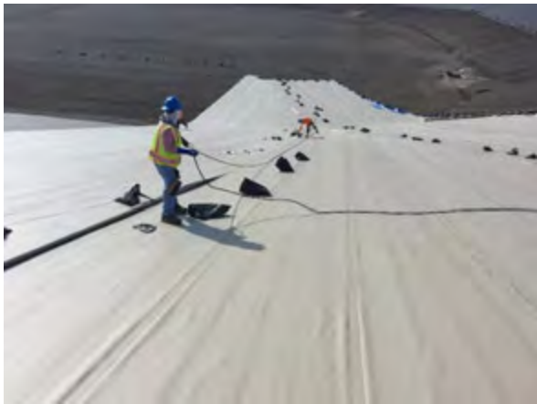
Figure 5. Floating cover panel seaming progress.
