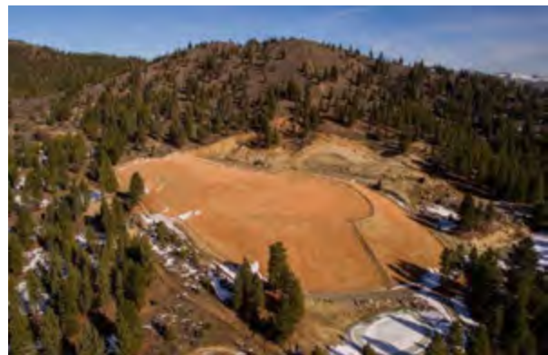
Portola Landfill, California (Tan Turf)
