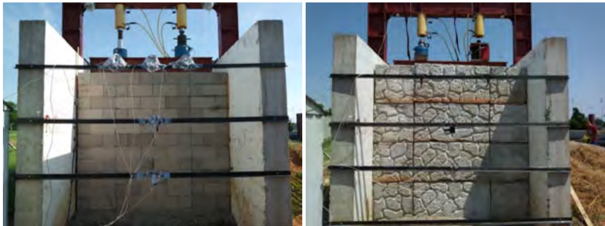
Figure 2. Elevation views of GRS abutment models #1 (left) and #2 (right) at end of construction (Doger 2020, Doger and Hatami 2020).
