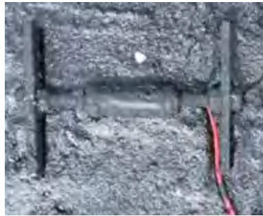
Figure 2. Typical asphalt strain gauge installed in the old asphalt.
