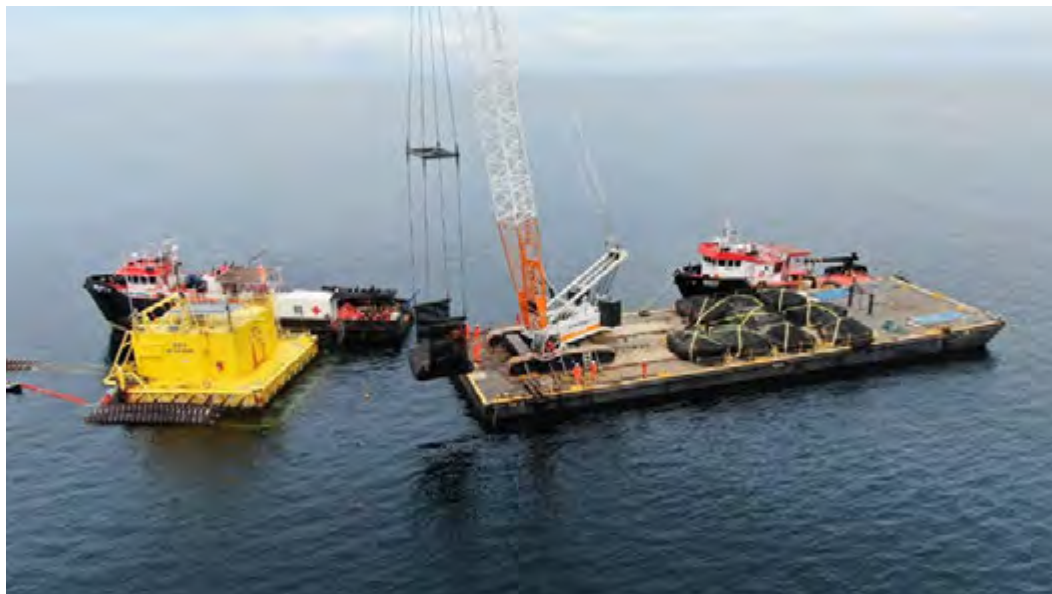
Figure 4 – Geotextile Bag Lifting Harness and Installation
