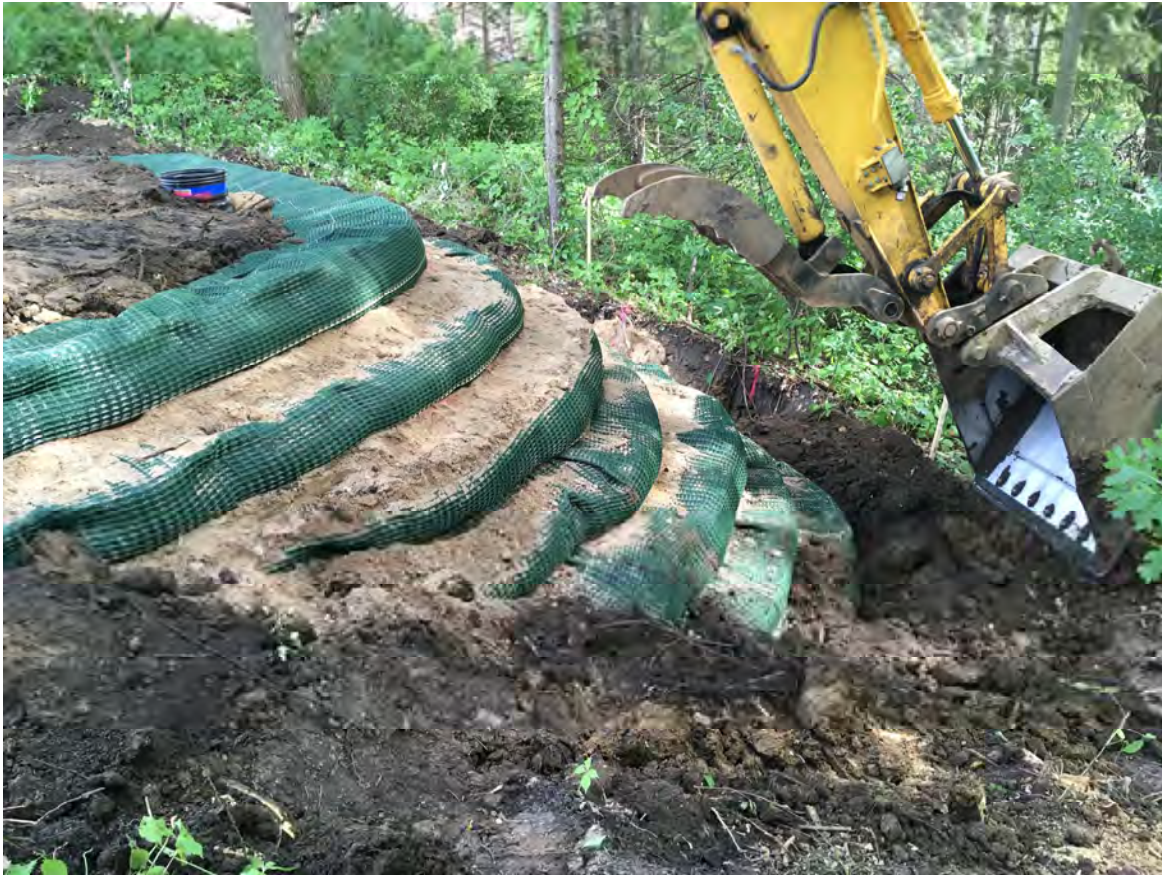
Figure 8. Partially completed reinforced soil slope at Mounds View HS project.
