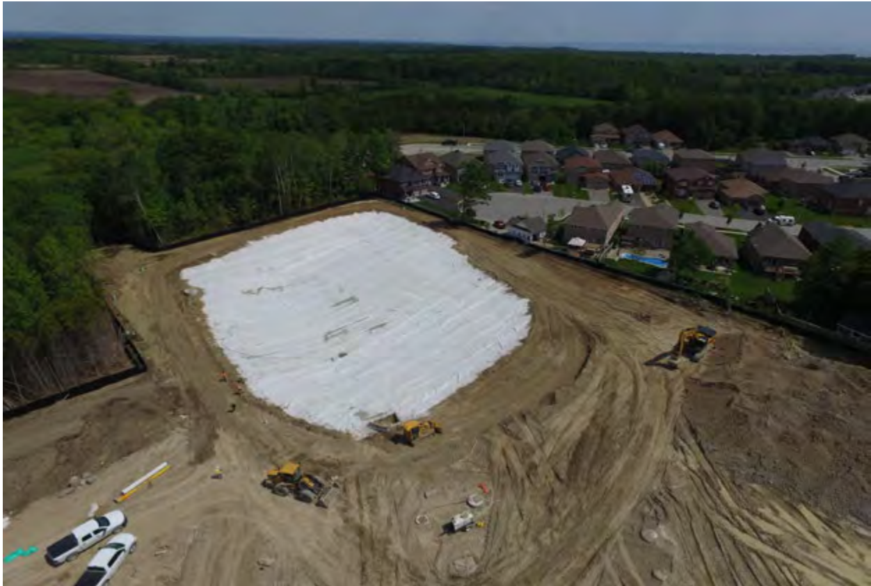
Figure 2. Scrim-Reinforced GCL left exposed for 3 days in a SWM Pond application.
