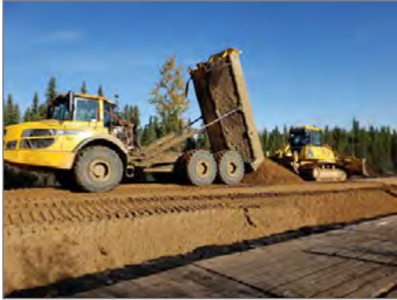
Figure 5. Temporary matted workspace (left) and compaction of fill material (right)
