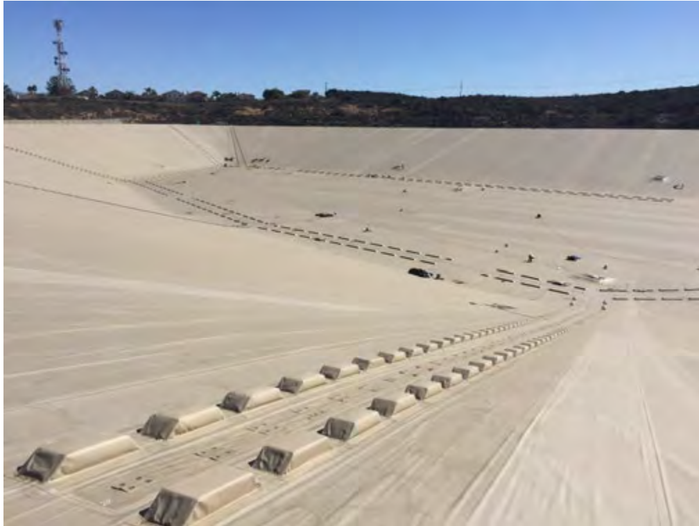
Figure 9. Floating cover system view with prefabricated appurtenances for the project.
