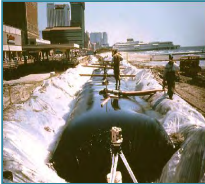
Figure 3: First geotextile tubes installed in the United States (Atlantic City, New Jersey in 1993).
