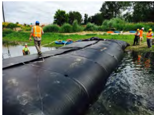
Figure 9. 8' Cofferdams being installed - Toppenish, WA
