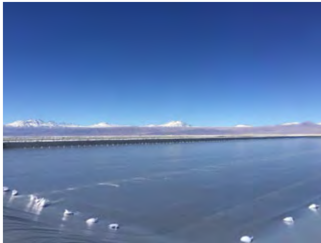
Photo 1. Open sky mining: typical view for a covered pond with PVC geomembrane
