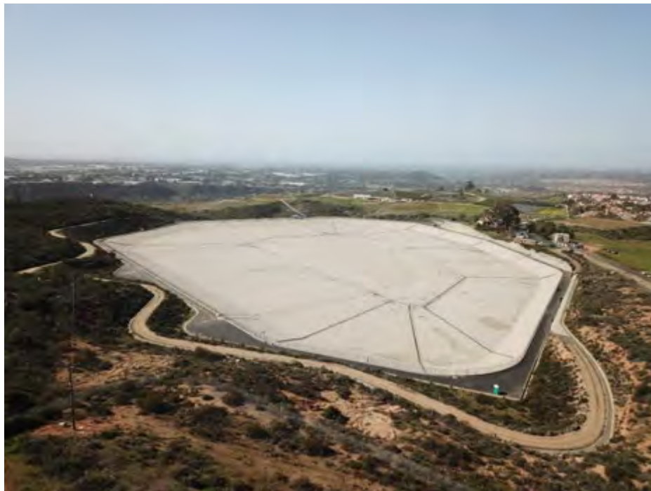
Figure 10. Aerial view of completed floating cover system with high aesthetic value.
