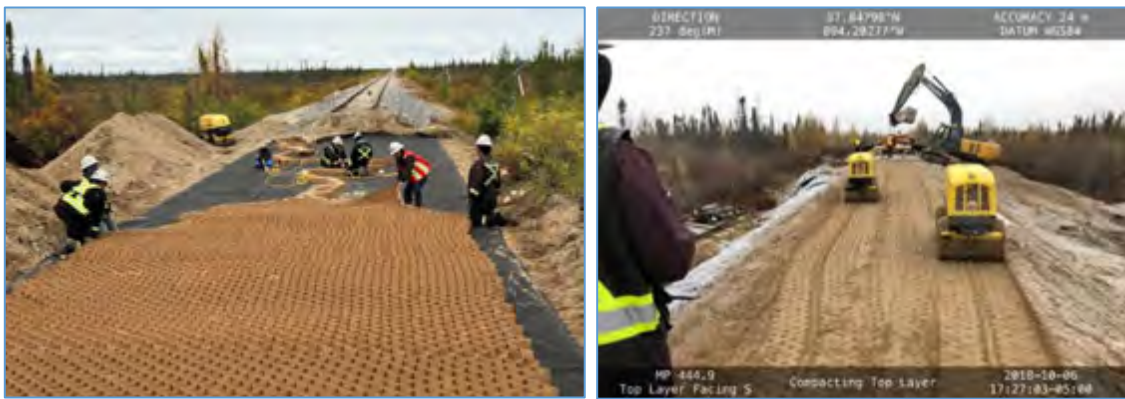
Figure 6. Geocell installation and compaction
