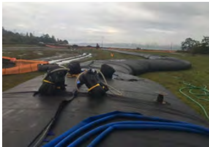
Figure 6. Kilisut Cofferdams being deployed in low tide
