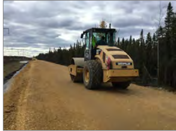
Figure 5. Temporary matted workspace (left) and compaction of fill material (right)
