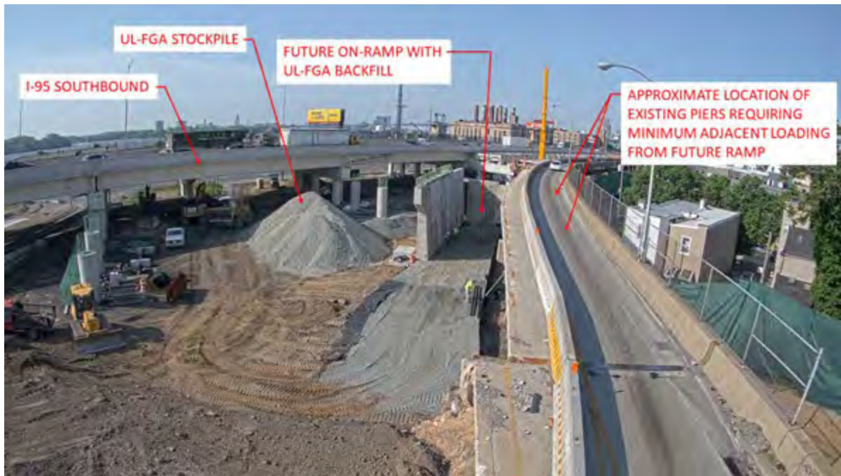
Figure 3. Photograph of the future on-ramp with UL-FGA MSE backfill.
