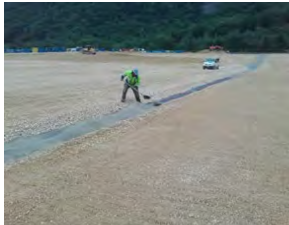
Figure 14. Backfilling of the gauges
