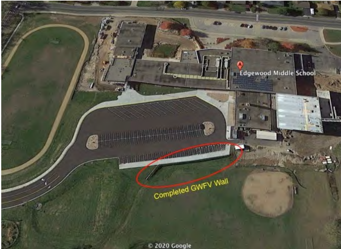
Figure 4. Edgewood MS construction site, showing completed engineered vegetated wall system in October of 2019 (looking west); courtesy of Google Earth.
