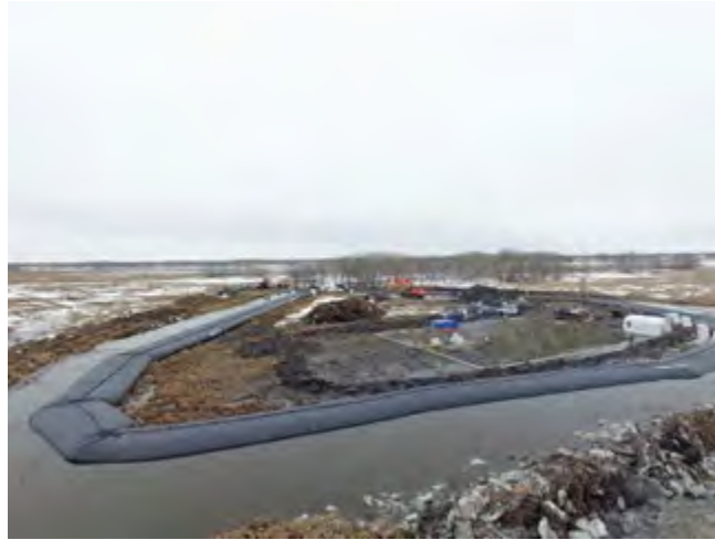
Figure 3. 6' Geosynthetic cofferdams for pipeline repair in Manitoba, Canada
