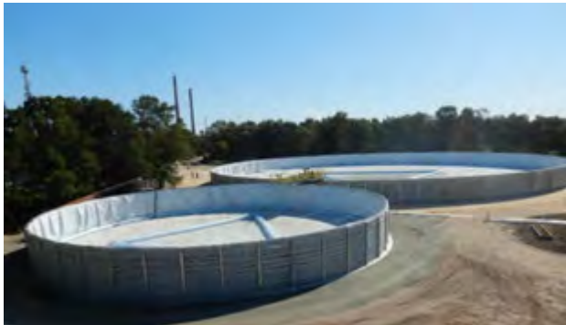
Figure 5. Tanks at handover.
