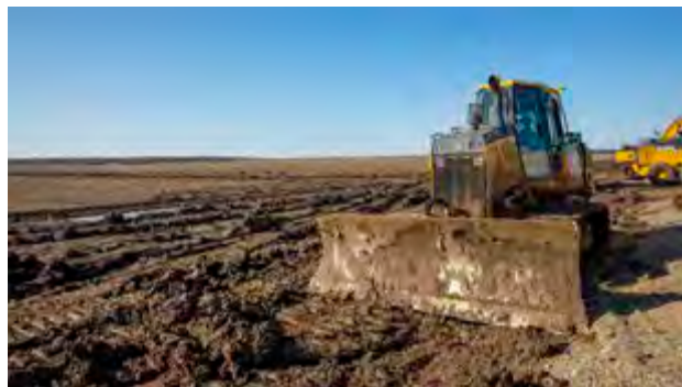
Figure 5. Site at Chicot Energy Center (pre-construction) (Segrave, 2019)
