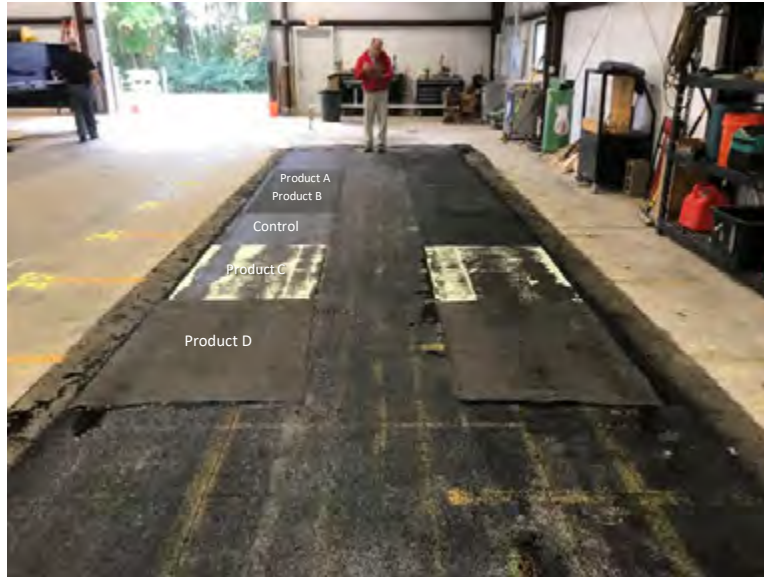
Figure 7: Installed interlayer materials prior to asphalt overlay.
