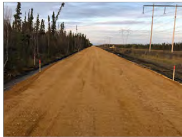
Figure 6. Top layer gravel fill placed in NPA geocell.
