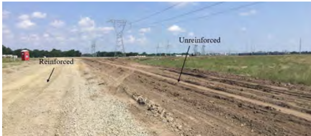
Figure 10. Reinforced Access Road vs. Unreinforced Conditions
