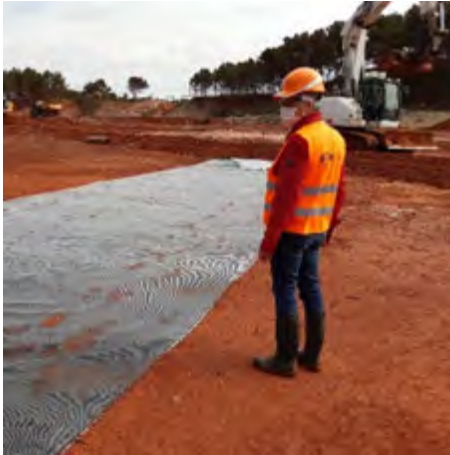
Figure 8. Installation of reinforcement geosynthetic
