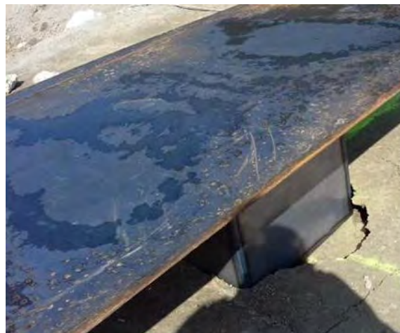
Figure 8. Steel plates on the steel cube
