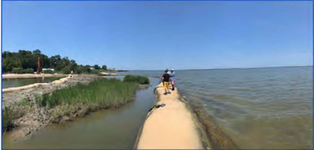
Figure 7 Dredging Fill In-between Geotextile Structure
