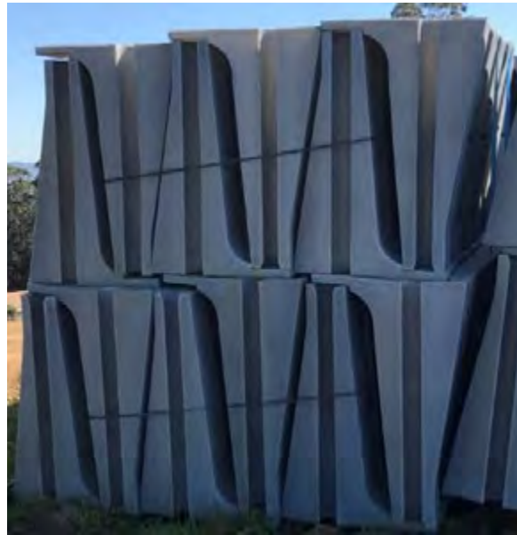
Figure 2. Stacked barrier walls.
