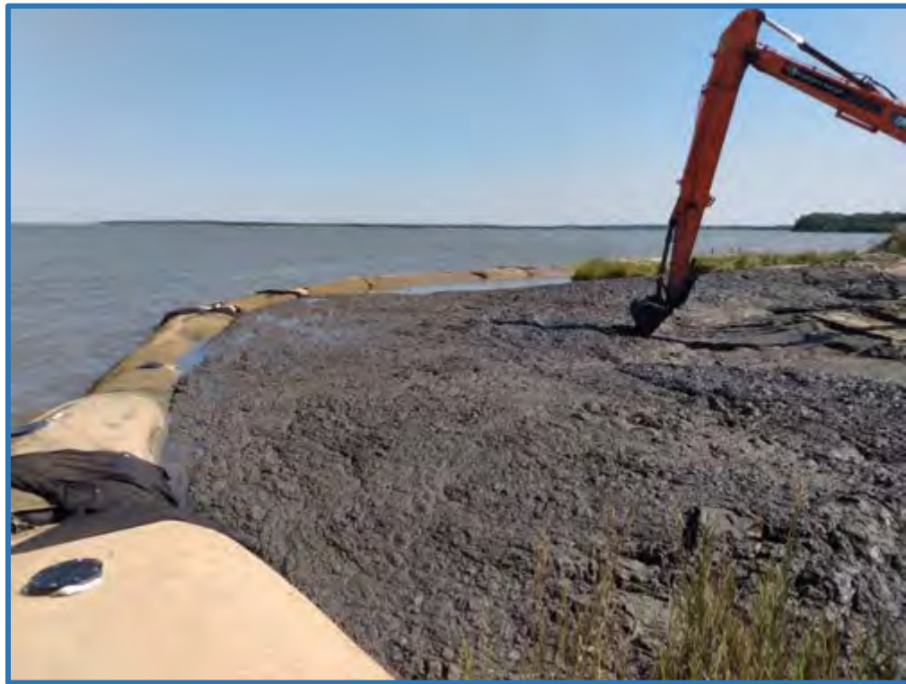
Figure 8 Dredging Backfill
