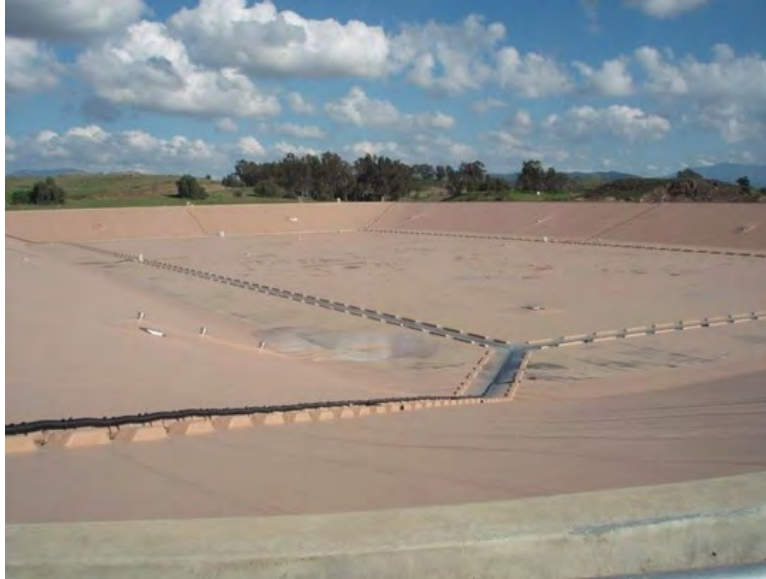
Figure 2. MWDS Skinner Reservoir. CSPE Defined Sump 2013
