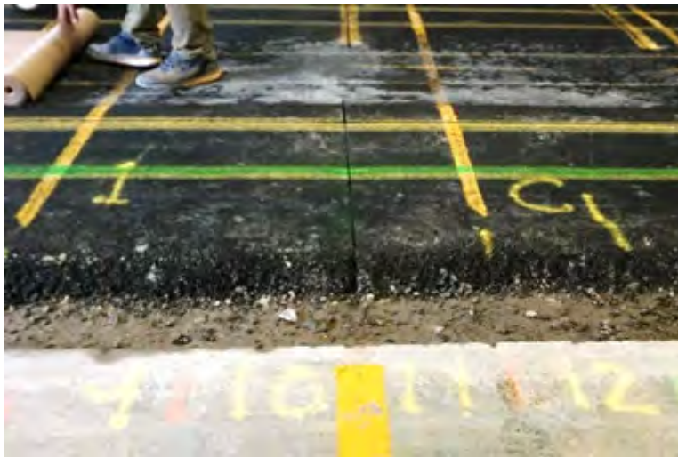
Figure 2: View of typical section with sawcut.
