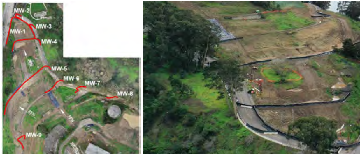
Figure 3. Aerial view (left) and side view (right) of the barrier wall basin locations.
