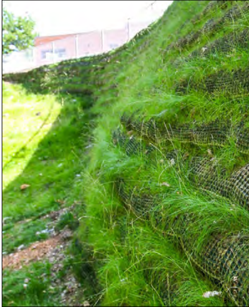
Figure 10. Vegetation coverage on face of the GWFV wall at Mounds View HS as of June 2020.
