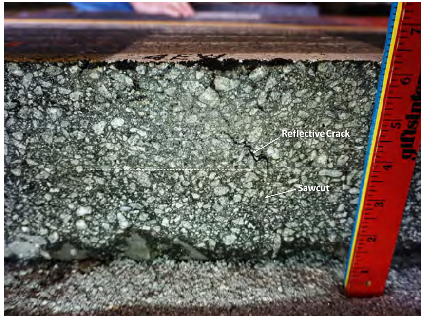
Figure 12: Profile view of Test Section 3, Control.
