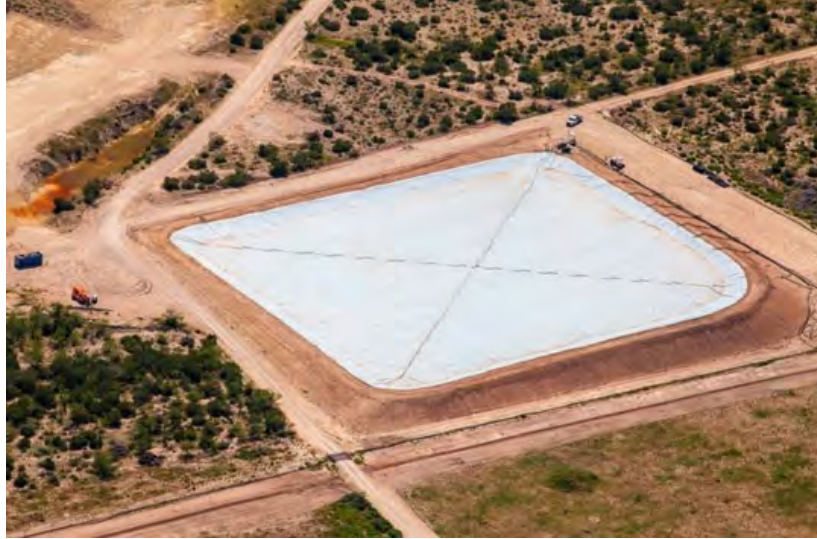
Figure 5. Evaporation Control Cover, Permian Basin, Texas in 2014
