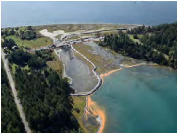
Figure 8. Aerial view of completed Kilisut Cofferdam installation
