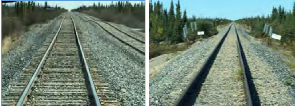
Figure 1. The condition of railway line in May 2016.
