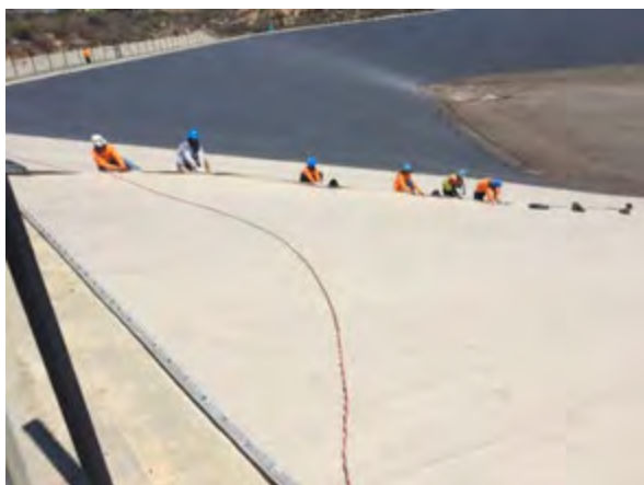
Figure 7. Positioning of the floating cover and wrinkle removal.
