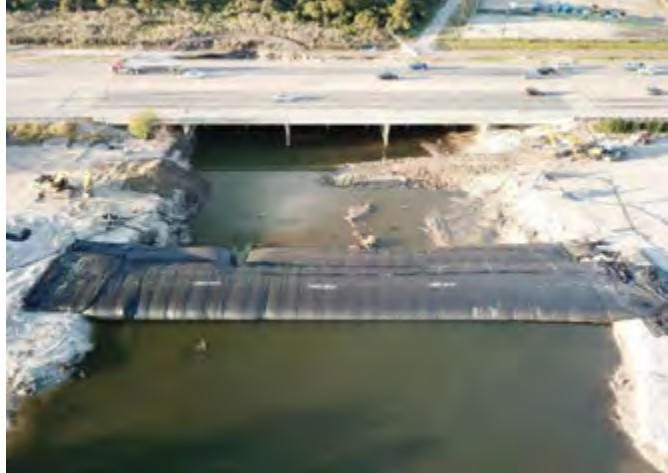
Figure 2. USACE 10' & 8' Cofferdam - Baytown, TX
