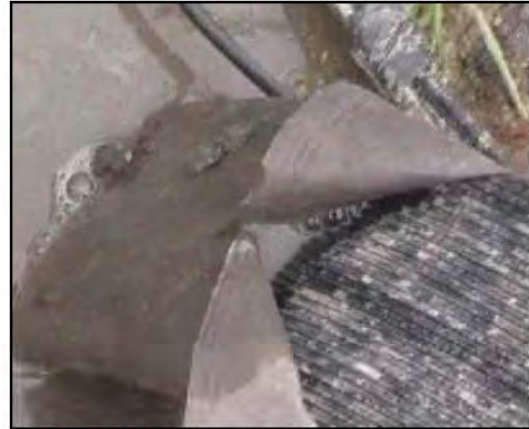
Figure 4: Discharge of ground water at EVD
