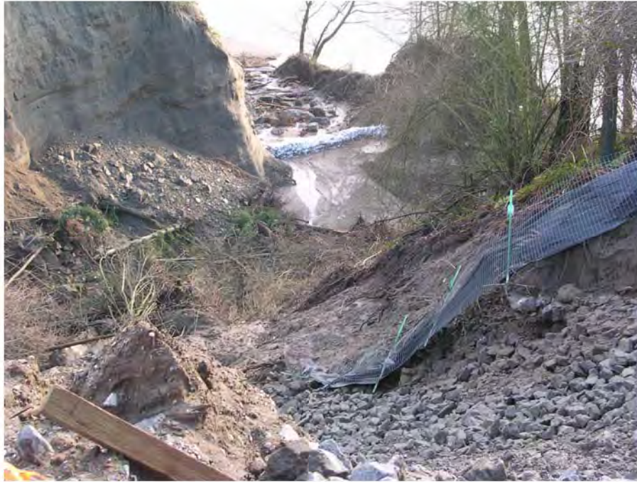
Figure 3: Ravine erosion, note sediment trap at ravine mouth. (used with permission of Shannon & Wilson)
