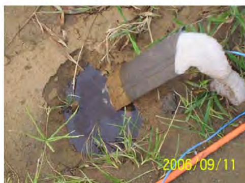
Figure 9: Discharge of groundwater from Cathode
