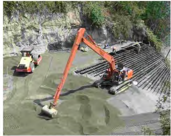
Figure 7: Geocell placement on steep slope with confined work area. (used with permission of Shannon & Wilson)
