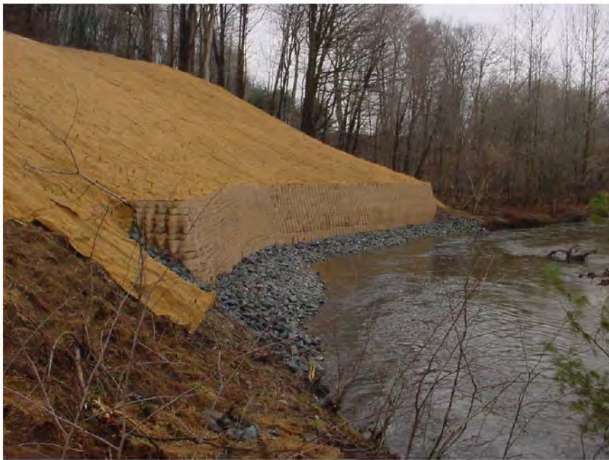
Figure 8 Completed Project at Sawmill River
