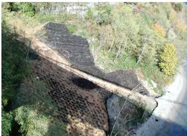
Figure 9: Completed 30 m high geocell slope. (used with permission Shannon & Wilson).
