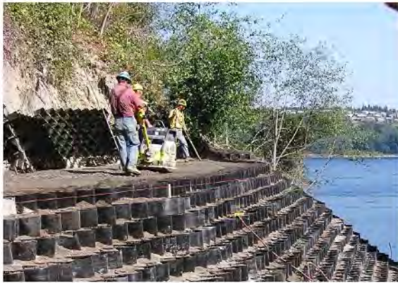
Figure 7: Geocell placement on steep slope with confined work area. (used with permission of Shannon & Wilson)
