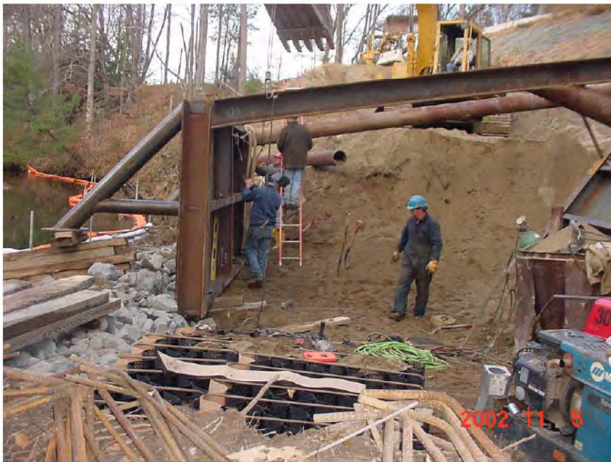
Figure 6 Temporary Shoring at Sawmill River
