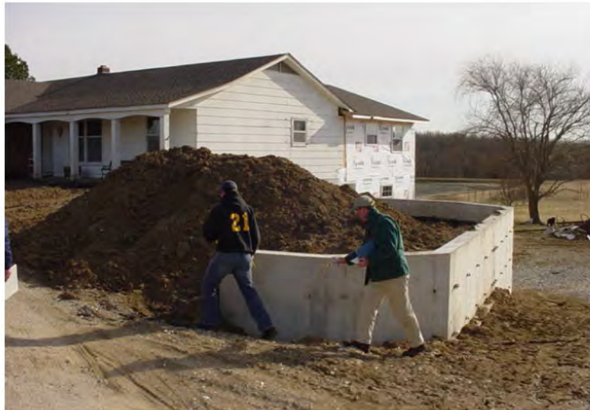
Figure 1 - Existing concrete retaining wall constructed October/November 2005 (February 2006)
