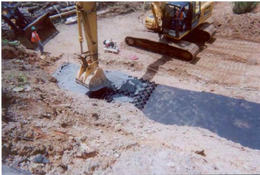
Figure 15 Granular Material for Geocell Infill
