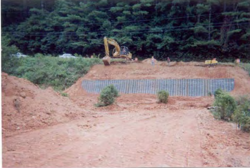
Figure 17 Rabun County EWP Site 3 Near Completion
