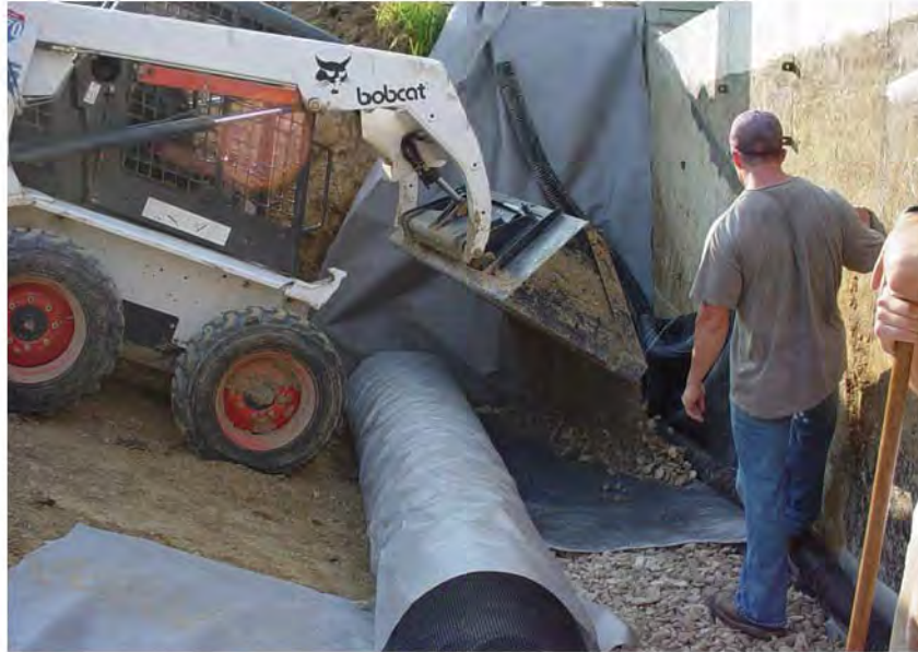
Figure 7 - Placement of 2nd layer with geotextile reinforcement and gravel backfill (July 17, 2006)
