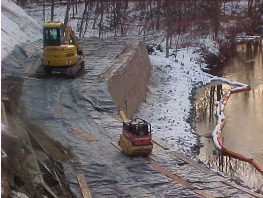
Figure 7 Finishing Geocell wall at Sawmill River
