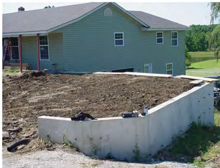
Figure 10 - Grading of finished geotextile wrap-face wall (July 24, 2006)
