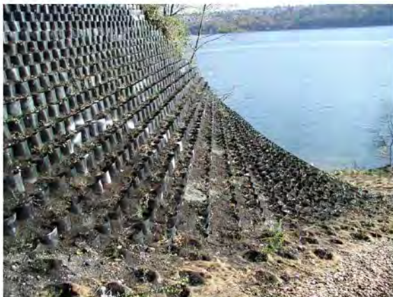
Figure 8: Completed slopes. Note variable spacing of geocell panels to match existing slope (left) and geocells placed between existing trees (right). TRM slope protection and plantings on flatter terrain (right). (used with permission Shannon & Wilson)
