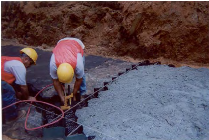
Figure 16 Attaching adjacent section of Geocell
