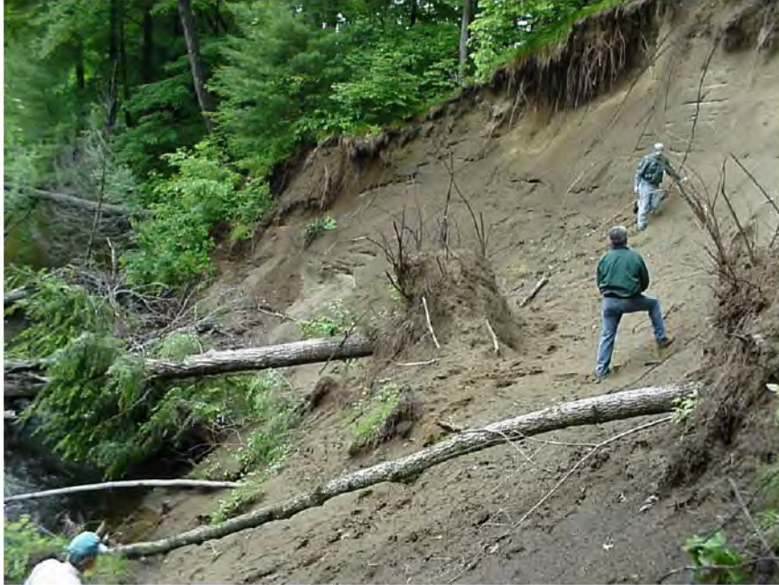
Figure 1 Sawmill River Bank Failure
