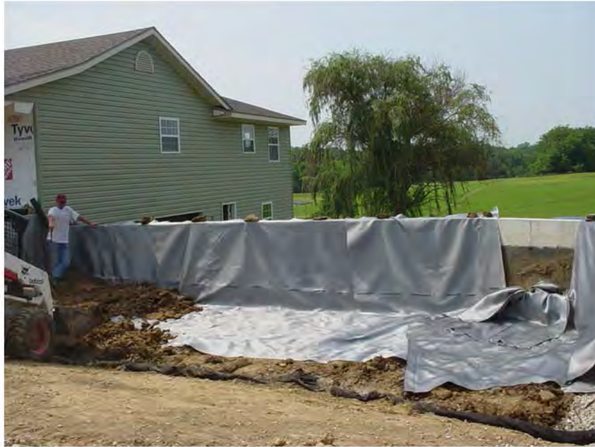
Figure 8 - Installation of CL backfill on geotextile reinforcement - 5th lift (July 19, 2006)
