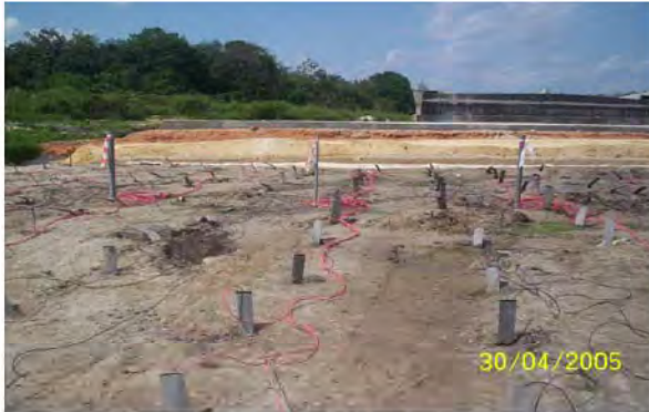
Figure 3: Setup at site
