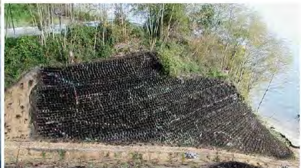
Figure 9: Completed 30 m high geocell slope. (used with permission Shannon & Wilson).
