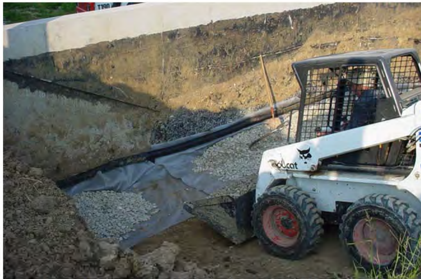
Figure 6- Placement of the gravel leveling pad (July 17, 2006)
