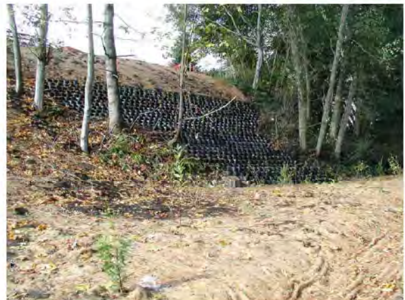
Figure 8: Completed slopes. Note variable spacing of geocell panels to match existing slope (left) and geocells placed between existing trees (right). TRM slope protection and plantings on flatter terrain (right). (used with permission Shannon & Wilson)
