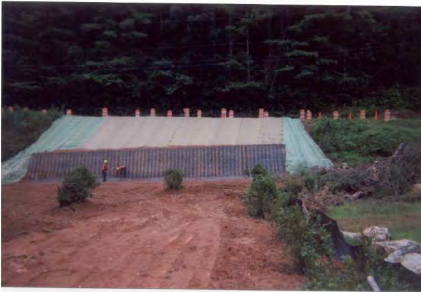
Figure 18 Rabun County EWP Site 3 Completed
