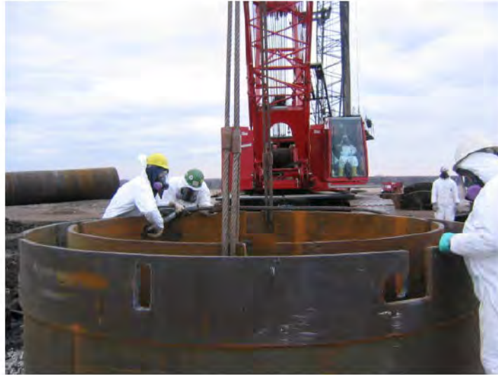
Figure 9. – Shaft excavation at Cleanout D-14
