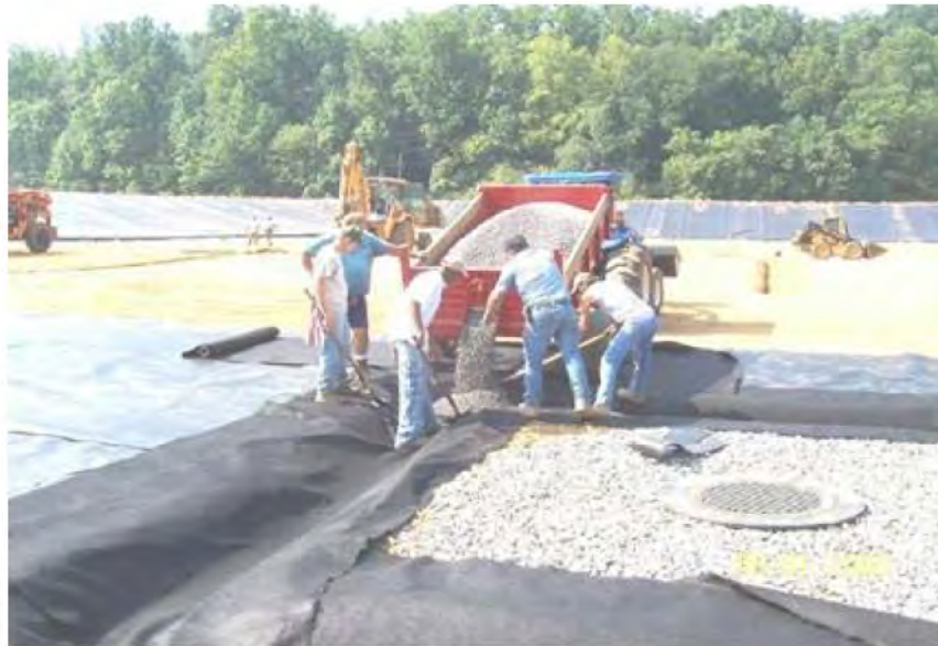
Figure 4 Anchor Trench Construction
