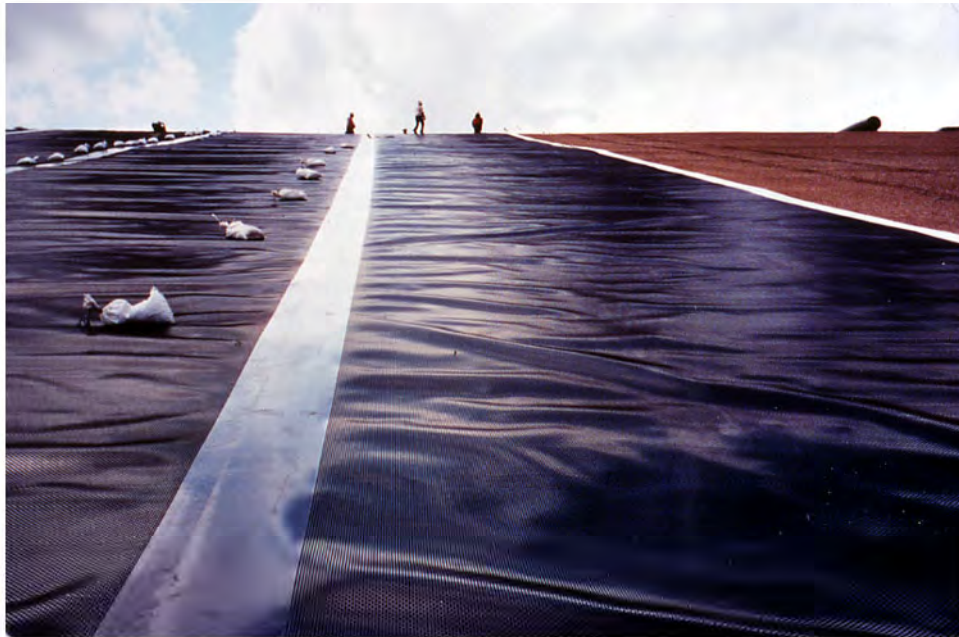
Figure 7. Structured Drain Profile on a Slope Prior to Geotextile/Cover Soils Placement
