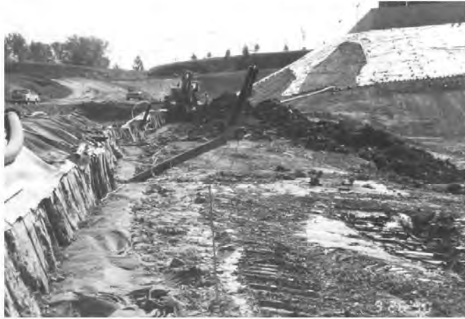
Figure 5. – A-North riser at tie-in to sub-cell D
