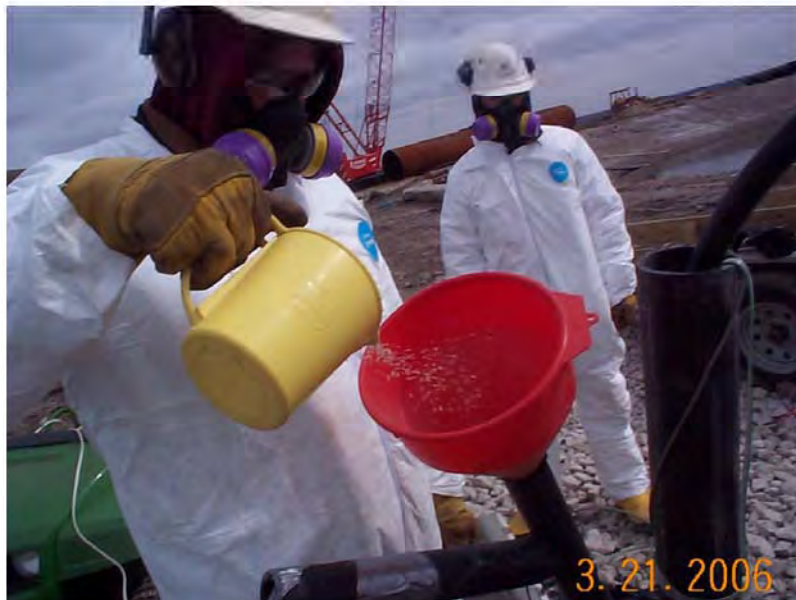
Figure 11. –Filter sand placement in Riser B
